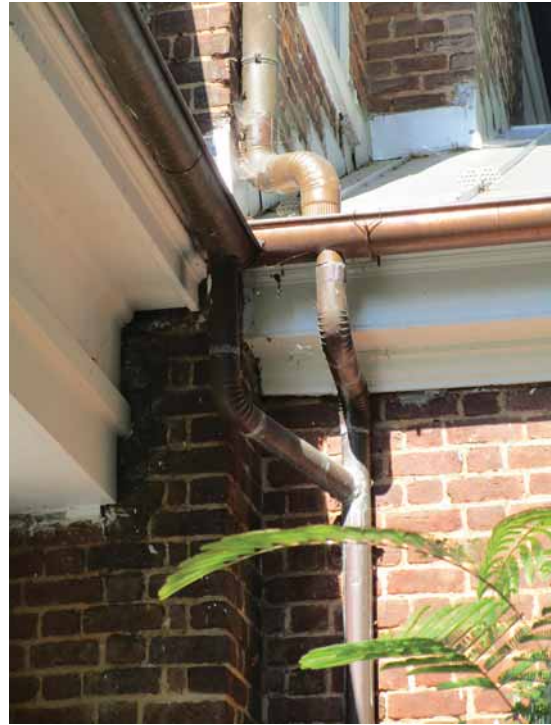
Figure 260. Many of the gutter downspouts on the house follow a circuitous route to the ground. In this location, north of the east porch, three gutters drain into one downspout. JGWA, 2024.
