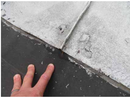
Figure 257. (Above) The standing-seam sheet-metal roofs of the north and south wings are of different ages and conditions. The roof on the south wing has several coats of aluminized roof coating. Some of this has chipped, and some areas of rust staining exist. JGWA, 2024.
