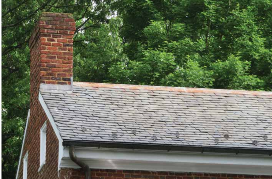
Figure 255. Slate shingles cover the central section of the roof, which shows signs of its age through missing, broken, and displaced slate. Regular maintenance has countered some of the age-related deterioration. JGWA, 2024.
