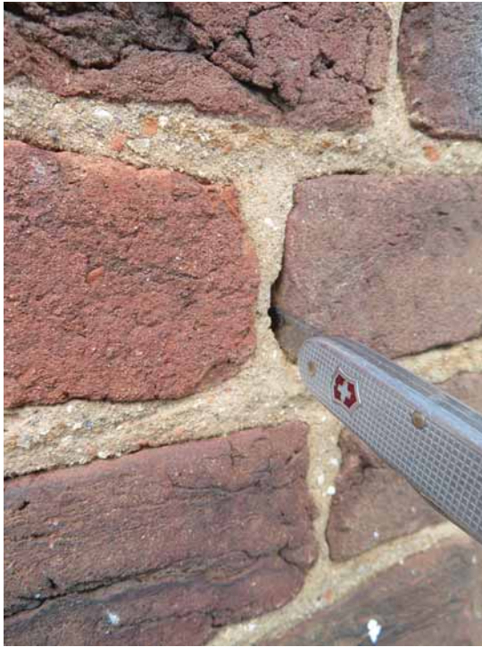
Figure 263. (Left) Head joints, the vertical joints at the small ends of individual bricks, are often not filled as well as the bed joints below each brick during construction. When the surface joint in these locations fails, a void often exists behind the surface. JGWA, 2024.
