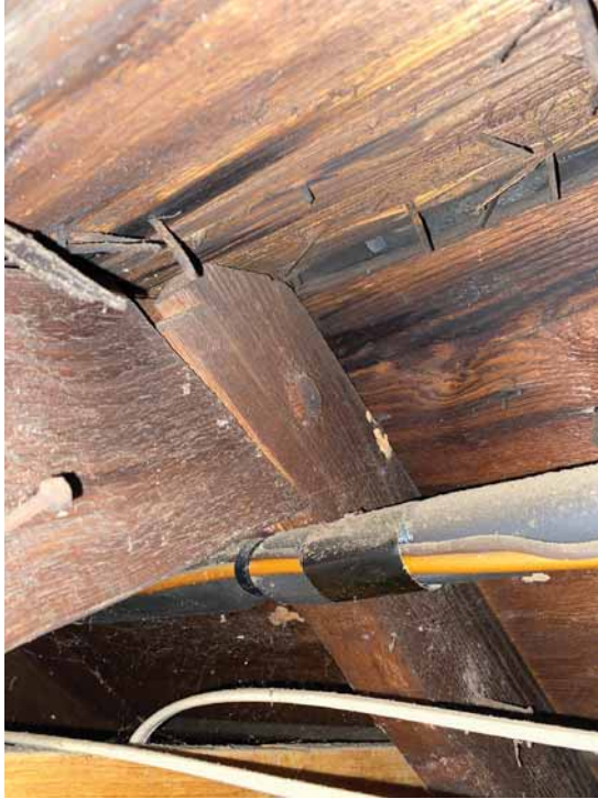
Figure 251. (Left) The rafters meet at mortise-and-tenon joints at the peak of the gable. JGWA, 2024.
