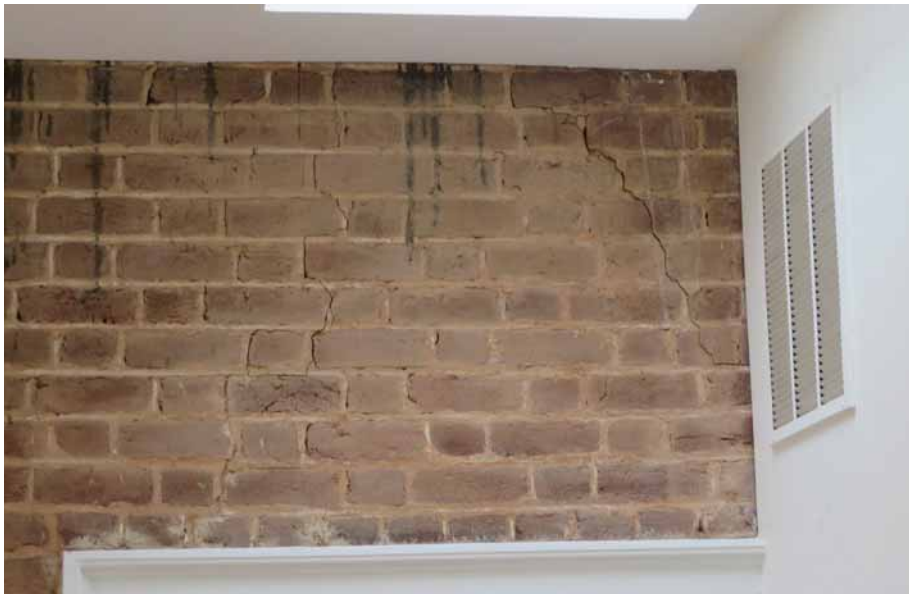
Figure 278. Settlement cracks can be seen in the well-preserved exposed brickwork above two of the doorways in the southwest addition (109). In the image, one of the cracks is over the doorway to the west room (105). JGWA, 2024.
