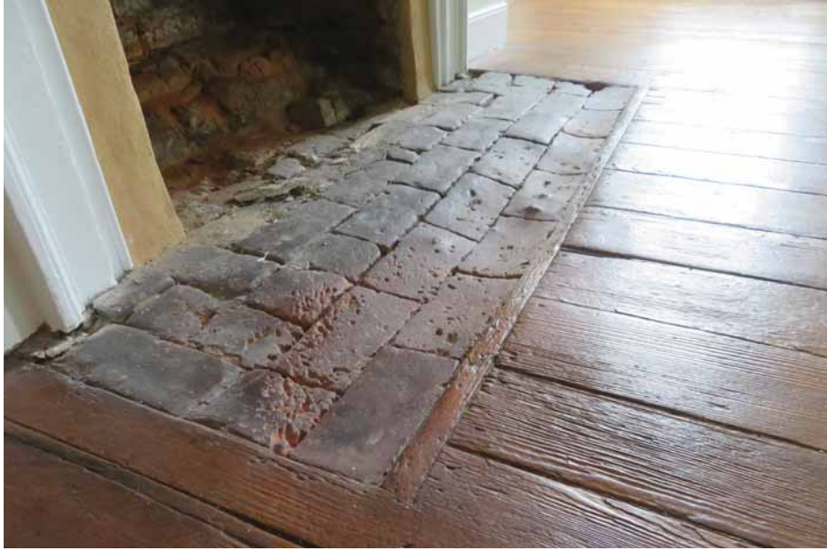
Figure 279. The brick thresholds of each fireplace are worn and the mortar joints eroded, but in the east bedroom (201) this condition is particularly severe. The wood flooring adjacent to the hearths is often similarly worn. JGWA, 2024.
