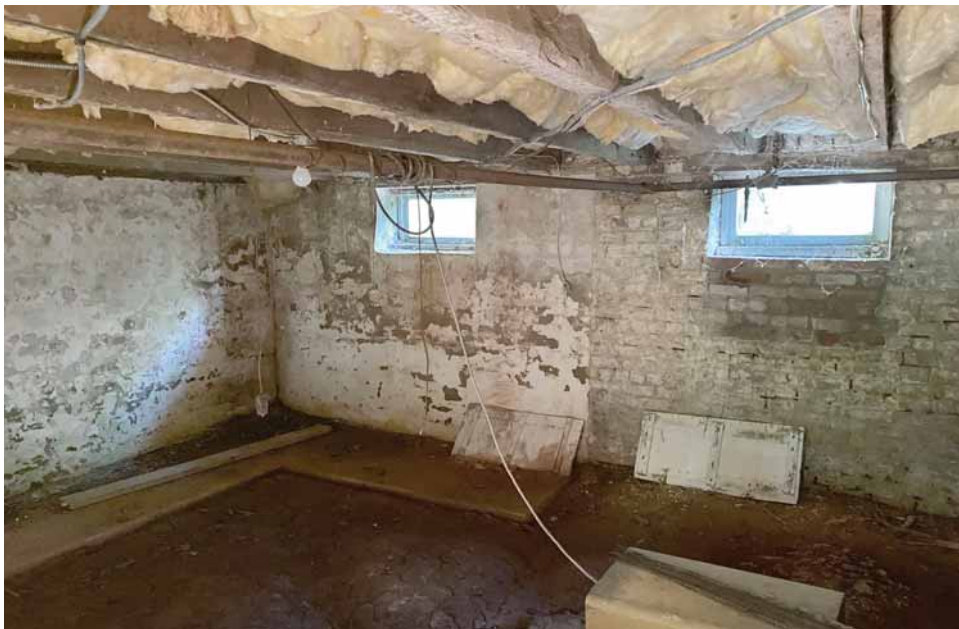
Figure 211. The north basement (002), looking south (upper image) towards the arched support for the fireplace above; and northeast (lower image). Note the brick infill below the windows, indicating their original size. JGWA, 2024.
