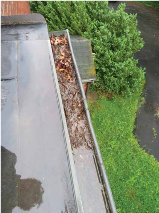
Figure 259. Clogged or nearly clogged gutters exist at all sides of the building. The sheet-metal gutter to the left of this image is intended to prevent water from running down the brick wall below; however there is water damage on the brick below. The asphalt roof on the entrance to the south basement is nearing the end of its service life. JGWA, 2024.
