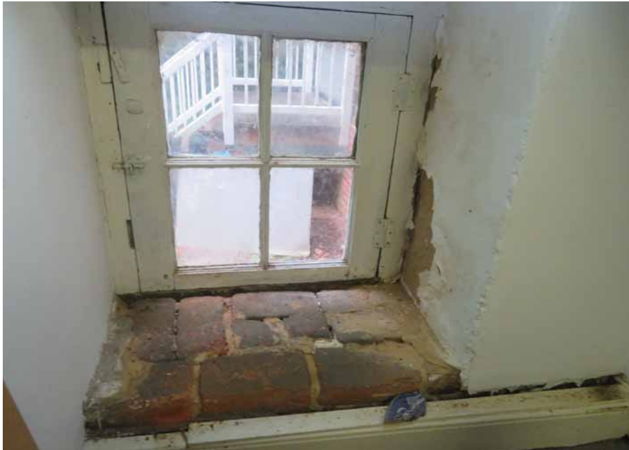
Figure 277. The plaster failure on the east side of the small window in the storage room under the stairs (106) is the result of moisture ingress. In this location, overflow from the roof has caused an area of staining on the exterior face of the wall and related damage on the interior. JGWA, 2024.
