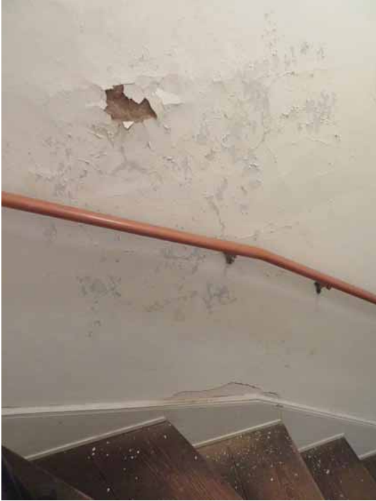
Figure 275. The north wall of the north stair (C101) is in extremely deteriorated condition. This is the result of moisture ingress from the exterior where the north wing and main blocks of the building meet and roof water runs down the face of the exterior wall. JGWA, 2024.
