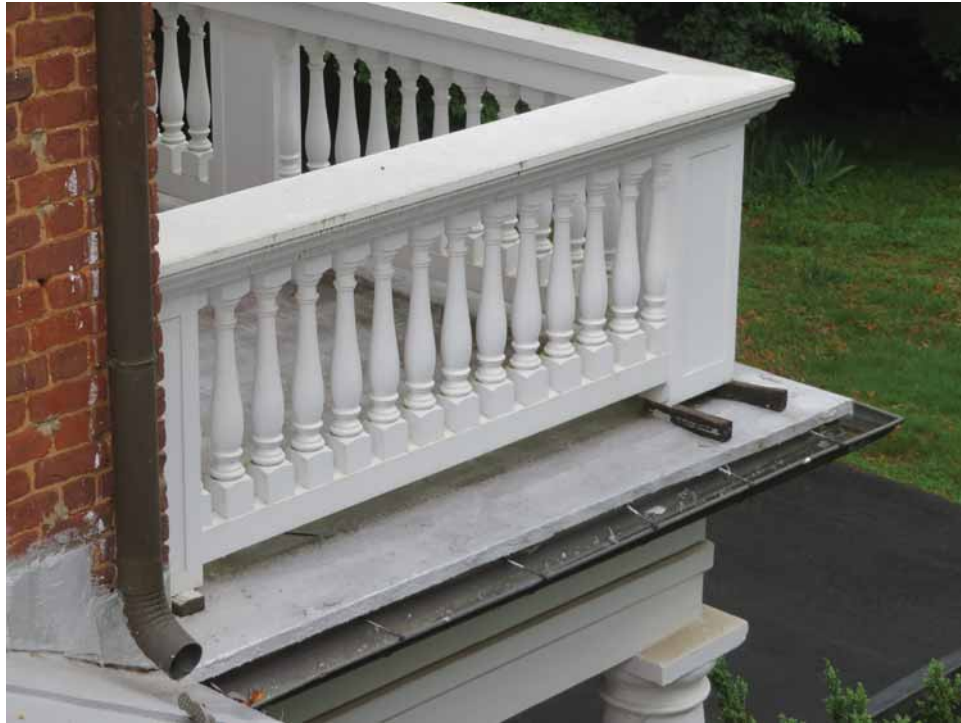
Figure 261. (Above) The rooftop balustrade on the east entrance porch was constructed in 1997–1998. Because it lacks a drip edge, there is surface staining and some biological growth on the painted surfaces below the cap rail. The plinths rest on exposed pressure-treated blocking. JGWA, 2024.
