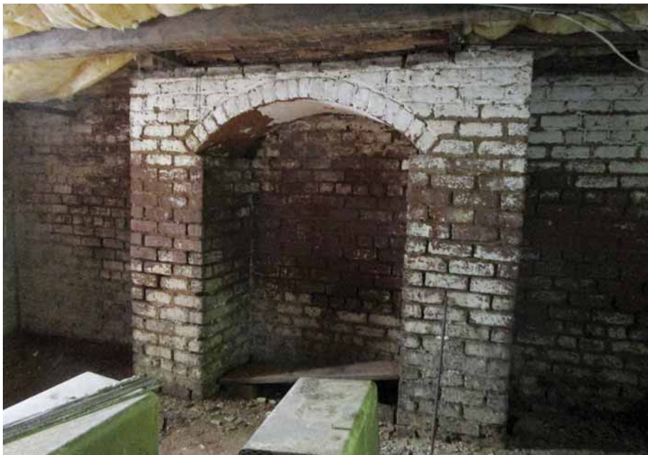
Figure 272. Evidence of rising damp can be seen across the midsection of the hearth support in Room 002 where the limewash has fallen away from the deteriorated face of the brick. There are also deteriorated mortar joints in this section of the wall. JGWA, 2024.
