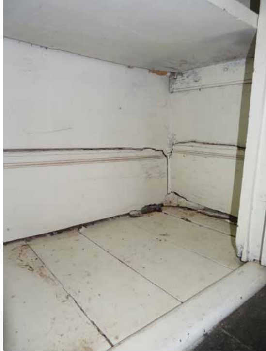
Figure 276. The floorboards under the built-in cupboard in the northwest corner of the west room (105) have dropped out of position, as has the baseboard above. This condition is a result of moisture-based deterioration adjacent to a failed roof leader. JGWA, 2024.
