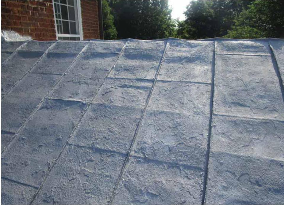
Figure 257. (Above) The standing-seam sheet-metal roofs of the north and south wings are of different ages and conditions. The roof on the south wing has several coats of aluminized roof coating. Some of this has chipped, and some areas of rust staining exist. JGWA, 2024.
