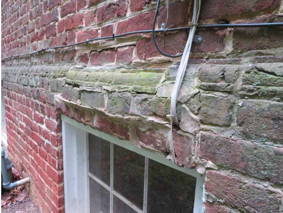
Figure 264. (Below) In many instances, there is displacement of the bricks where the molded brick water table passes over the basement windows. This condition is most advanced at the westernmost window on the north side of the main block of the house. JGWA, 2024.
