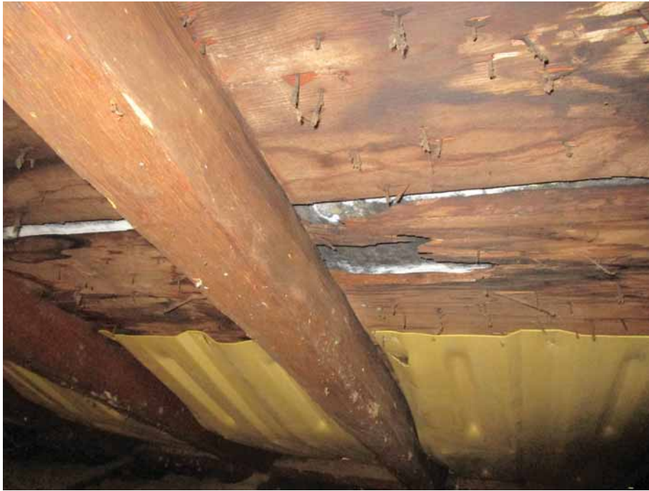
Figure 281. Rotted roof sheathing was left in place in some locations when the roof of the north wing was replaced. In other areas extensive repairs to framing and decking were undertaken. JGWA, 2024.
