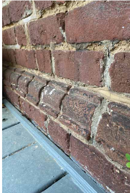
Figure 186. A molded brick course trims the top of the water table. JGWA, 2024.
