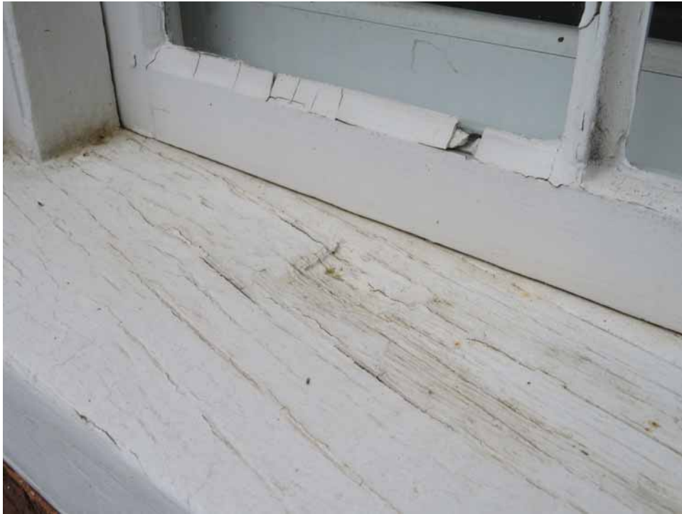
Figure 267. (Above) Failing glazing compound surrounding individual panes of glass and checked wood and cracked paint at the sills are common problems at the original windows. These problem conditions are most advanced where regular and rapid cycles of heating and cooling take place. JGWA, 2024.
