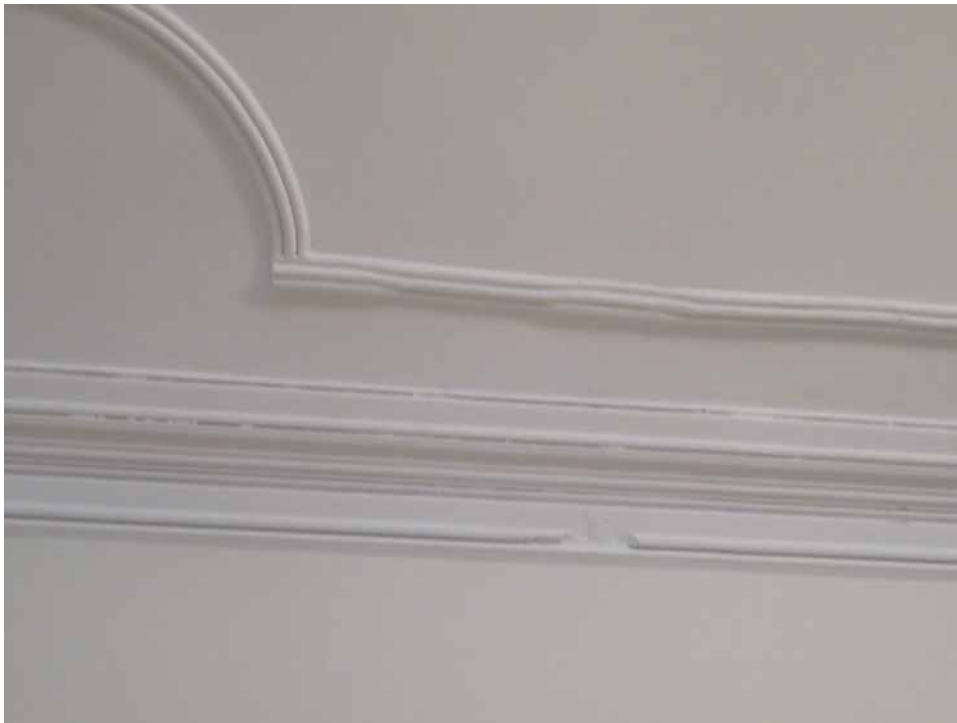
Figure 274. (Below) The plaster ceiling in the entrance hall (101) has been renewed and repaired on numerous occasions. Buildup of paint coatings has obscured some of the details and shadow lines. In some areas cracking of the plaster has resulted from movement and uneven support. JGWA, 2024.
