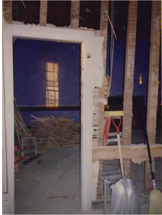
Figure 248. The second-floor bathroom (T206) during the 1997–1998 work, after the lath and plaster were removed. Courtesy of Nancy O'Brien.
