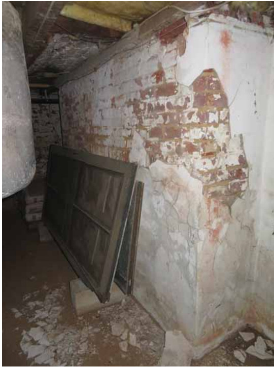
Figure 273. (Left) The cementitious render that was applied to much of the brick wall surface in the south basement (001) has fallen away in sheets where it has trapped rising moisture. In these locations, the brick is more damaged than in areas where only limewash was applied to the brick surfaces. JGWA, 2024.
