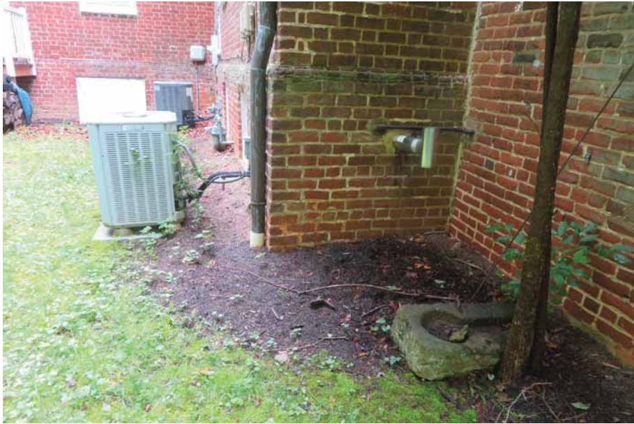
Figure 271. The north side of the central block of the house is a repository for numerous pieces of mechanical, electrical, and telecommunications equipment. It is also the exit point for the direct vent of Oak Lawn's boiler. JGWA, 2024.
