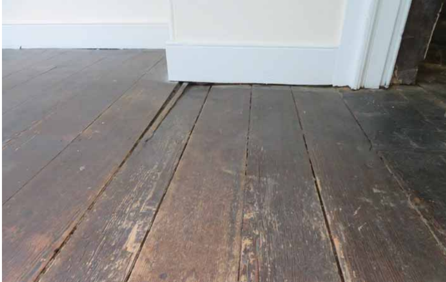
Figure 280. The west end of the floor boards to the south of the fireplace in the west bedroom (205) have dropped out of position. This condition is likely the result of moisture-based deterioration where the roofs above the kitchen and the southwest addition merge. JGWA, 2024.
