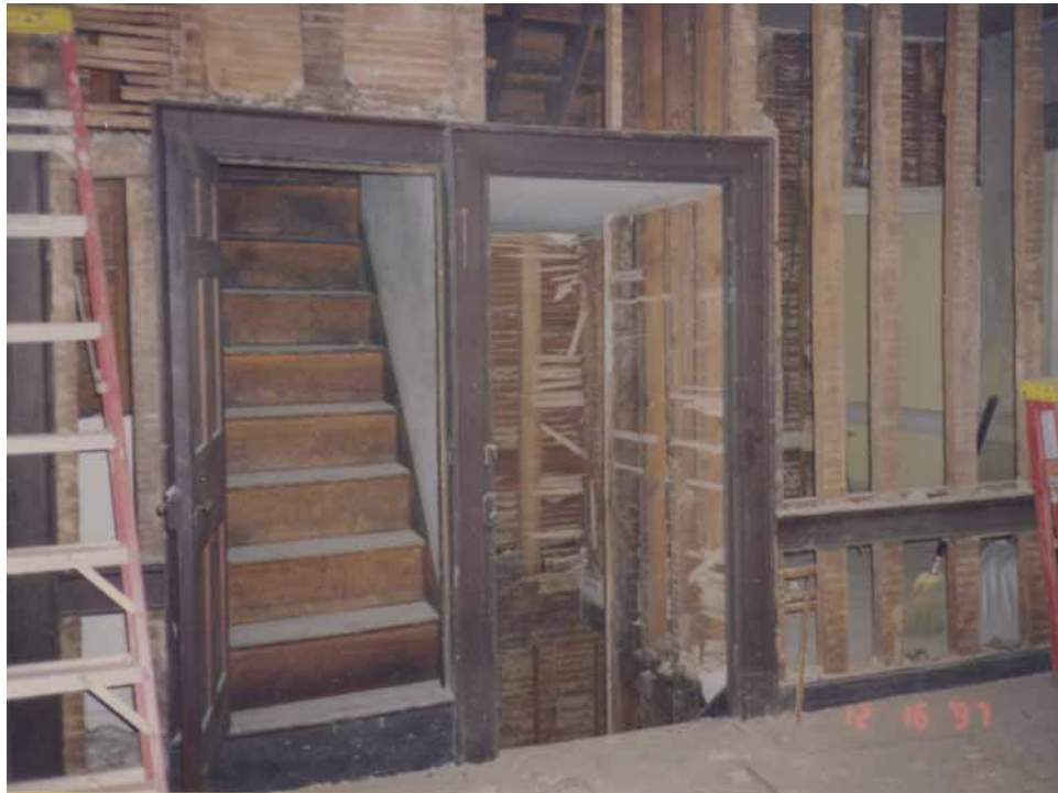
Figure 246. The west bedroom (205) during the 1997–1998 work. Courtesy of Nancy O'Brien.
