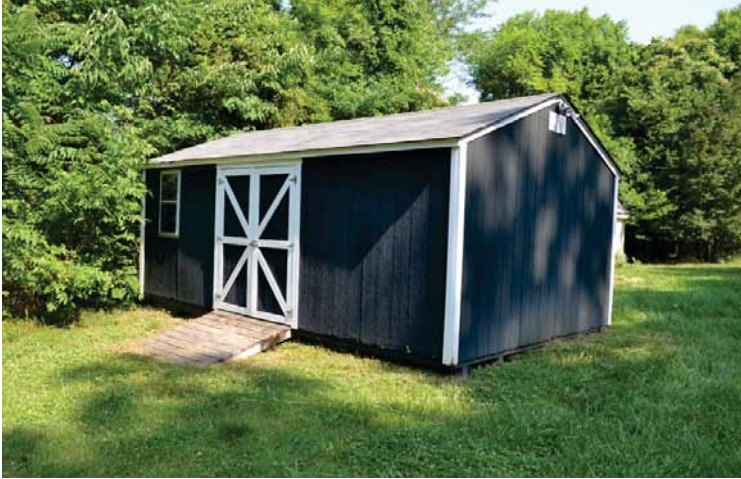
Figure 107. The prefabricated shed. LSHLA, 2024.
