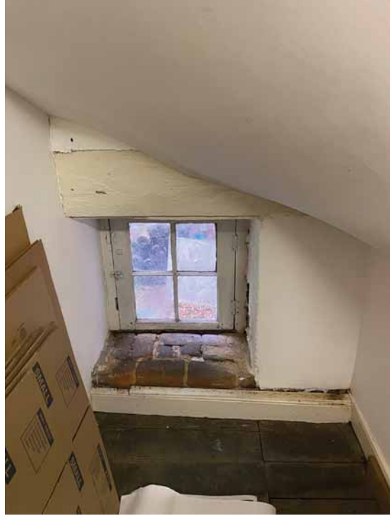
Figure 237. The storage under the stairs (106), looking north. JGWA, 2024.
