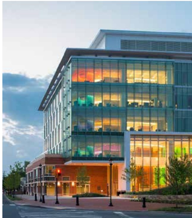
Exterior View of the Battle Building
