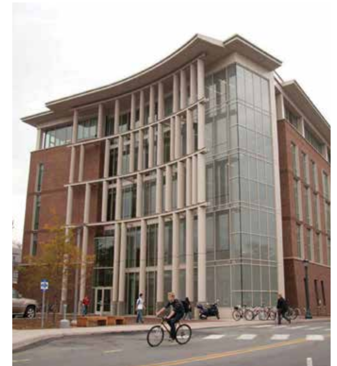
Exterior View of Rice Hall, Whitehead Road and Engineer's Way
