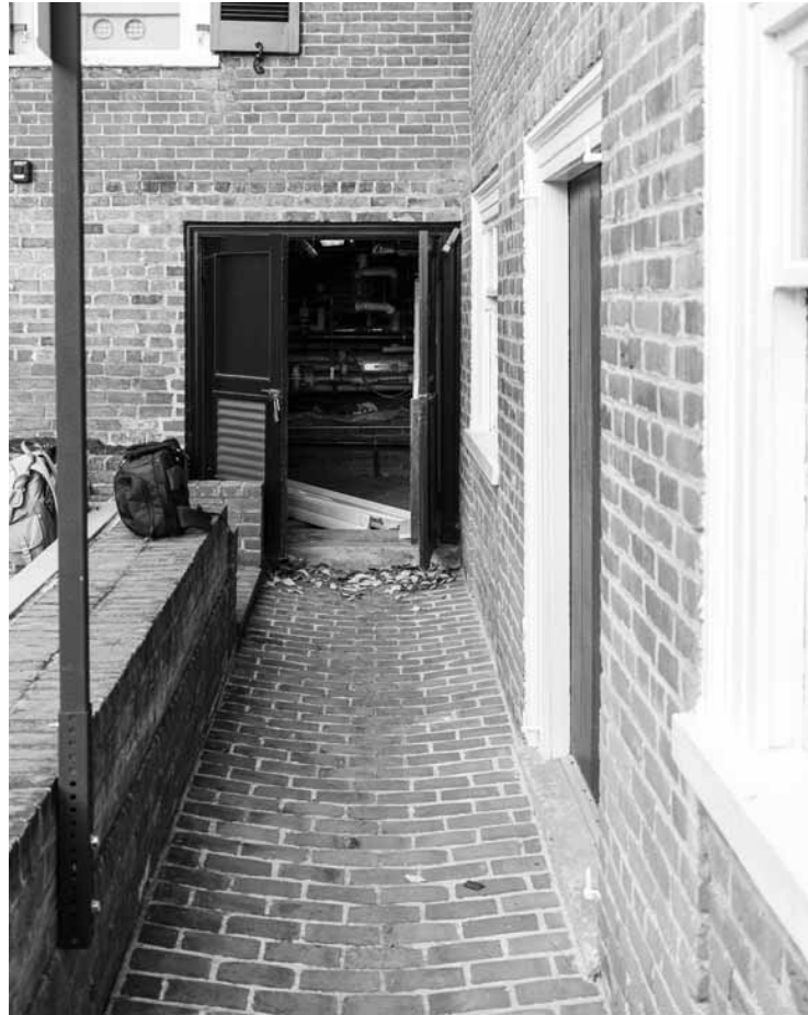
Figure 152. University of Virginia, Charlottesville, Virginia: 2 East Lawn cellar door, from area-way adjoining cellar at Pavilion II. Note that this area-way configuration must be early to accommodate the door from cellar of Pavilion II here, whose sill would otherwise be below grade.
