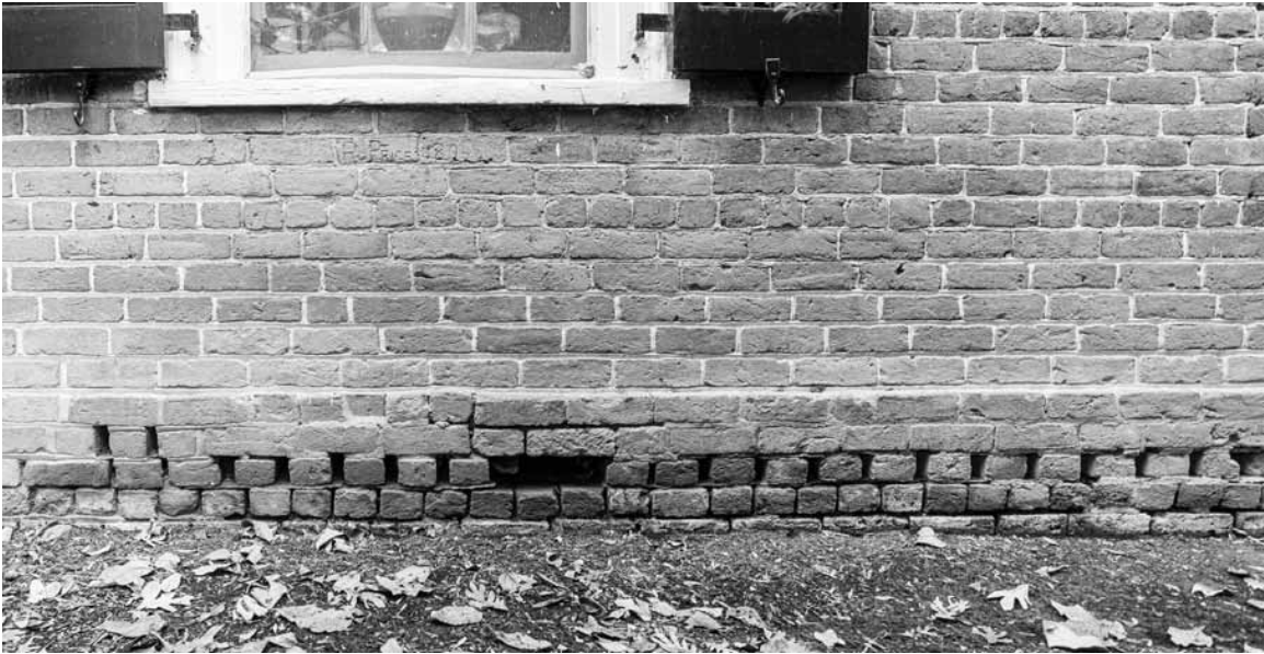
Figure 48. University of Virginia, Charlottesville, Virginia: West Range 5-15, detail of vent holes with slate inserted at rear of rooms in 1858, at 13 West Range, Poe Room.
