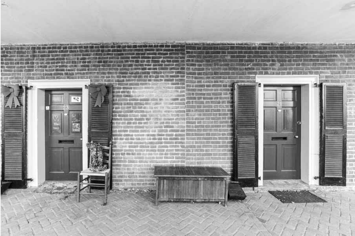
Figure 112. University of Virginia, Charlottesville, Virginia: entry to student rooms 21 and 23. West Lawn. Note seam in masonry reflecting construction of 23-33 previous to room 21. Note, too, the use of 3-course common bond at 23-33 and Flemish at 21, at the right.
