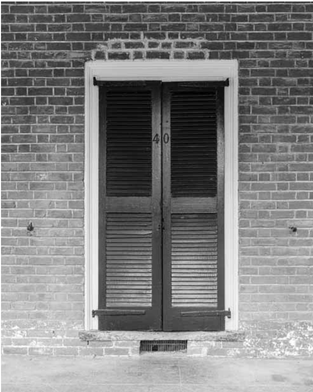
Figure 114. University of Virginia, Charlottesville, Virginia, 40 East Range door opening with blinds closed. Note re-pointed masonry above door.
