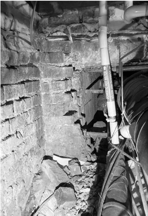
Figure 74. University of Virginia, Charlottesville, Virginia: crawl space under 28-46 East Range, showing partition penetration for systems in north wall of space below room 46.
