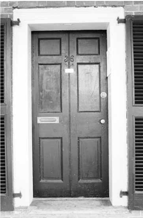
Figure 22. 36 East Lawn, University of Virginia, Charlottesville, Virginia: detail of double doors, as converted to single leaf. Photograph by Murray Howard, March, 1997, in situ.
