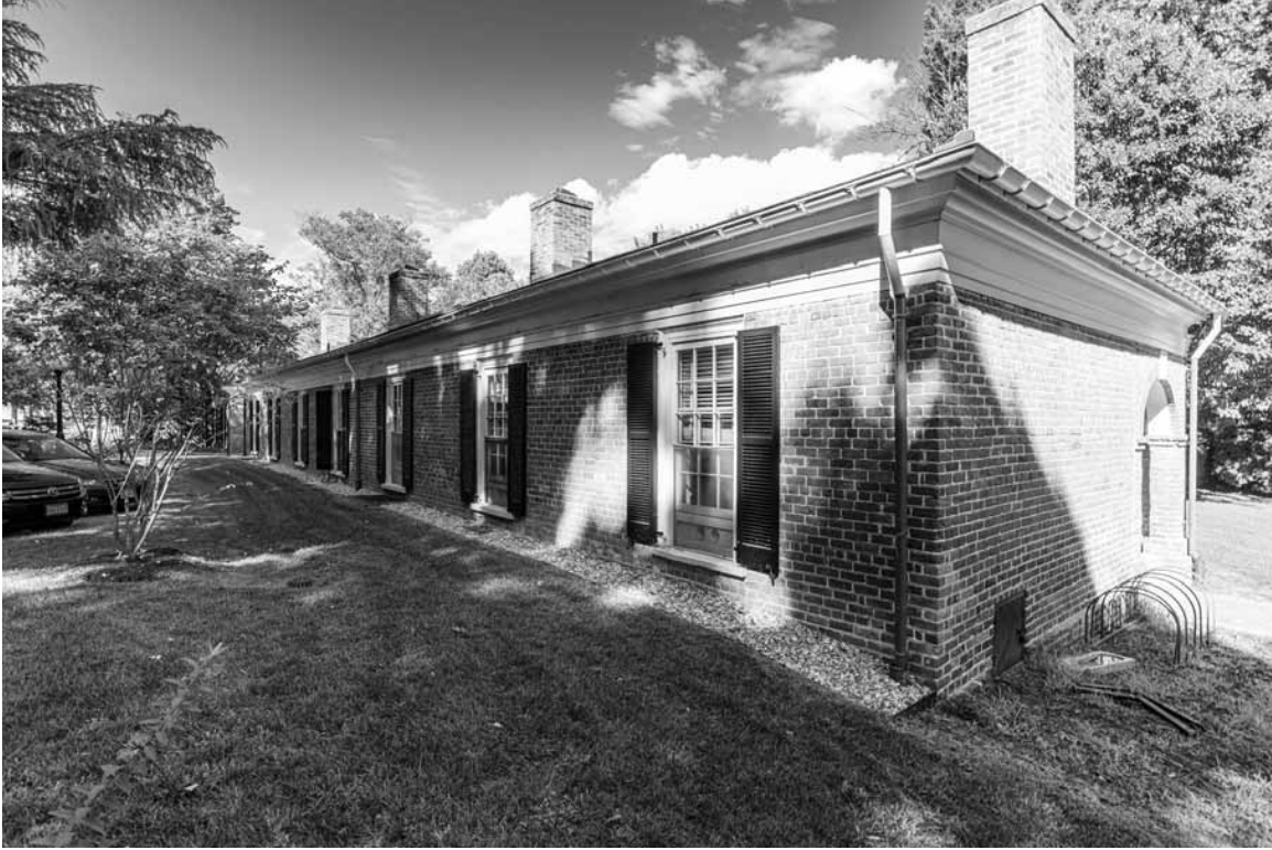
Figure 175. University of Virginia, Charlottesville, Virginia, East Range 6 to 18, rear. Note how present grade at rear comes within three courses of brick of the window sills.
