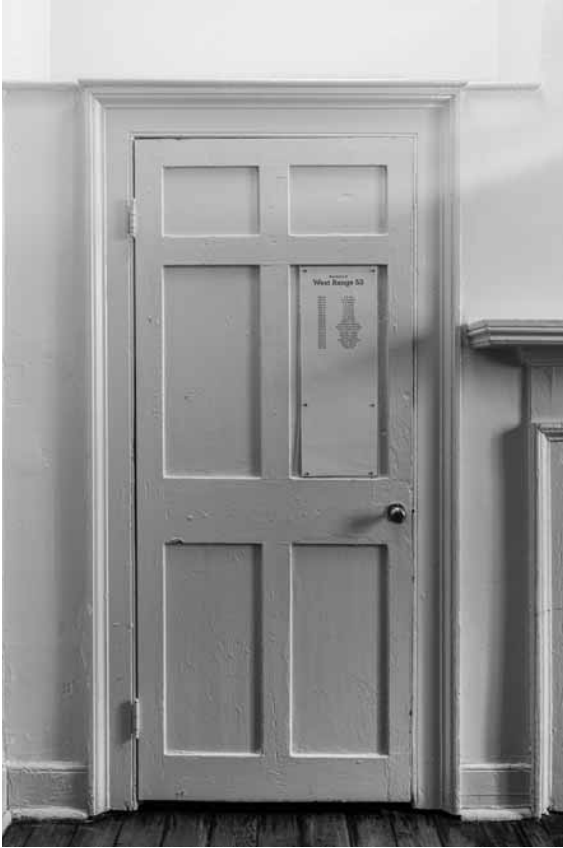
Figure 98. University of Virginia, Charlottesville, Virginia, 53 West Range, closet door detail.
