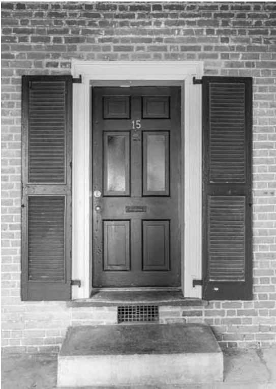
Figure 49. University of Virginia, Charlottesville, Virginia, West Range 15. Note seam and closers below door sill and infill masonry on either side of grate, showing where door and floor have been raised.
