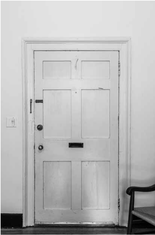
Figure 16. University of Virginia, Charlottesville, Virginia: 10 East Lawn, detail of door interior.
