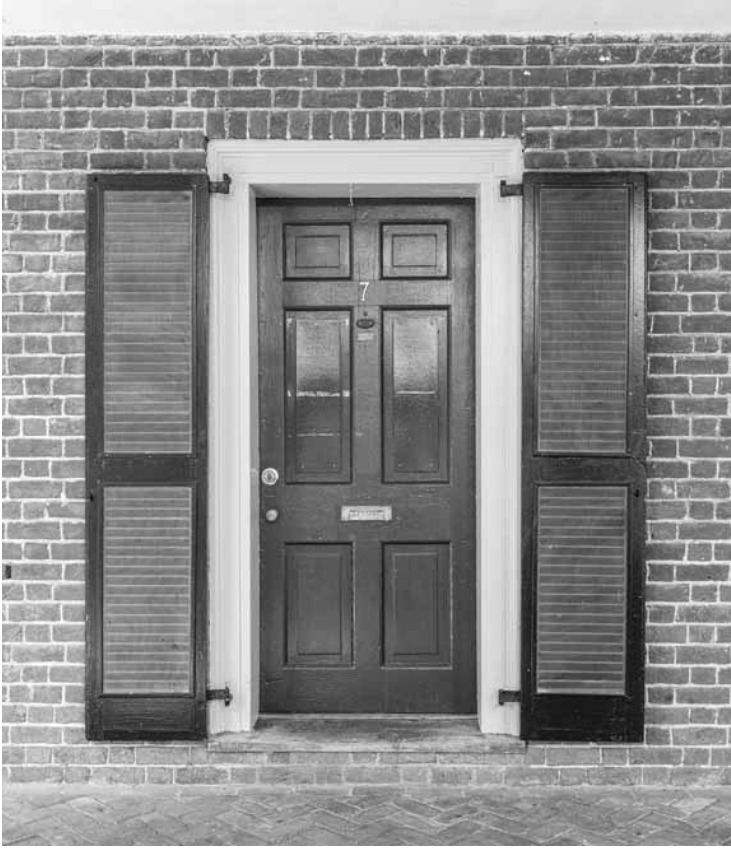
Figure 137. University of Virginia, Charlottesville, Virginia: 7 West Lawn. Note rowlock course above door.
