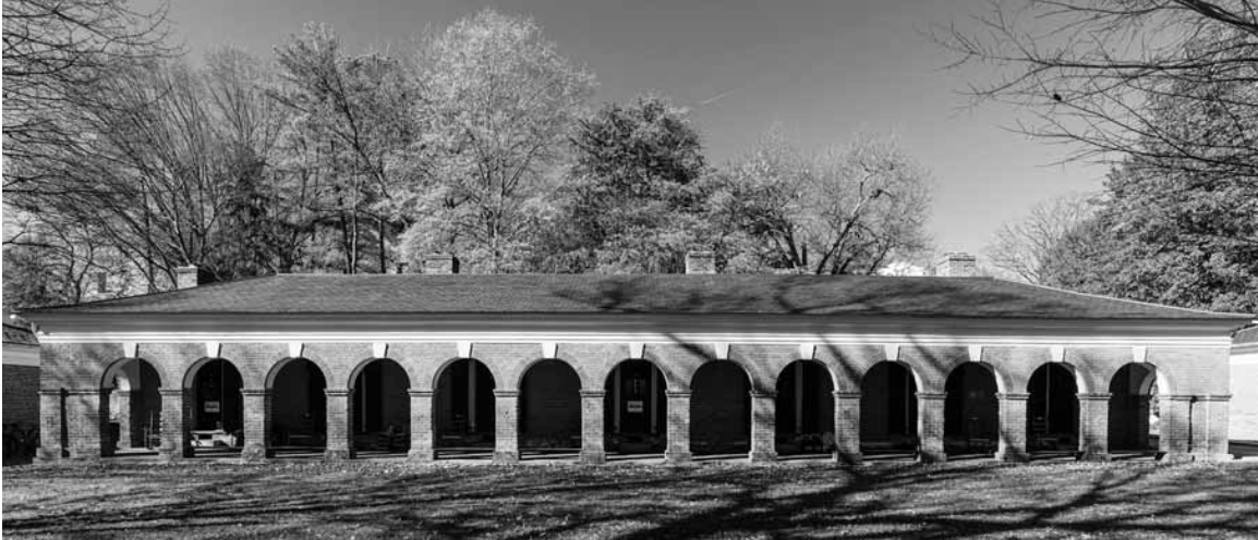
Figure 105. University of Virginia, Charlottesville, Virginia: 6-18 East Range, arcade.
