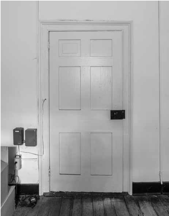
Figure 93. University of Virginia, Charlottesville, Virginia: 13 West Range door. Note replaced panel at upper left.
