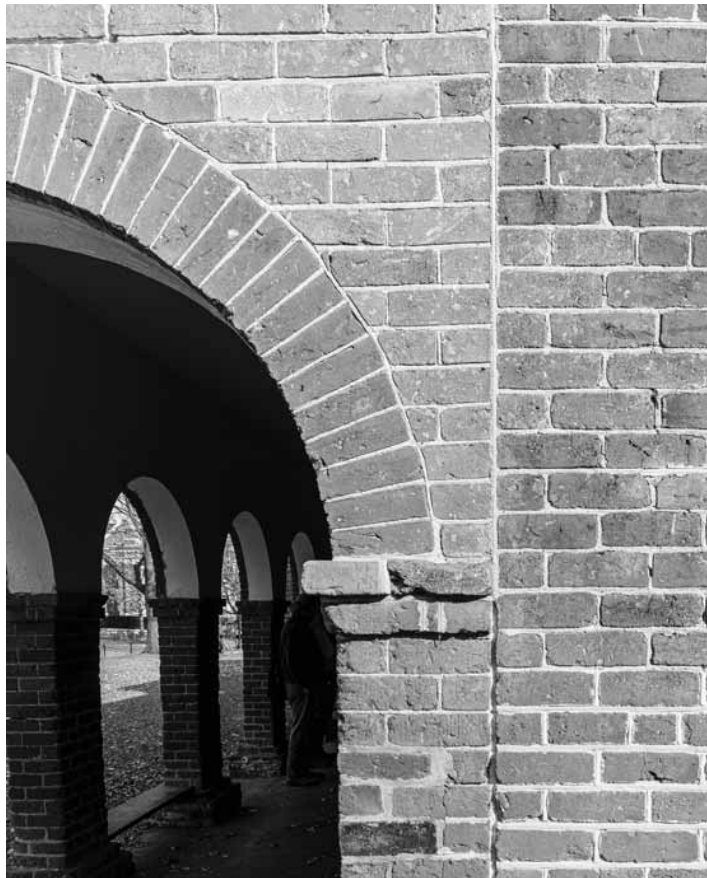
Figure 106. University of Virginia, Charlottesville, Virginia: 17-27 West Range. Note seam between arcade and body of dormitories.
