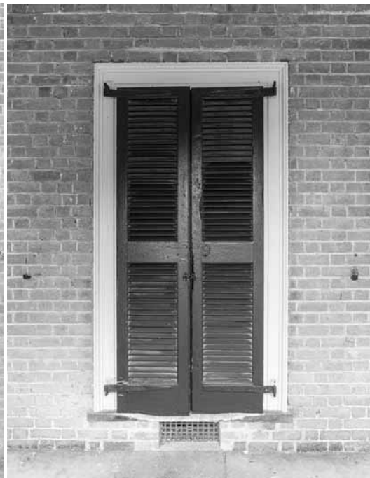
Figure 116. University of Virginia, Charlottesville, Virginia: 9 West Range with shutters closed.
