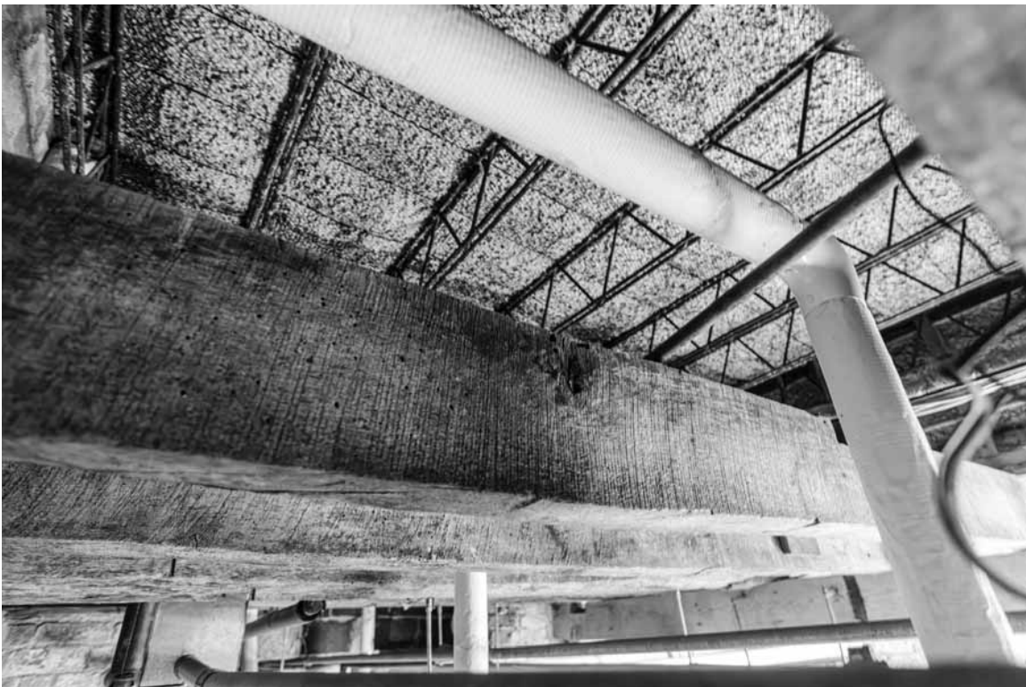
Figure 71. University of Virginia, Charlottesville, Virginia: East Range 24, cellar, showing hewn and pit-sawn joists bedded in joist pockets and raised floor above on metal truss joists.
