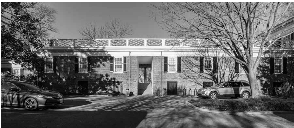
Figure 65. University of Virginia, Charlottesville, Virginia: 36-48 East Lawn, rear.
