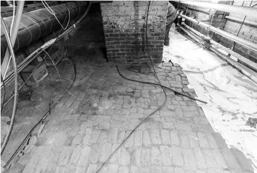
Figure 182. University of Virginia, Charlottesville, Virginia: 26 East Range cellar, showing floor paved with a mixture of bats and whole bricks.
