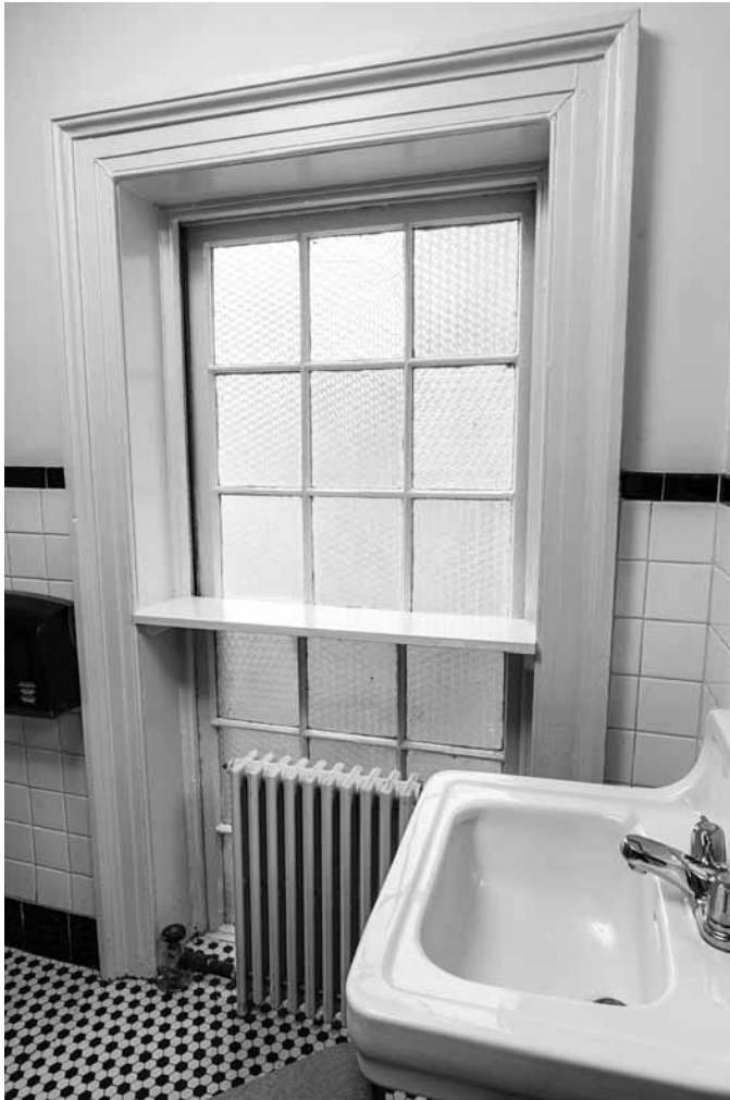
Figure 179. University of Virginia, Charlottesville, Virginia, 24 East Range, view of original window with surviving sash, currently in south bathroom of Center for Teaching Excellence (Hotel D).
