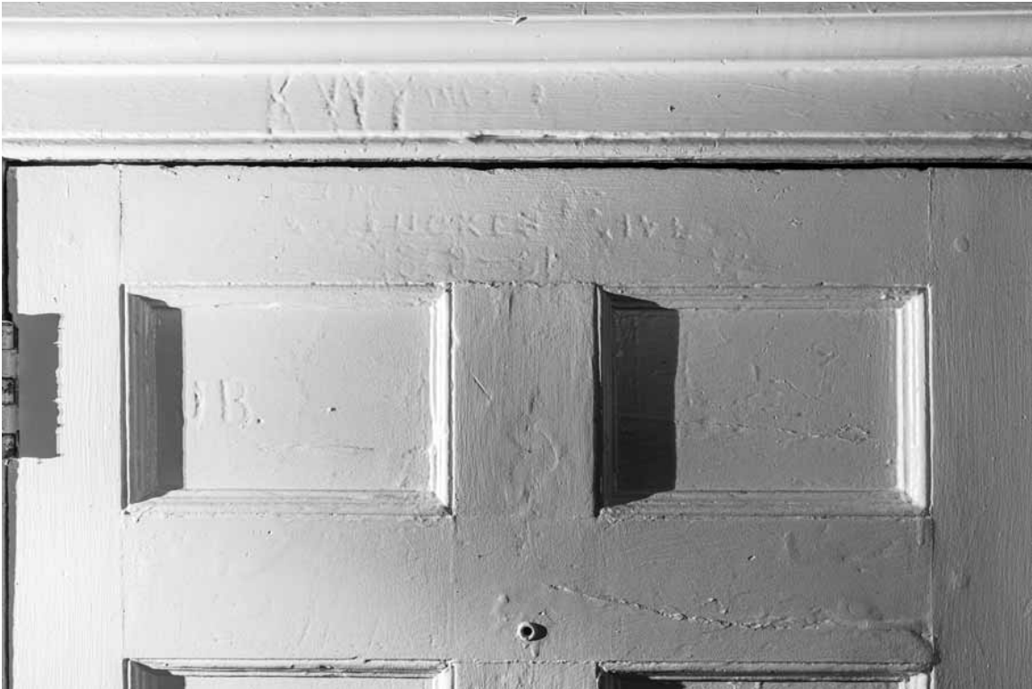
Figure 51. University of Virginia, Charlottesville, Virginia, West Lawn 37, detail of interior face of original door leaf with graffiti, including "JB" and "TUCKER [?] IV, 1859-61". Note that casing is also original except for back-band.
