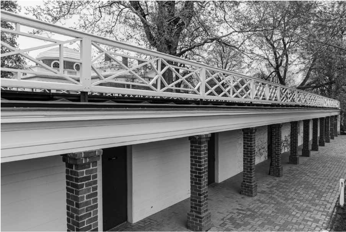
Figure 12. Monticello, Albemarle County, Virginia, begun 1768, enlarged and improved 1796-1809. View of mansion from service wing, showing square brick piers and Tuscan entablature. This composition of elements is what Jefferson initially envisioned for the colonnade fronting the Lawn dormitories.
