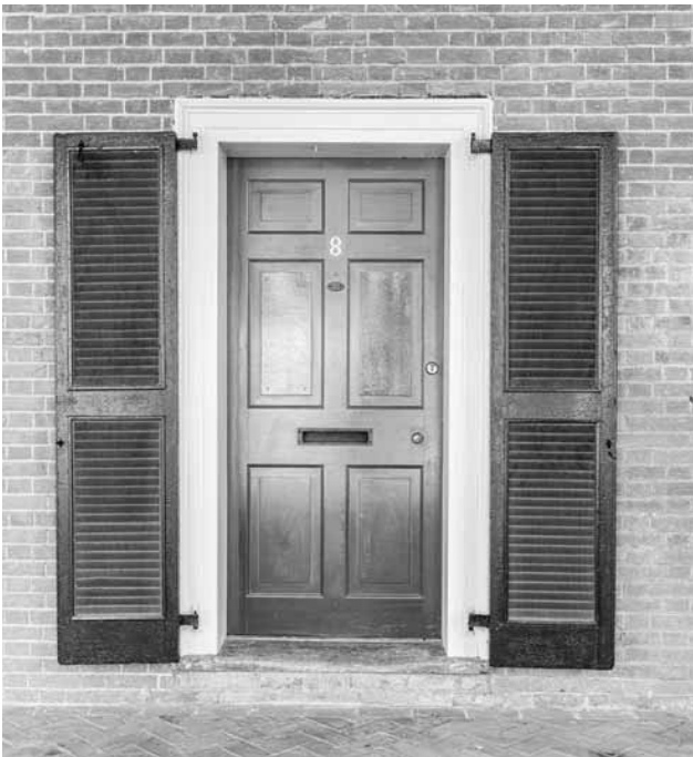
Figure 115. University of Virginia, Charlottesville, Virginia: 8 East Lawn, door installed 2012.
