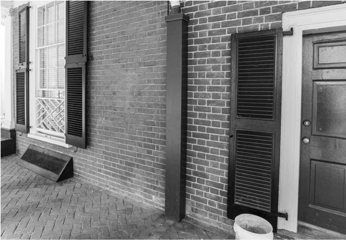
Figure 69. University of Virginia, Charlottesville, Virginia, West Lawn. Comparison of Pavilion IX masonry at left with smooth, oil-struck brick and 53 West Lawn at right, with sand-struck brick.
