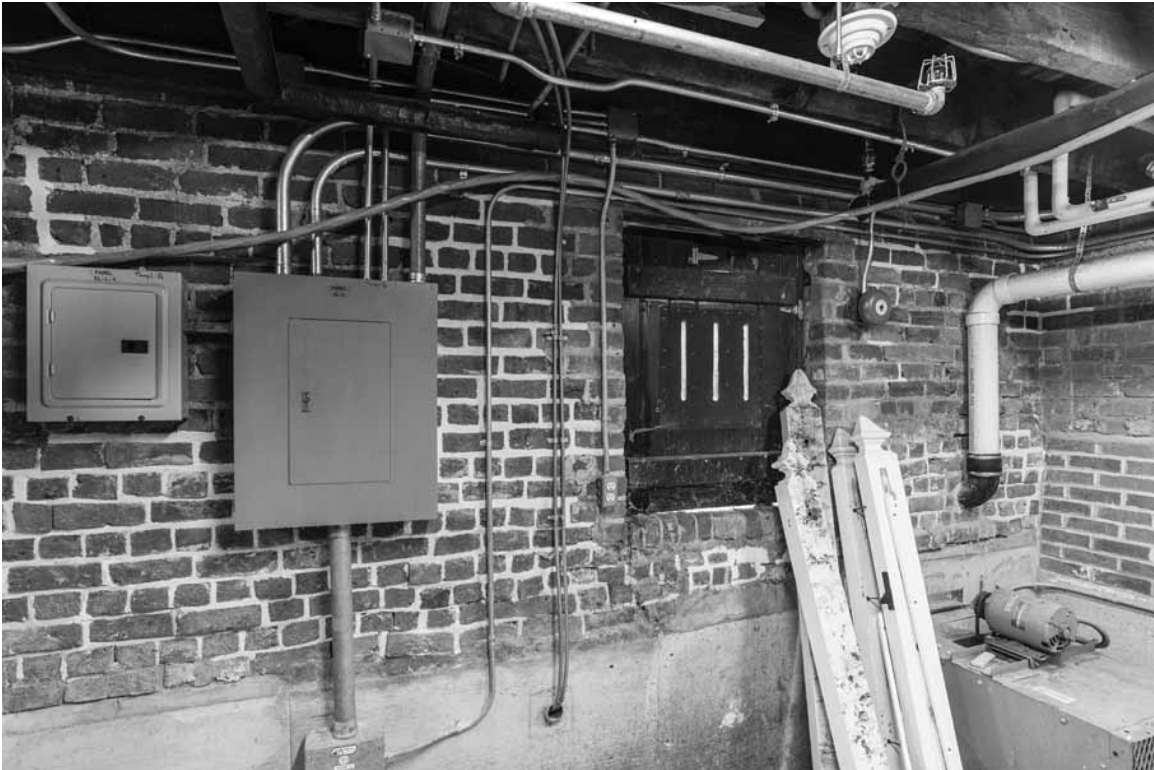
Figure 149. University of Virginia, Charlottesville, Virginia: East Lawn 4 cellar, showing concrete underpinning, repointing and new brick around inserted access hatch.
