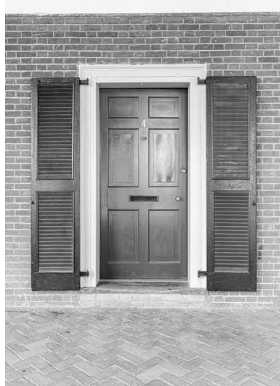
Figure 94. University of Virginia, Charlottesville, Virginia: 4 East Lawn, installed 2012.
