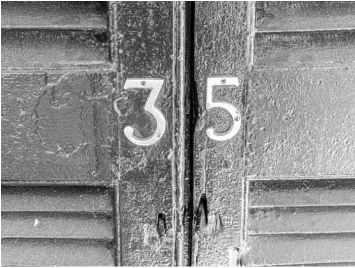
Figure 117. University of Virginia, Charlottesville, Virginia, 35 West Lawn with shutters closed, showing paint line from early plate latch at left, behind 3.
