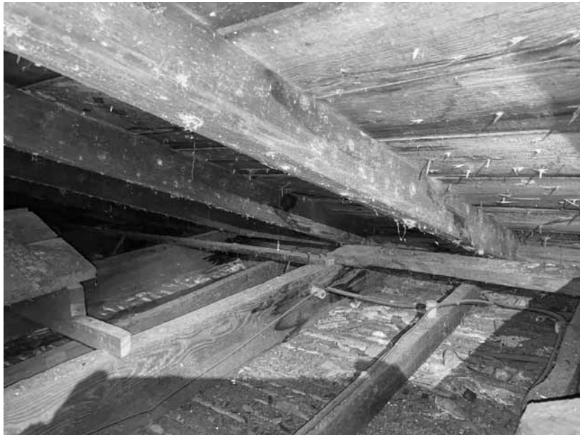
Figure 118. University of Virginia, Charlottesville, Virginia: attic of 5-15 West Range under 1837 roof. View of original joists and lath-and-plaster ceiling.
