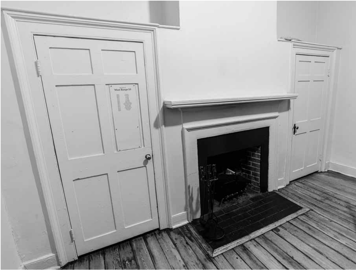
Figure 18. University of Virginia, Charlottesville, Virginia, West Range 53, view of surviving original closets and mantel, the only complete set of such elements to remain in place on Grounds.
