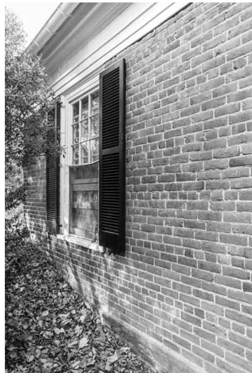
Figure 69. University of Virginia, Charlottesville, Virginia, West Lawn. Comparison of Pavilion IX masonry at left with smooth, oil-struck brick and 53 West Lawn at right, with sand-struck brick.
