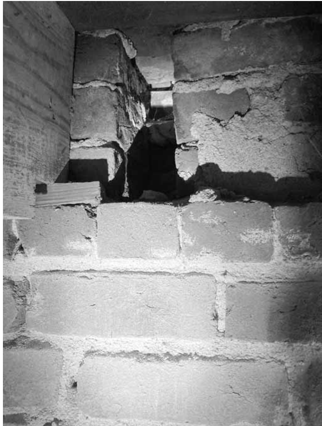
Figure 72. University of Virginia, Charlottesville, Virginia: crawl space under 17-21 West Range, with detail of original joist pocket and modern replacement framing.
