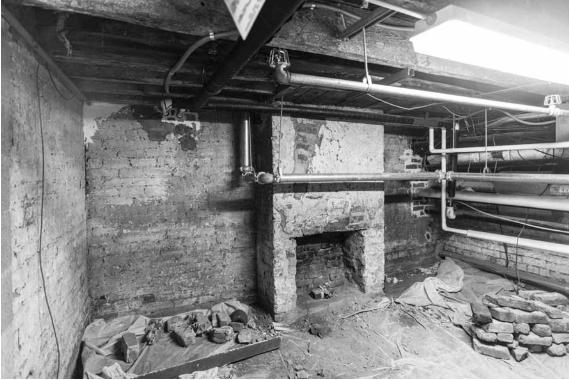
Figure 160. University of Virginia, Charlottesville, Virginia: East Lawn 22 cellar, showing limewashed walls and ceiling joists and retrofitted fireplace.
