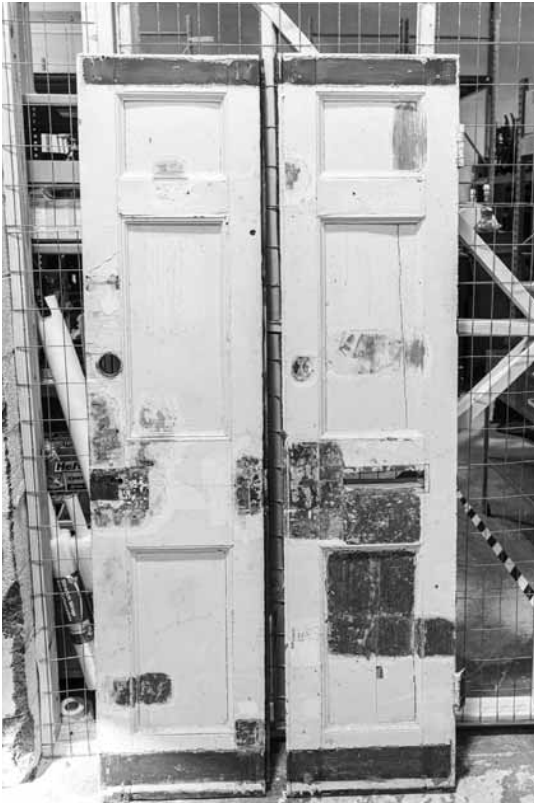
Figure 164. University of Virginia, Charlottesville, Virginia: double doors removed from 36 East Lawn, interior face. Note grained paint exposed in voids at top and bottom of doors for battens (since removed) used to join doors into single leaf.
