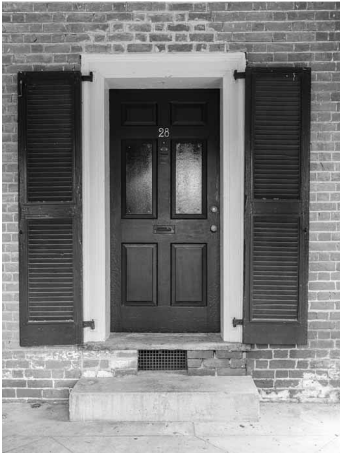
Figure 119. University of Virginia, Charlottesville, Virginia, 28 East Range, detail of door raised to accommodate raised floor. Note seams in masonry below sill, repointed masonry above head, and cut brick just below head, all consistent with the door being raised two or three courses.
