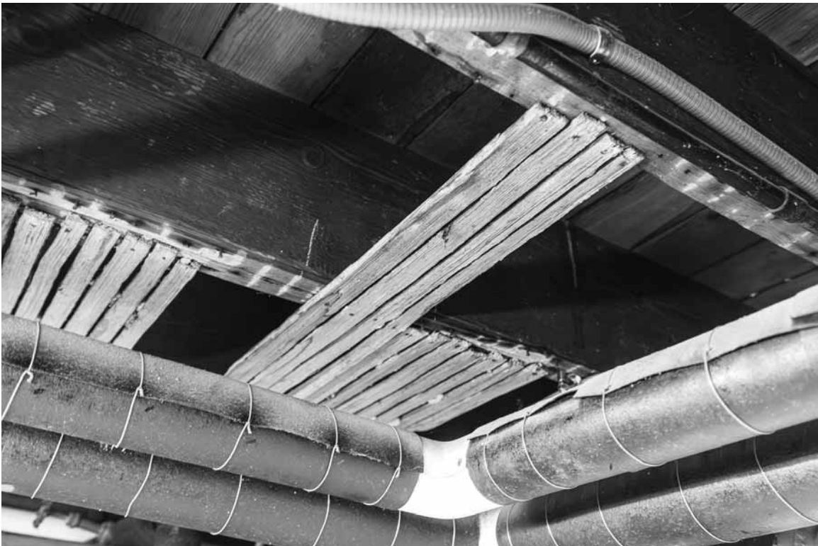
Figure 67. University of Virginia, Charlottesville, Virginia: East Lawn 24 cellar, showing ceiling lath.
