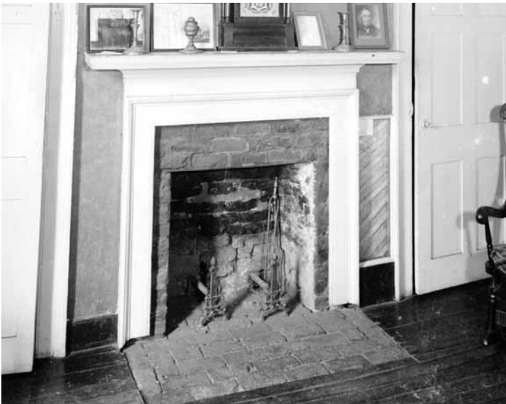
Figure 99. University of Virginia, detail of Holsinger photograph of Poe Room, 13 West Range, c. 1900, before removal of closets. Note area of removed plaster to expose diagonal lath between mantel and closet door.
