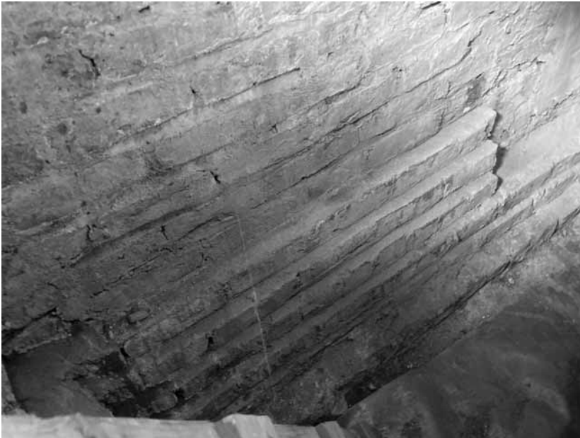
Figure 68. University of Virginia, Charlottesville, Virginia: cellar below East Range student room 54, detail of stepped spread footing at base of west wall.
