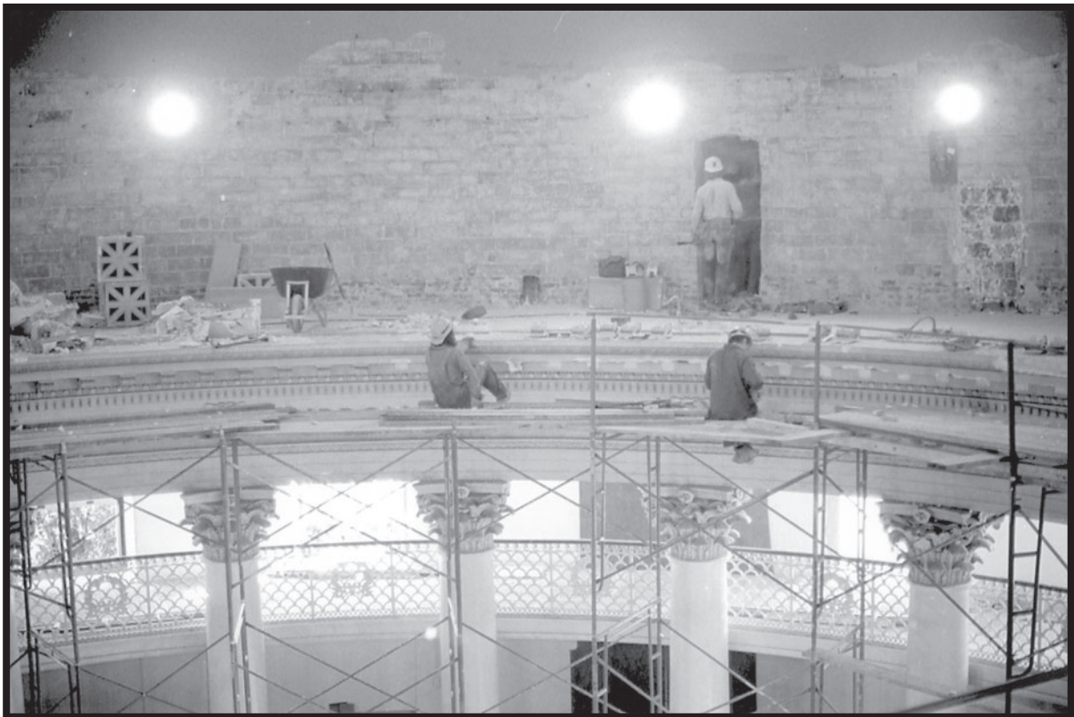
FIGURE 107. The interior of the Rotunda during demolition, 1974. The brick that was laid up against the original outer wall in 1898 to support the Guastavino tile dome conceals any pre-fire evidence that might remain on the walls.
