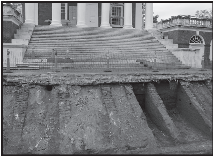
FIGURE 143. The north facade of the Rotunda, the north steps to Rotunda, and the supporting brick buttresses (foreground).
