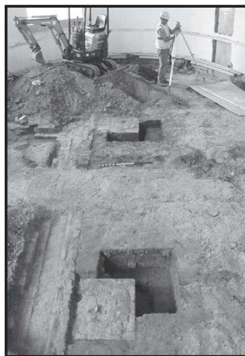
FIGURE 139. Lower east oval room, looking south, showing centrally located brick piers (top and bottom), adjacent excavation units, and remnant McKim, Mead and White brick conduit (left of piers).
