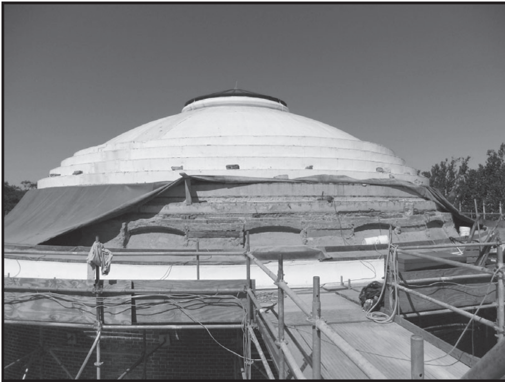
FIGURE 229. Removal of the lower step rings during the roof work uncovered a series of perimeter arches and piers.
