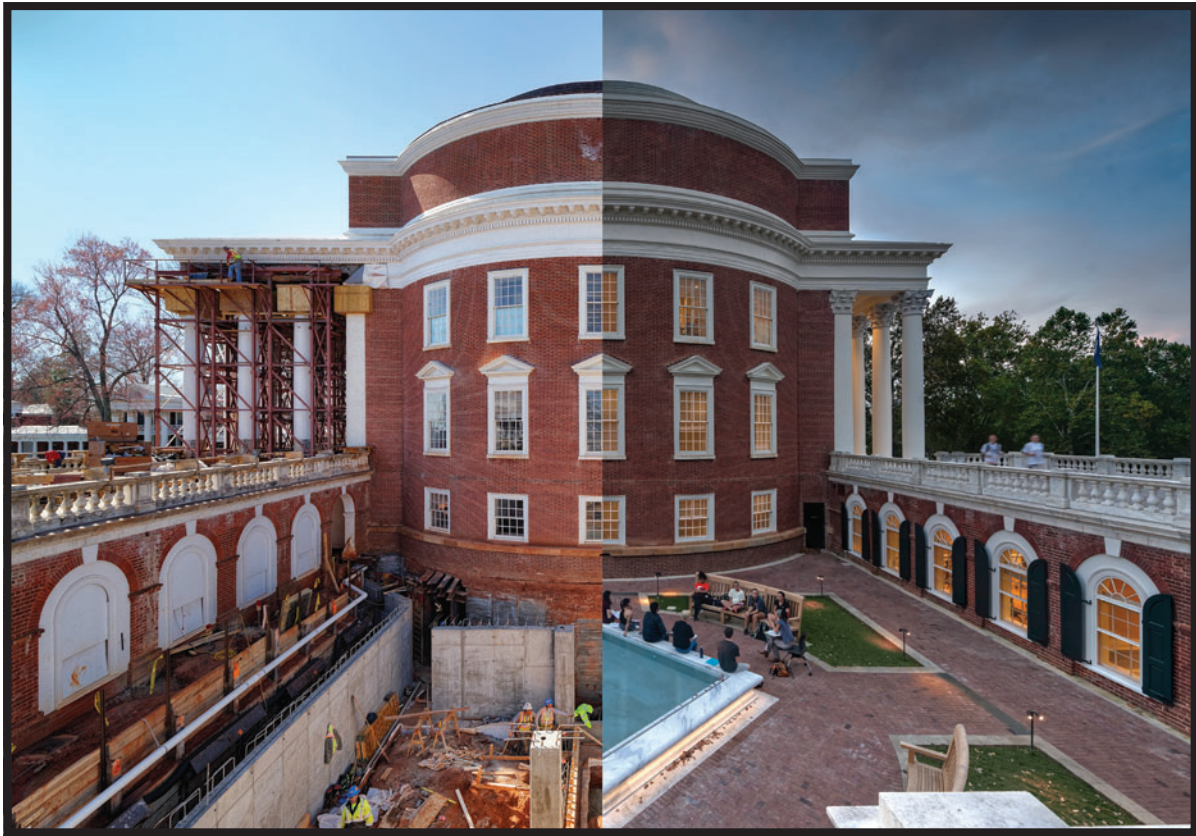
The Rotunda: (left) during construction, showing the excavation and underpinning for the mechanical vault below the east courtyard; (right), view of the completed restoration and renovation, 2016.
