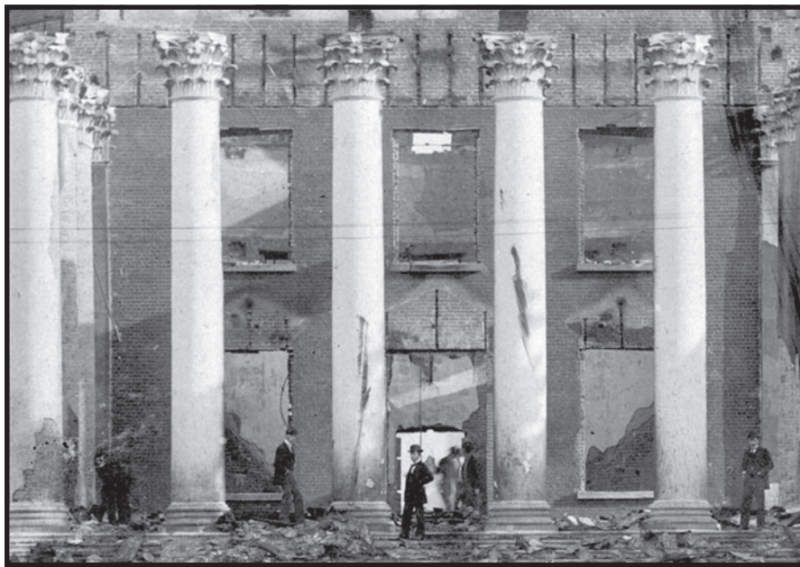
FIGURE 54. Detail of the October 28, 1895, photograph. The locations of the original nailing grounds and the outlines of the pediments are clearly shown above the first-story openings. Fragments of the original interior finishes can be seen through the openings.
