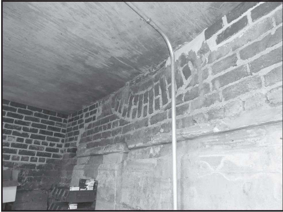
FIGURE 223. Inverted arches in the original foundation, now revealed in corridor C003 and room M004.
