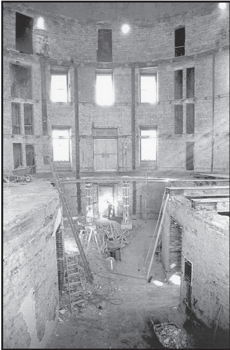
FIGURE 111. The interior during demolition, January 30, 1974. The ground-floor walls to the right and left survive from the original construction.
