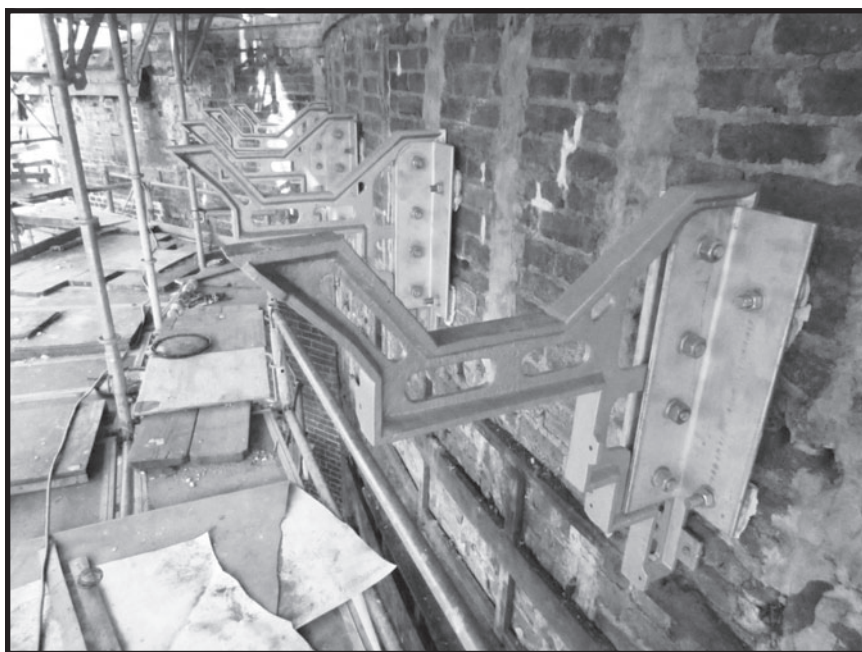
FIGURE 230. Reinstallation of the exterior cornice brackets. The McKim, Mead and White brackets were cleaned and recoated, and new angles were added to provide additional support.
