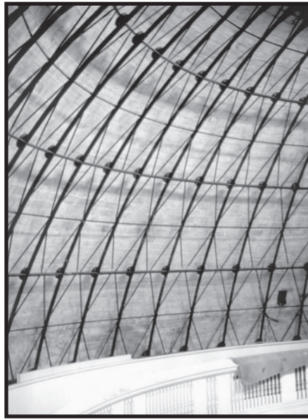
FIGURE 115. Framework for the acoustical ceiling in the Dome Room, October 10, 1975.
