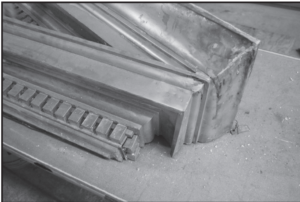
FIGURE 180. Copper pediment from ground-floor window during restoration.
