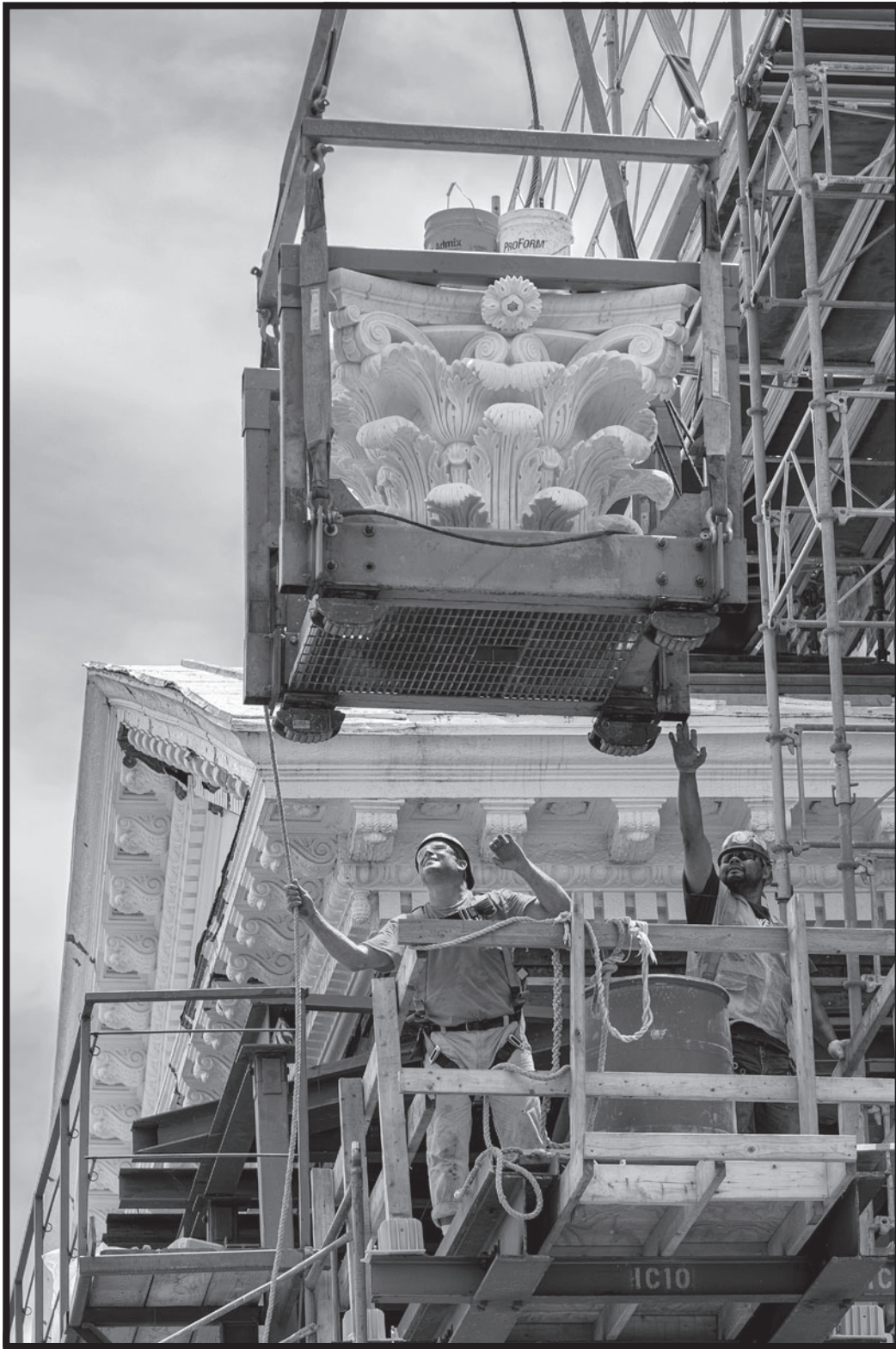
FIGURE 119. Installation of one of the new marble capitals, 2016.
