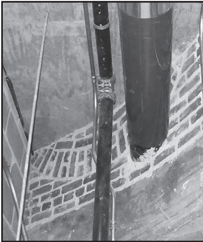
FIGURE 223. Inverted arches in the original foundation, now revealed in corridor C003 and room M004.
