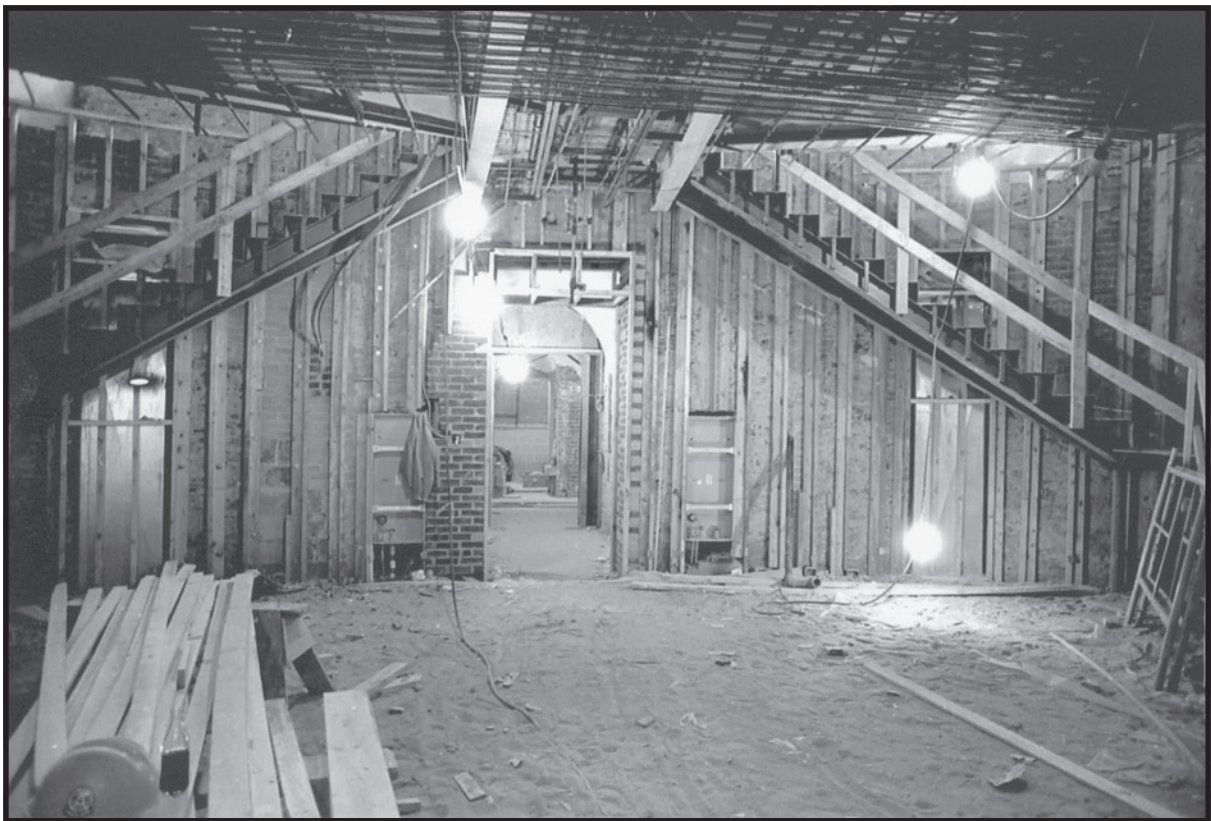
FIGURE 114. Construction of the ground floor looking south, May 8, 1975. The steel for the new stairs is in place.
