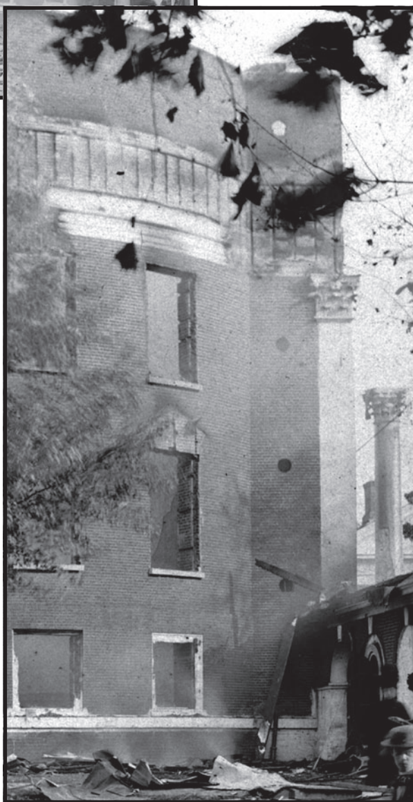
FIGURE 56. Detail of the 1895 view from the west, showing evidence of the window reveals and the round openings in the west face of the south portico.
