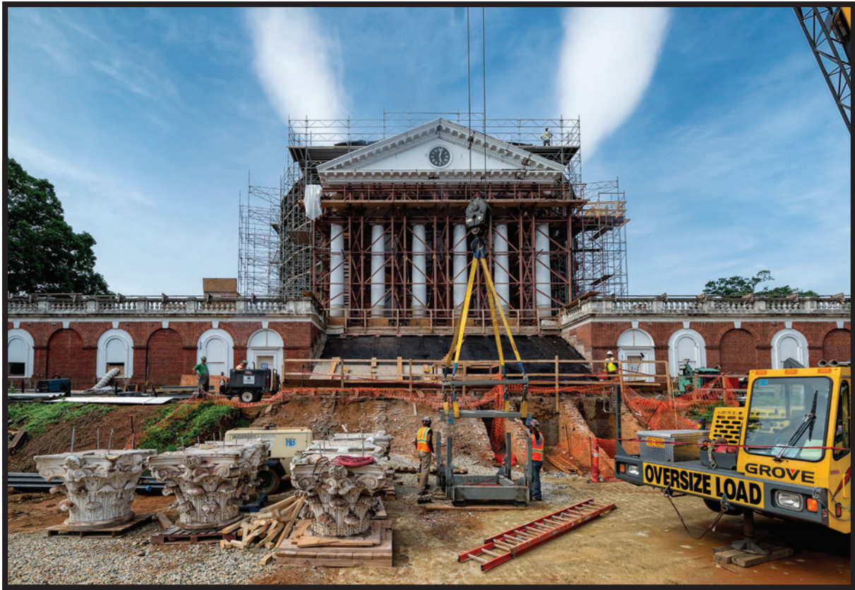
The Rotunda under construction, June 2016. In this view from the north, the 1890s capitals have been removed and sit in the foreground. Note the exposed buttresses beneath the north stairs.
