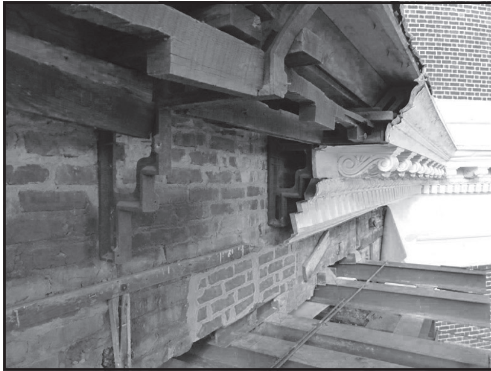
FIGURE 174. Intermediate cornice and support system revealed during restoration.
