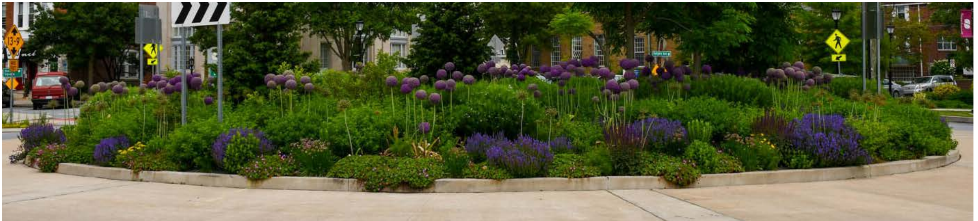
Swarthmore College Roundabout - 60ft diameter with 15ft concrete skirt and mountable curb
