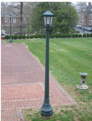
General Path Lighting, King Edgewater K-56 metal halide or LED luminaire on 12' cast aluminum or cast iron octagonal pole, Rookwood shutter green, pebbled lenses
