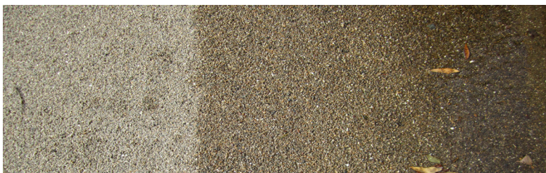
Addastone Resin Bounded Surface System. Above picture taken after rain in Poe Alley.
