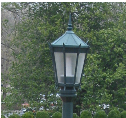
General Path Lighting, King Edgewater K-56 metal halide or LED luminaire on 12' cast aluminum or cast iron octagonal pole, Rookwood shutter green, pebbled lenses
