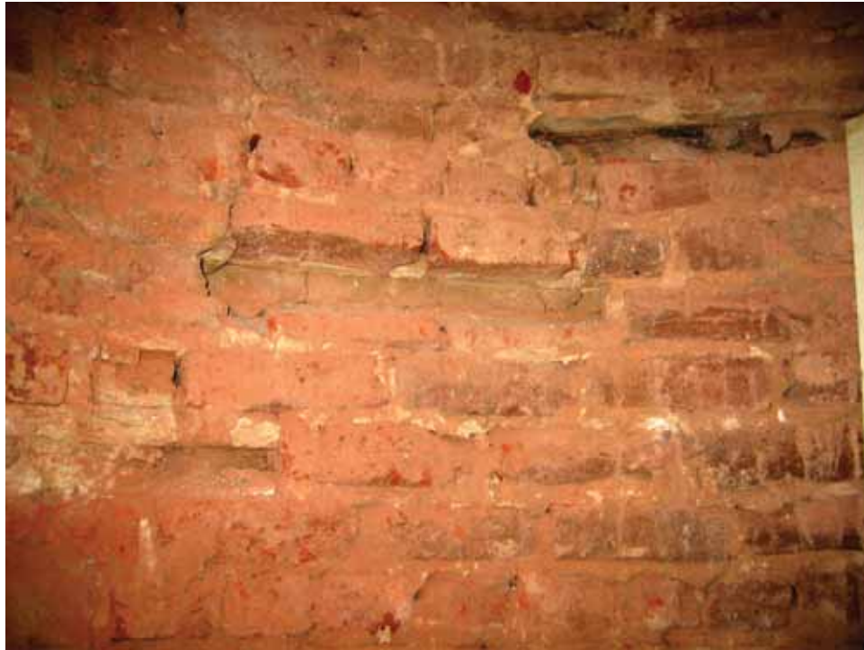
Recesses for stair treads in stairwell of 105. [JGWA, 2005]
