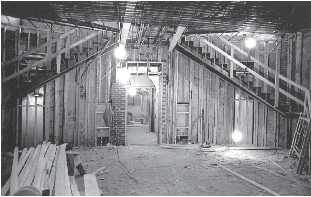
Figure 113. Construction of the ground floor, looking south, May 8, 1975. The steel for the new stairs is in place. [Special Collections, UVA]
