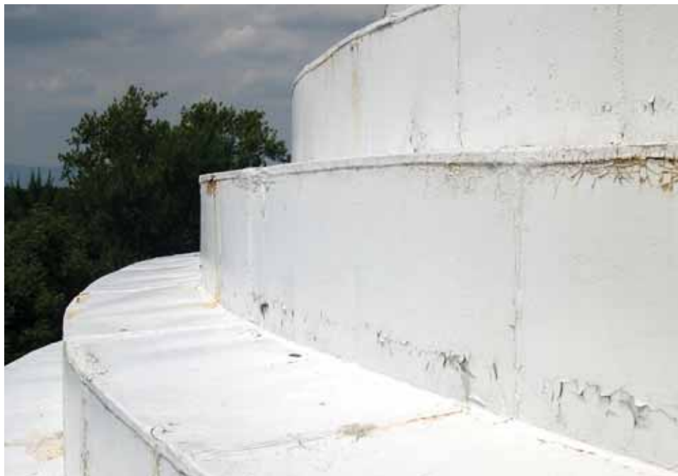
Rotunda, Roof. The painted finish on the terne-coated sheet metal roofing of the dome is crazed and rust stained; this condition is pronounced on the north elevation. [JGWA, 2006]
