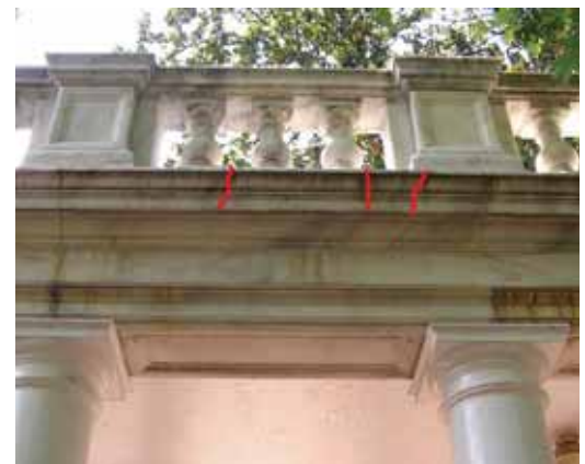
Figure 10: Vertical hairline cracks were observed in the marble cornice and lintels.
