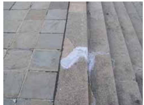
Figure 18: Attempts to repair the spalling concrete at the interface of the slate pavers and cracks running down the stairs are failing.
