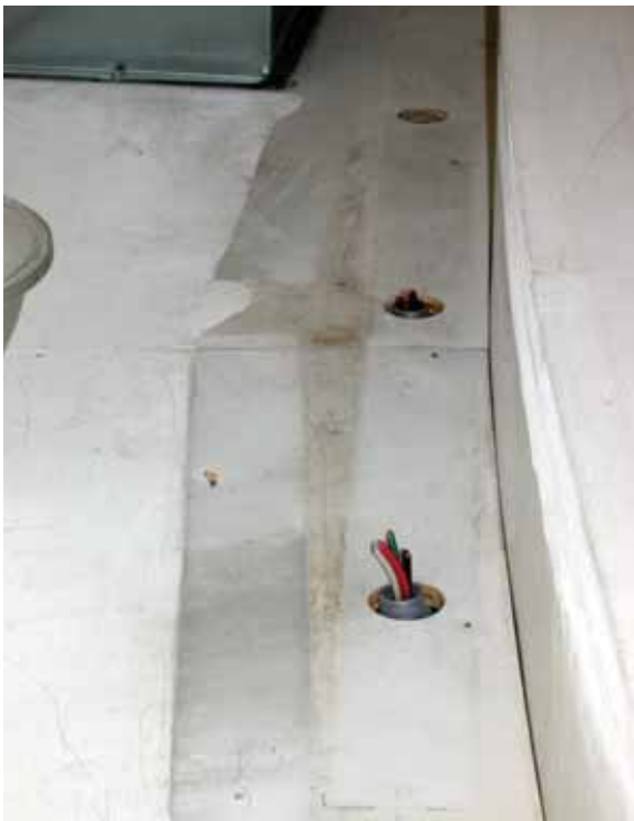
The fluorescent strip lighting fixtures at the base of the dome were removed in December 2006 as part of the mold remediation project. Exposed conductors protruding from conduit remain; these conductors may present an electrical shock hazard. [JGWA, 2006 (top), 2007 (bottom)]
