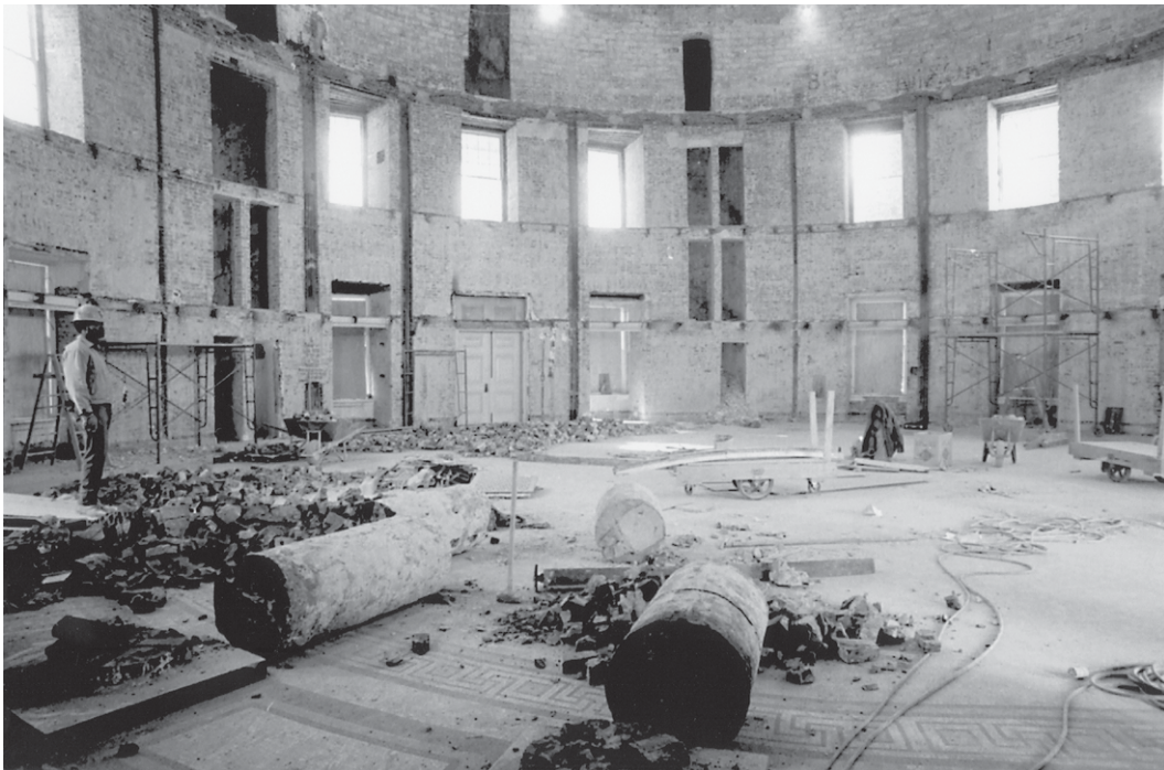
Figure 107. Two views of the interior of the Rotunda during the 1974 demolition [n.d]. The brick laid up against the original outer wall in 1898 (to support the Guastavino tile dome) conceals any pre-fire evidence that might remain on the walls.[Special Collections, UVA]
