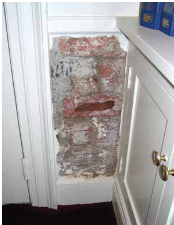
The plaster finish is missing from the south wall of the office of the Vice President for Student Affairs (124), west of the door opening and below the chair rail. The hollow clay tile wall construction is exposed. [JGWA, 2006]
