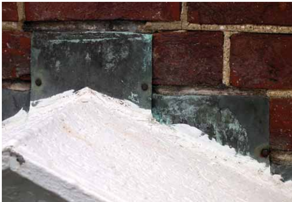
Rotunda, West Elevation. The copper step flashing above the pediments of the first floor windows is nailed into the masonry with ferrous cut nails. Galvanic corrosion is attacking the nails. [JGWA, 2006]
