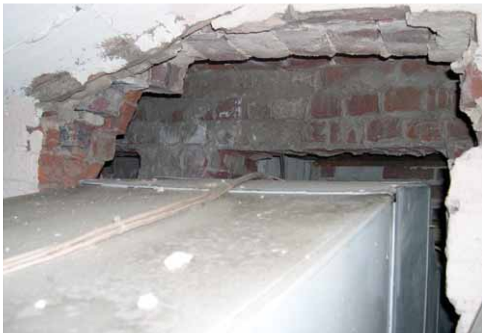
Large duct penetrations have been made in the north wall of the South Portico Attic (402) without providing lintels to support the brick construction above. [JGWA, 2006]
