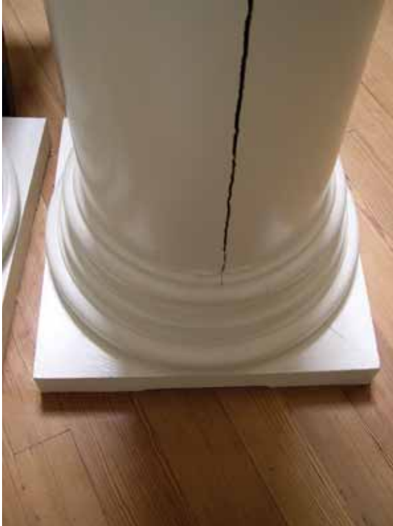
One column in each pair of columns encircling the Dome Room (301) has two vertical cracks, opposed 180 degrees from one another. The cracked wood columns have structural steel columns within them. [JGWA, 2006]
