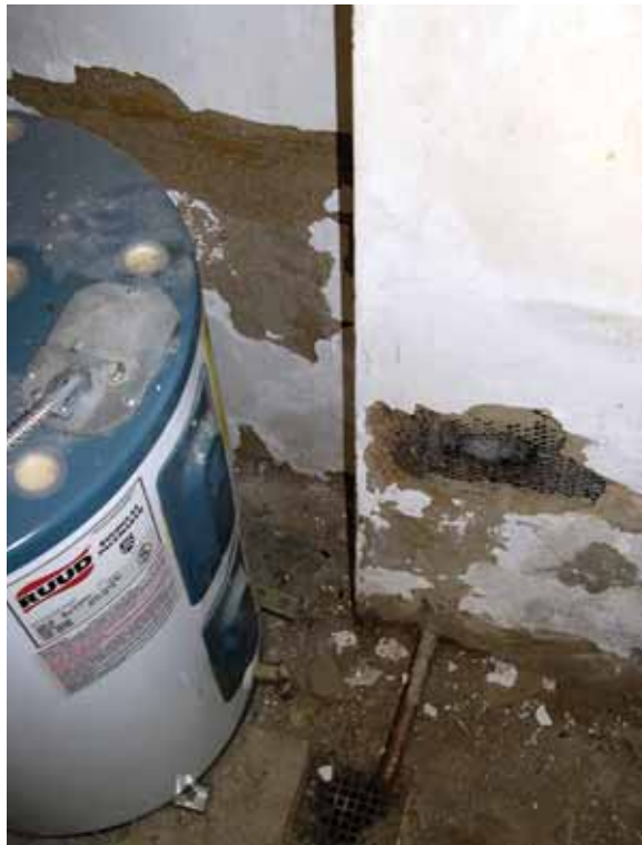
Rising damp has caused the wall plaster in Closet (T102B) to deteriorate, exposing the metal lath and brown coats of plaster. [JGWA, 2006]
