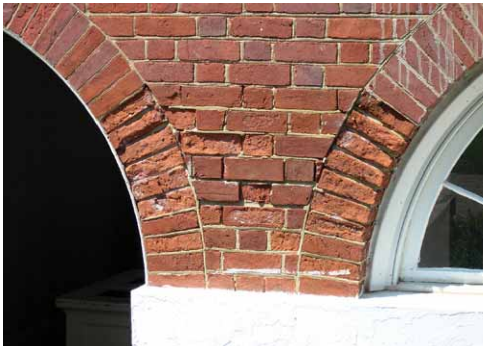
Southeast Wing, South Elevation. The brickwork has been grit-blasted, leaving an eroded surface. The brick is spalling in isolated locations, and there are lime-run (calcium carbonate) deposits on the brickwork beneath the marble cornice. [JGWA, 2006]
