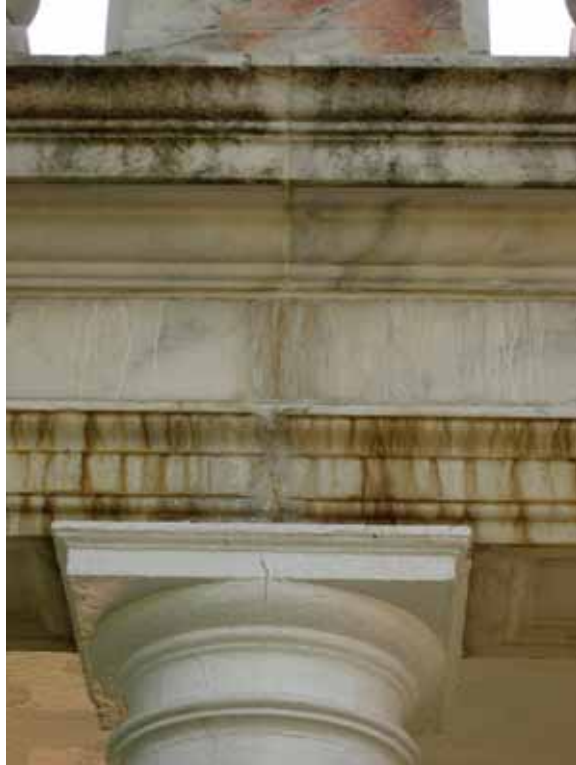
West Colonnade, West Elevation. There are lime-run (calcium carbonate) deposits at the vertical joints in the marble entablature, and rust colored staining on the architrave. This deterioration has resulted from water percolating through the terrace construction above. [JGWA, 2006]
