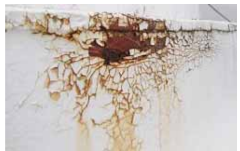
Figure 19: The metal roofing is corroding and exfoliating causing the paint to peel and blister, this is especially evident at joints and corner seams.
