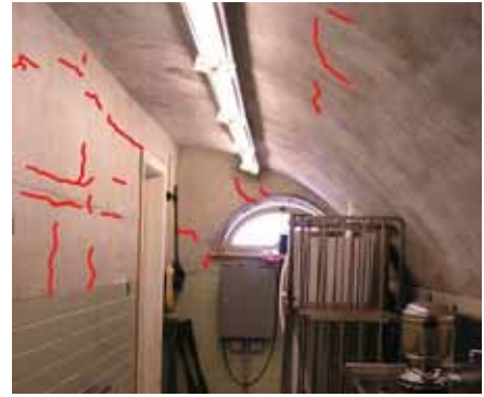
Figure 15: The walls and ceiling of the catering room below the south stairs has numerous cracks.
