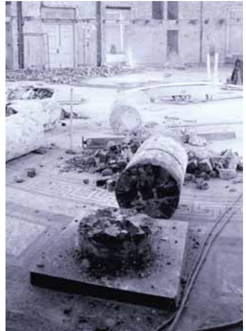
Figure 2: The McKim, Mead & White interior columns were built up brick columns. (Picture from 1970 Restoration provided by John G. Waite Associates)
