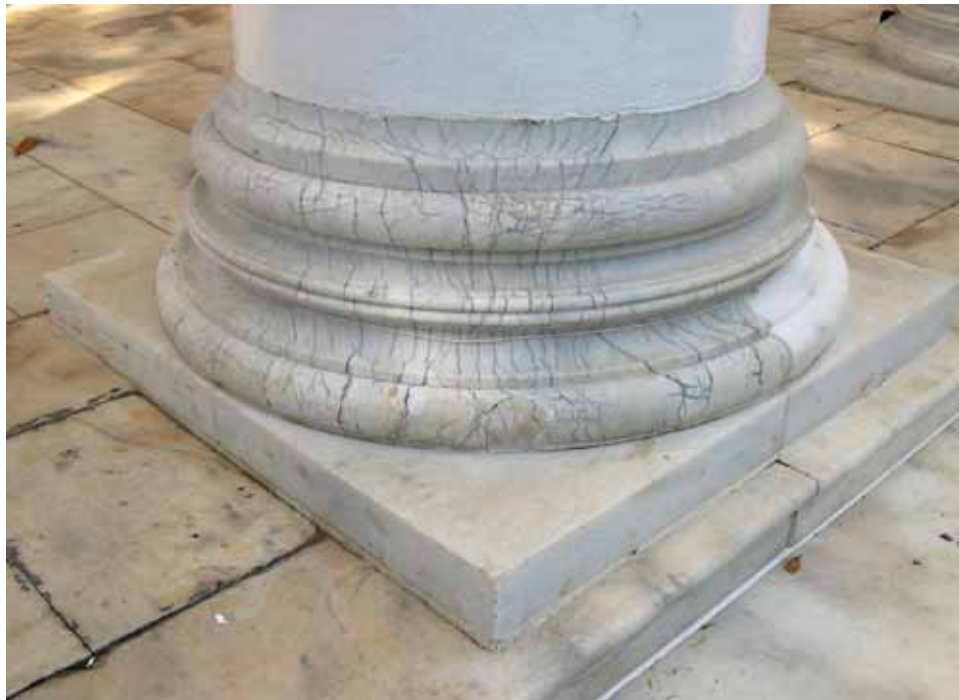
South Portico. The marble column bases have networks of cracks. [JGWA, 2006]
