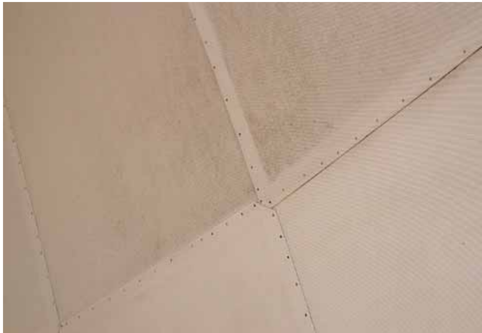
Some of the vinyl-coated, perforated metal acoustic ceiling panels that line the dome are discolored. Mold was growing on the surface of individual panels prior to the December 2006 mold remediation project. Many of the rivets used to fasten the ceiling panels are rusted. [JGWA, 2006]
