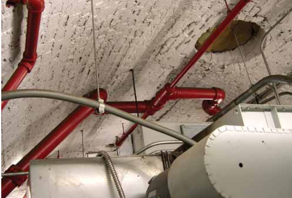
The clearance space for mechanical, electrical, telephone, and sprinkler equipment in Mechanical Room (108) is inadequate and does not meet current building codes. [JGWA, 2006]
