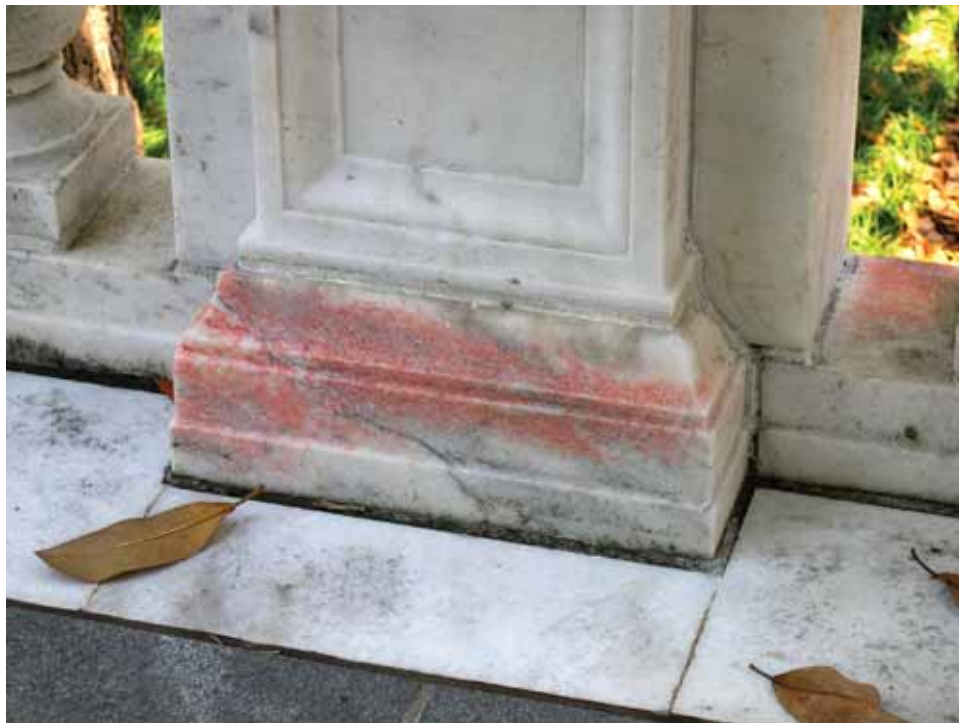
West Terrace. There is vivid orange “staining” along the bottom rails of the marble balustrades; this appears to be subsurface biological growth. [JGWA, 2006]
