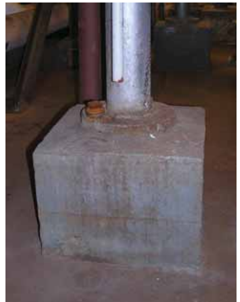
Figure 31: A steel pipe column with a concrete base found in the mechanical room below the north stairs.
