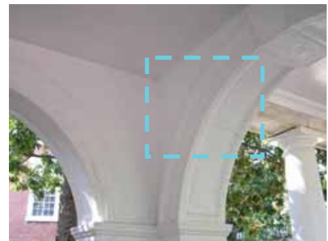
Figure 8: Transitional pavilion at east terrace -- arch cracking at lines of unbalanced thrust.
