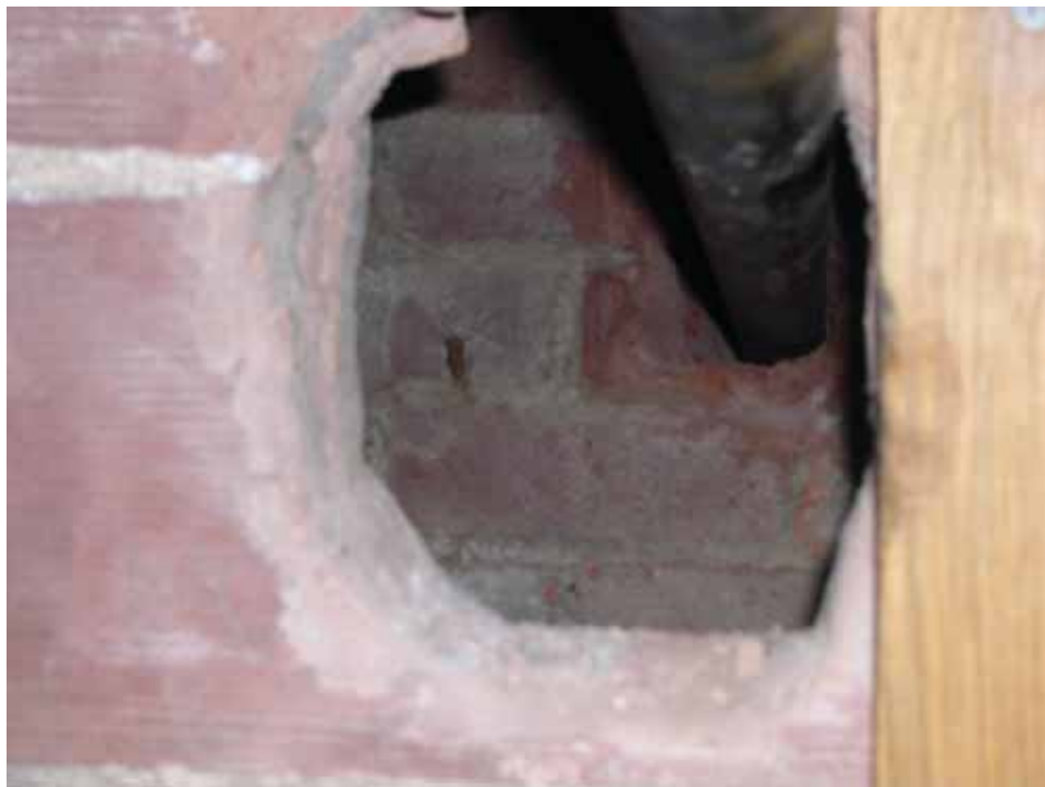
The Guastavino tile dome is visible within the Upper Gallery duct enclosure (left). Below, the outer dome is visible through a hole in the inner dome. [JGWA, 2006]
