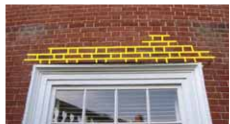
Figure 3: Above the windows in the cylindrical walls of the Rotunda the first few rows of brick have been repointed, likely from 1970s restoration and lintel replacement (altered mortar highlighted for clarity).
