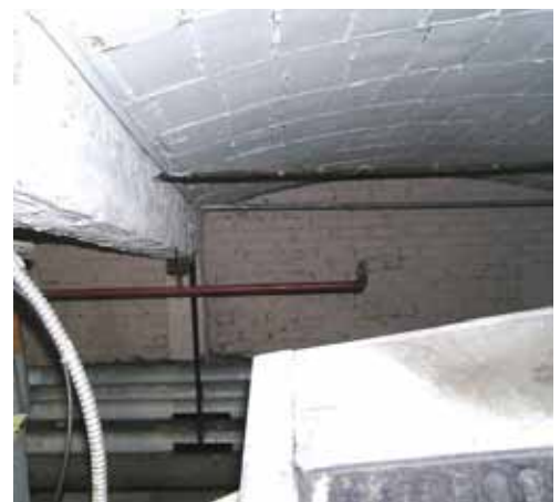
Figure 25: South Portico Roof Framing
