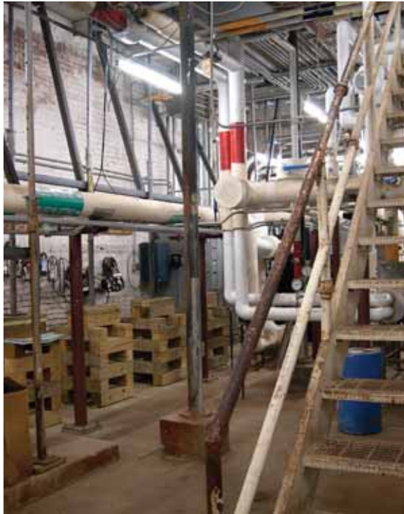
Generations of temporary shoring have been introduced in the Mechanical Room beneath the north portico to support the ceiling and terrace construction above. [JGWA, 2006]
