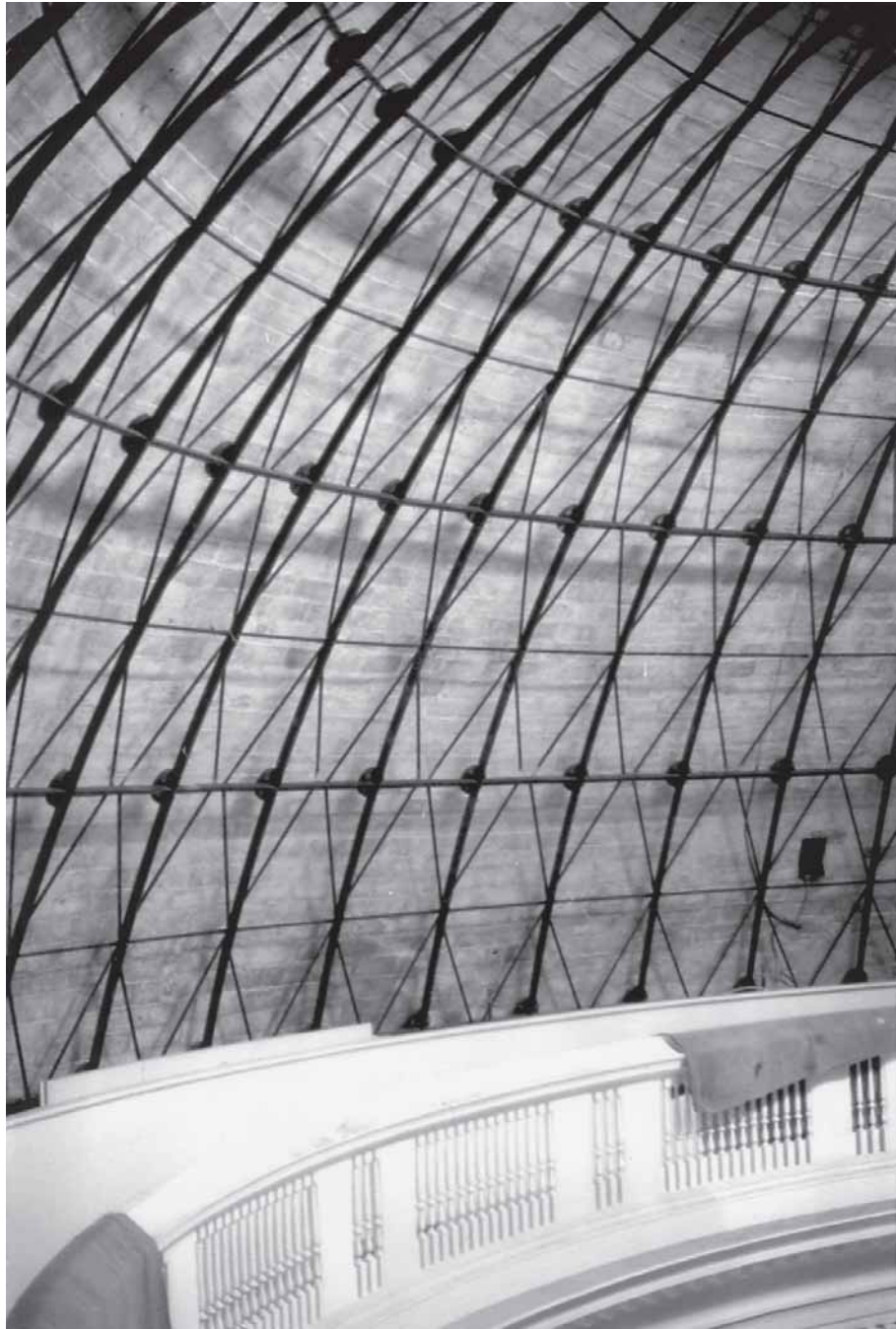
Figure 114. Framework for the Dome Room acoustical ceiling, October 10, 1975. [Special Collections, UVA]
