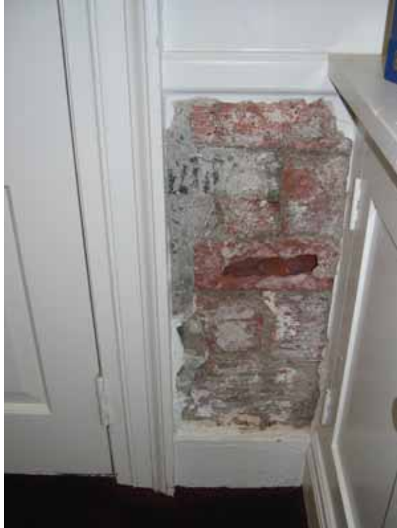
Southwest Wing, 124, looking southeast (top); section of exposed terra cotta tile in south wall of 124. [JGWA, 2006]
