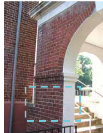
Figure 5: South end of East Arcade. Cracking and rotation in end pier.
