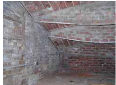
Figure 21: North Portico Attic Ribbed Vaulting
