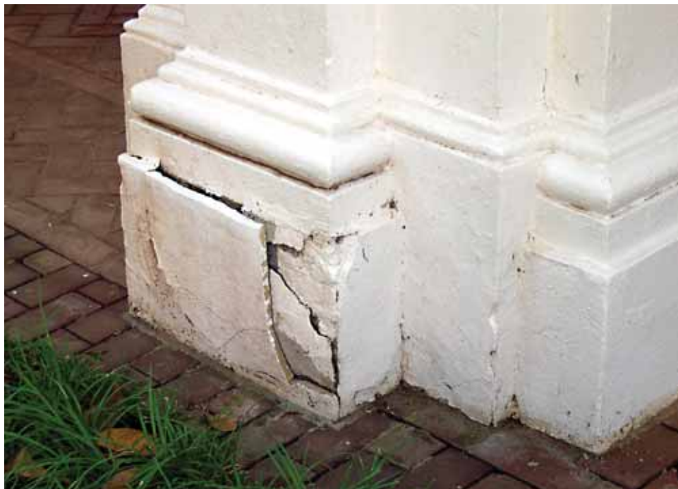
East Colonnade, West Elevation. The parging on the pier at the north end of the colonnade has seperated from the underlying brick construction. [JGWA, 2006]
