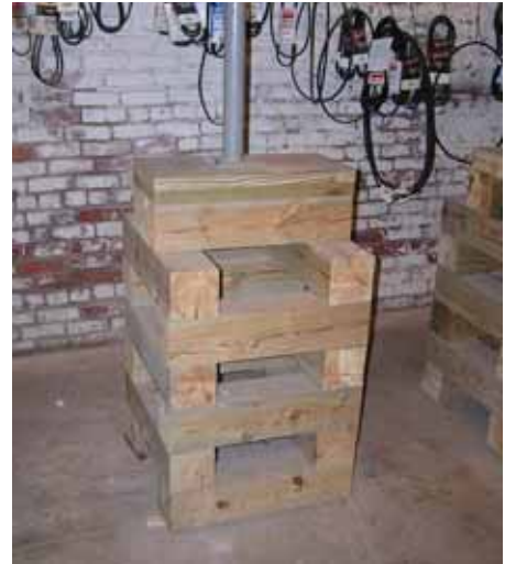
Figure 32: Extra columns were added to the space below the north stairs.
