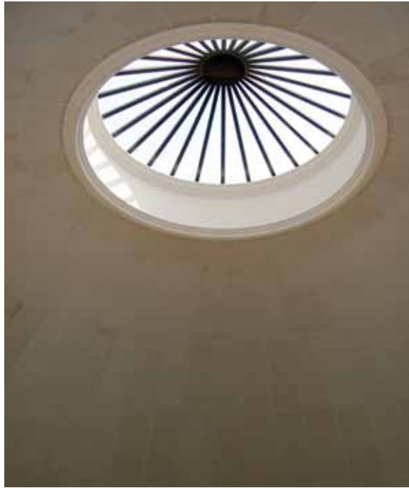
The glass of the skylight oculus is heavily abraded; from the interior, it appears to have a spider-web network of cracks. [JGWA, 2006]
