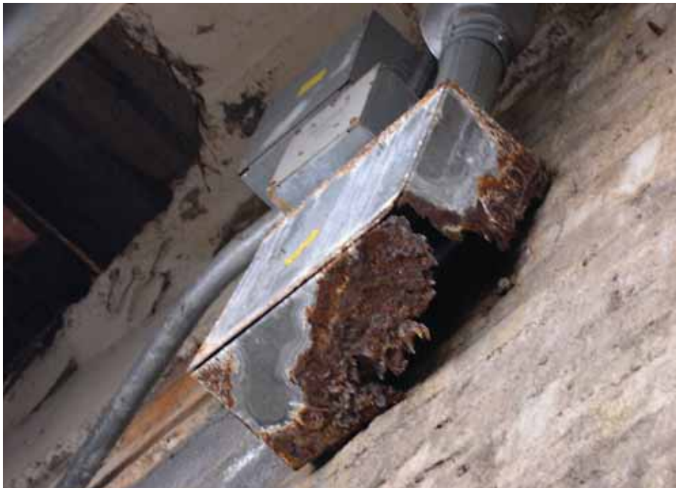
Significant problems with water infiltration in the Mechanical Room beneath the north portico have lead to advanced deterioration of equipment and fixtures. [JGWA, 2006]
