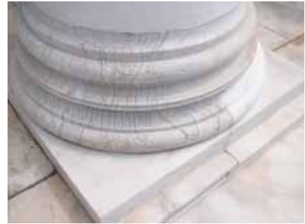
Figure 11: Many column bases have extensive surface cracking. The smooth white surface to the right is a replacement piece of stone, a Dutchman repair.
