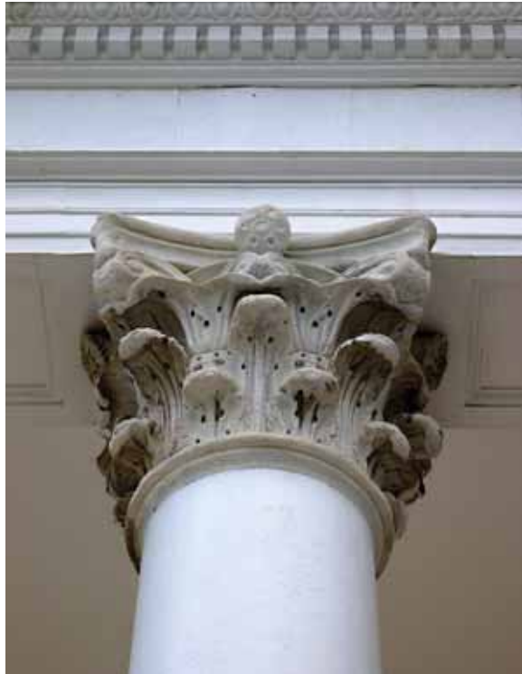
South Portico. The outer, exposed surfaces of the marble capitals are eroded. There are yellow-brown to black gypsum deposits on the inner, protected surfaces of the capitals. [JGWA, 2006]
