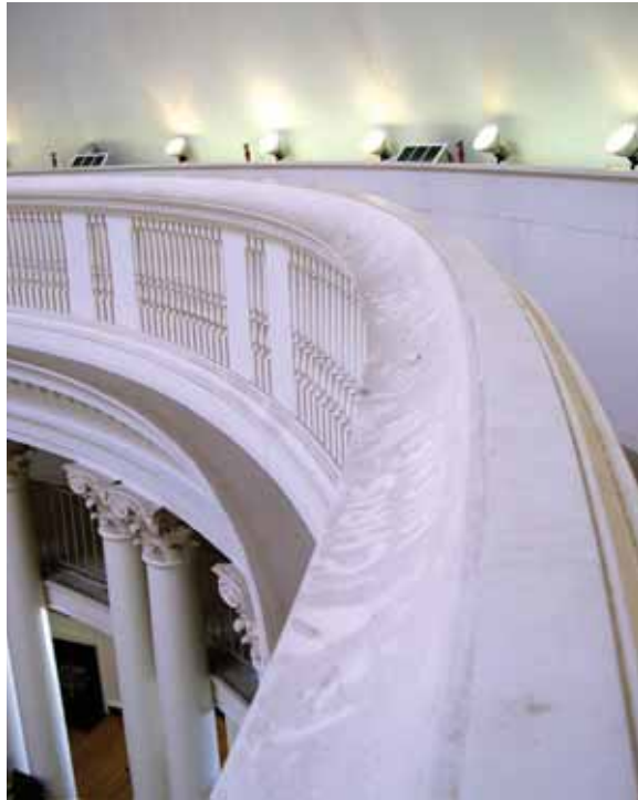
Prior to a December 2006 mold remediation project the Upper Gallery (C501) railing was covered with dust and mold growth. [JGWA, 2006]
