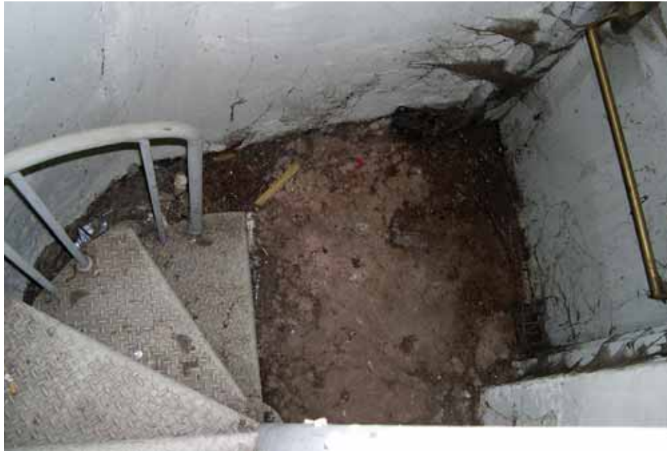
The emergency exit door (left) and floor slab (above) of the Northwest Fire Stair (C117) are dirty and covered with cob webs. The illuminated exit sign is not working. [JGWA, 2006]
