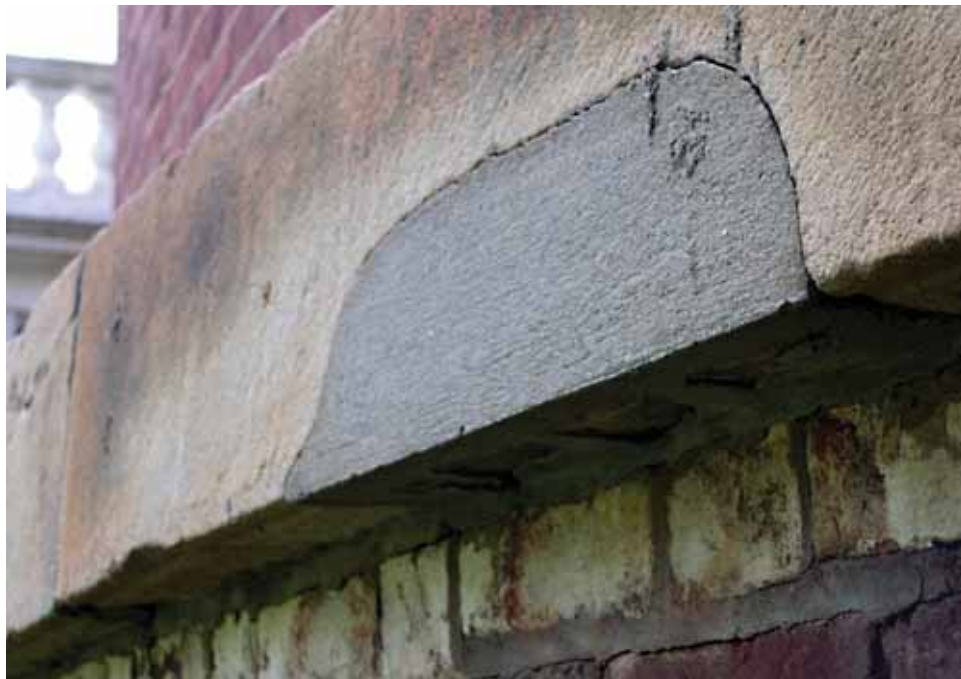
Rotunda, East Elevation. The sandstone water table is chipped and broken at its outer face, overhanging edge, and butted joints. A large brick-and-mortar repair to the sandstone beneath the center window has failed. [JGWA, 2006]
