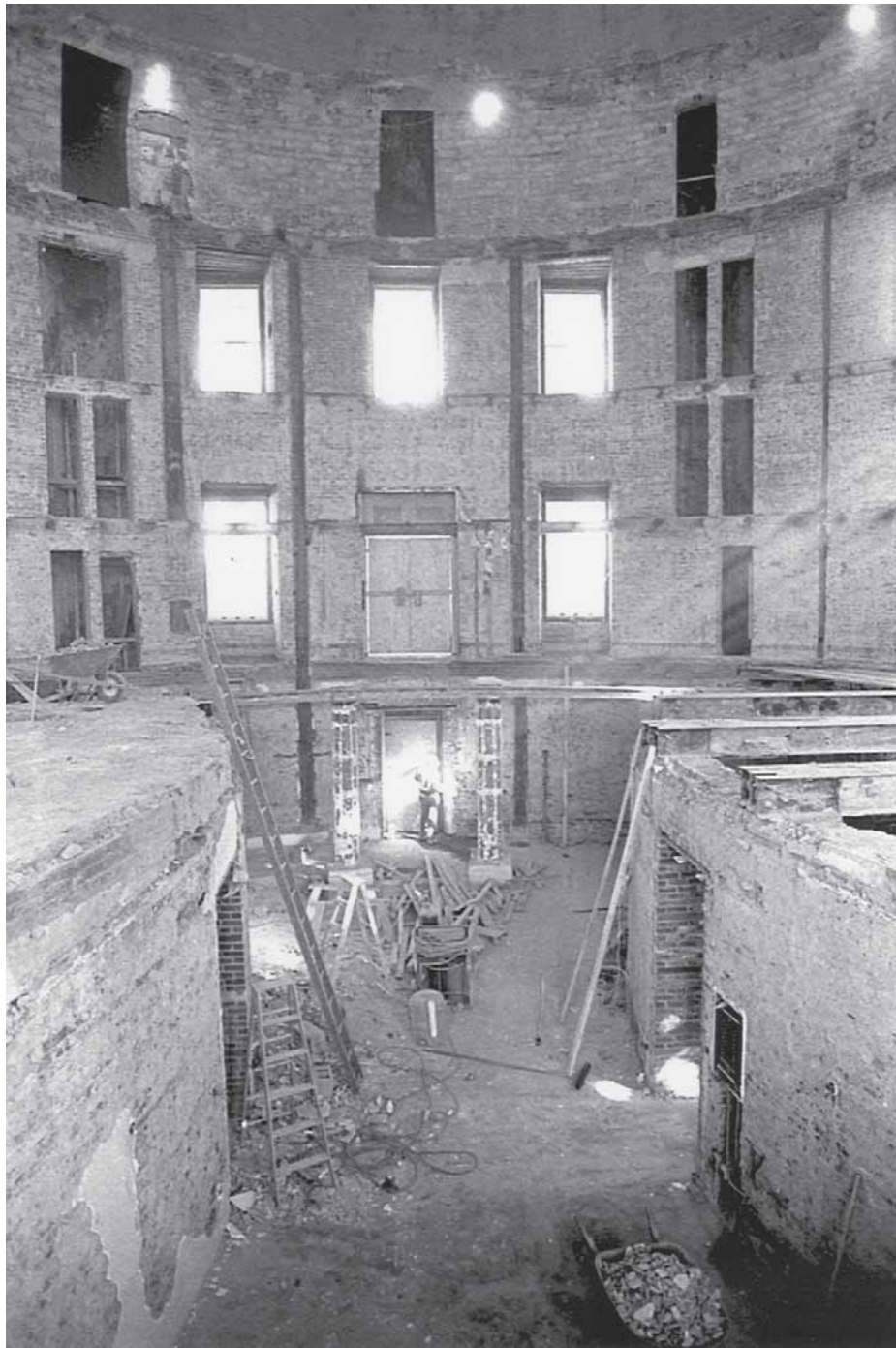
Figure 110. The interior of the Rotunda during demolition, January 30, 1974. The basement walls to the right and left survive from the original construction. [Special Collections, UVA]
