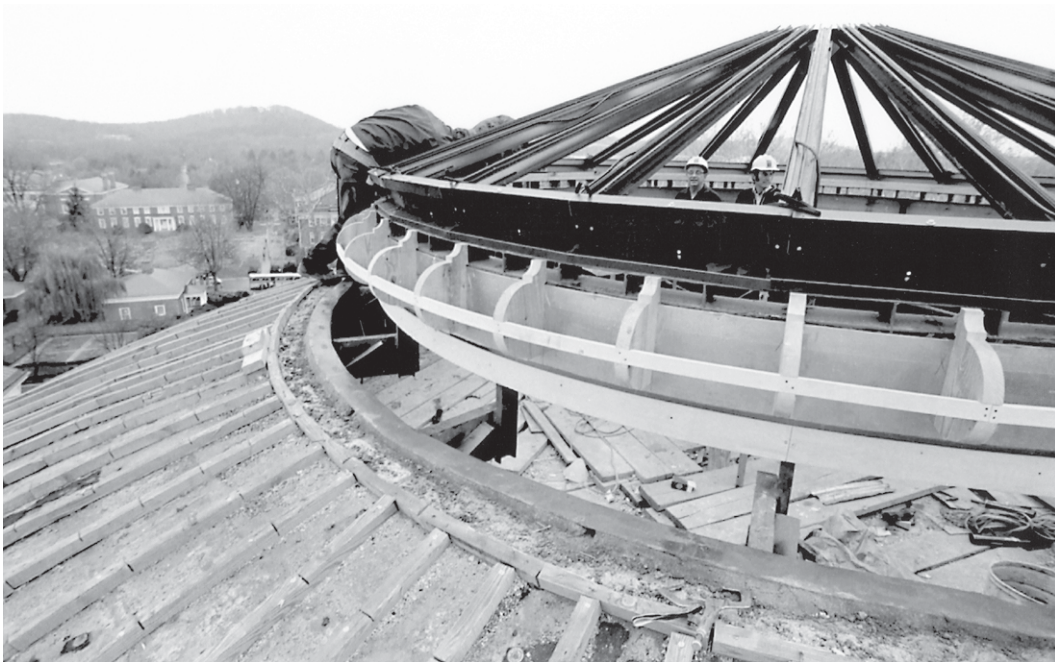
Figure 112. The new extruded aluminum skylight frame during the reconstruction of the skylight, November 18, 1974. [Special Collections, UVA]
