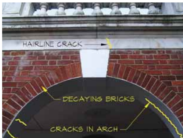
Figure 9: North end of west terrace masonry cracking and deterioration.
