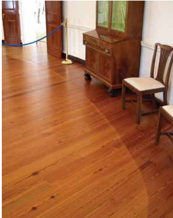
The floor finish in the President's Reception Room (Upper West Oval Room 201) is discolored as a result of UV degradation. This was made apparent by the removal of the large oval rug that was located in the center of the room. [JGWA, 2006]
