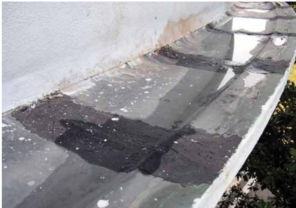
Rotunda, West Elevation. The seams in the copper sheet metal gutter above the intermediate cornice have been repaired with fiber-reinforced elastomeric seam tape. The tape is failing from long-term exposure. [JGWA, 2006]
