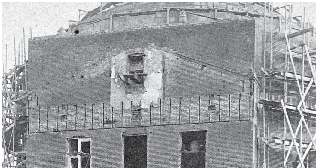
Detail of Figure 75. Construction evidence revealed in this image indicates that the upper section of the entablature did not wrap around onto the north elevation; rather, Jefferson placed a full pediment on this elevation.
