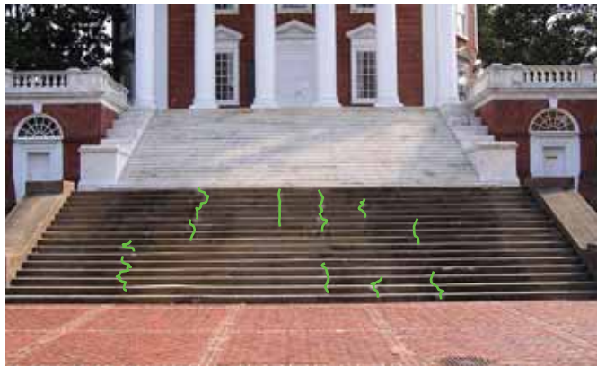
Figure 17: The north stairs approaching the Rotunda have several cracks and patches.
