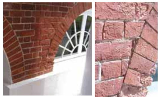
Figure 12: The bricks between the arch windows show significant material decomposition corresponding to areas of increased water penetration.
