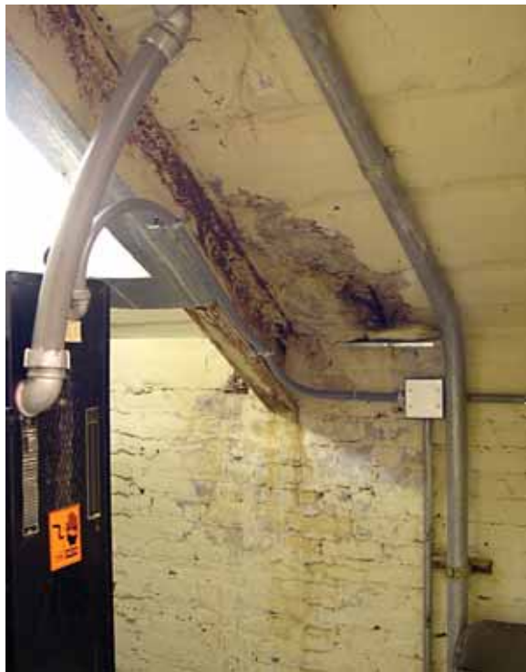
The exposed steel beam supporting the sloped concrete ceiling of Elevator Machine Room (110A) has significant surface rust. The rust is more advanced at the beam's bearing point in the north wall. Galvanized sheet metal and acrylic glazing have been installed above the elevator machinery to protect the equipment from water infiltration occurring in the north portico steps above. [JGWA, 2006]
