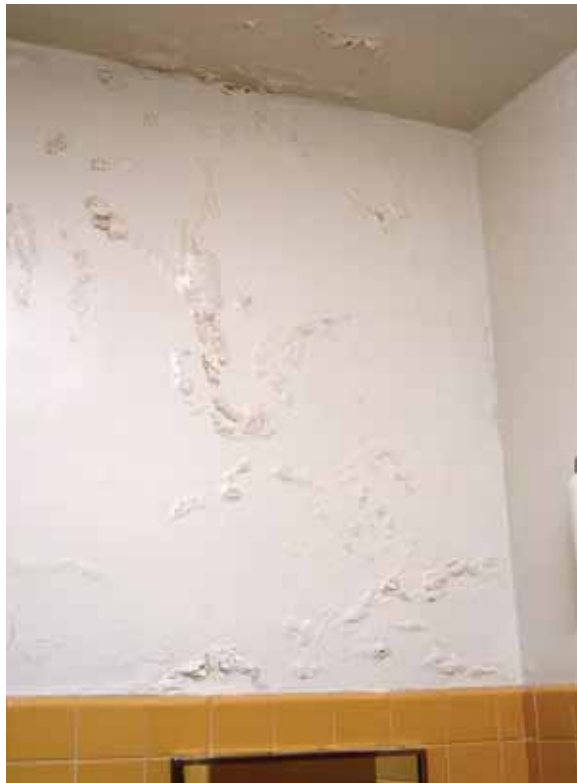
The plaster wall and ceiling surfaces in the northeast corner of the Men's Toilet Room (T113) are badly blistered. The plaster is friable, and the painted finish is peeling as a result of water infiltration. [JGWA, 2006]
