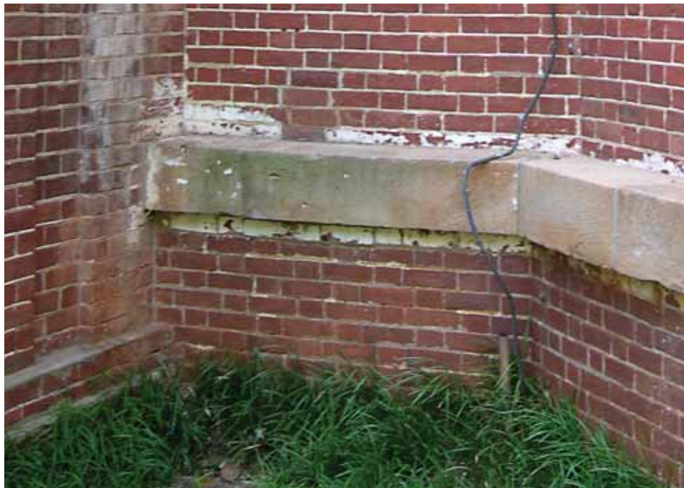
Rotunda, East Elevation. Evidence of paint coatings remains on the brickwork above and below the stone water table at the south end of the wall. The lightning down-conductor cable has been pulled loose from the wall, and there are lime-run (calcium carbonate) deposits on the brickwork. [JGWA, 2006]
