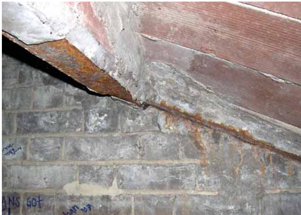
The steel plates and ledgers for the ribs of the tile vaulting in the North Portico Attic (401) are rusting; minimal delamination of the steel is occurring. [JGWA, 2006]
