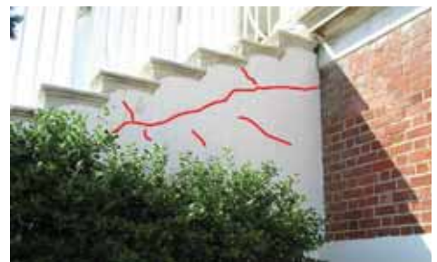
Figure 14: A sloping crack running below the stairs was observed on the east elevation.
