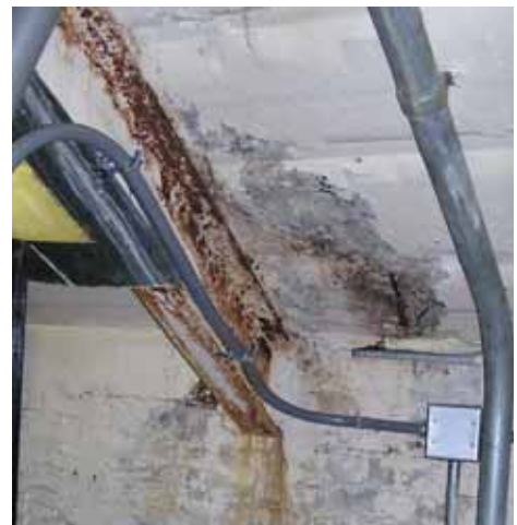
Figure 33: Due to water infiltration, the steel support of the North Stair is corroding. The structure is exposed in Storage Rooms No. 109 and 110.
