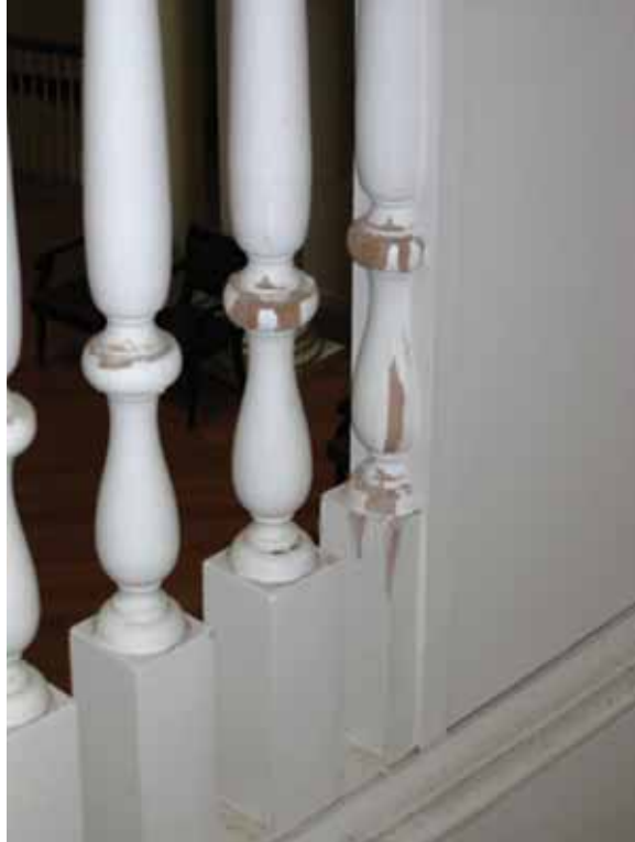
The paint on the balusters of the Upper Gallery (C501) railing is peeling; the wood substrate is exposed. [JGWA, 2006]
