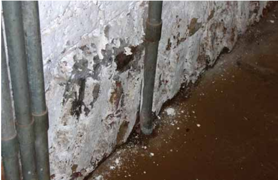
There is rising damp in the masonry construction of the north and east walls of Mechanical Room (108). The painted wall finish is peeling, and efflorescence has formed on the masonry. [JGWA, 2006]
