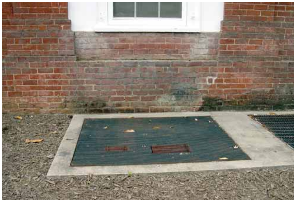
Northeast Wing, North Elevation. The painted surfaces have chalked and stained the brickwork. There is dark biological staining on the brick near the rusted areaway grates. [JGWA, 2006]
