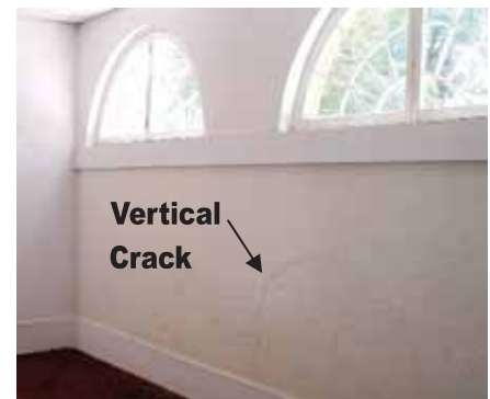
Figure 13: South terrace corridor – interior cracking below windows.
