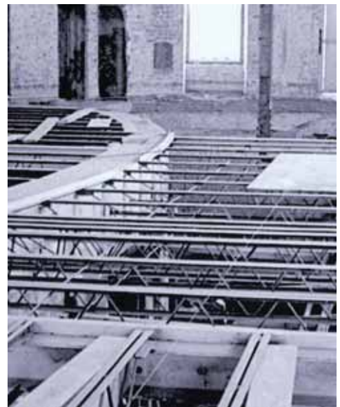
Figure 1: In the 1970s the first and second floor framing was replaced with steel beams and open-web steel joists. (Picture from 1970 Restoration provided by John G. Waite Associates)
