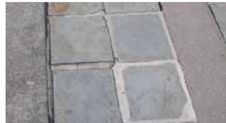
Figure 16: The terrace on the north side has obviously been repaired several times and remains in a deteriorated state.
