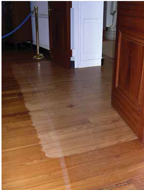
Floor sanding in the Center Hall (C202/C203) was continued through the east entry of the President's Reception Room (Upper West Oval Room 201). This refinishing work and the perimeter abrasion from a large oval rug have caused discoloration and uneven wear in the heart pine flooring. [JGWA, 2006]
