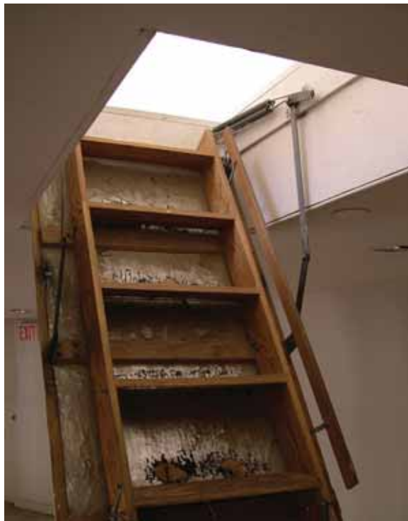
Middle Gallery C401).[JGWA, 2006]The folding ladder stairs providing access to the Upper Gallery of the Dome Room (C501) are of a residential character and quality. The stairs and the reveals of the stair openings are dirty, worn, and abraded. [JGWA, 2006]
