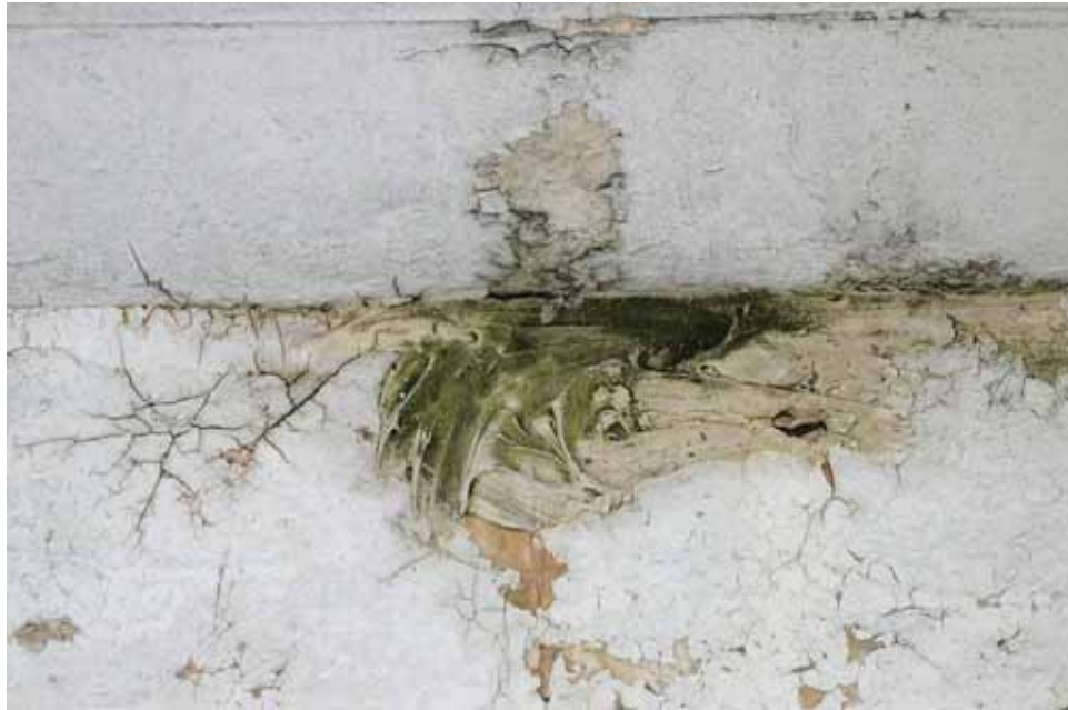
Rotunda, Roof. Inadequate attempts have been made to cover areas of exposed sheet metal on the steps at the base of the dome with smeared sealant. The sealant is supporting the growth of algae.[JGWA, 2006]
