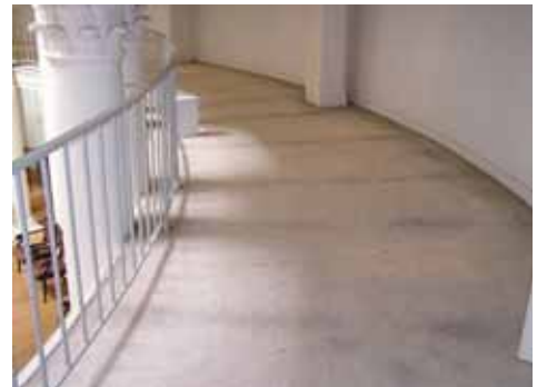
Figure 30: Radiating black stains are visible on the carpet in the middle gallery.
