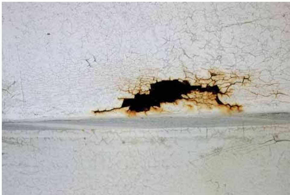
Rotunda, Roof. The painted finish on the terne-coated roofing of the dome is crazed and peeling; the underlying sheet metal is rusting through. [JGWA, 2006]
