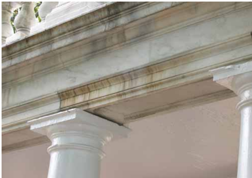
East Colonnade, East Elevation. The marble entablature and soffit have been soiled and stained by rainwater run-off, originating in the terrace construction above. [JGWA, 2006]
