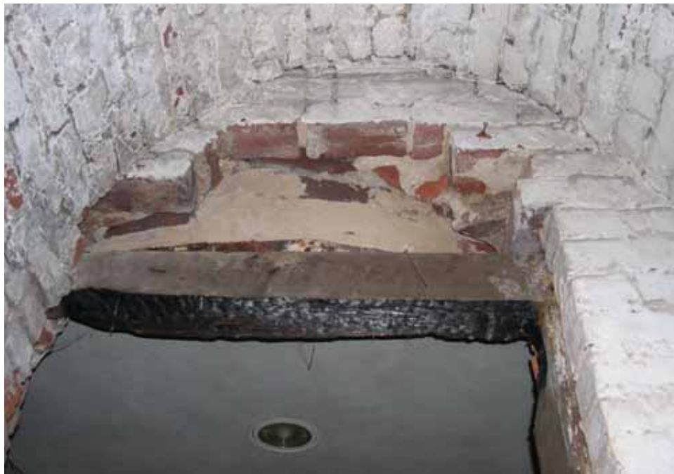
Closet/Passage 105, charred lintel at north opening. [JGWA, 2006]
