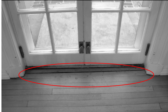
Wide gaps at floorboards (Item 2).
