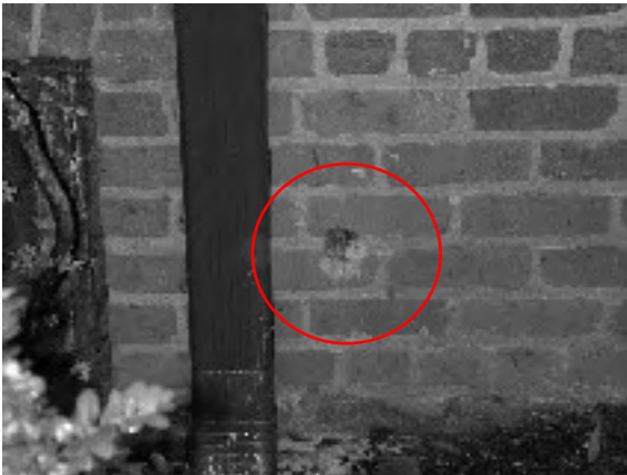
Pipe in wall beside downspout (Item 2).
