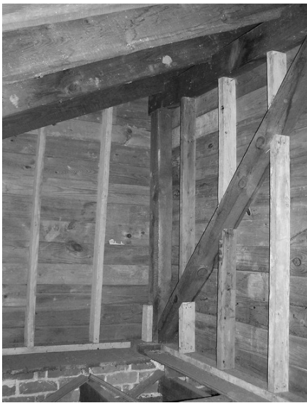
Photo 5: The knee wall supporting the roof above the portico.
