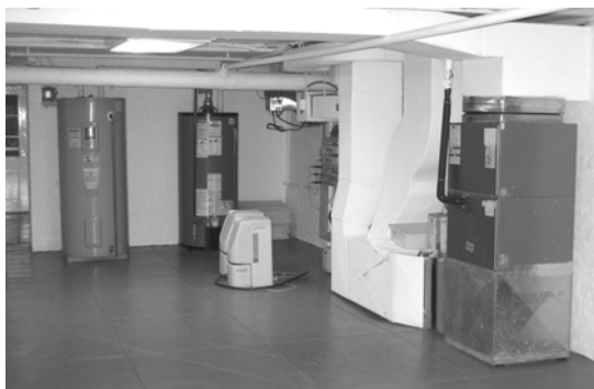
Water heaters in basement (Item 1) AH#1, floor-mounted dehumidifiers also shown.
