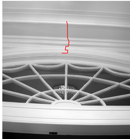
Separation of wood joints and cracked plaster (Item 3).
