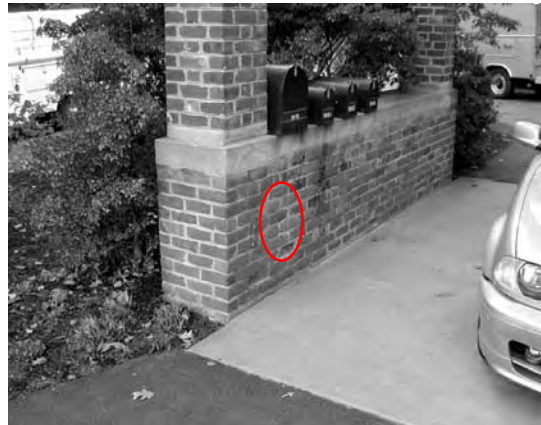
Brick deterioration on porte cochere cheek (Item 3).
