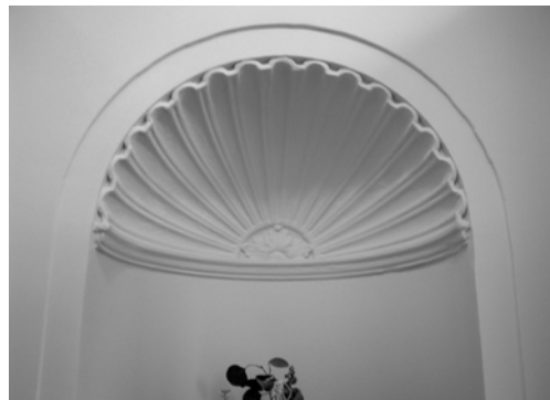
Paint build - up on clam-shell detail (Item 8).
