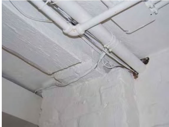
Photo 14: The bottom of the beam in Room B02 is notched near the support.
