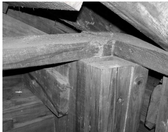
Photo 2: Built up of wood column at the corner of the portico roof.
