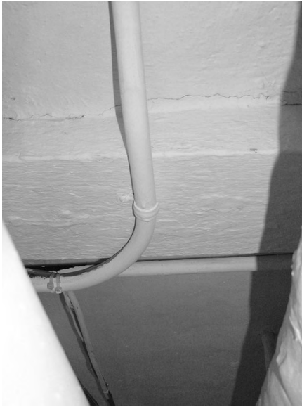
Photo 13: Paint cracking between first-floor girder and ceiling indicative of movement.
