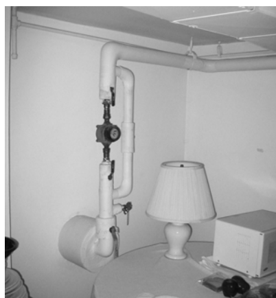
Domestic water service and meter (Item 1).
