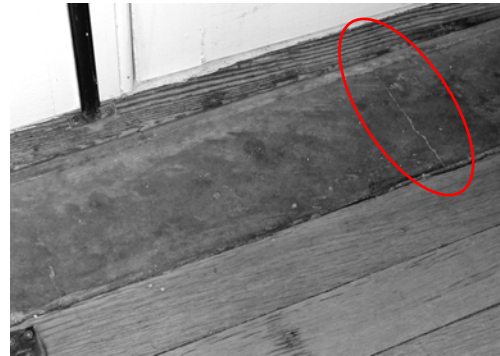
Cracked concrete threshold (Item 5).
