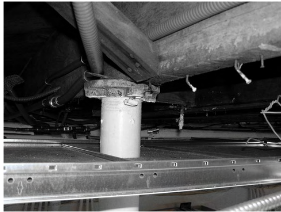
Photo 18: Pipe column tenuous top connection.
