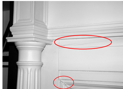
Open joints and cracking of wood (Items 8 & 9).
