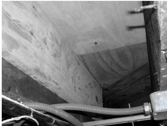
Photo 19: In Room B01 a new wood sister and plywood floor replacement address apparent deterioration over the window in the northeast corner.
