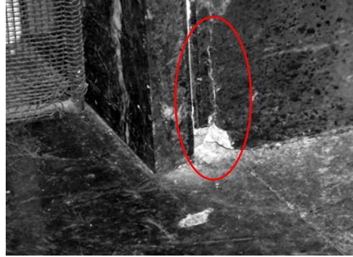
Crack in firebox masonry (Item 7).
