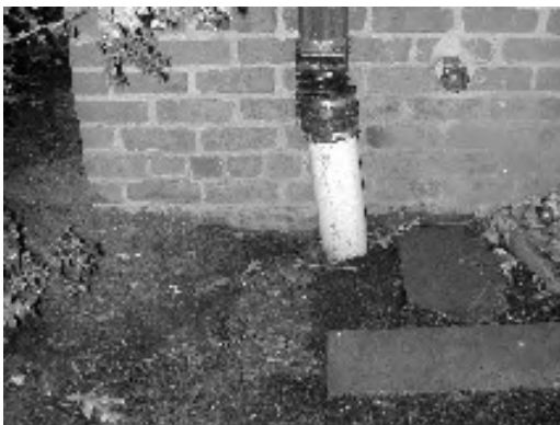
Depressed grade around downspout boot (Item 1).
