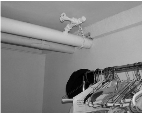
Photo 15: The 8"x10" first-floor girder between Rooms B08 and B10 suffers from several service penetrations.
