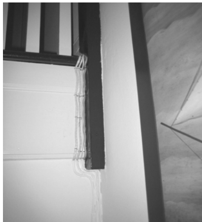
Surface-mounted cabling at of Stair 119 (Item 2).
