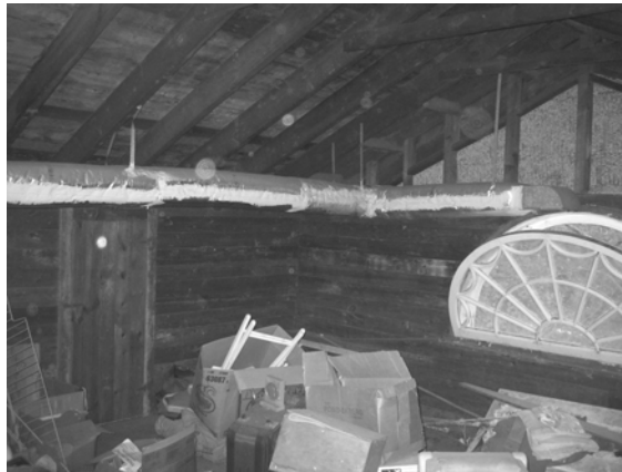
Outside air intake duct in Attic 304 (Item 6).
