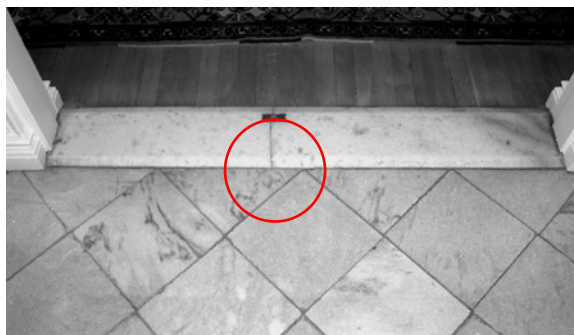
Cracked marble threshold (Item 2).
