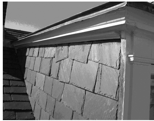
Loose slates at dormer side-wall (Item 4).
