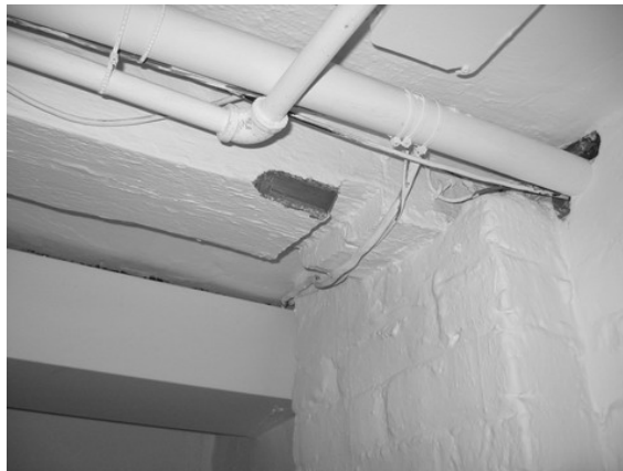
Photo 26: Probe 3 wood sample from 8"x10" girder in Room B02 located adjacent to existing notch.
