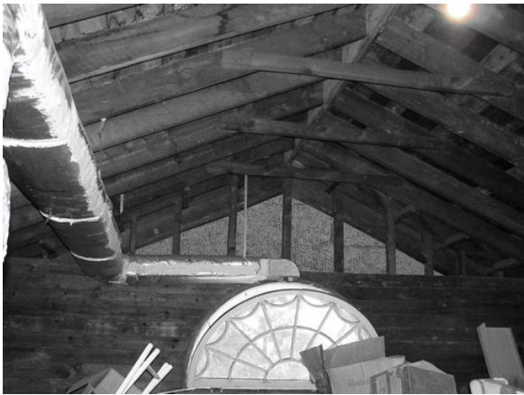
Photo 3: The roof structure above the portico (Room 304) with the absence of the 4x6 post indicated in the original drawings.
