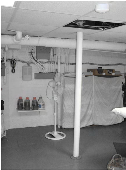
Photo 17: Pipe column in Room B01 below first-floor wall between kitchen and pantry.
