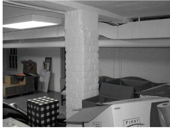
Photo 12: A brick masonry pier in the center of Room B02 supporting the timber girder above.
