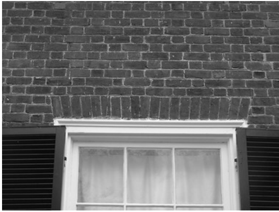
Shallow flat arch at exterior wall openings (Item 3).
