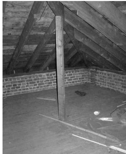
Photo 4 (right): A 4x4 post supporting the hip beam.
