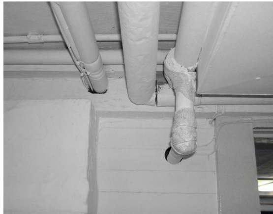
Photo 16: Several penetrations made through the 8"x10" first-floor girder between Rooms B09 and B04.
