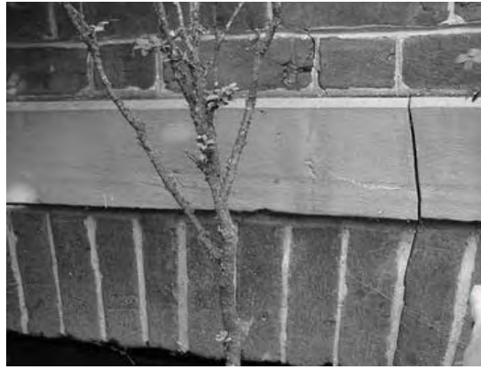
Flat arch and stone watertable cracking (Item 3).
