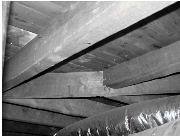
Photo 6: The shallow hipped roof construction of the center section of the roof surrounding the skylight.
