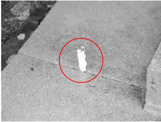
Deteriorated joint in portico steps. Knife blade buried in joint is 4" long (Portico, Item 1).
