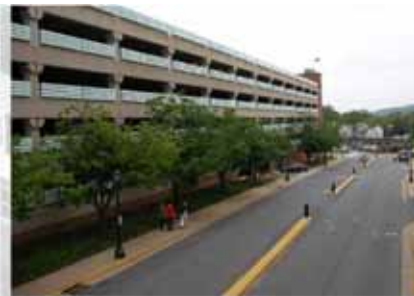
VIEW OF EAST GARAGE
