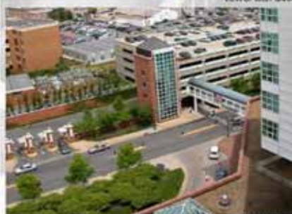
VIEW OF HOSPITAL DROP OFF PLAZA
