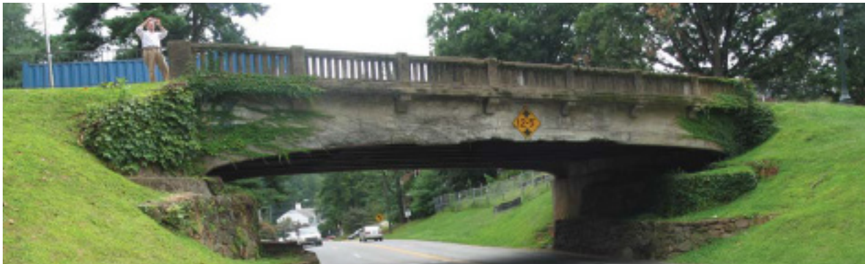
McCormick Road Bridge
