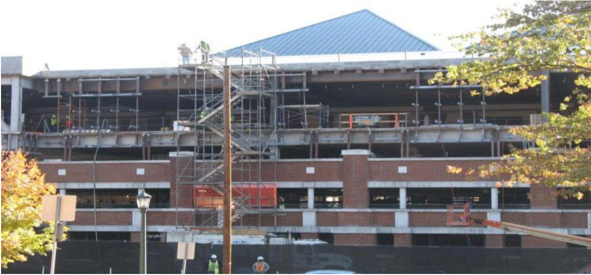
Progress of Construction
