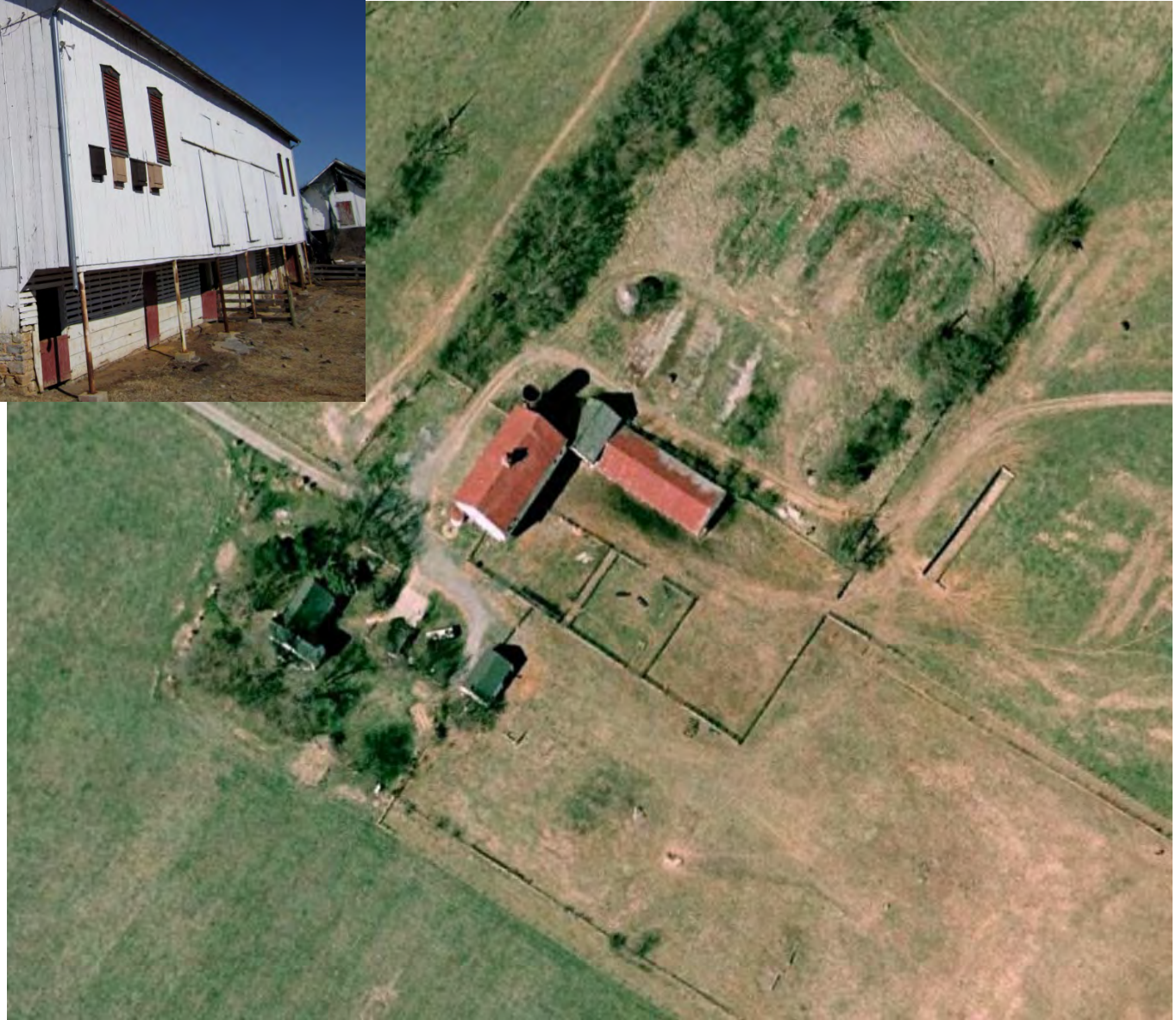
Relocation of Maintenance Facilities to Garver Farm
