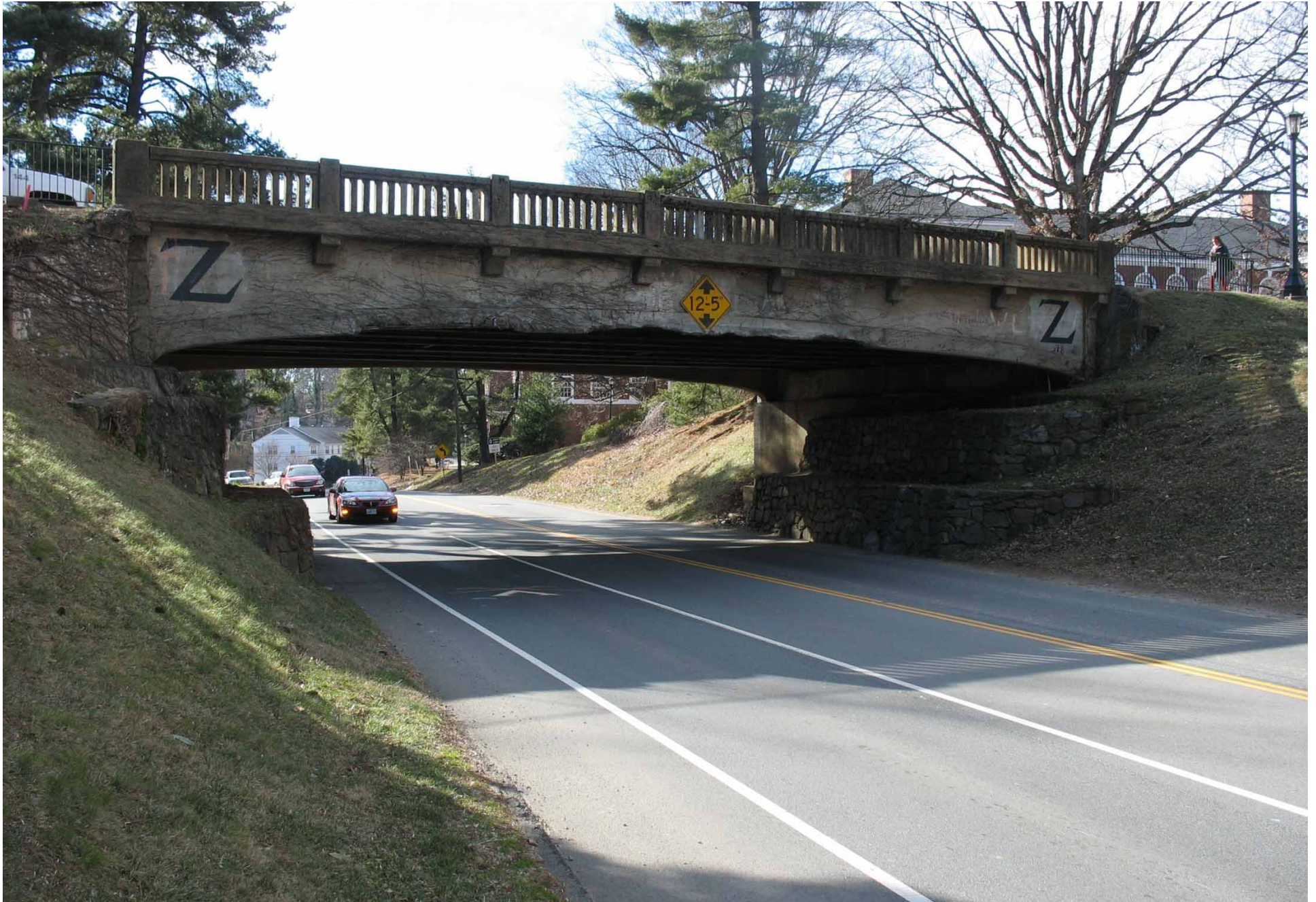
McCormick Bridge from Emmet Street
