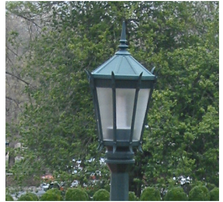
General Path Lighting, King Edgewater K-56 metal halide or LED luminaire on 12' cast aluminum or cast iron octagonal pole, Rookwood shutter green, pebbled lenses
