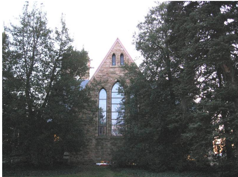
Figure 3.6 North façade. (QE|A, 2006)
