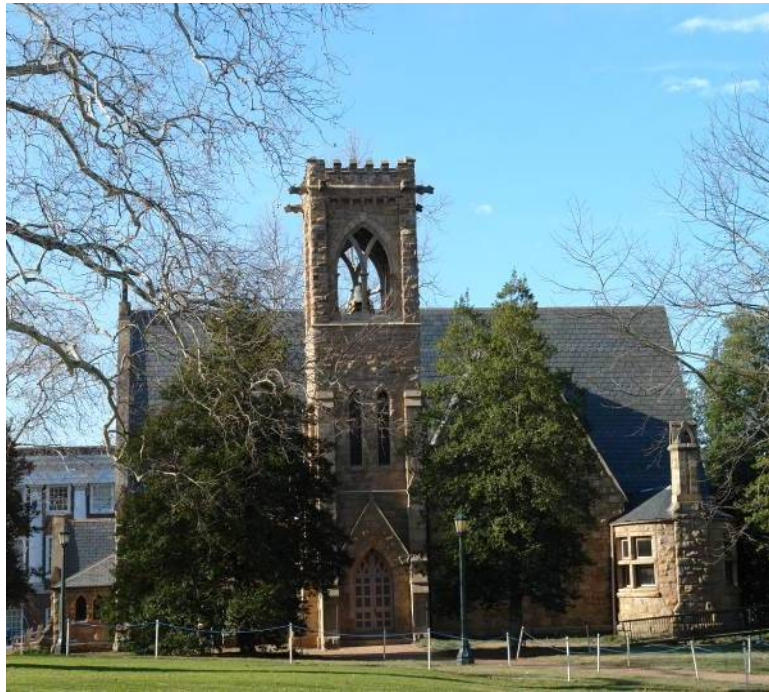
Figure 3.4 East façade. (QE|A, 2006)
