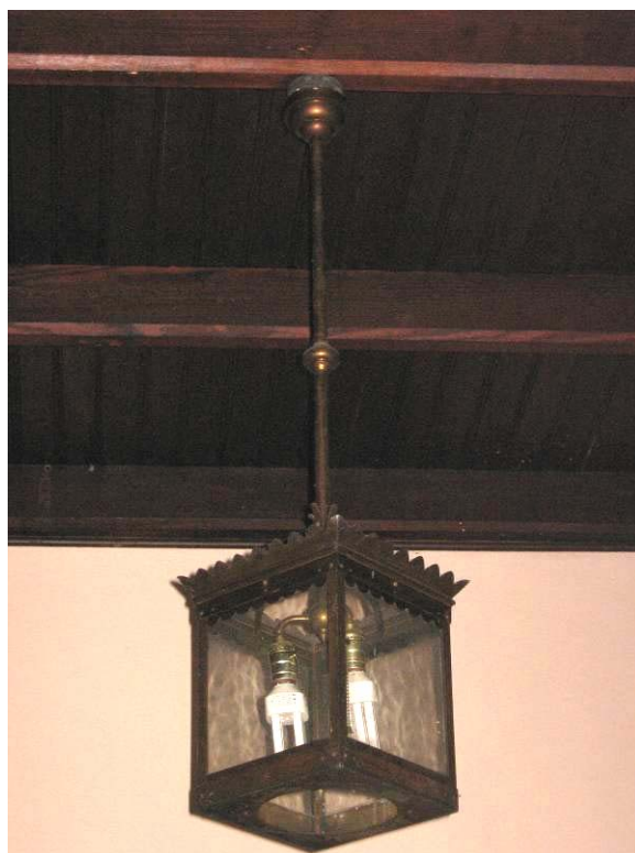
Figure 3.93 Pendant light fixture in the vestry. (QE|A, 2006)
