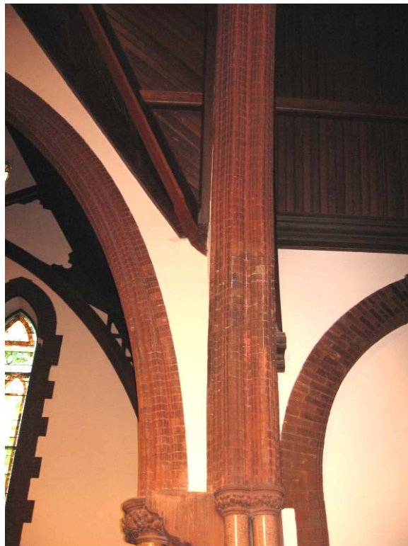
Figure 3.51 Detail of the pressed brick arches at the east transept. (QE|A, 2006)
