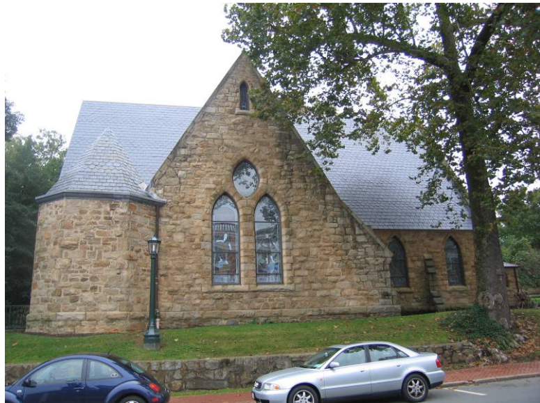
Figure 3.7 West façade. (QE|A, 2006)
