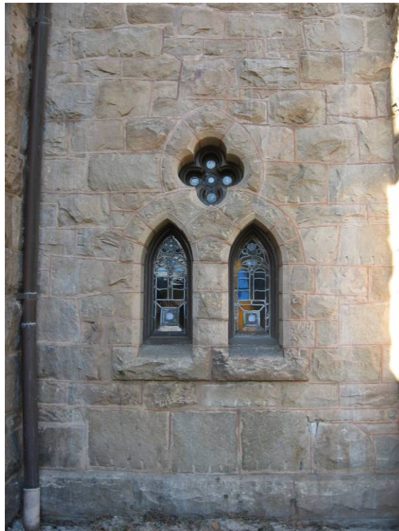
Figure 3.3 Detail of lower south façade of bell tower. (QE|A, 2006)
