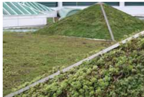
UVA HOSPITAL GREEN ROOF
