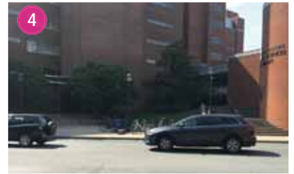
PINN HALL ENTRY AND TERRACE
