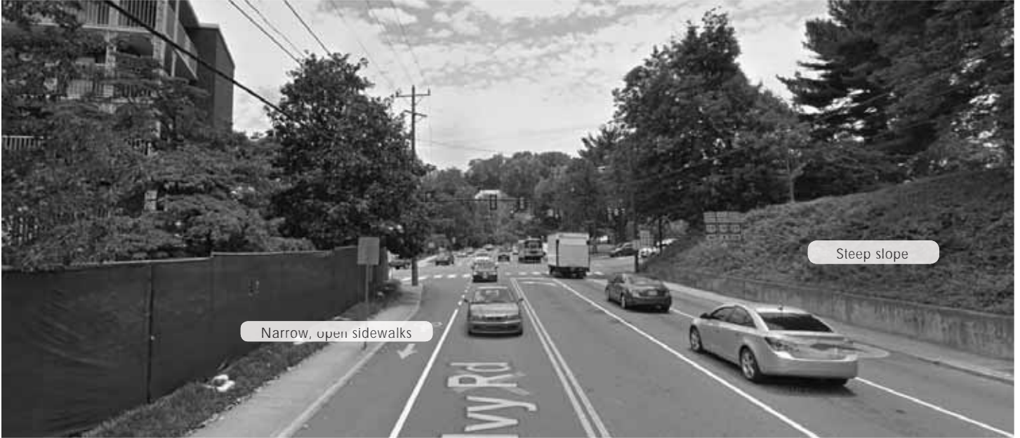
IVY ROAD—EXISTING CONDITION
