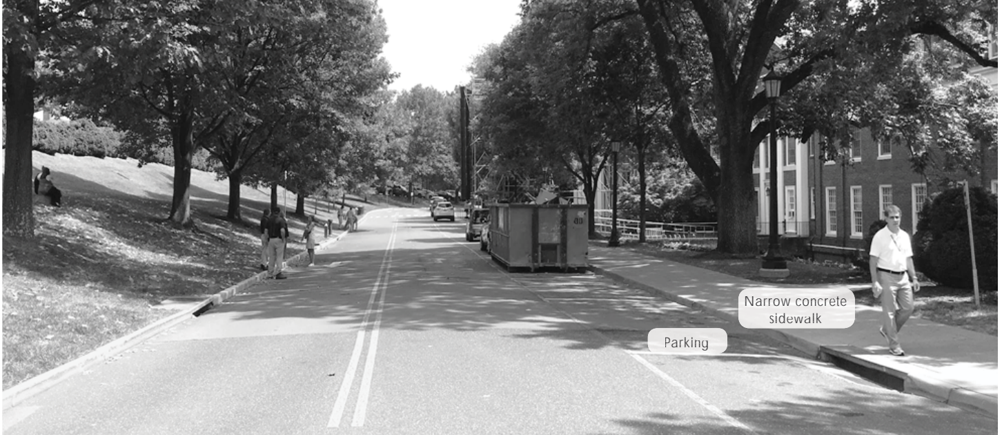
HOSPITAL DRIVE-EXISTING CONDITION
