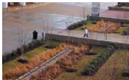
BIOFILTRATION AT ARENA
