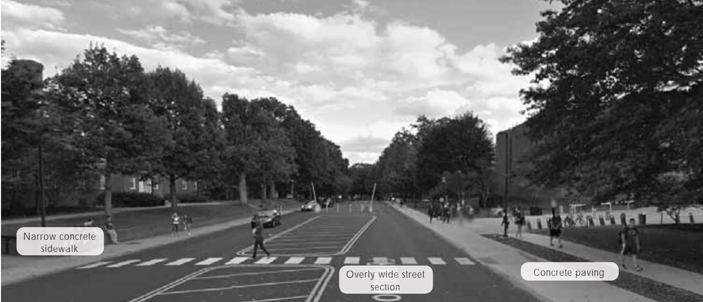
MCCORMICK ROAD-EXISTING CONDITION
