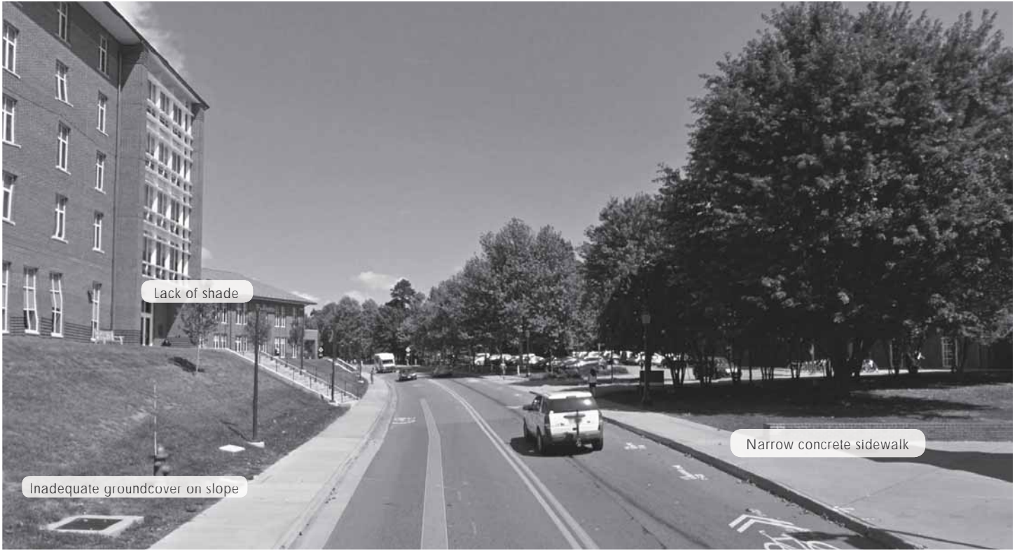
ALDERMAN ROAD-EXISTING CONDITION
