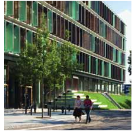
CROSSING AND ACCESS
