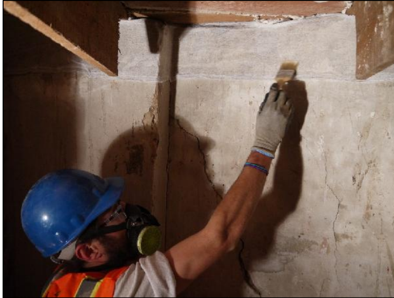
Figure 3: Adhering cheese cloth to tissue paper with B72 solution.
