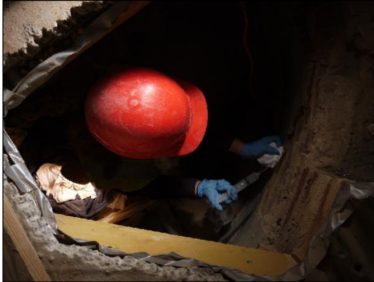
Figure 7: Injecting B72 solution between plaster and brick, space above ceiling.
