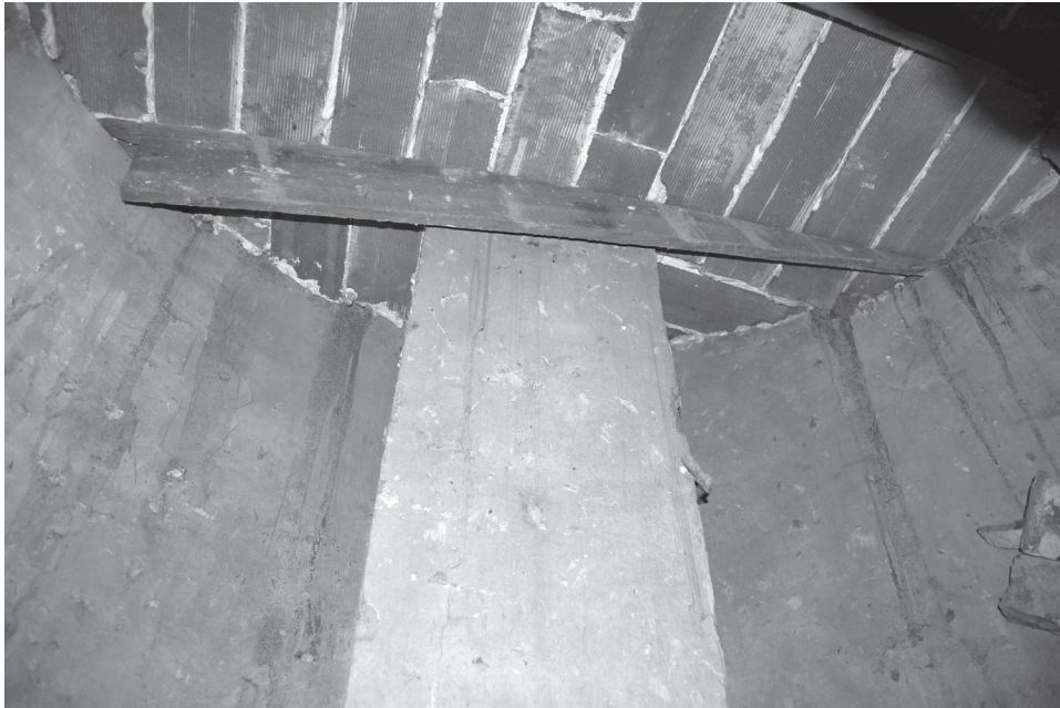
Figure 49. Center flue and circa 1897 Guastavino tile ceiling (above) and view up through center flue (left). [JGWA, 2014]
