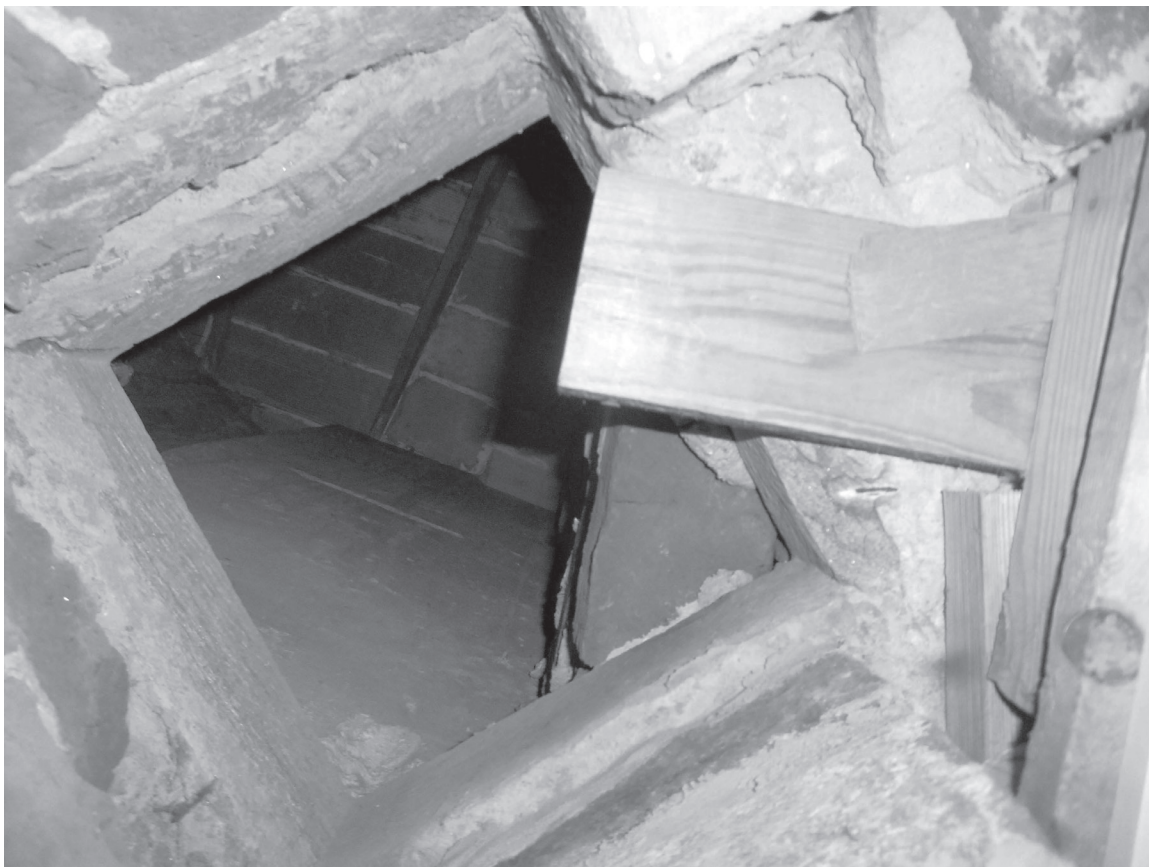
Figure 36. View up through one of the fire boxes discovered in the 1976 work, showing a glimpse of the large cavity above, partially finished in plaster. [JGWA, 2013]
