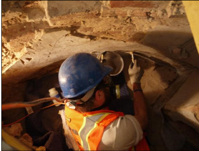
Figure 5: Applying tissue paper with B72 solution, space above ceiling.
