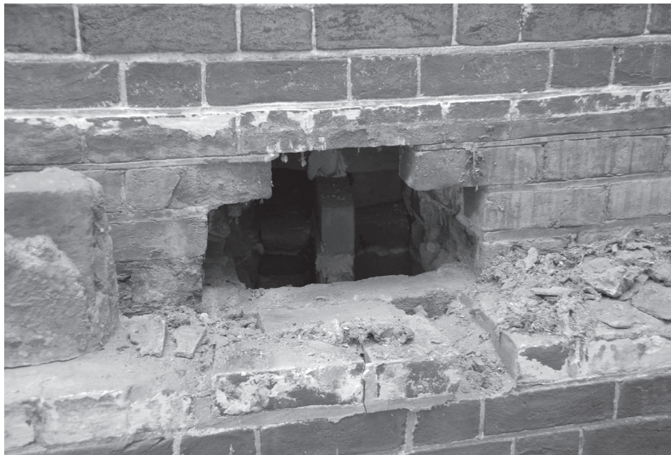
Figure 37. The stone water table on the east facade of the Rotunda drum, adjacent to the chemical hearth, was removed to reveal the fresh air intake for the chemical hearth at the north end of the east oval room. The lower edge of the stone water table, seen in the upper photograph, was chipped out to accommodate the fresh air intake. [JGWA, 2012-2013]
