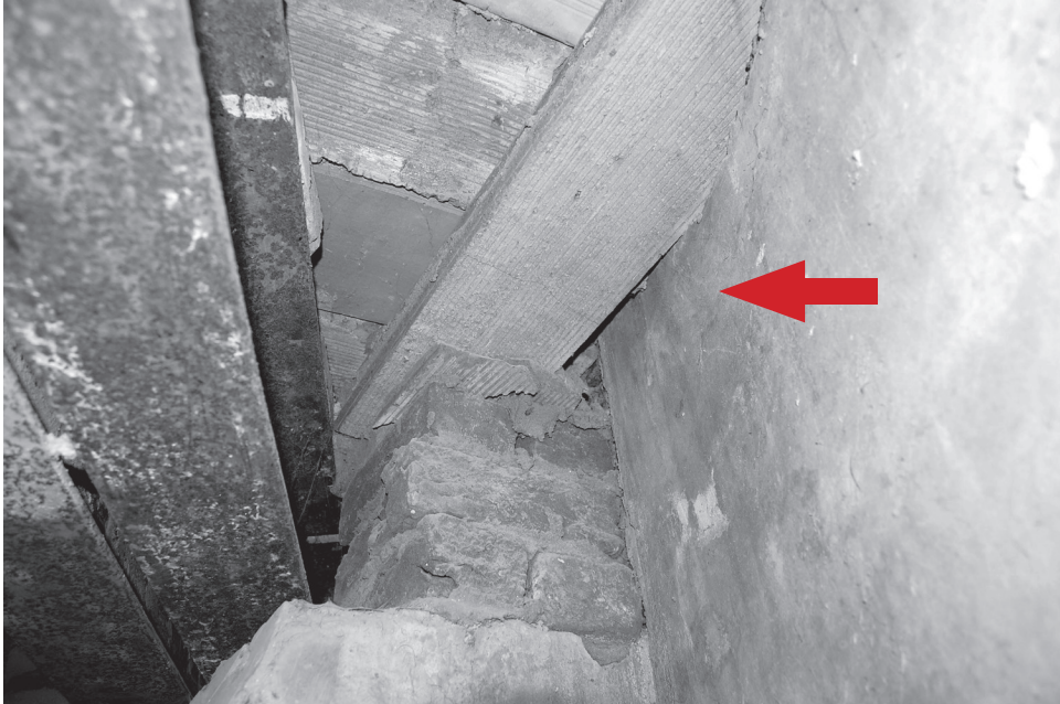
Figure 53. The plaster wall finish of the chemical hearth appears to continue above the second floor level. [JGWA, 2013]
