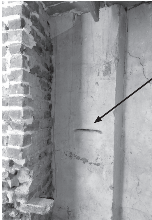
Figure 46. (Left) West pier with slit for damper control of the flue beyond. [JGWA, 2014]
