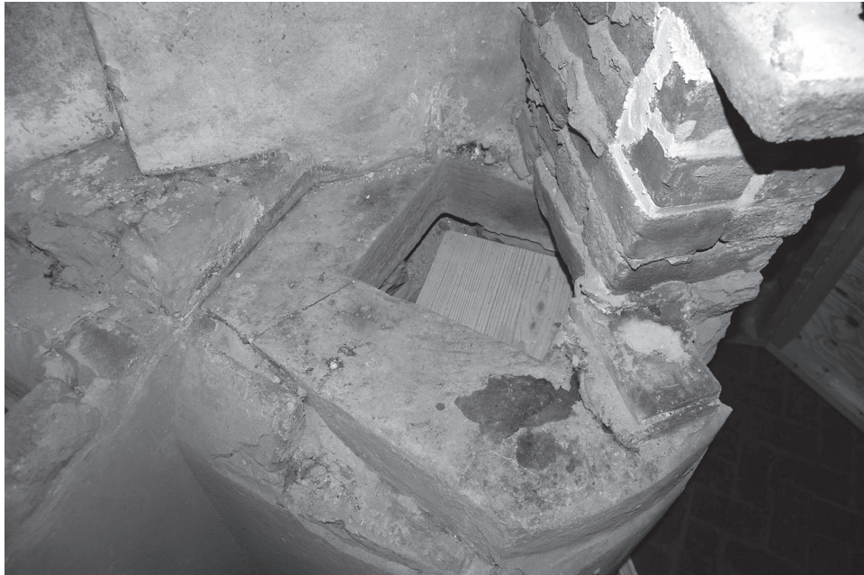
Figure 52. West station counter. A fragment of the brick infill wall construction that concealed the chemical hearth can be seen bearing on the stone counter top. [JGWA, 2014]
