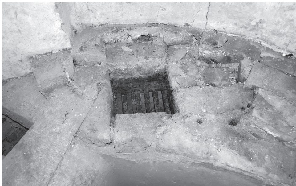
Figure 47. (Below) West intermediate station with cast-iron grate. [JGWA, 2014]
