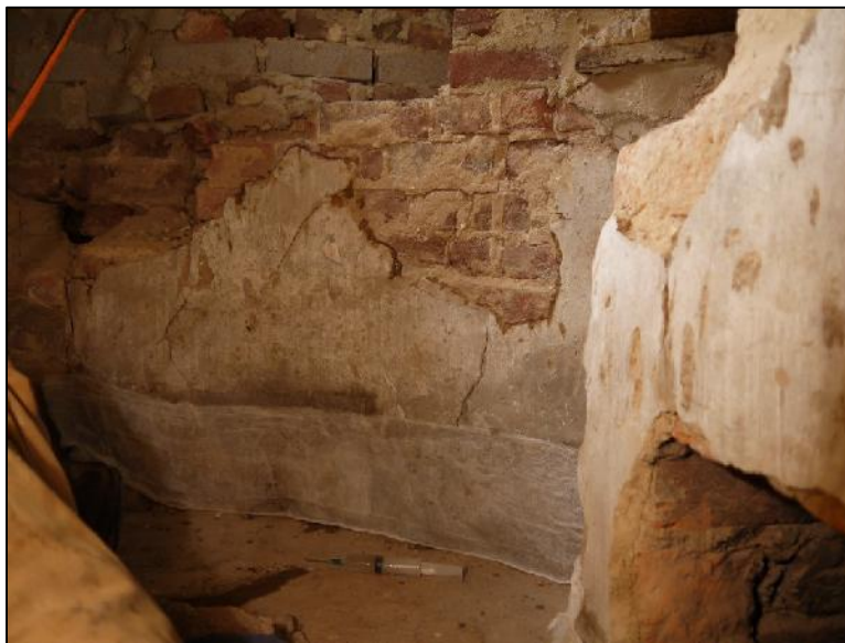
Figure 8: Plaster above ceiling after adhesive injections and application of facing.
