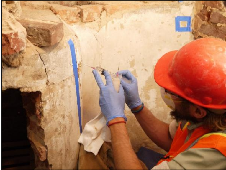
Figure 1: Additional B72 injections to the hearth plaster.
