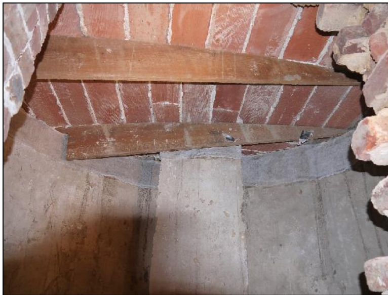
Figure 4: View of completed facing application below the Guastavino ceiling tiles.
