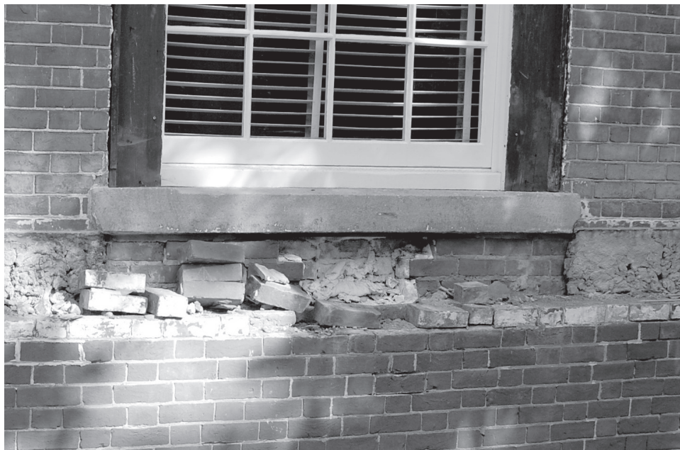
Figure 38. The stone water table on the east facade of the Rotunda drum. The water table at the center window, behind the chimney mass, was removed to investigate possible air duct locations. A cutout in the stone water table, seen in the upper photograph, filled with mortar and brick, may have been the location of a fresh air intake for the main hearth on the east wall of the Lower East Oval Room.[JGWA 2012-2013]
