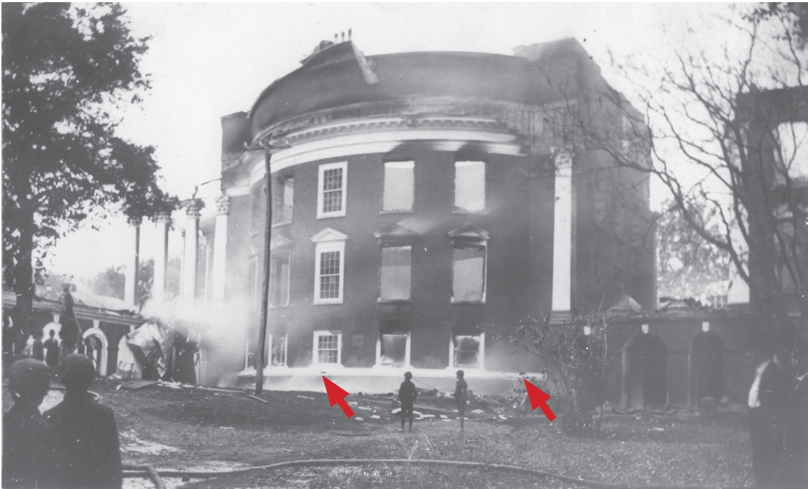
Figure 34. East elevation of the Rotunda after the 1895 fire. Note column in east oval room (in the upper photograph) and the exposed vents in the water table (lower photograph). [RG-30/1/10.011, UVSC]
