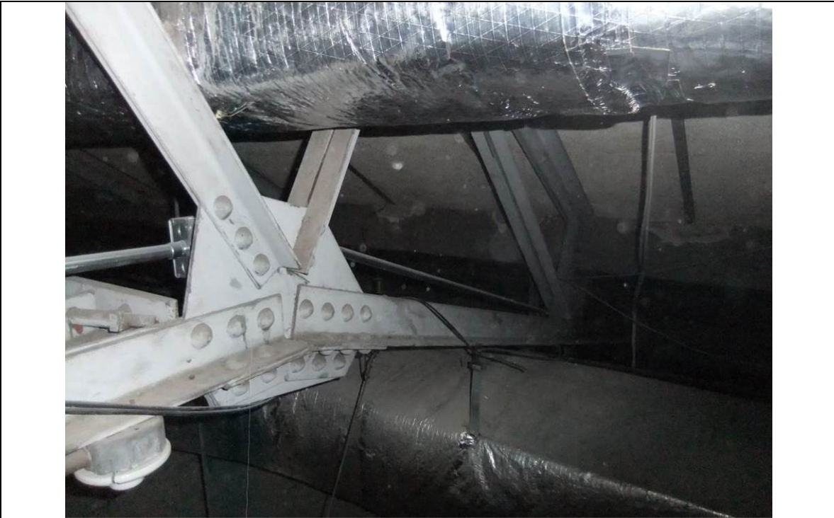
Figure 1.2.4.1-3: Typical riveted connections of roof truss. Note: Bottom chord panel members slope. Photograph by Robert Silman Associates, November 2012.
