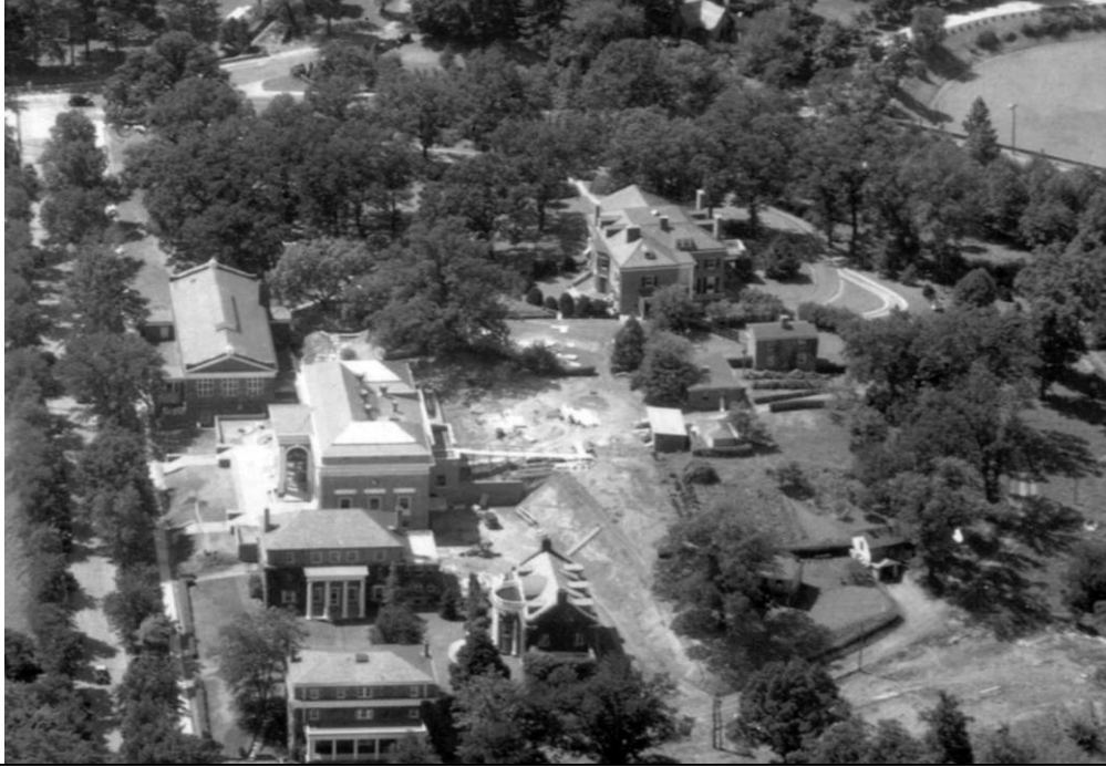
Figure 1.3.1-1: Detail view of the prominent sitting and use of terraces to shape the Bayly landscape visible in this oblique aerial view to the south late in the original construction, 1934. University of Virginia, Special Collections Library.
