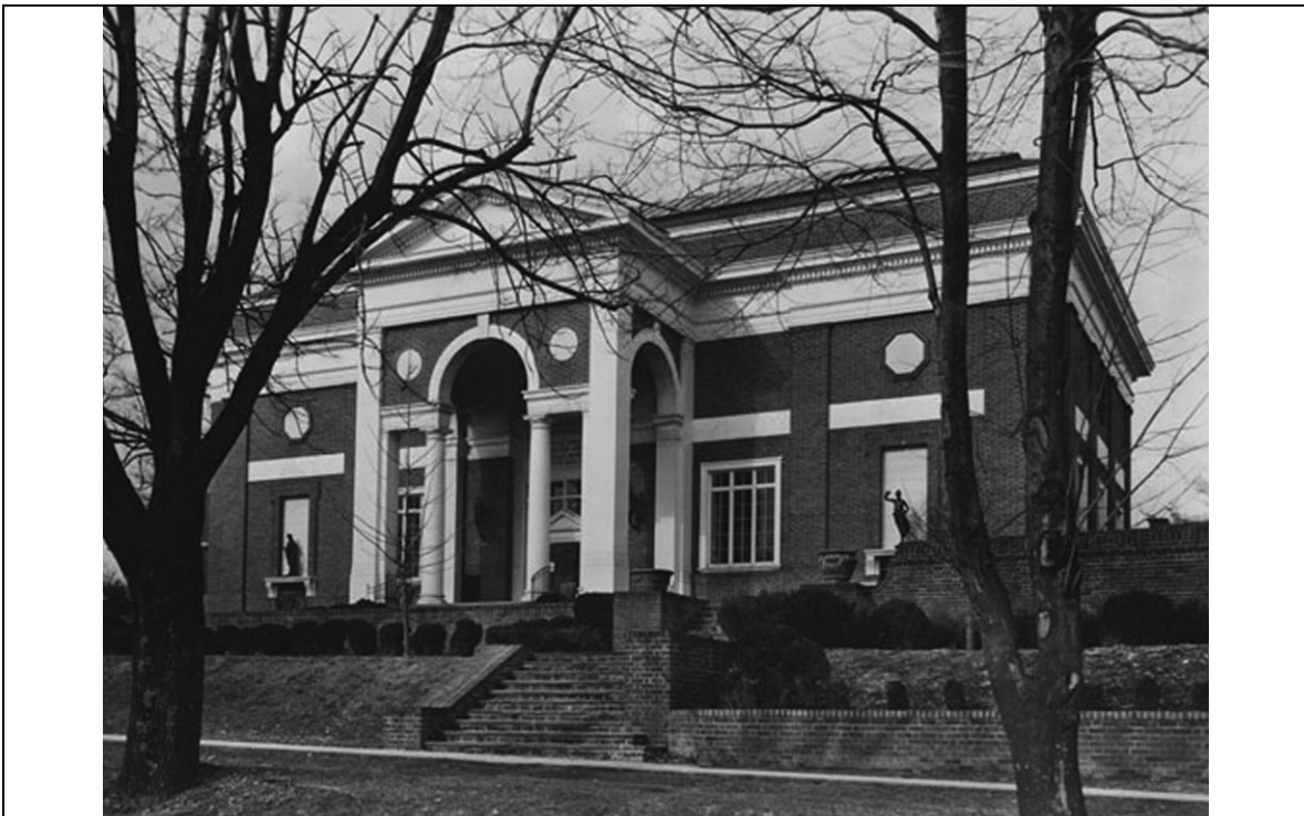
Figure 1.1.1-8: Apparent landscape modifications from 1935 to 1945 include a low brick wall and boxwood shrubs along the sidewalk to the right. University of Virginia, Special Collections Library-Visual History Collection. Print 07463.
