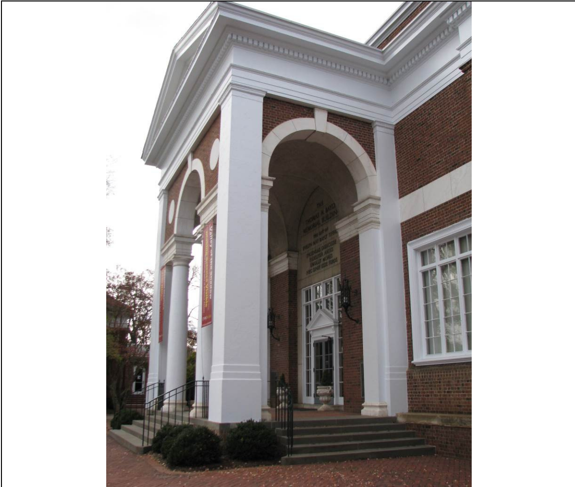
Figure 1.3.2-7: East fenestration. Photograph by John Milner Architects, November 2012.
