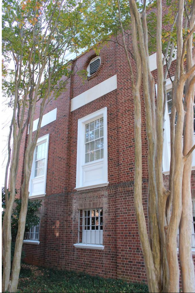
Figure 1.3.2-9: North fenestration. Photograph by John Milner Architects, November 2012.
