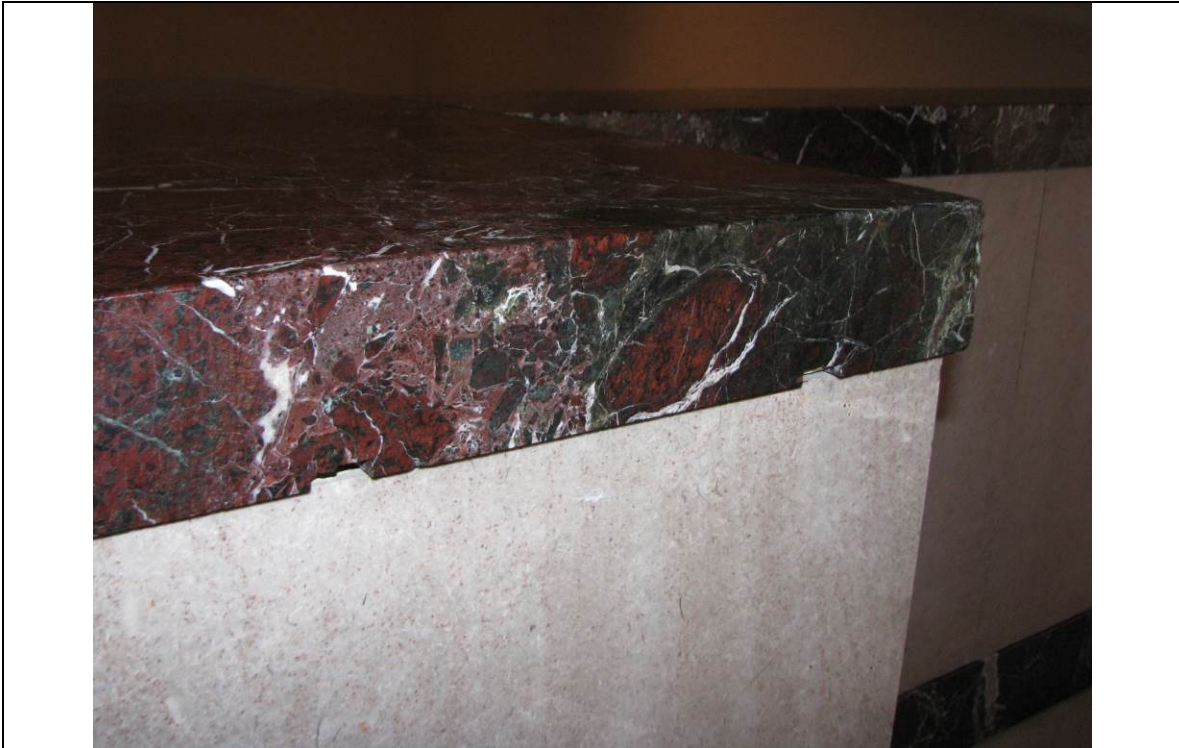
Figure 1.2.3-34: Chipped Levanto capstone at stair wall. Photograph by John Milner Architects, November 2012.
