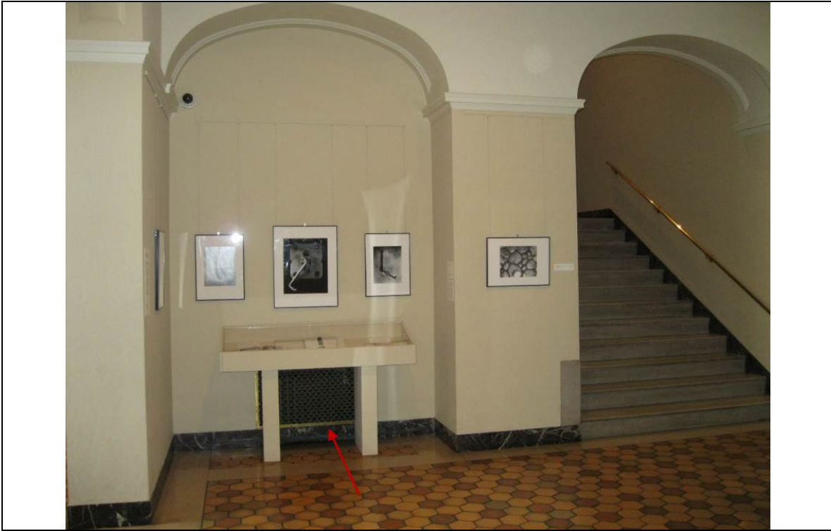
Figure 1.2.4.2-2: Radiator grille in first-floor Stair Hall. Photograph by T. Newbold, December 2012.
