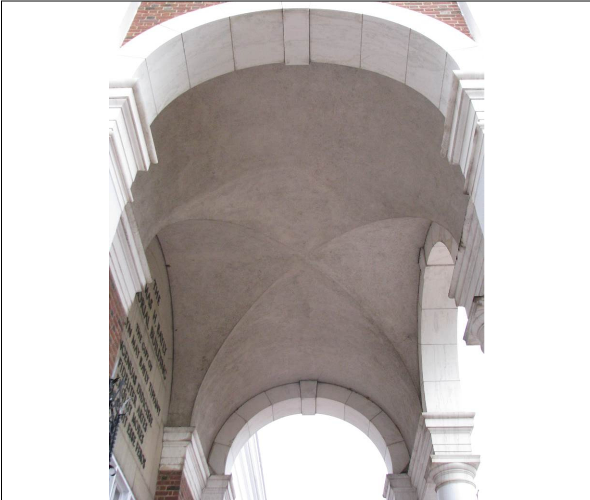
Figure 1.3.2-6: Vaulted ceiling of Portico. Photograph by John Milner Architects, November 2012.
