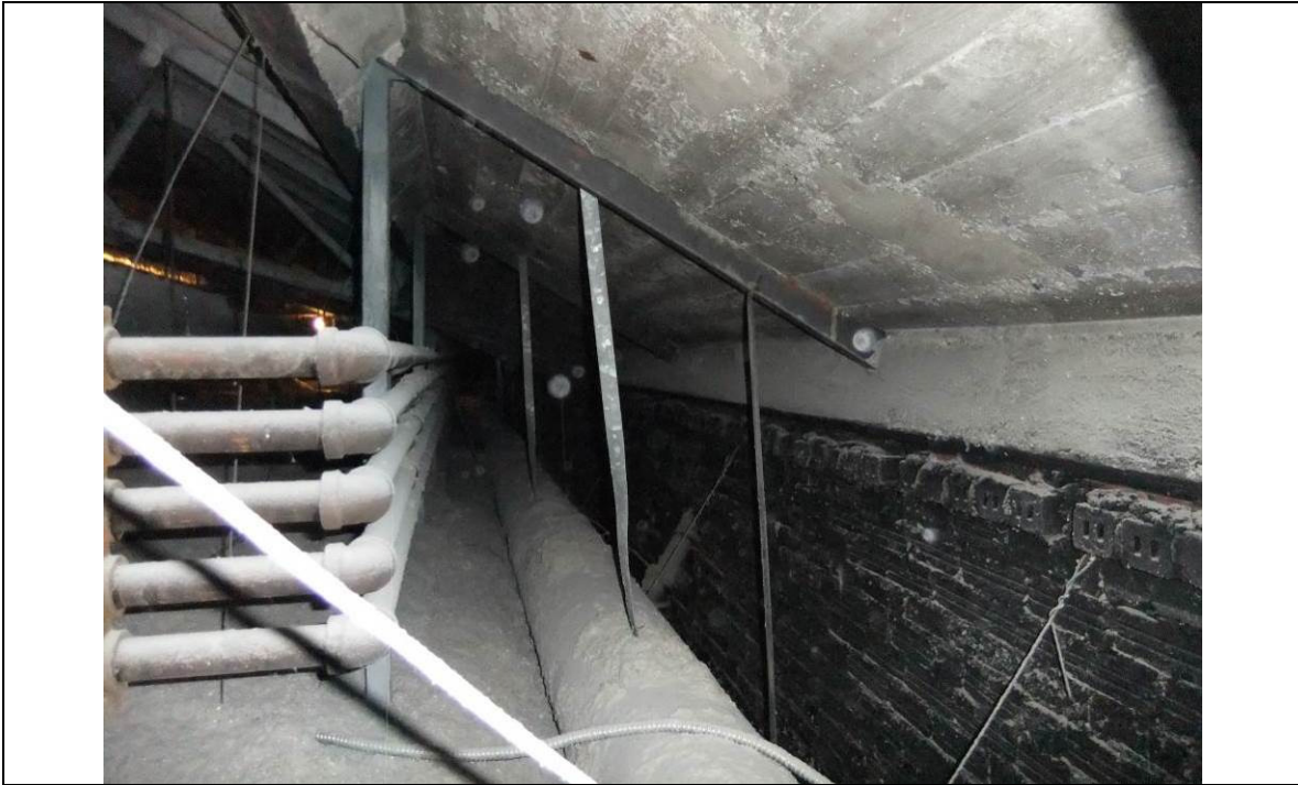
Figure 1.2.4.1-7: Original perimeter cinder-concrete slab and concrete-encased steel beams remain. Photograph by Robert Silman Associates, November 2012.
