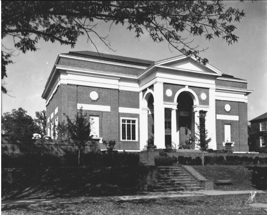
Figure 1.1.1-6: The in-process Bayly landscape construction shows newly installed trees, plantings, steps, and walls along the Rugby Road frontage in about 1935. University of Virginia, Special Collections Library, Hosinger Studio Collections.
