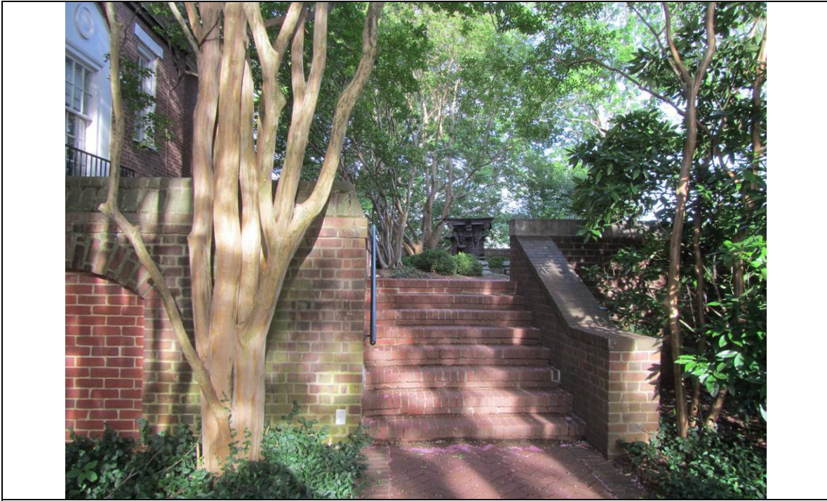
Figure 1.2.1-6: Brick steps and handrail between the East Terraces and the north side of the Bayly Building flanked by crepe myrtle trees. Photograph by Heritage Landscapes, June 2012.
