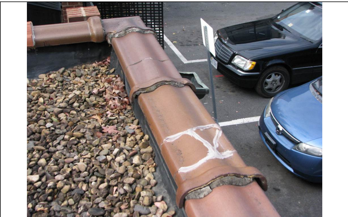
Figure 1.2.3-27: Sealant and mortar repairs at Annex parapet copings. Photograph by John Milner Architects, November 2012.
