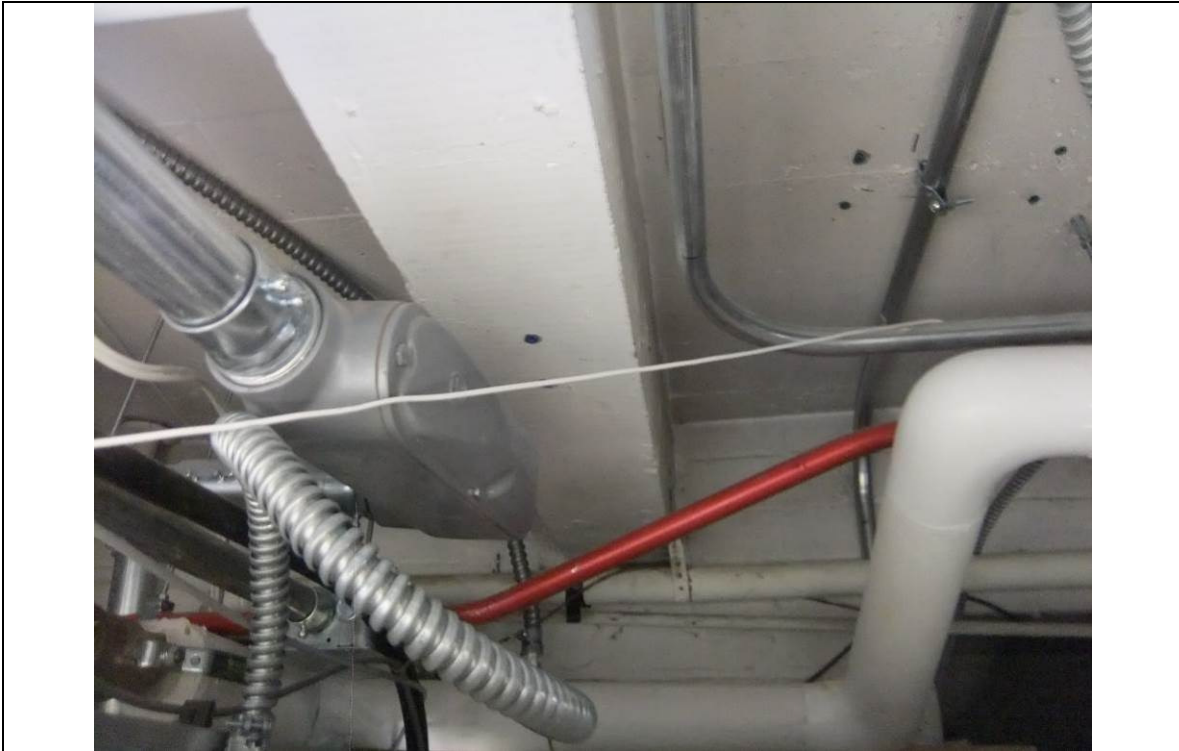
Figure 1.2.4.1-13: First-floor concrete-encased beam. Photograph by Robert Silman Associates, November 2012.
