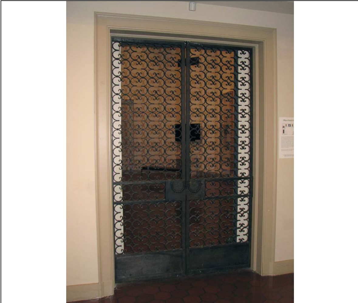
Figure 1.3.2-22: Gallery F door, as viewed from interior of gallery. Photograph by John Milner Architects, November 2012.
