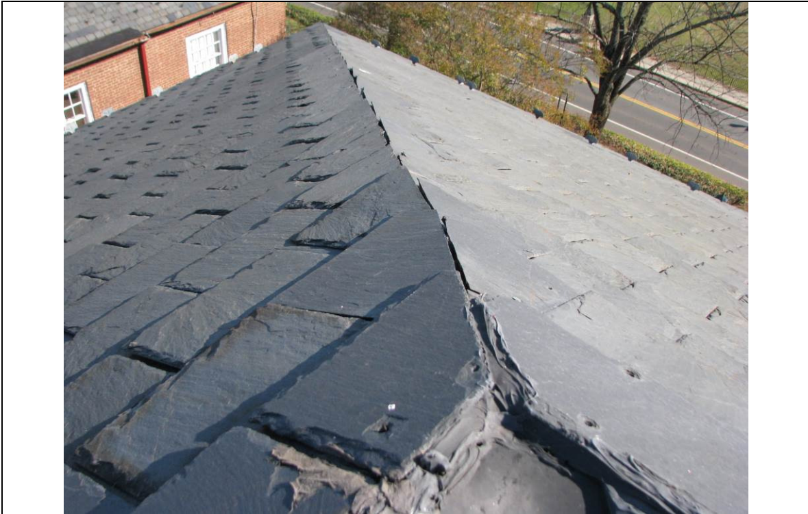
Figure 1.2.3-22: Mitered hip joint and caulked open ridge. Photograph by John Milner Architects, November 2012.
