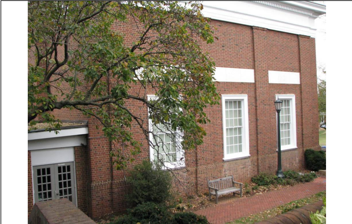
Figure 1.3.2-8: South fenestration. Photograph by John Milner Architects, November 2012.
