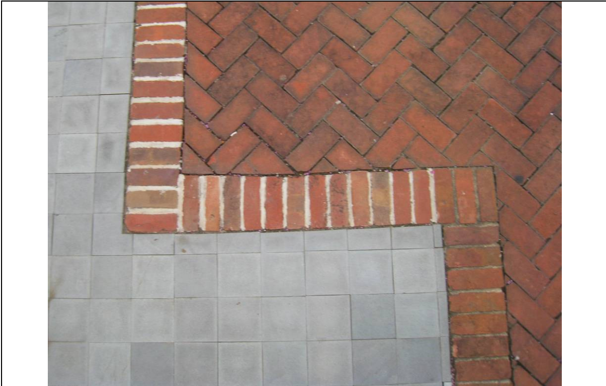
Figure 1.3.1-15: Brick-framed bluestone pavers fill the original island planting beds in the brick surface of the upper terrace. Note the recent bright mortar repair. Photograph by Heritage Landscapes, June 2012.
