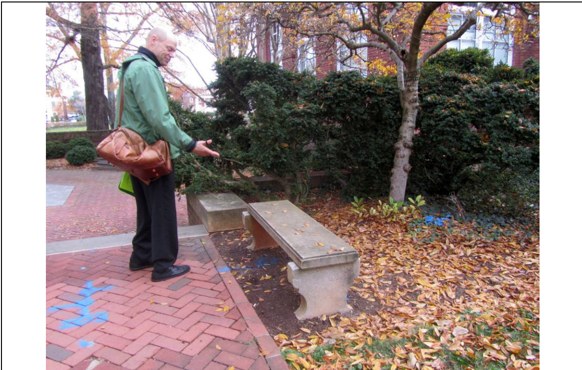
Figure 1.3.1-19: Concrete seat and legs of a bench in a nonhistoric position within the South Garden. Photograph by Heritage Landscapes, November 2012.
