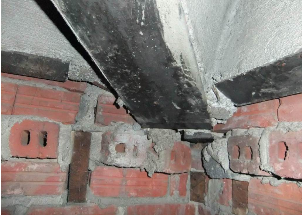
Figure 1.2.4.1-5: Bearing of steel hip rafter. Note: Use of hollow brick and wood outriggers to support eave. Photograph by Robert Silman Associates, November 2012.
