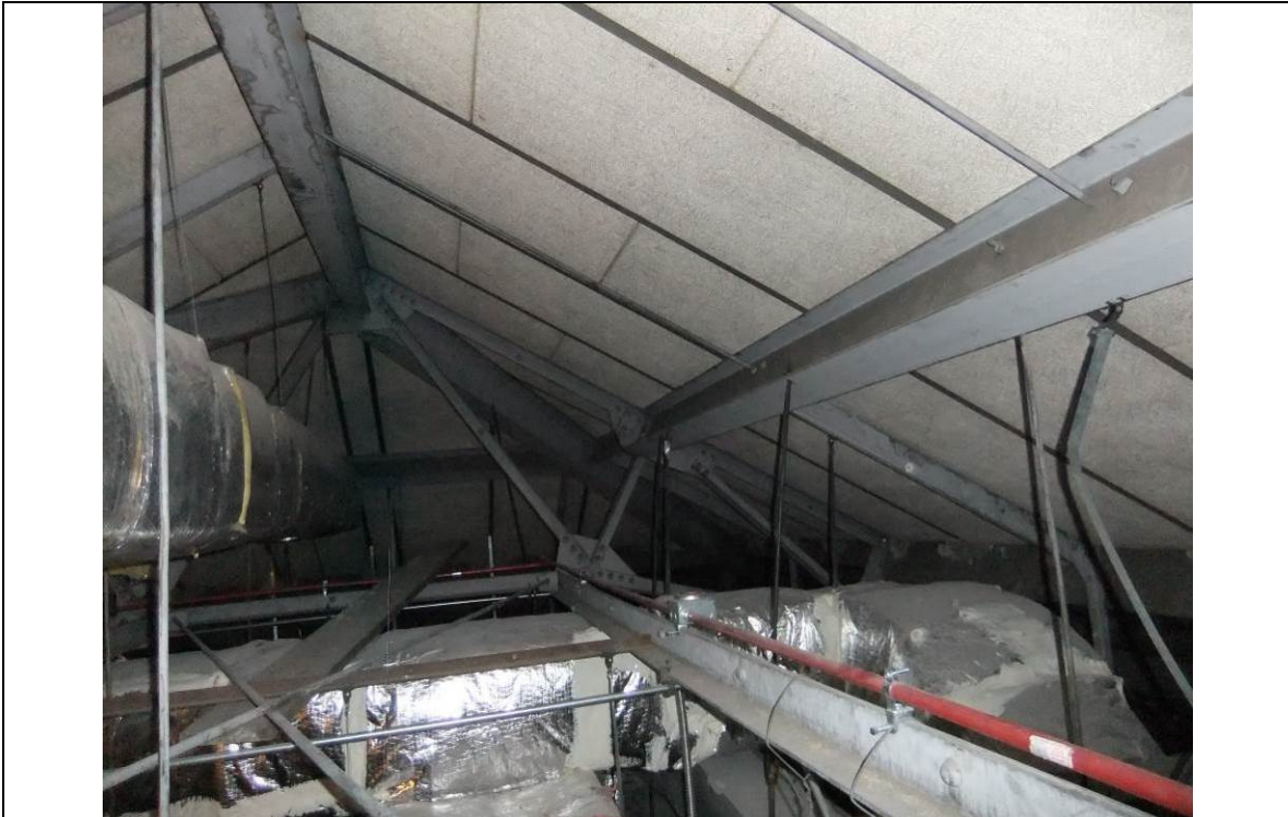
Figure 1.2.4.1-2: Steel roof truss (modified Fink). Note: Tectum roof deck installed. Photograph by Robert Silman Associates, November 2012.
