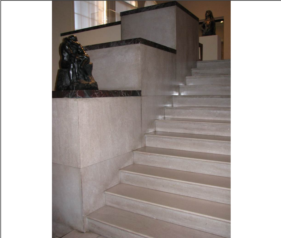
Figure 1.3.2-16: Upper Stair Hall, as viewed from main stairway. Photograph by John Milner Architects, November 2012.
