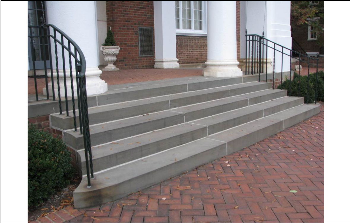
Figure 1.2.3-15: Iron stains at handrail anchor points. Photograph by John Milner Architects, November 2012.
