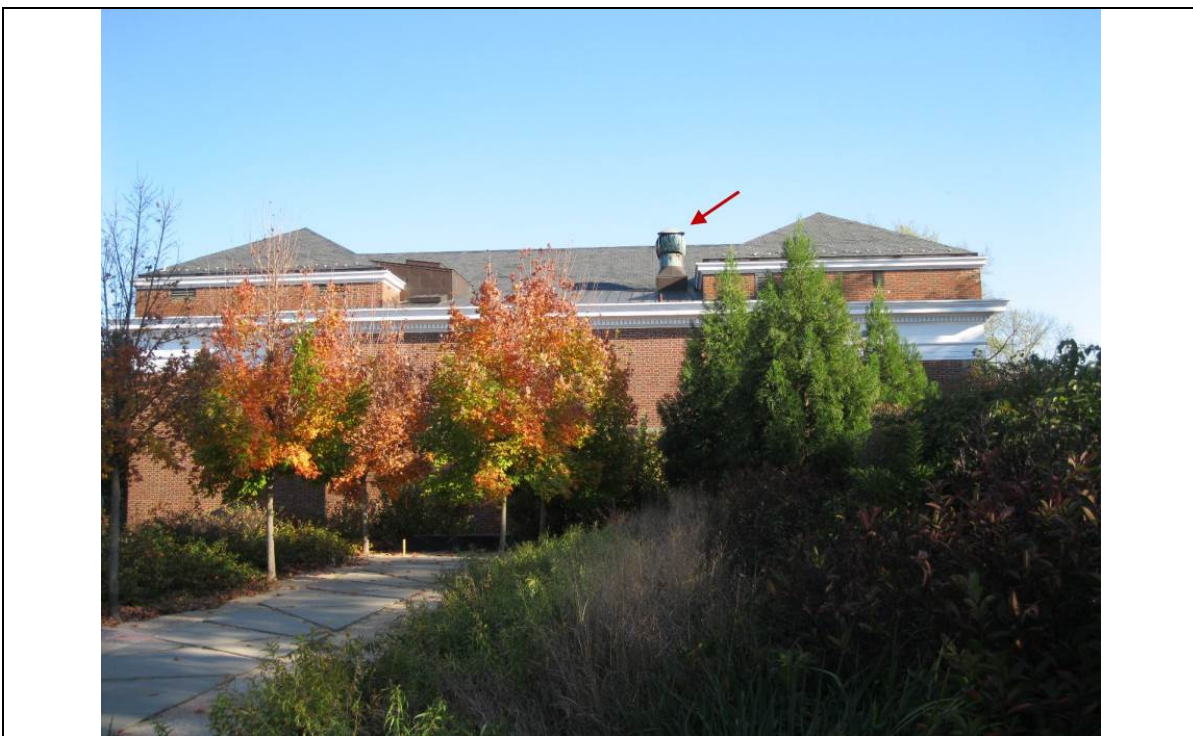
Figure 1.2.4.2-9: One remaining attic ventilator. Photograph by T. Newbold, December 2012.
