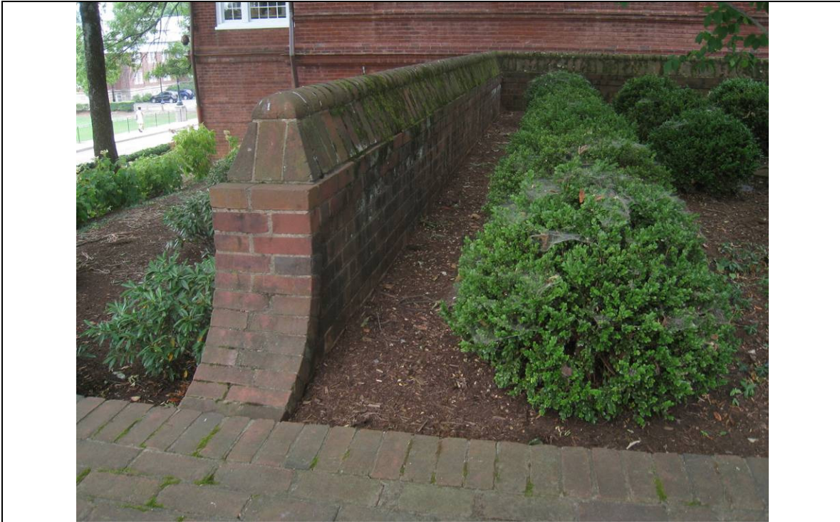
Figure 1.3.1-17: Molded brick coping on the southeastern parapet wall of the upper terrace and custom curved end wall. Photograph by Heritage Landscapes, July 2012.
