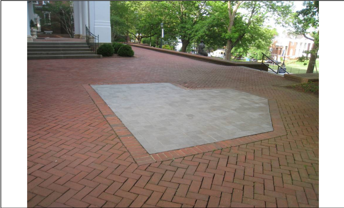
Figure 1.2.1-4: Steps to main entry and brick paving at upper terrace with flush stone infill over former planting bed. Photograph by Heritage Landscapes, June 2012.
