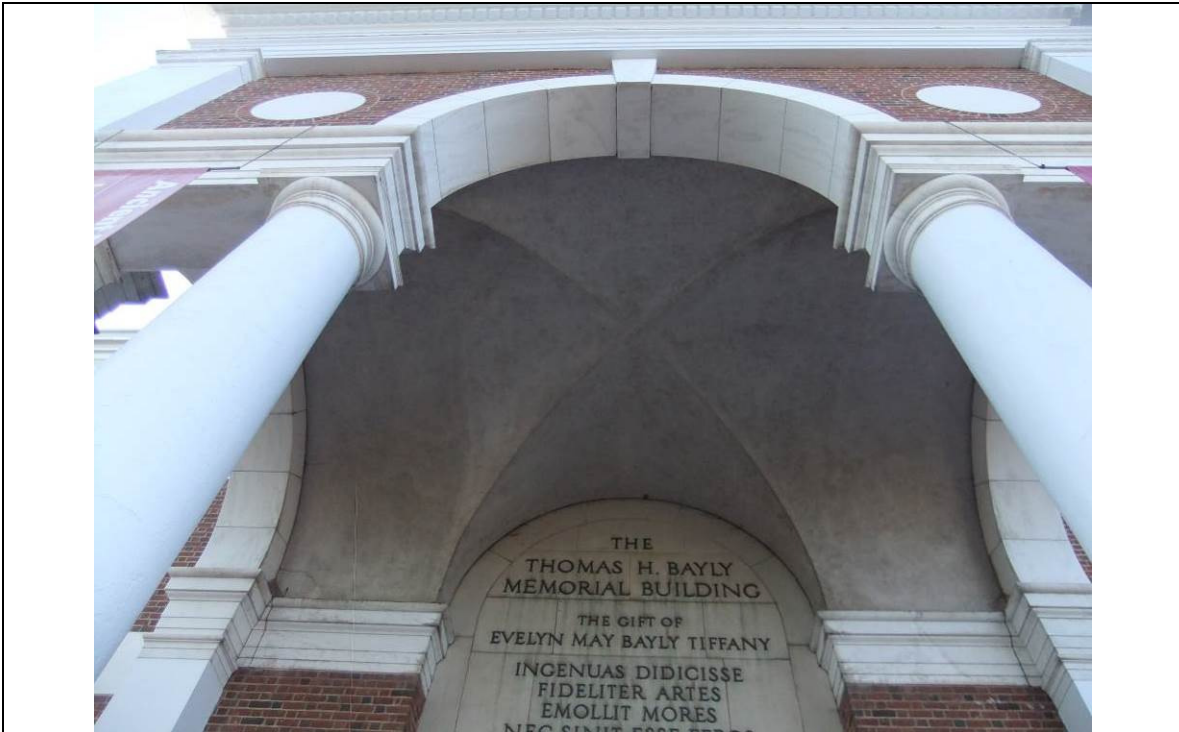
Figure 1.2.4.1-16: Underside of stucco Portico along East elevation. Photograph by Robert Silman Associates, November 2012.
