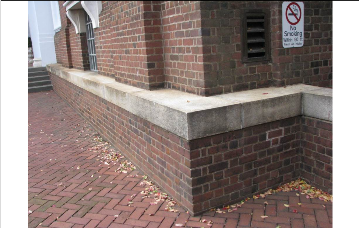
Figure 1.2.3-10: Soiled granite course. Photograph by John Milner Architects, November 2012.
