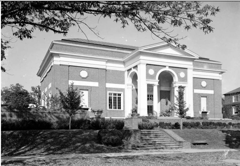
Figure 1.3.1-2: The completed landscape of the East Terraces portraying brick and stone steps, brick walls, ground-cover slopes, young ginkgo trees, and boxwood shrubs from Rugby Road, c. 1938. University of Virginia, Special Collections Library, Holsinger Studio Collections.
