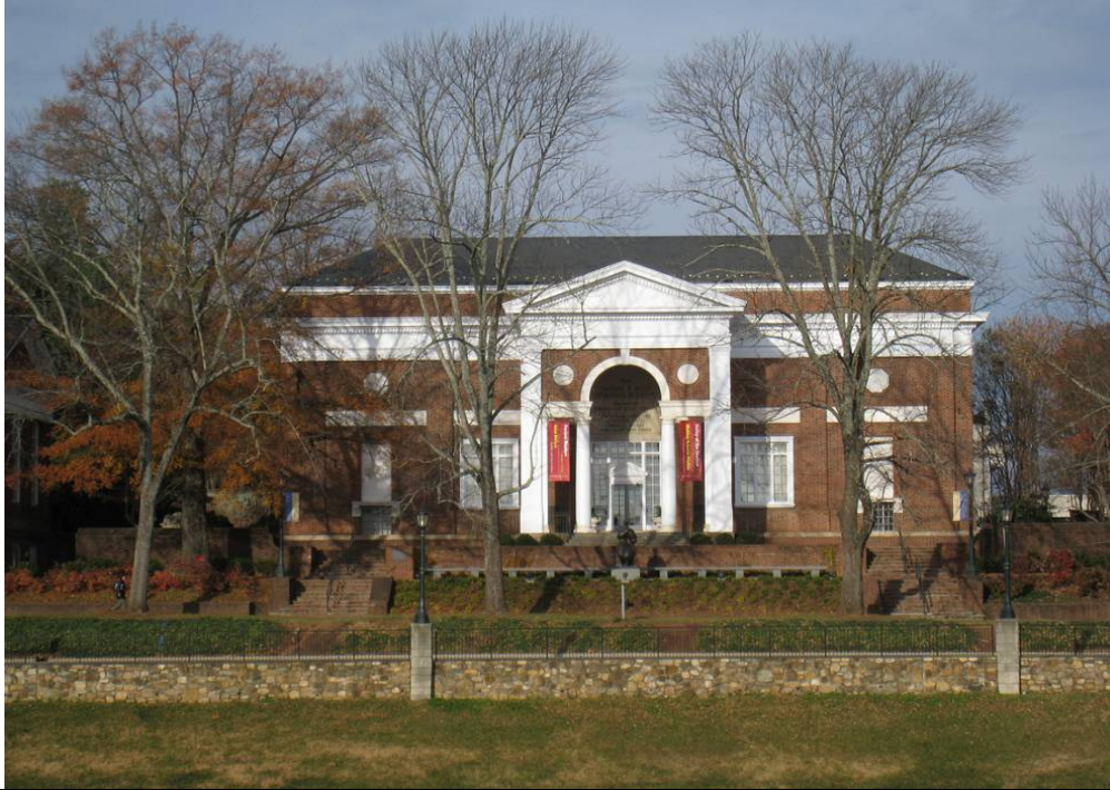
Figure 1.2.1-2 Slopes and steps provide transition between grades in terraced levels between Rugby Road and the entrance of the Bayly Building. Photograph by Heritage Landscapes, November 2012.
