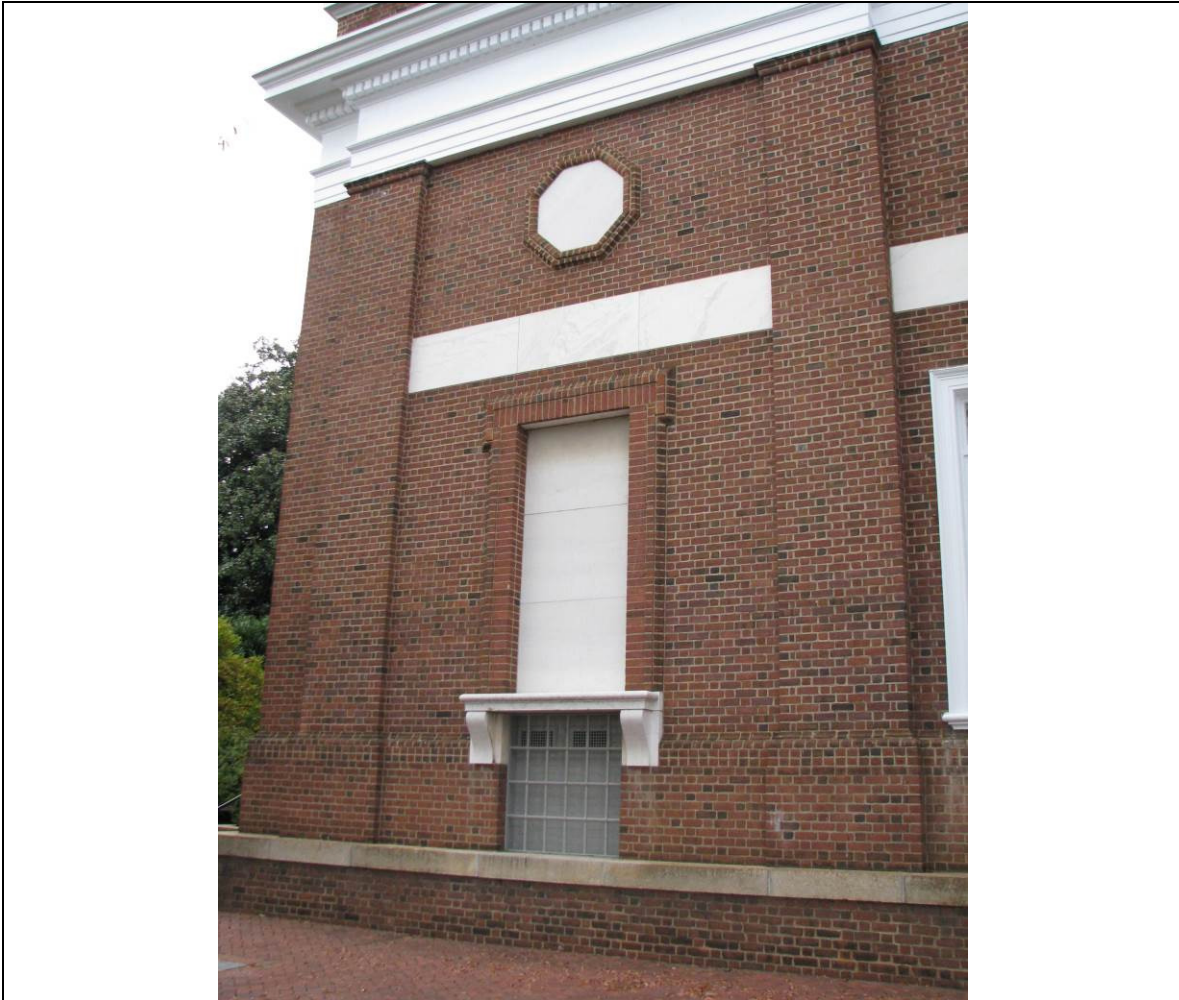
Figure 1.3.2-3: Blind window at East facade. Photograph by John Milner Architects, November 2012.
