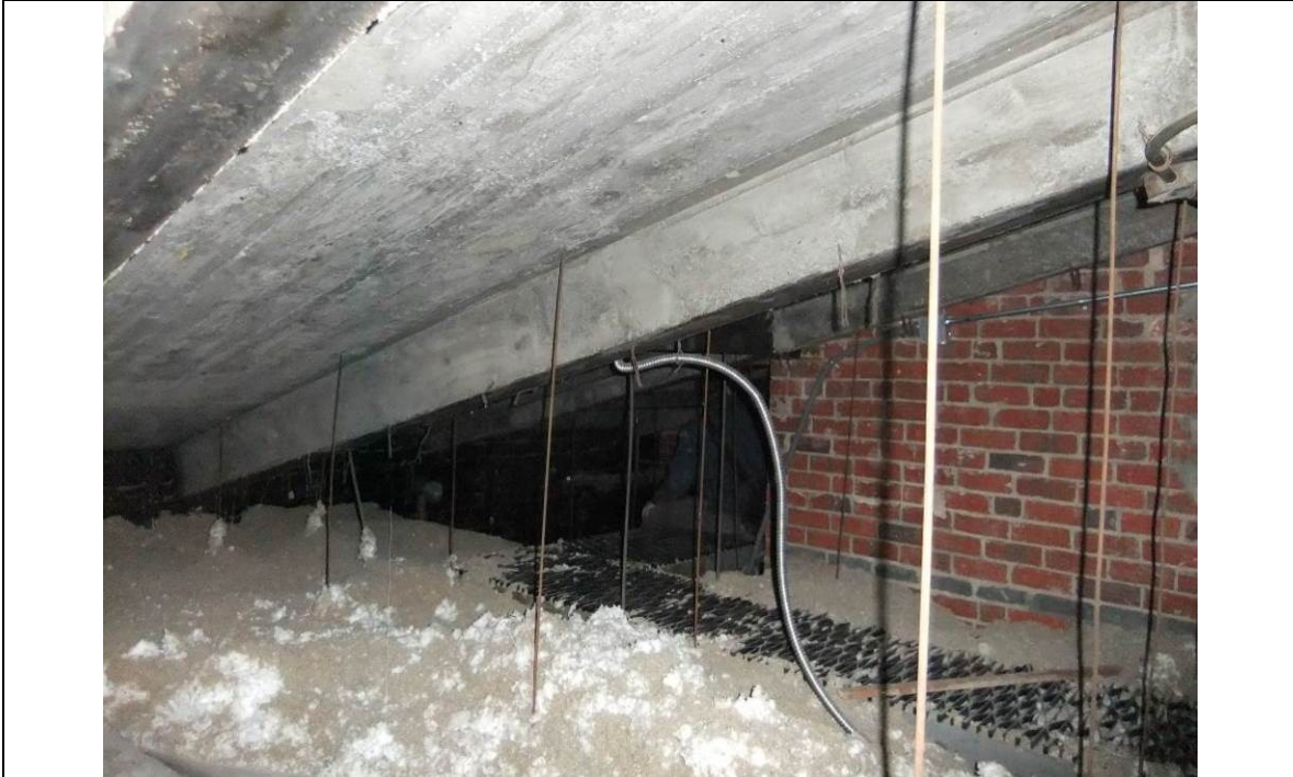
Figure 1.2.4.1-8: Reinforced cast-in-place concrete roof slab and supporting concrete-encased steel framing. Note: Presence of catwalk and insulation. Photograph by Robert Silman Associates, November 2012.
