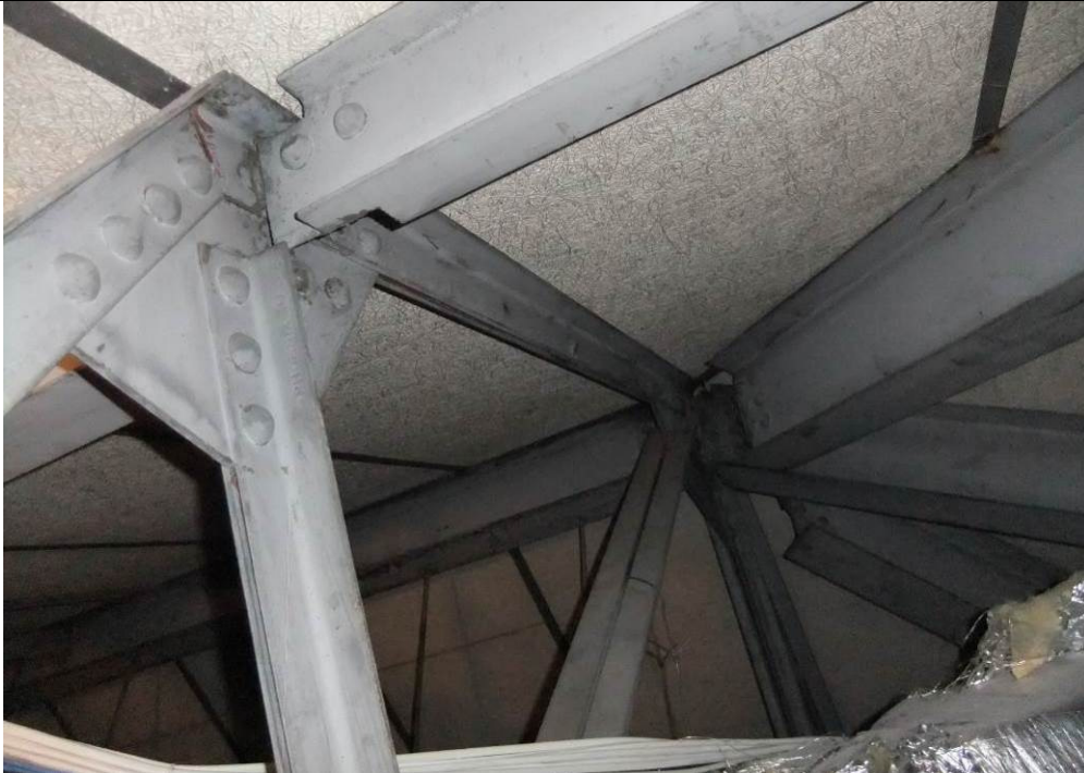
Figure 1.2.4.1-6: Roof retrofit with Tectum roof panels. Note: Bulb-tee purlins welded to original truss and associated wide flange purlins. Photograph by Robert Silman Associates, November 2012.
