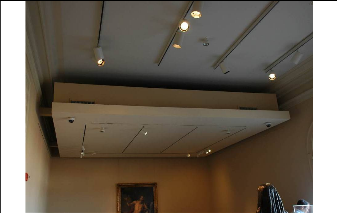
Figure 1.3.2-26: Non-character-defining air-distribution system suspended beneath Upper Stair Hall ceiling. Photograph by John Milner Architects, November 2012.
