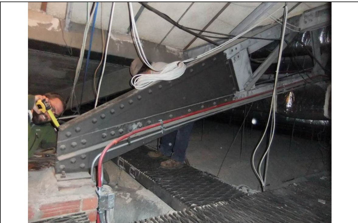
Figure 1.2.4.1-4: Bearing of roof truss on interior brick masonry wall. Note: Gusset plates and hung catwalk. Photograph by Robert Silman Associates, November 2012.
