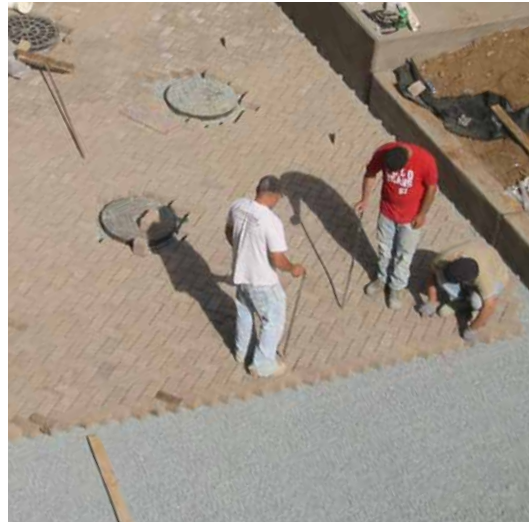
Installation of pervious pavers over a cistern
