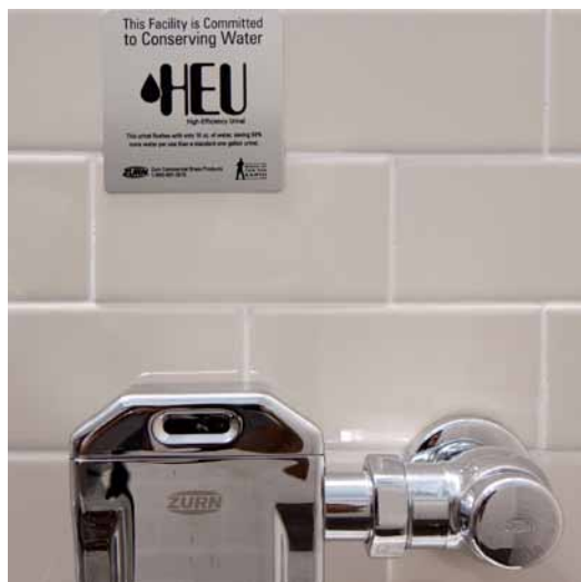
A low-flow pint-per-flush urinal in Gibson Hall
