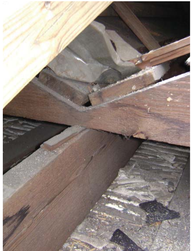
Figures 36 & 37 Details of the “serrated lath” type roof over the student rooms.
