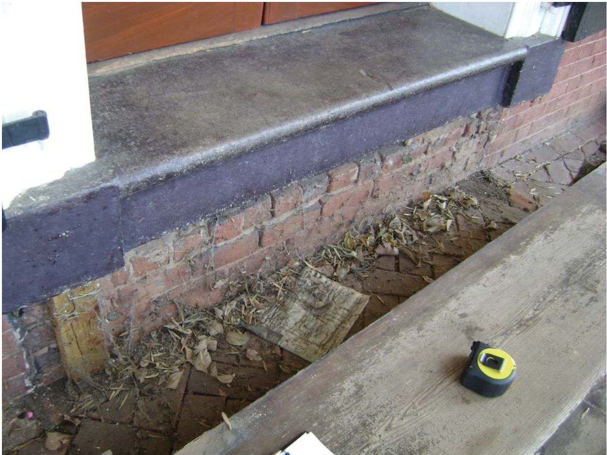
Figure 46 The brick surface behind the entry steps is made up of later infill suggesting this space may have originally contained an opening of sorts, possibly similar that found behind the steps at Pavilion VI. Paint lines exist on the pavilion walls to either side of the infill suggesting wood steps may have butted against the wall here.
