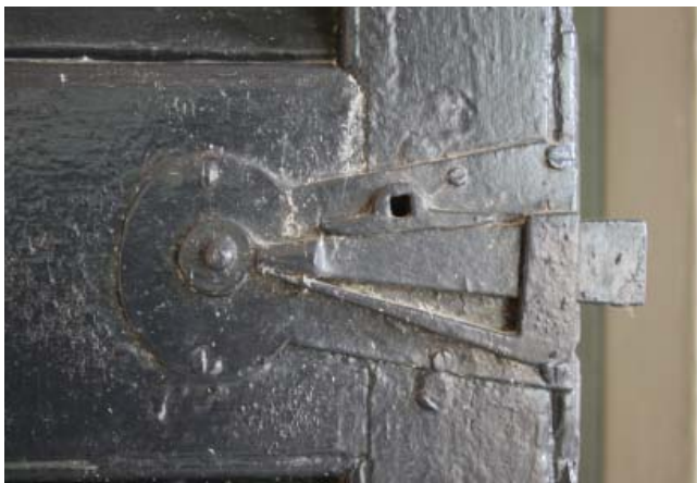
Figure 43 Door blind at No. 13, West Range. Detail of surface mounted plate latch. While ghosts for this type of latch survive on other blinds along the West Range, this example was the only one found remaining.
