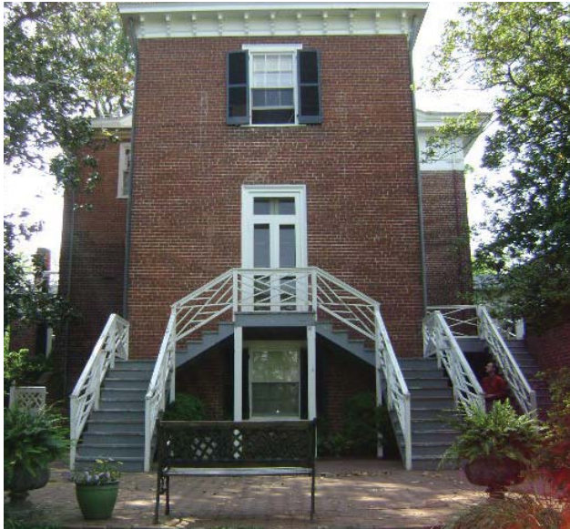
Figure 24 East (rear) elevation of Pavilion X. Paint ghosts support archival documentation indicating a one story porch at this elevation.
