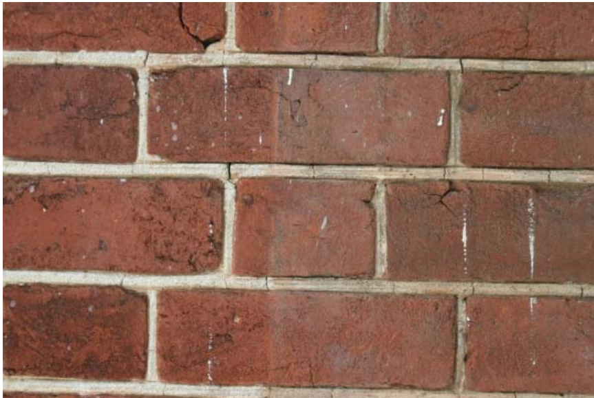
Figure 34 Pavilion X west elevation. Detail of oil struck bricks laid in Flemish bond. Colorwash and penciling still survives in sheltered areas of this elevation.
