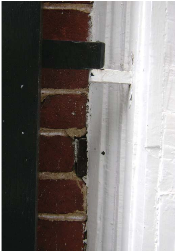
Figure 39 A portion of the original sill for the window in figure 37 remains buried in the masonry wall.
