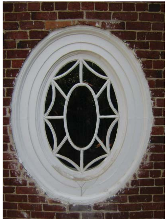
Figure 44 South elliptical window. Note the crude manner in which this window was installed. The elliptical windows disrupt the original fenestration pattern and clearly read as an afterthought.
