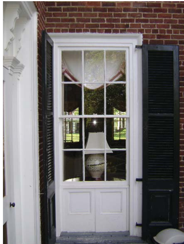
Figure 39a East elevation, north window. This window was modified when the 1877-8 addition was built. The window was turned into a door providing access to a wood porch and later converted back into a window.
