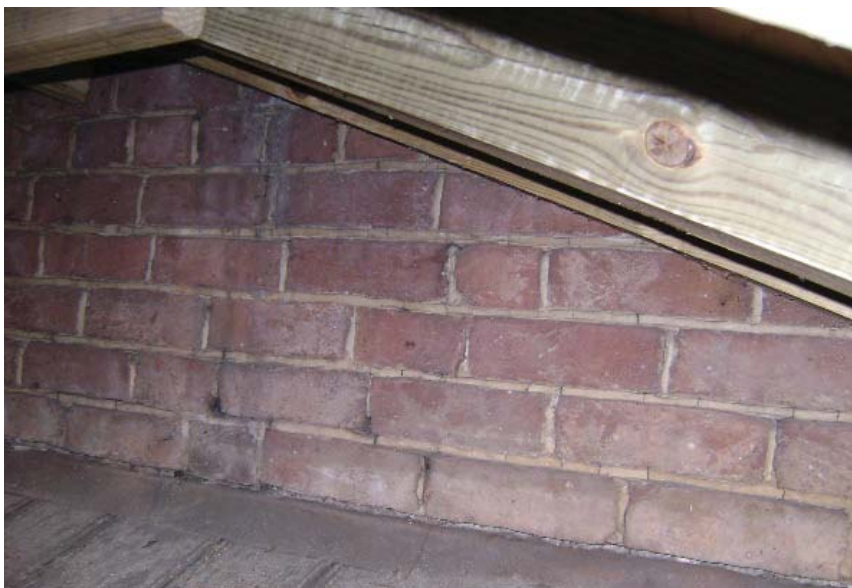
Figure 35 Attic space of student room north of Pavilion X. Portions of encapsulated brickwork survive on the north and south walls providing period examples of the original joint finish and appearance. Note the serrated roof at the bottom of the image.
