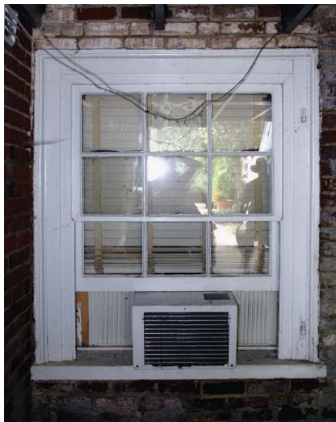
Figure 22 & 23 One set of pintles are located on the right side of the north cellar window on the east elevation. It is believed the rear stair passed in front of a portion of the cellar windows resulting in the condition illustrated above resulting in the need for only one set of pintles.
