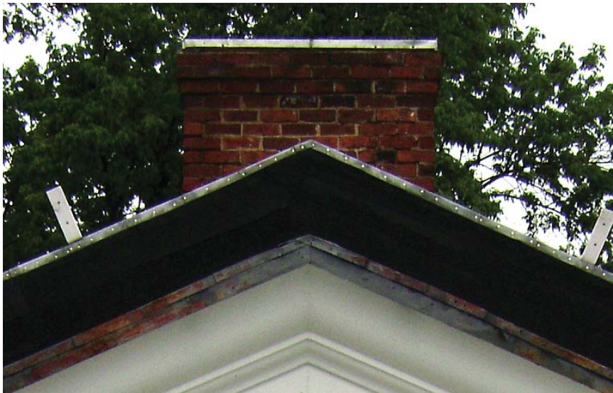
Figure 33 New stainless steel brackets were installed during the 1987 roof restoration in anticipation of restoring the parapet at a later date.
