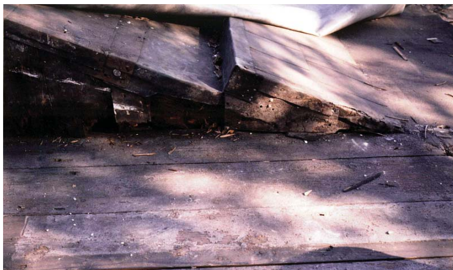
Figure 30 Detail of the original Philadelphia gutter.
