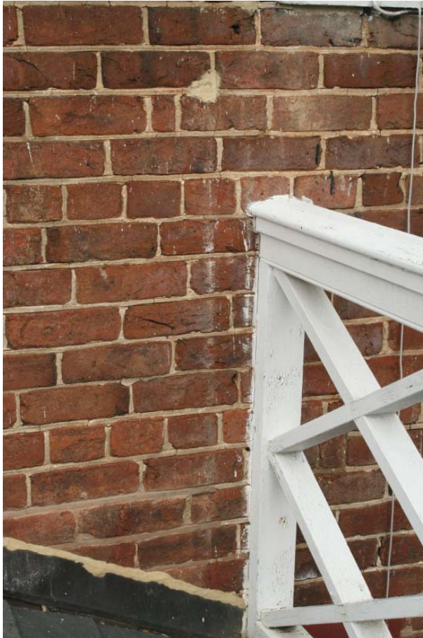
Figures 38 Scars and ghosts show the location of where the original Chinese rail joined the side-walls of Pavilion X.
