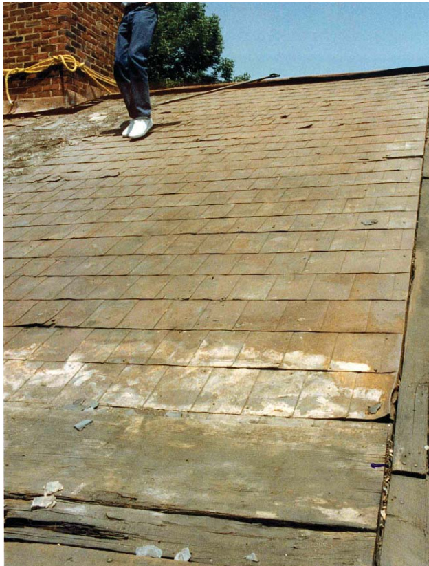
Figures 26, 27, 28 Jefferson's tin plated iron roof uncovered during the removal of the later period standing seam roof. Summer 1987.
