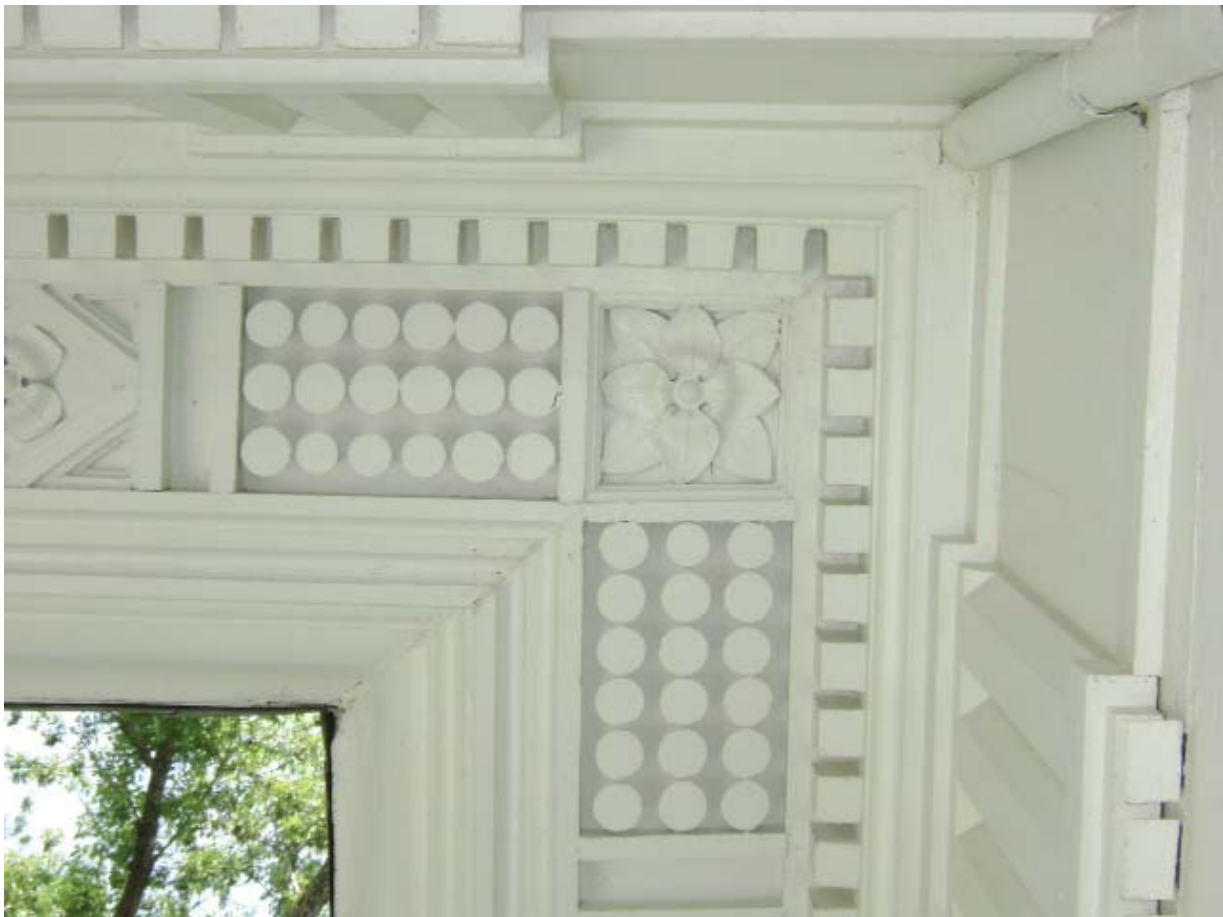
Detail of cornice and frieze of entablature.
