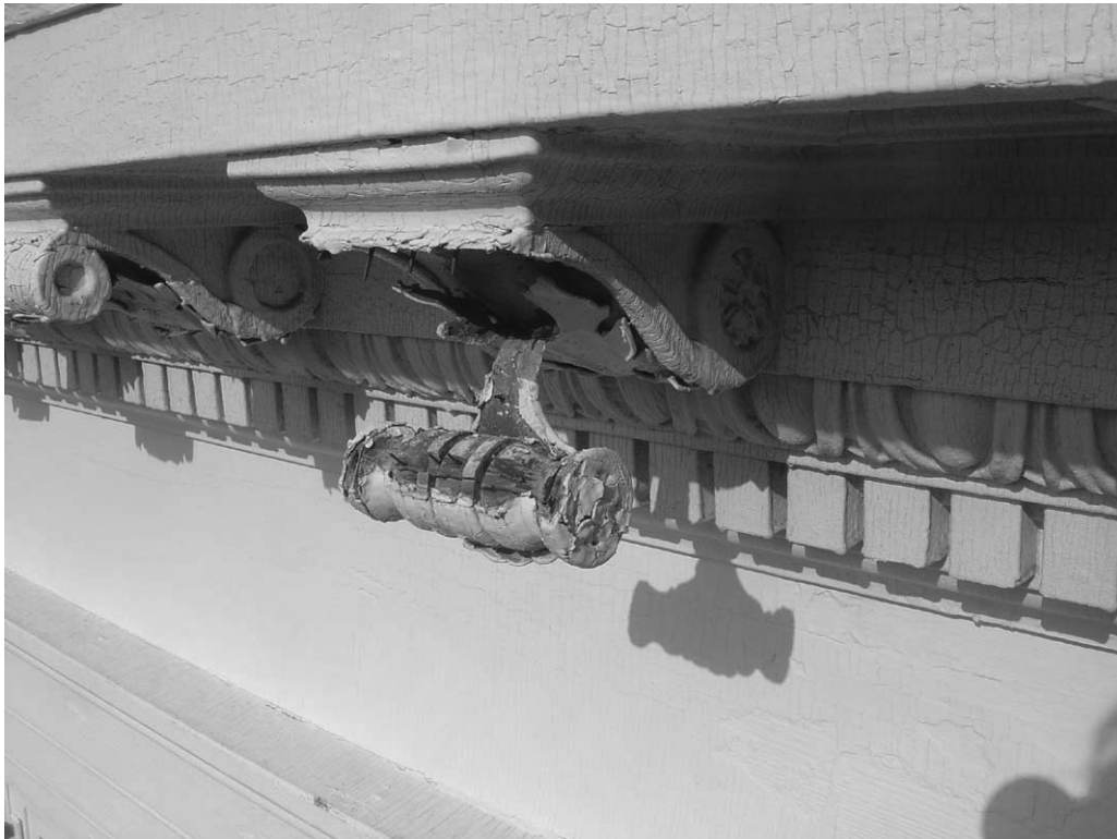
Inferior quality replacement material is failing throughout the entablature. July 2005
