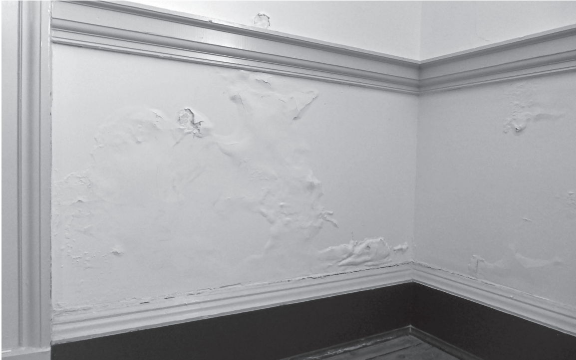
The painted wall plaster in the northeast corner of room 103 is blistered and friable. The damage has been caused by water infiltration that is attributable to a backup in the storm water drainage system at the northeast downspout.
