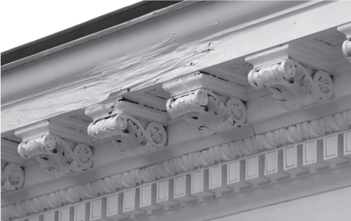
Leaks in the seams of the sheet metal roofing and rust-through perforations in the sheet metal are causing the wood cornice moldings and modillions of the north elevation to rot.
