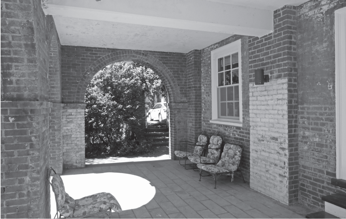
In this view towards the south end of the east porch worn and peeling paint, efflorescence, and algae are visible.
