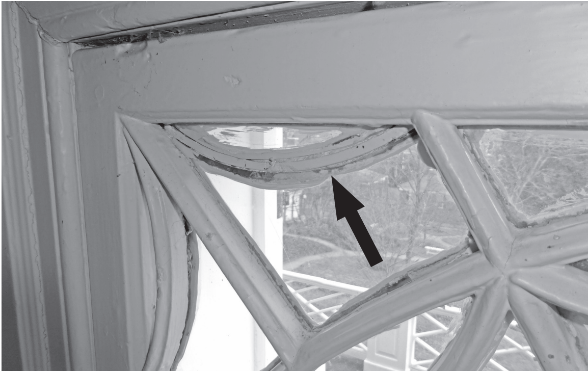
The interior face of the segmental muntin at the first floor east door transom is missing. It is one of three muntins missing at the transom. The build-up of paint coatings has obscured the molding profiles of the sash.
