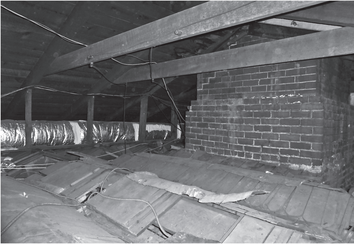
Attic above 1823 pavilion, looking northeast, with the surviving ridge-and-furrow roof and sheet metal flashing in the foreground.
