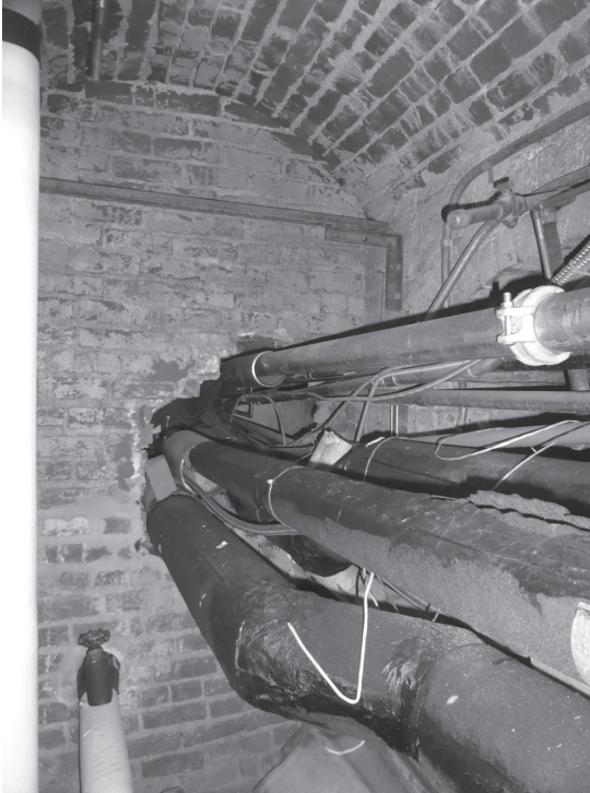
The brick masonry above the opening at the south end of B14 is unsupported.
