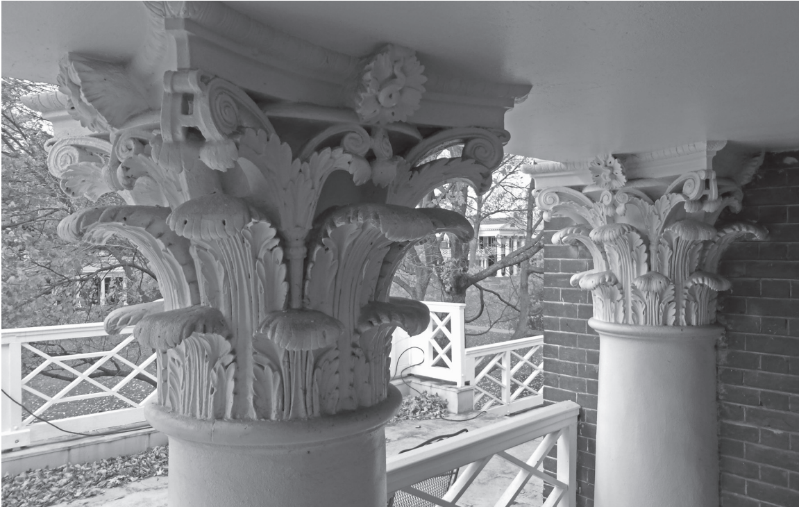
The Corinthian capitals have been painted, obscuring the original marble surface. The painted finish is dirty, and there is paint overspray on the adjacent brick.
