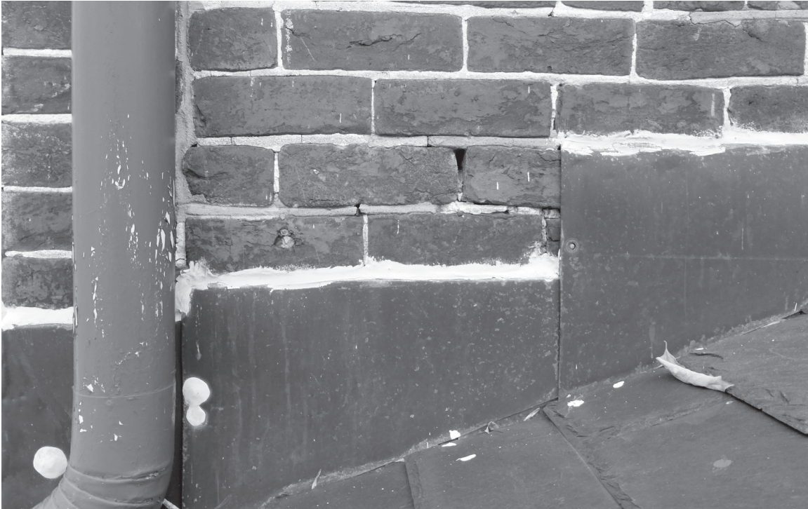
The mortar in the brick wall construction near the second floor, southwest corner of the pavilion has failed; the mortar is eroded, cracked, and missing. An excessive application of sealant at the roof flashing detracts from the appearance of the building construction.
