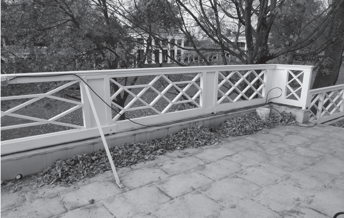
The flat-lock seam sheet metal roofing above the colonnade is compromised by penetrations for the attachment of the railing and railing braces. The scuppers draining to the west are clogged with leaves and debris.
