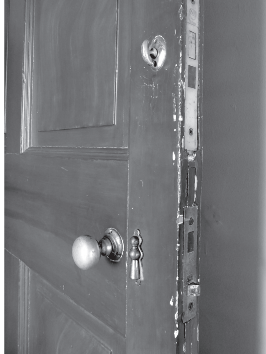
The coatings at the exposed edges of the faux-finish grained doors are chipped and abraded.
