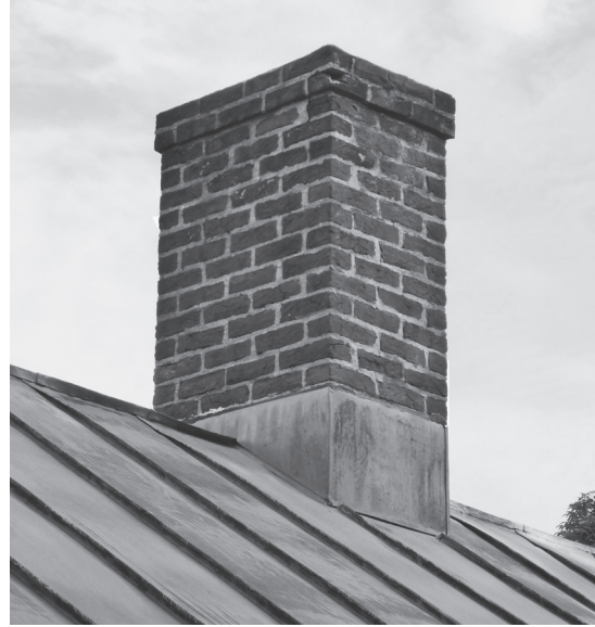
Figure 44. Chimney and standing seam roof.
