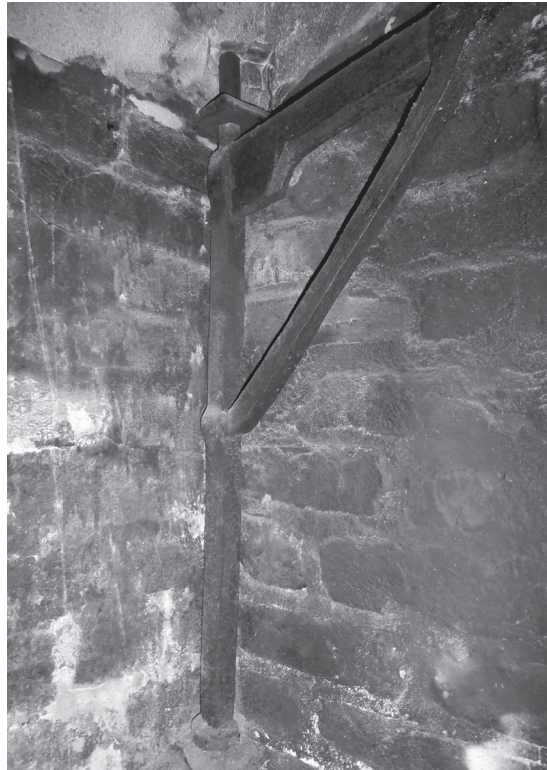
Figure 54. The original pot crane survives in the fireplace.
