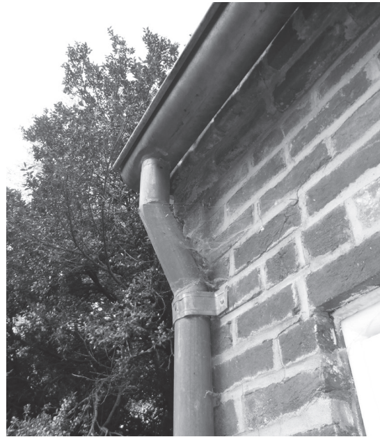
Figure 64. There is stepped cracking of the repointed mortar joints on the east elevation of the cottage, at the upper southeast corner. The mortar has been heavily applied and buttered over the edges of the bricks.
