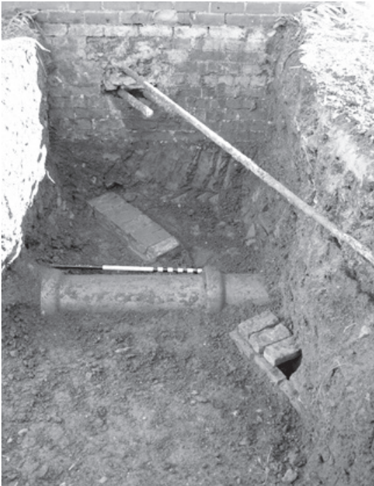
Figure 29. A mortared brick box drain adjacent to and west of the circa 1900 southwest addition to Pavilion IX. The subsequent installation of a 12-inch diameter terra cotta storm water line severed the brick box drain.
