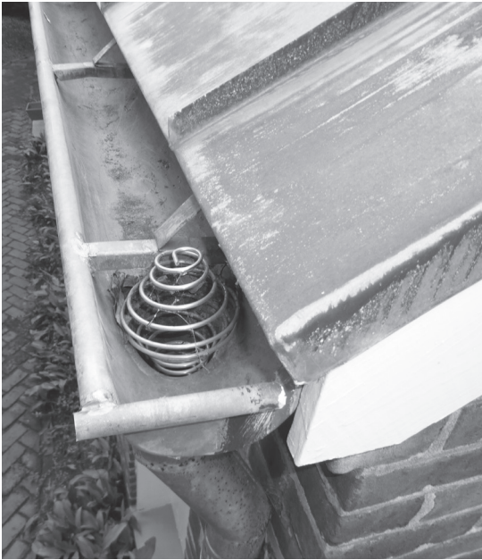
Figure 63. The terne-coated stainless-steel sheet metal roofing developed an abnormal oxidation with a brown “rusted” appearance. The roof was painted between August and October 2017, obscuring this condition.
