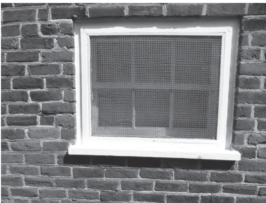
Figure 72. The hardware cloth covering the insect screens at the window openings is visually obtrusive.
