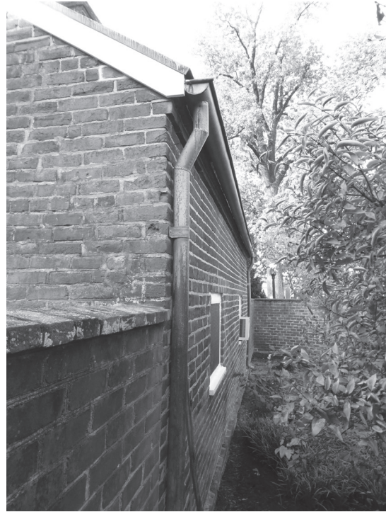
Figure 68. The brick masonry on the north elevation of the cottage, at the northwest corner, has eroded mortar joints and broken brick. Algae and lichen are growing on the brick.
