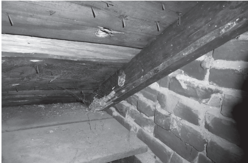
Figure 76. The base of the west roof rafter adjacent to the north gable wall is rotted. The mortar at the interior face of the gable wall is deteriorated.
