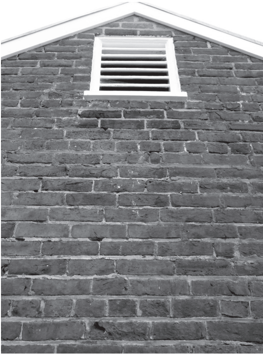
Figure 69. There are open pockets in the mortar joints near the center of the north elevation.
