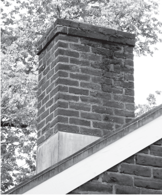
Figure 70. The mortar joints in the chimney construction above the roofline are deteriorated; the mortar is cracked and loose. Moss is growing in the mortar joints on the north elevation of the chimney, and the brick is soiled.
