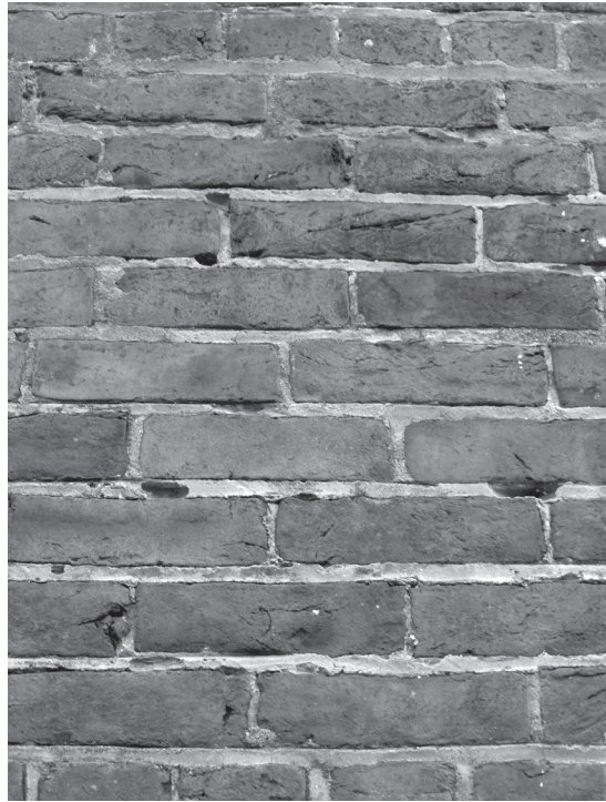
Figure 69. There are open pockets in the mortar joints near the center of the north elevation.
