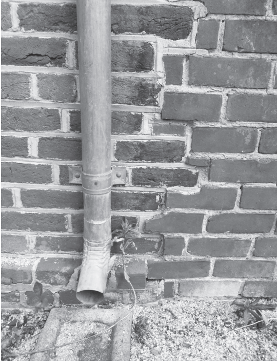
Figure 74. On the west elevation, the brickwork at the juncture of the garden wall and the southwest corner of the cottage is awkwardly resolved. The brick coursing is offset and does not align; there are open mortar joints near grade level.
