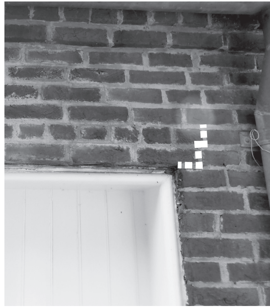
Figure 66. The pointing repairs made above the northeast door are muddled and irregular. The steel lintel above the door opening is rusted; the expanding rust may be jacking the masonry. Cracks have developed in the repair mortar at the north end of the lintel (highlighted by the dotted line).
