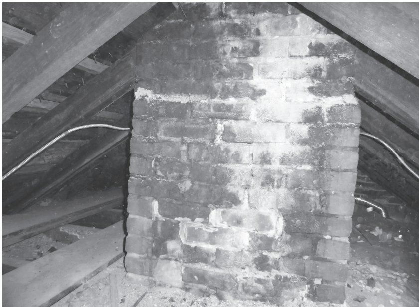
Figure 77. There are open joints in the brick chimney at the attic level. Mortar has been smeared on the face of the brick, and creosote appears to have migrated through the mortar joints.
