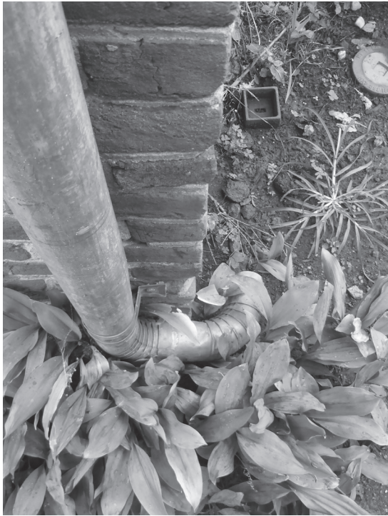
Figure 67. The downspout at the northeast corner drains to grade against the north elevation of the building.
