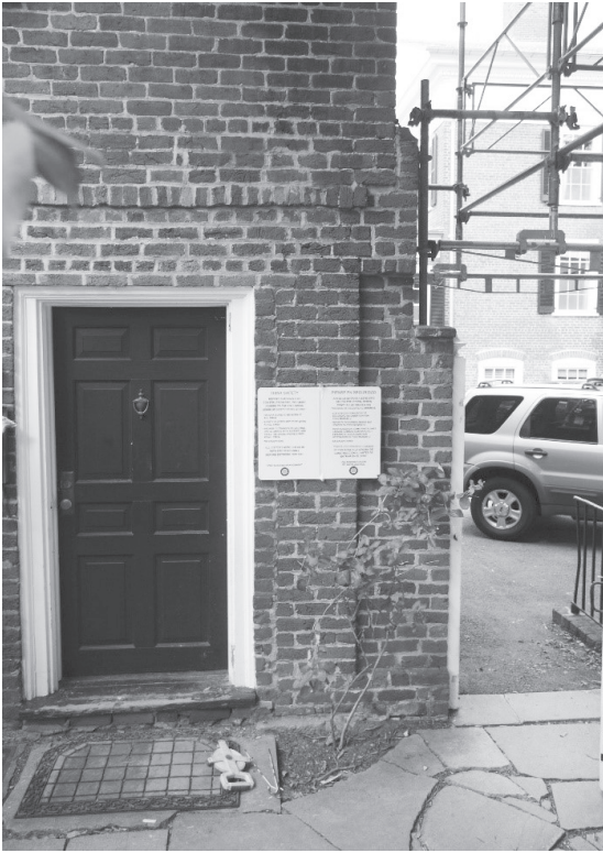
Figure 33. A late nineteenth-century expansion of the Mews (in the Pavilion III garden) incorporated an existing garden wall, complete with brick piers and a gate opening, into a new south façade.
