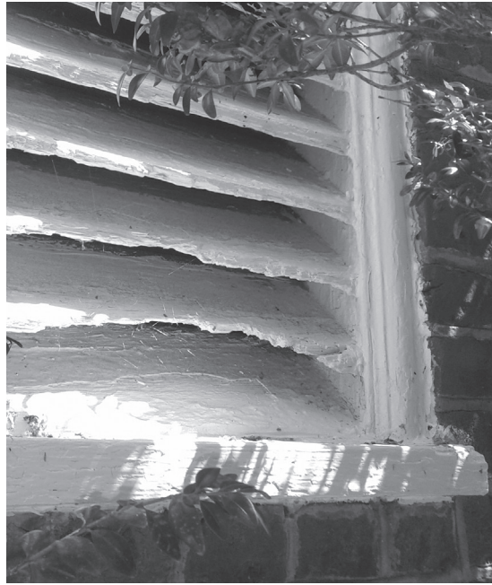
Figure 71. The painted wood slats of the louvered south gable vent are heavily eroded.
