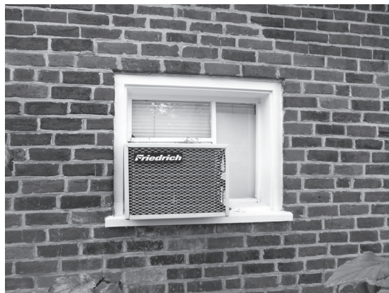
Figure 73. The air-conditioning unit in the southwest window opening is visually obtrusive. The sash has been altered to accommodate the air conditioner.
