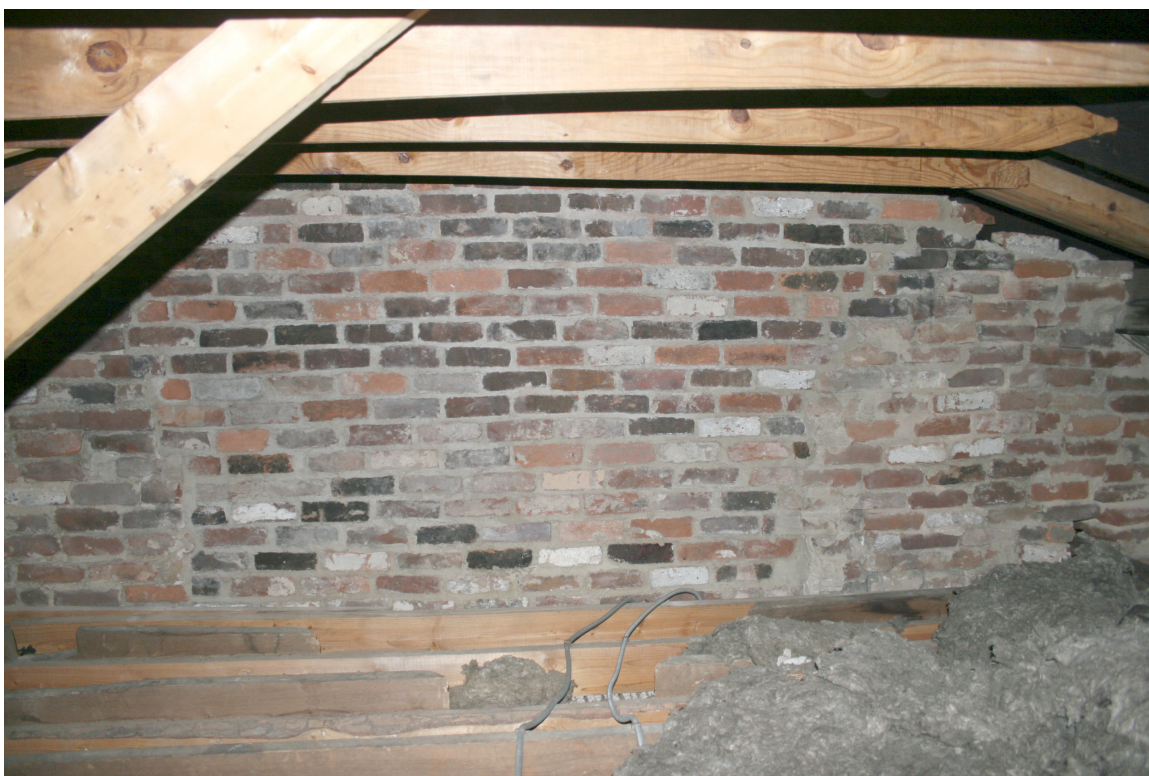
Attic above Room 210, Looking north. Rebuilt brickwork identifies location of c. 1855 chimney.
