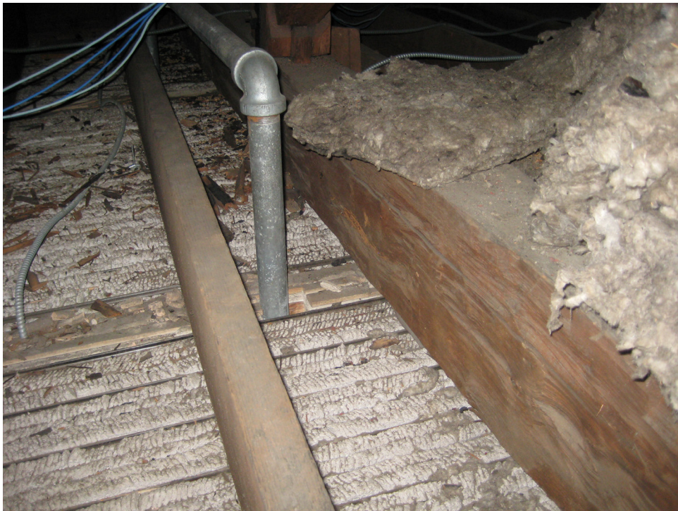
Photo 8 shows the second floor office wing ceiling from the attic side. Note the pipe and electrical wire passages are not fully sealed to prevent a fire spread route.
