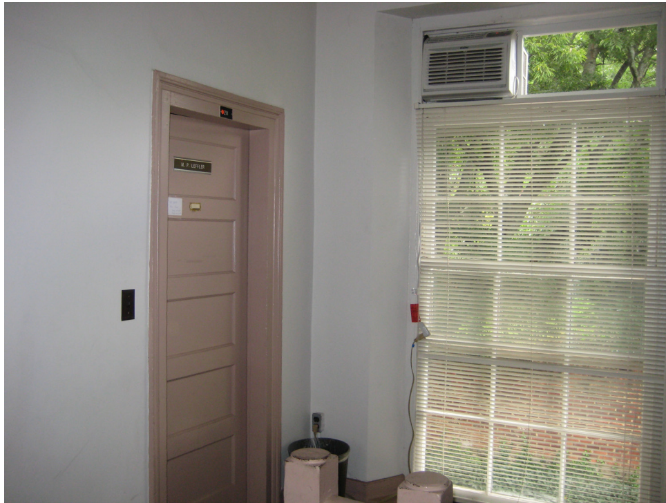
Photo 1 shows an air conditioner in the office section corridor. A dedicated circuit was installed for this unit however the duplex was not placed within reach of the air conditioner electric cord. Consequently an extension cord that is not designed for long term use is needed.
