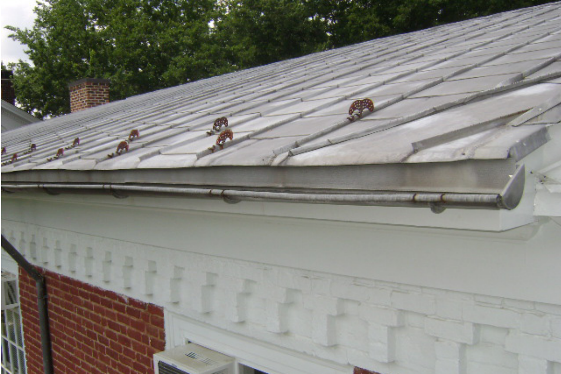
Bent gutter on east eave of Levering Hall
