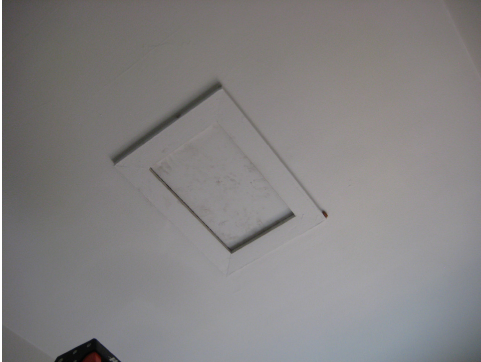
Photo 11 shows the attic access hatch in the office wing. This is a non-rated assembly which can readily fail during a fire and permit fire spread into the attic.
