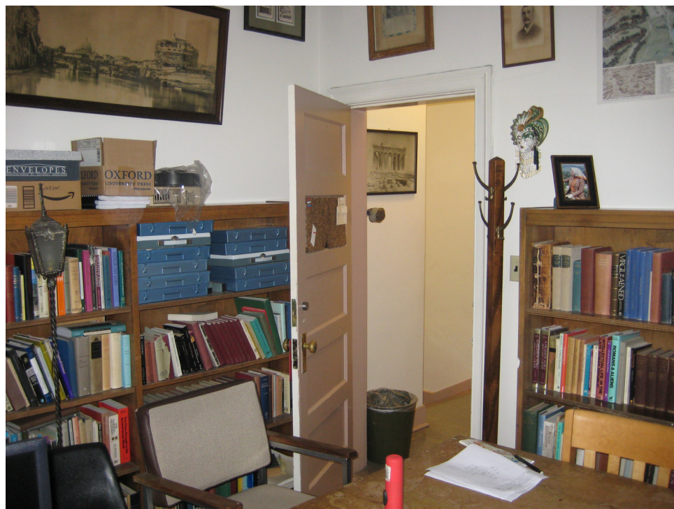
Photo 10 shows a typical office door. The fire resistance is negligible when it is closed, which for some doors is often not the case.
