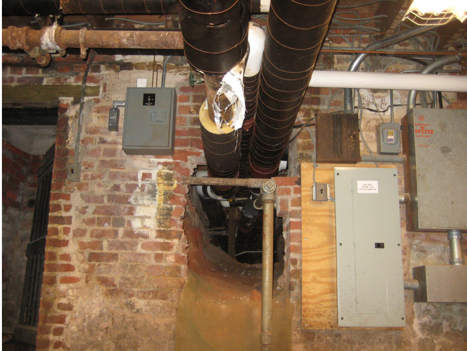
Photo 15 shows the basement mechanical space leading under the residential area. A fire that starts in the mechanical space is a high probability event that will not be contained.
