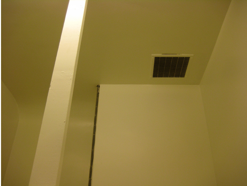
Photo 13 shows a second floor restroom vent that leads into the attic. A fire on the second floor can readily spread into the attic via this opening.
