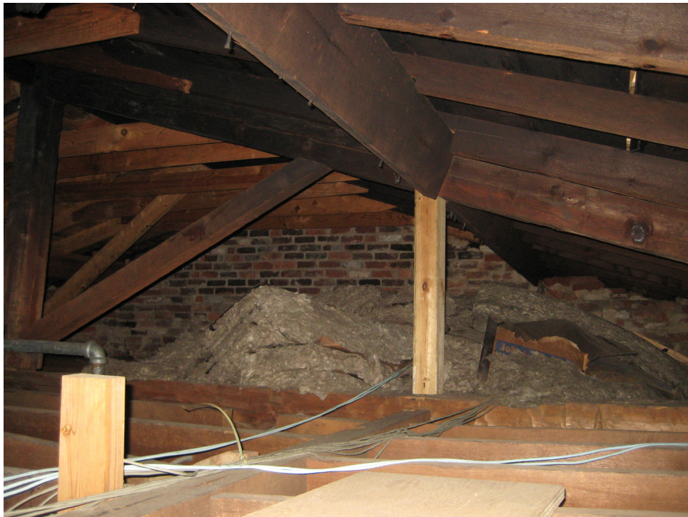
Photo 4 shows combustible framing elements that are found throughout the building
