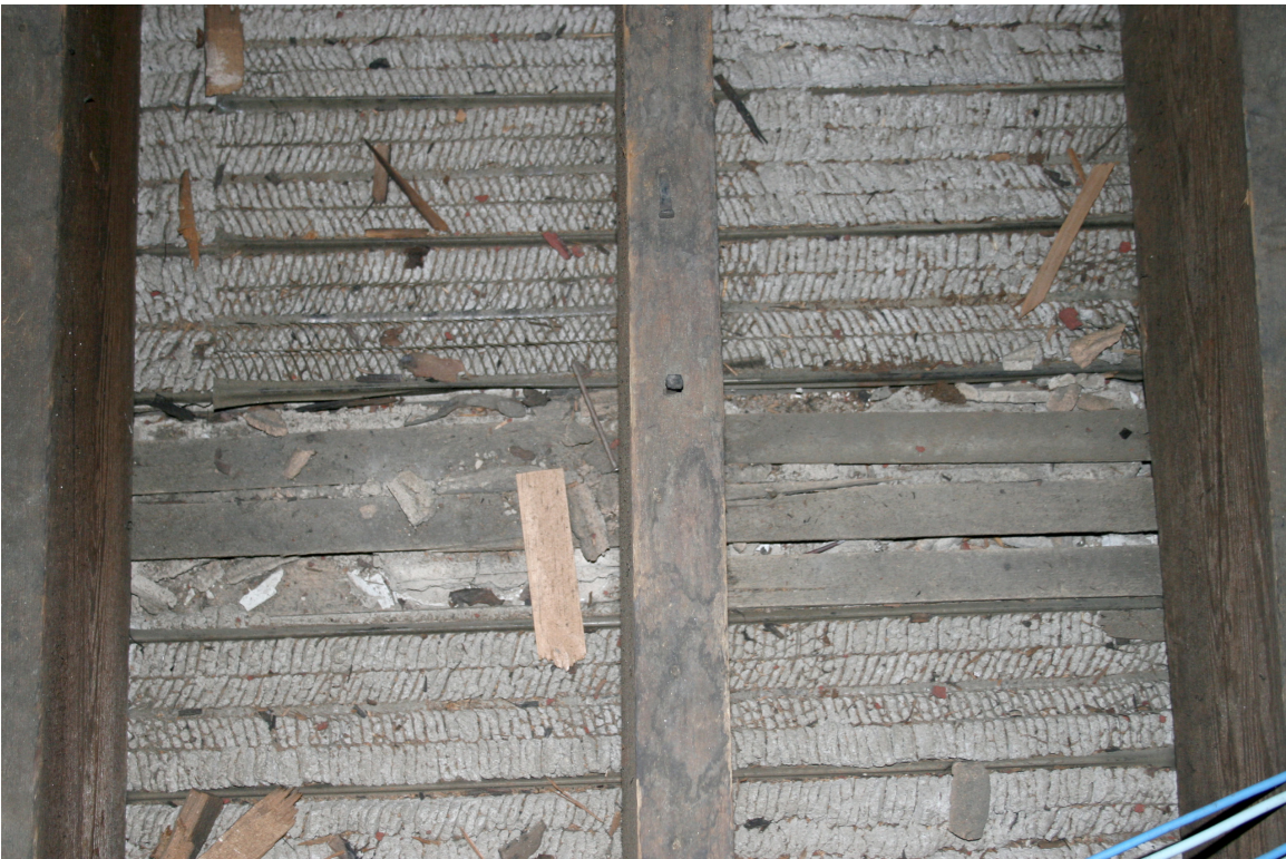
Attic above Room 213. Later walls have encapsulated portions of early ceiling lath and plaster.
