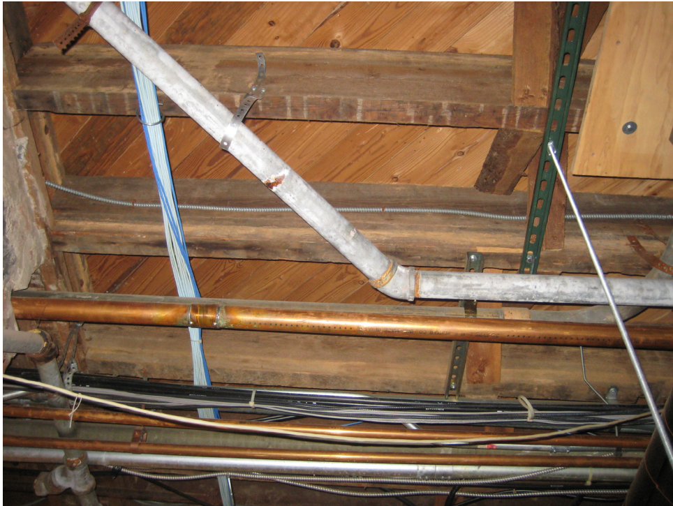
Photo 14. The basement ceiling is unprotected and has numerous cable and mechanical penetrations. A fire that originates in this space will be spread vertically to involve the first floor spaces within minutes.
