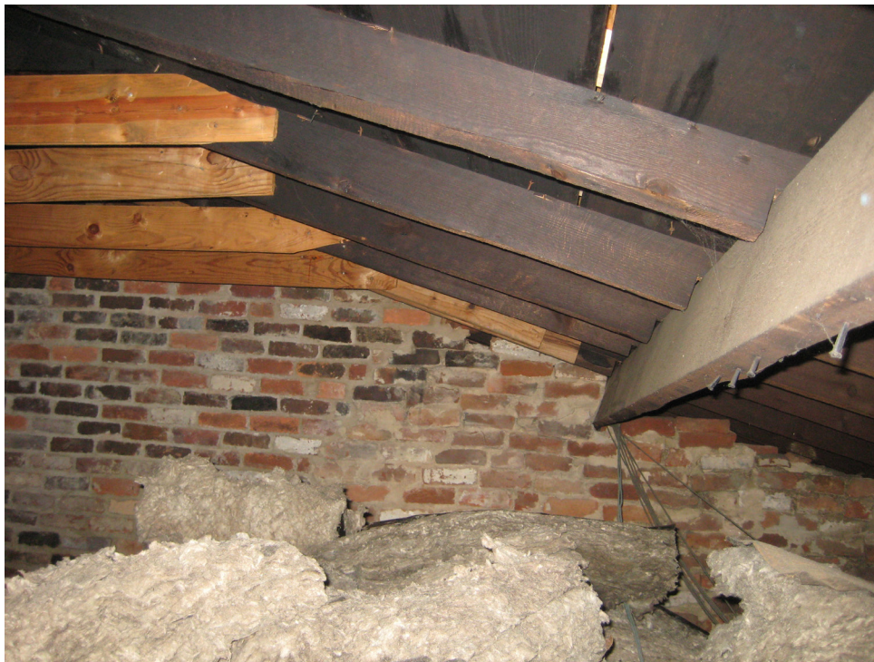
Photo 12 shows an example of an attic opening that will permit a fire to spread from one section of the attic to the adjacent space.
