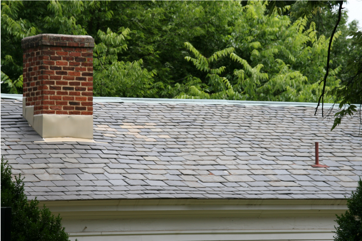
Typical condition of slate roof over Student Rooms
