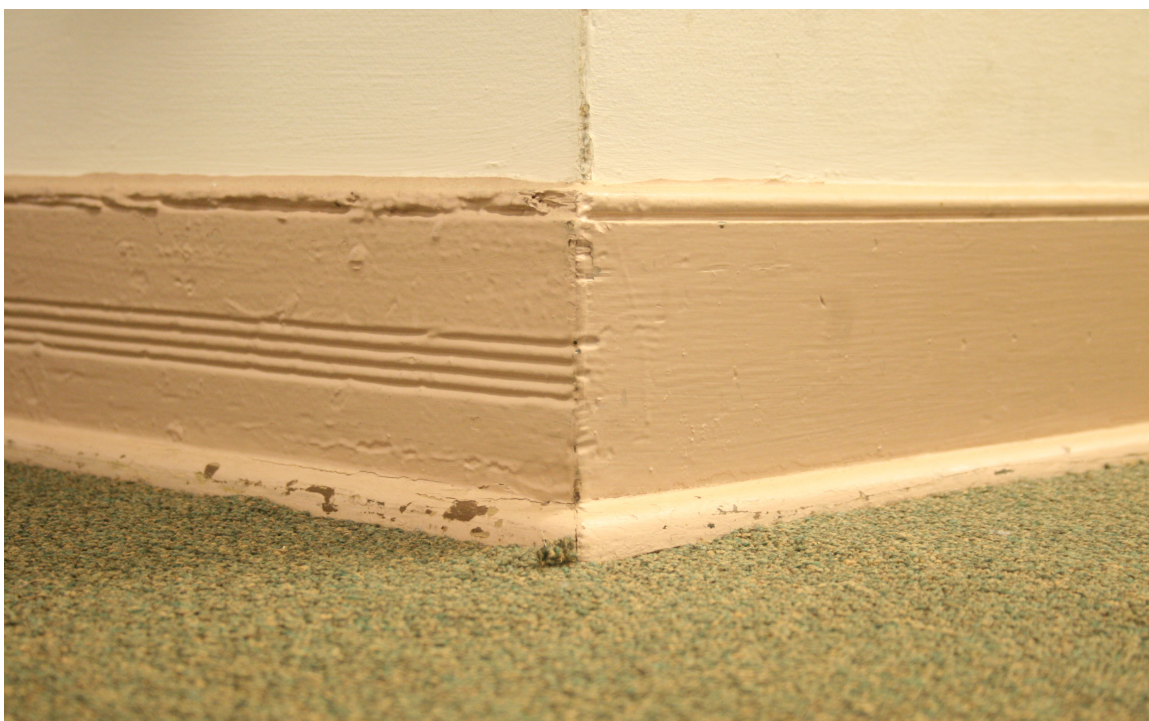
Room 105 Detail of baseboards. Differences reflect various periods of work.
