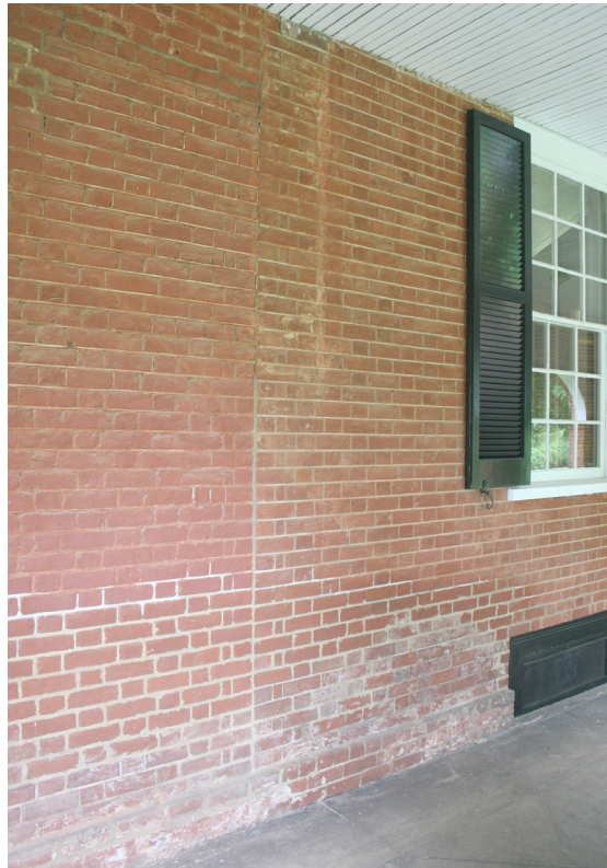
Scars and brick infill where Hotel F and Levering Hall meet
