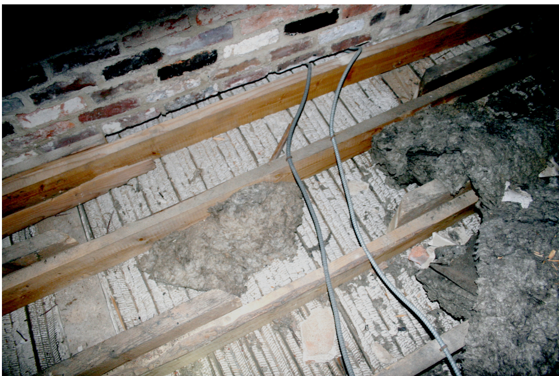
Attic above Room 210, Footprint of angled chimney mass remains in the original ceiling joists.
