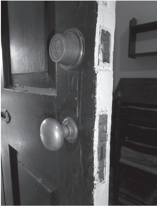
The leading edge of the door to student room 20 is abraded and poorly repaired where it was splintered adjacent to the mortises for the lockset and deadbolt.
