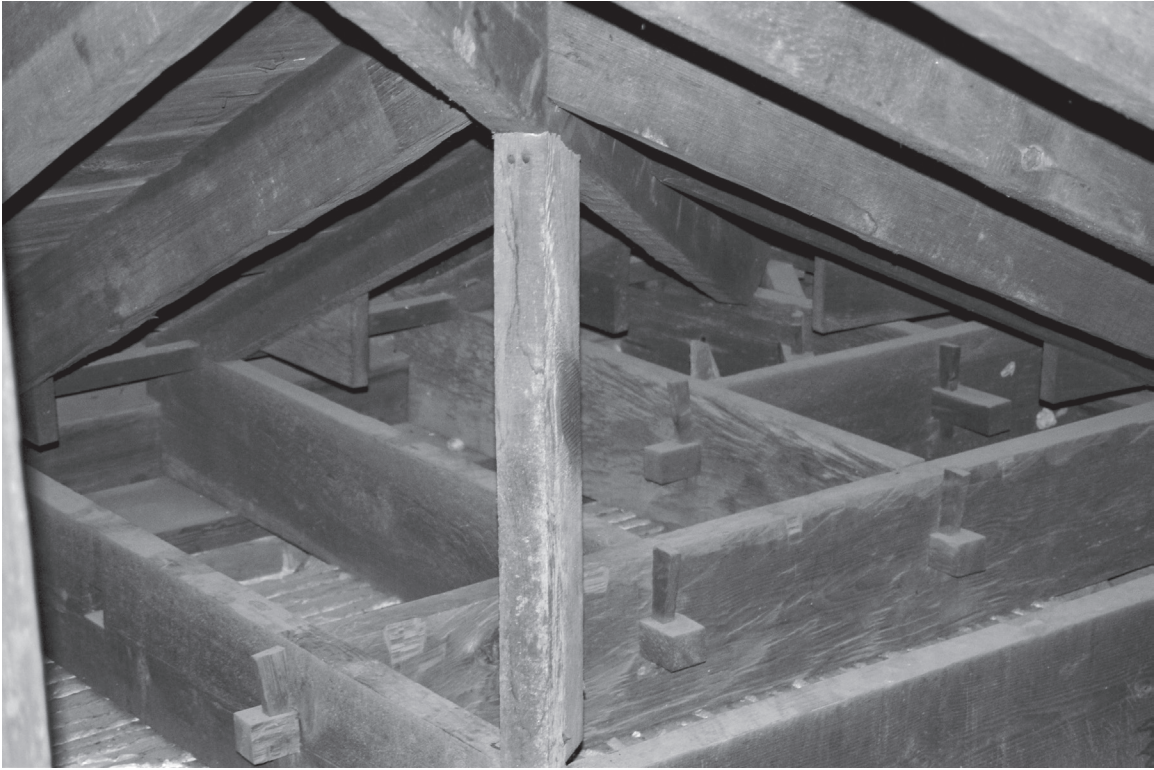
A corner of the hotel attic (above); and a view looking south (left) with the plaster-and-lath ceiling for the arcade to the left, and the metal lath and plaster inside the hotel to the right.
