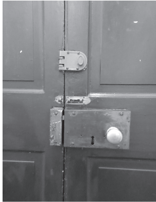
There are multiple generations of hardware on the door leaves at the west entrance; the slide bolt is missing the bolt.
