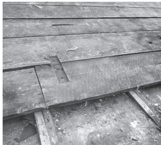
Mortise for parapet bracket in circular sawn, overframed sheathing.
