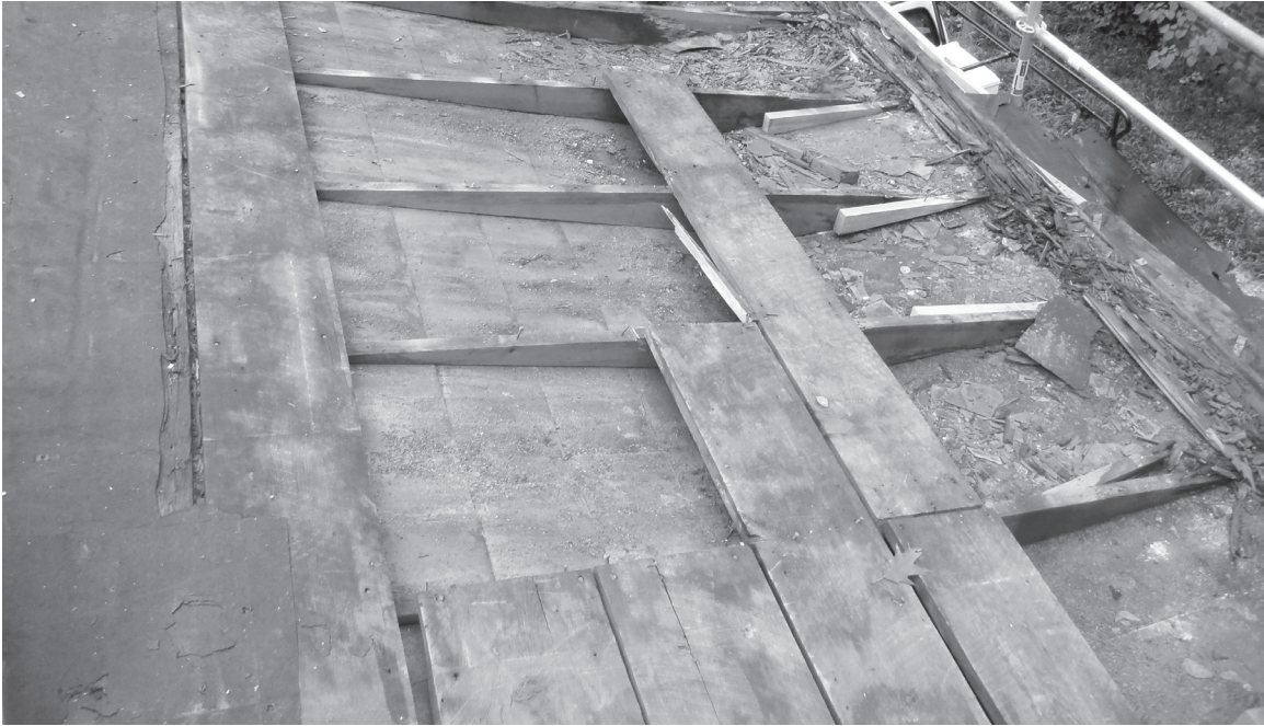
Overframed sheathing partially removed, exposing the tin-plate roofing below.
