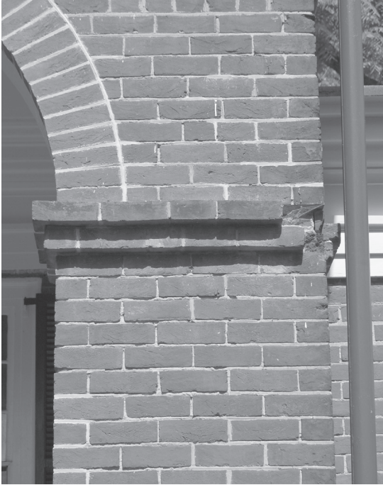
At the northeast corner of the hotel arcade, the corbelled brick at the springline of the arch is missing, and the mortar joints in the brick construction of the northeast pier are eroded.
