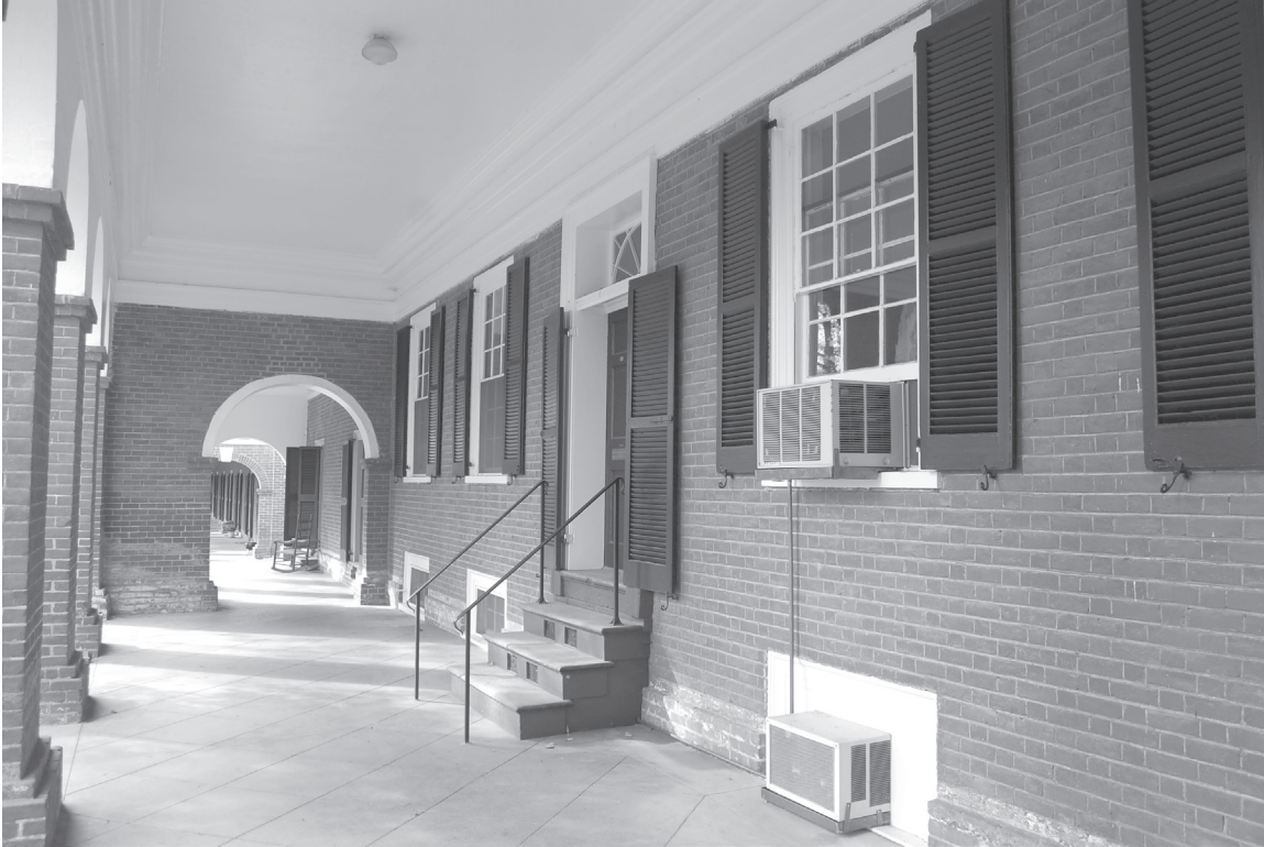
The window air-conditioning units and associated condensate drains on the east elevation of Hotel D are visually obtrusive and historically inappropriate.
