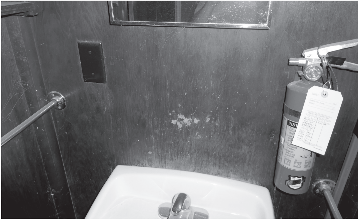
The wood paneling above the lavatory in the northwest corner of student room 20 is water-stained.
