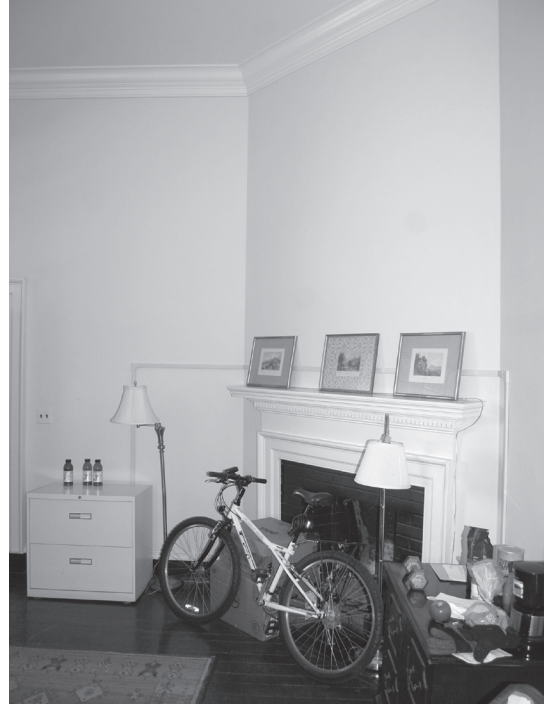
Electrical conduit has been run indiscriminately across wall surfaces. In 102, the conduit has been routed around the fireplace.
