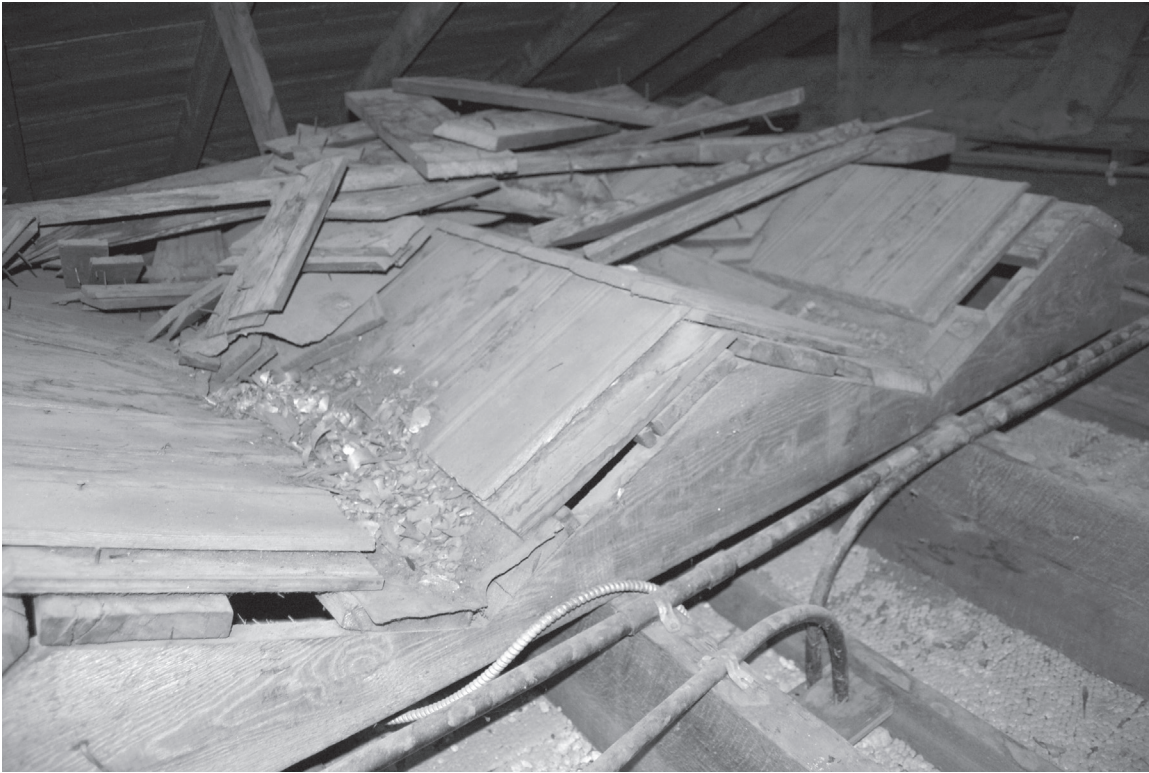
Section of original ridge and furrow roof in south student dormitory attic.
