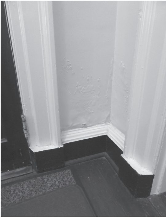
To either side of the west entrance in C101, the plaster above the baseboard is water damaged and friable.
