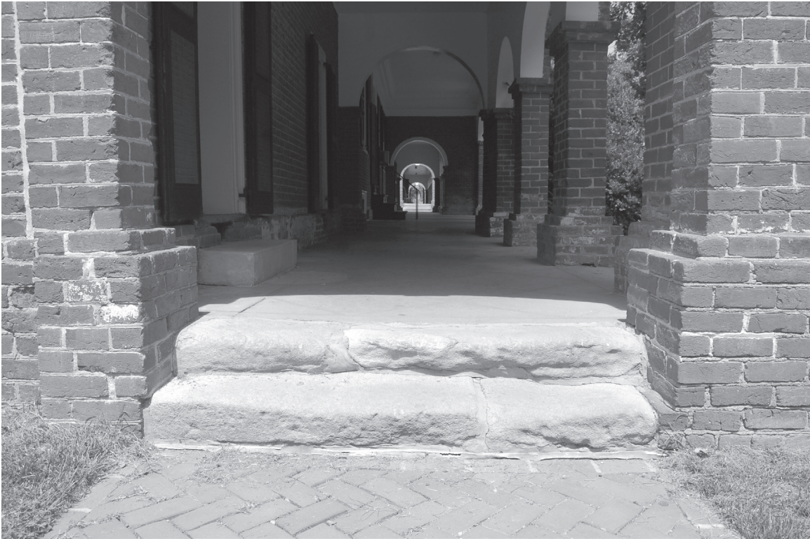
The sandstone steps and pointing at the south end of the arcade are eroded; the brickwork is eroded and spalled.
