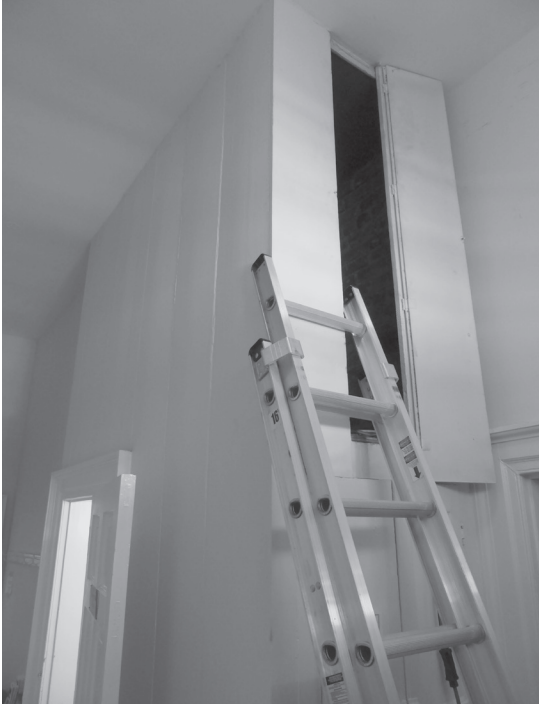
The narrow hinged door panel at the west end of the wood stair enclosure provides restricted access to the attic.
