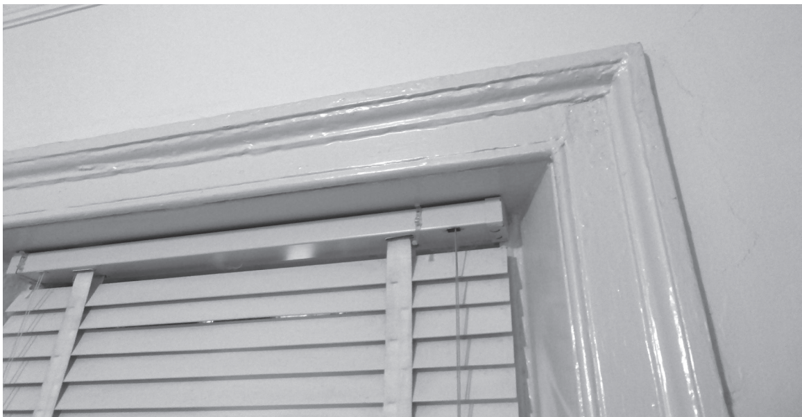
The window and door architraves have excessive paint buildup that obscures the architectural molding profiles, as seen at this window in student room 20.
