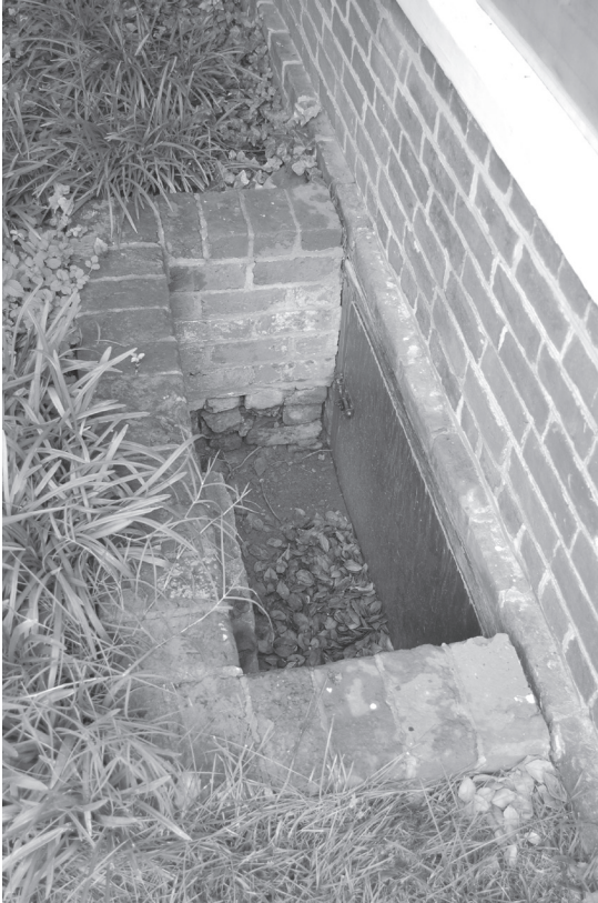
The brick construction of the areaway on the west elevation of the south dormitory is not tied into the wall construction of the building. The lower three courses of brick in the areaway are broken, missing and irregularly laid.
