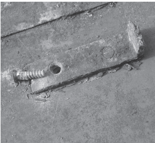
Parapet bracket with hand-cut screw.
