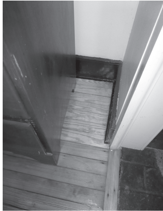
The grain pattern of the replacement flooring in the southeast corner of Student Room 20 is wide and irregular, and does not match the character of the adjacent flooring.
