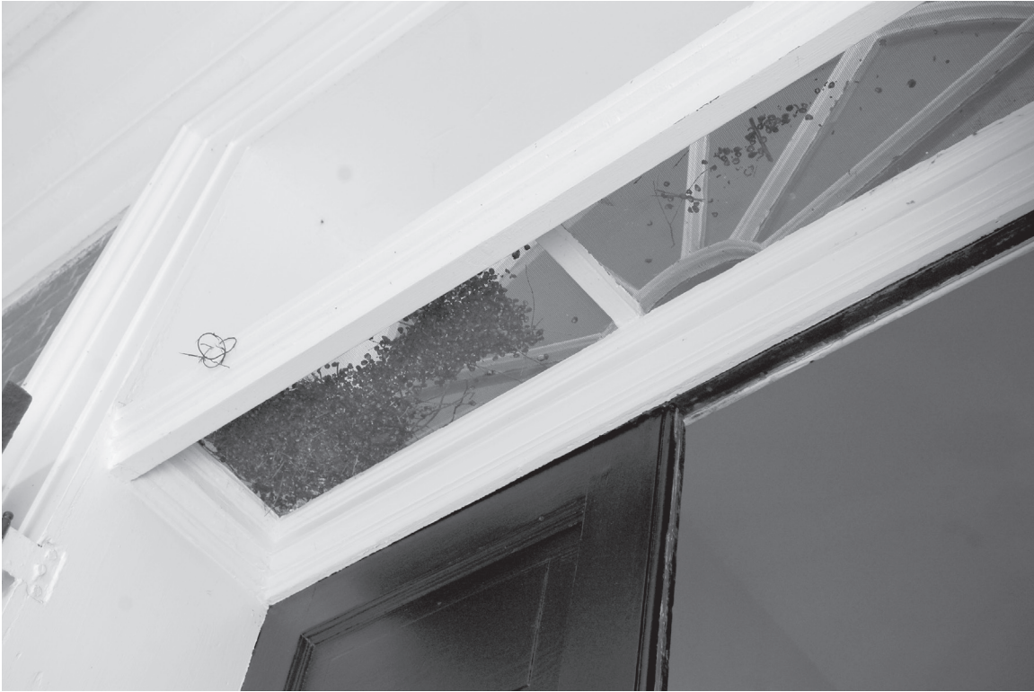
The horizontal screen below the door transom on the east elevation of Hotel D is covered with debris.
