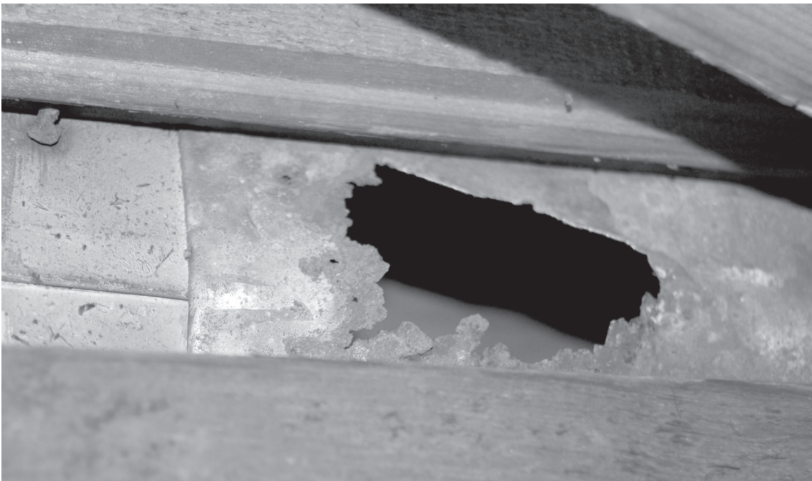
A section of the original tinplate in the south eave of Hotel D.
