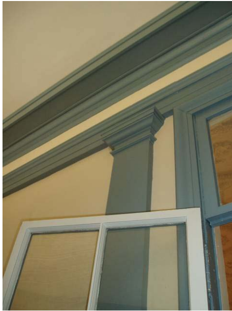
Existing trim at the upper level of the entry lobby, note that the base is extended to a chair rail height
