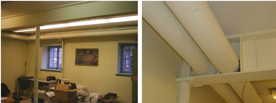
Figure 3: Basement room, SW corner. Note 3½" pipe column & beam
