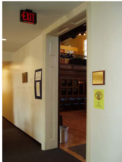
Now all that remains is the paneled jamb and profiled casing.
