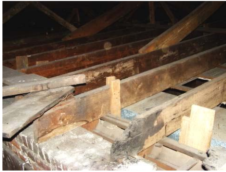
Figure 32: Localized joist bearing deterioration due to fire. Note lack of bridging and locking.
