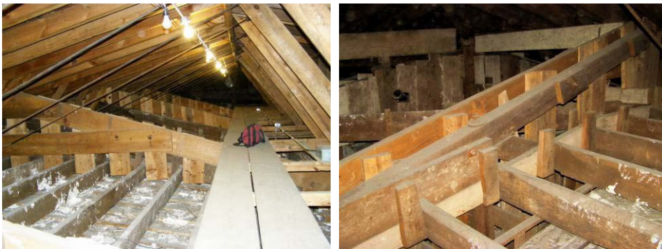
Figure 17: View of attic and roof framing, facing east (Truss A at left).
