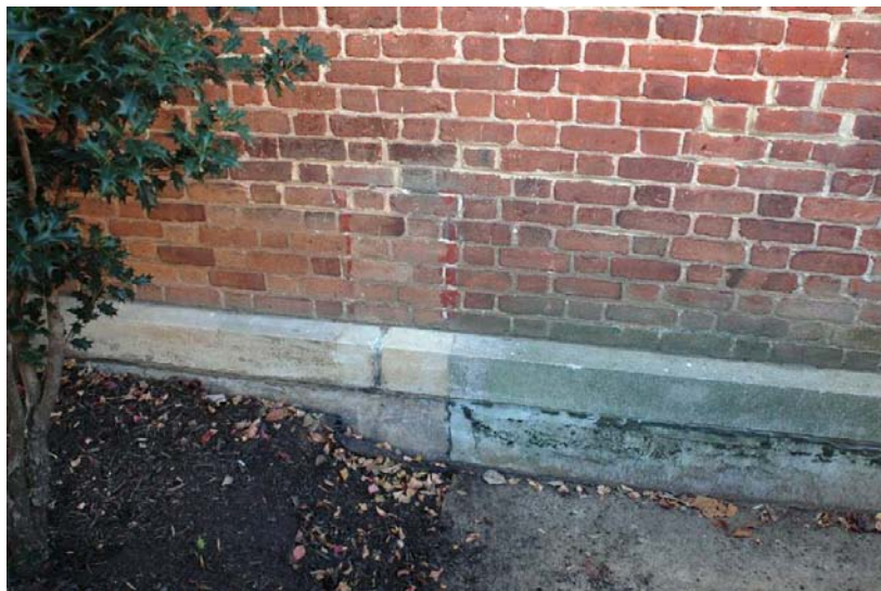
Scar from a previous retaining wall at the rear of the building.
