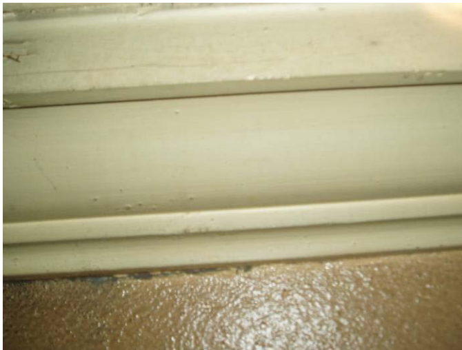
Remnant of original second floor wall and plaster cornice above the southeast part of the building
