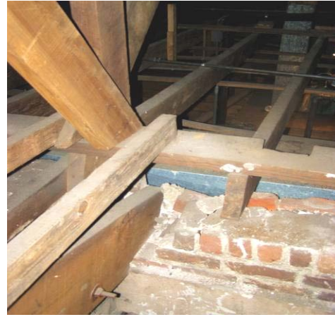
Figure 32: Localized joist bearing deterioration due to fire. Note lack of bridging and locking.
