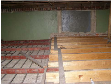
Figure 31: Change in ceiling framing over stairwell renovation.
