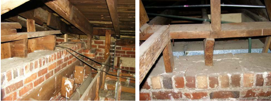
Figure 25: Corridor load-bearing brick masonry wall (left) and western Exterior wall beyond. Note rafters spanning from hip rafter to sill plate, ceiling joists (left) and suspended plaster ceiling over Dining Hall (right). Figure 26: Buckling ceiling joists (southern bay) at interior wall.
