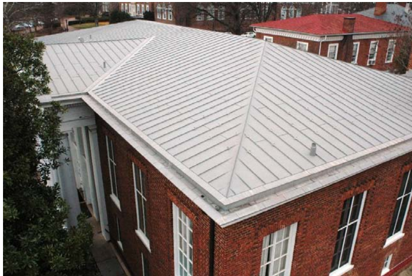
View from Southeast showing built-in gutter.
