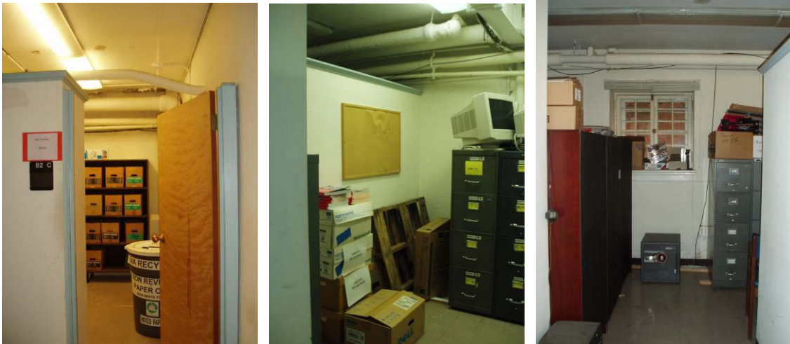
Typical Basement offices with partial height walls and exposed utilities at the ceiling
