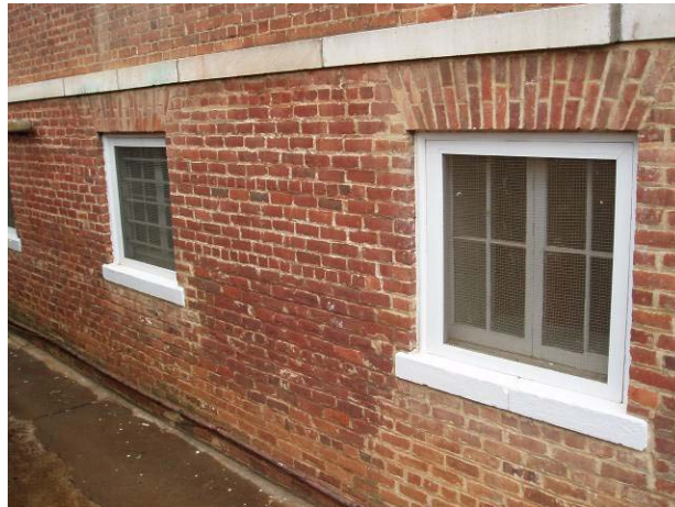
Poor drainage at the northwest corner of the building has caused deterioration in the walls
