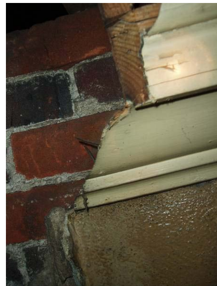
Remnant of original second floor wall and plaster cornice above the southeast part of the building
