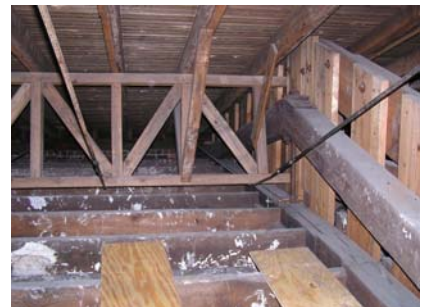
Photo 3: Reinforced Roof Trusses over original refectory hall
