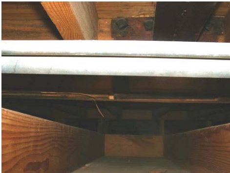
Figure 16: Ceiling and second floor framing at bracket.
