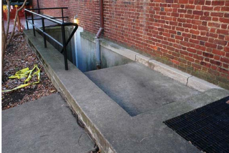
Rear entrance at north elevation
