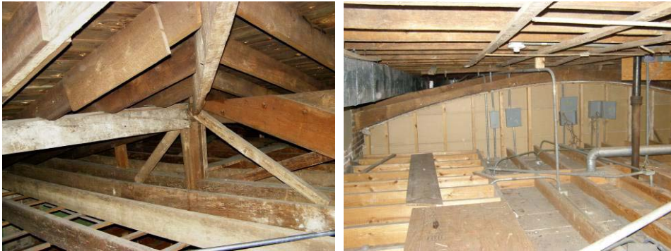
Figure 27: Hip rafter over Truss B in area above Staff Office 202. Figure 28: Looking east at vaulted ceiling spanning southern bay, note two layers of ceiling joists.
