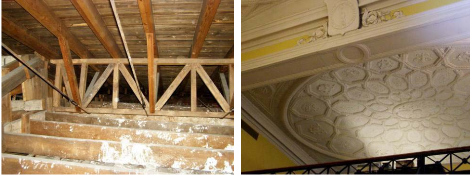
Figure 21: Knee wall truss, northern portion of attic.
