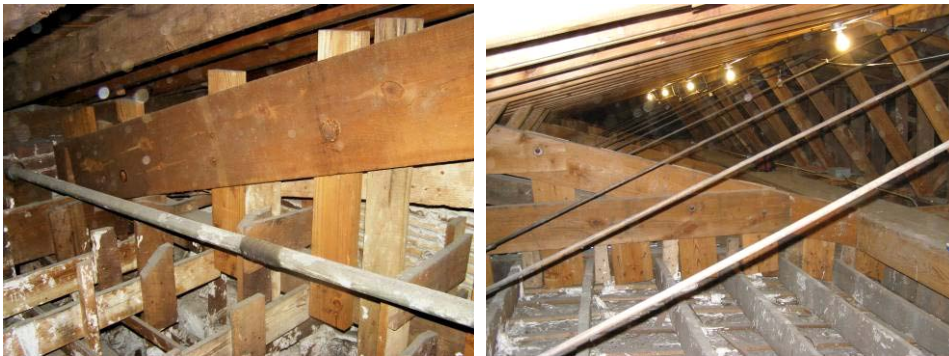
Figure 19: Truss 'A' top chord embedment in north load-bearing masonry wall beyond. Note timber hangers for suspended ceiling below.
