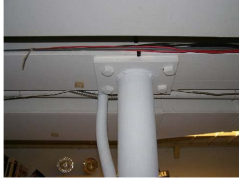
Figure 9: Steel post in basement office.
