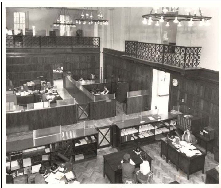
The 1959-60 design placed a mezzanine or balcony at the east end of the great hall matching the original one at the west end of the room and blocking the large fireplace on the east wall. Within the enclosed space was a large office which was subsequently converted to a conference room. The open space between the two mezzanines was subdivided with office partitions and counters.
