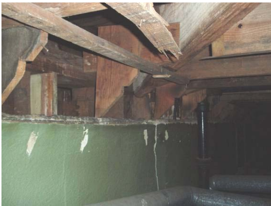
Form work for the historic plaster cornice above the now dropped ceiling over the southwest corner
