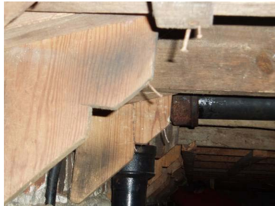
Form work for the historic plaster cornice above the now dropped ceiling over the southwest corner
