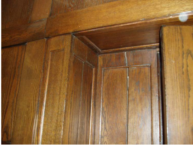
The doorway at the west end of the Great Hall originally contained double swinging doors; but has been altered to accommodate a single door.
