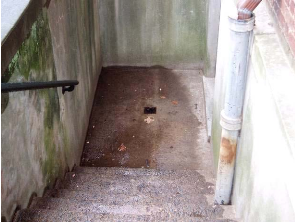
Floor drain and downspout at the exterior stair on the north side of the building
