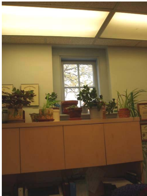
Offices are finished out with dropped acoustical ceilings and recessed fluorescent lighting fixtures
