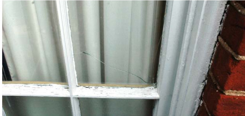
Most of the larger casements have at least one or two broken panes of glass and rot at rails and muntins in selected locations.
