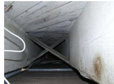
Photo 13: First Floor Framing – Note cross-bridging and diagonal subfloor boards
