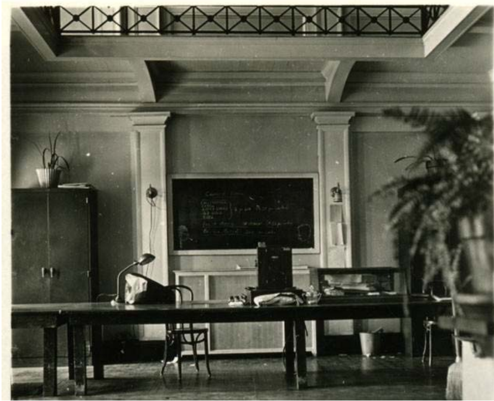
Historic photograph of the open Entrance Hall looking west; note the pilasters, cornice, and the balcony brackets and railing above.
