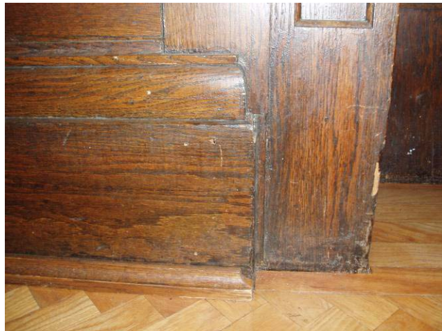
These photographs show the base board at the bottom of the wood wainscot in the Great Hall; taller than the remaining piece in the Entrance Hall but with a similar profile. Also visible is the historic wood, herringbone flooring; now stripped to a much lighter color than what is visible in historic photographs.
