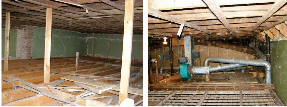
Figure 29: Hangers connect upper and lower ceiling joists.
