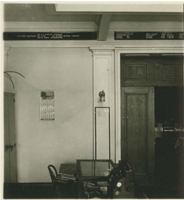
This historic photograph documents the original door and transom leading from the Entrance Hall into the Great Hall, as well as the pilasters, baseboard and cornice trim.
