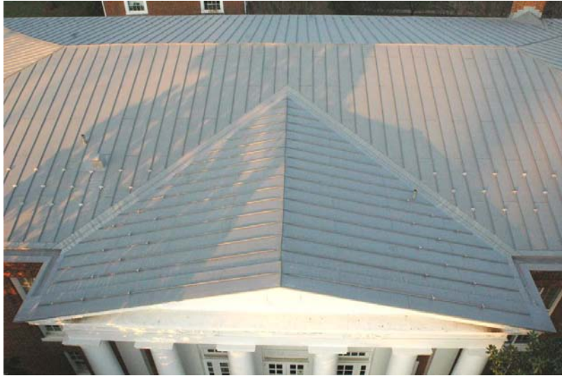
View of roof from south side.
