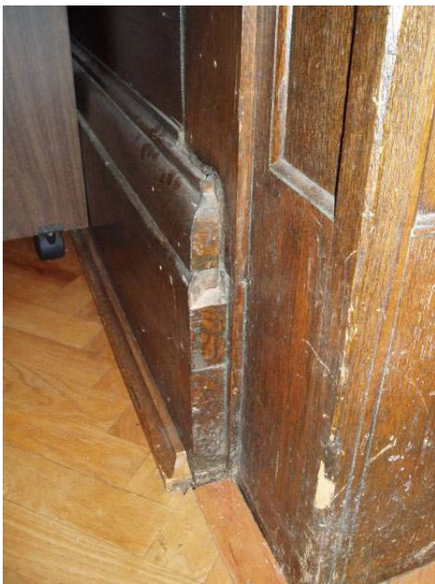
These photographs show the base board at the bottom of the wood wainscot in the Great Hall; taller than the remaining piece in the Entrance Hall but with a similar profile. Also visible is the historic wood, herringbone flooring; now stripped to a much lighter color than what is visible in historic photographs.
