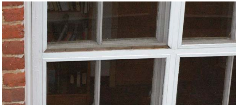
Most of the larger casements have at least one or two broken panes of glass and rot at rails and muntins in selected locations.
