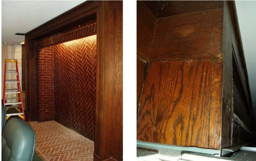
The dropped ceiling under the added west mezzanine obscures the upper part of the Fireplace Surround. The photo on the right shows what remains above the ceiling.
