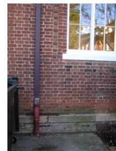
Photo 10: Downspout and Dumpster North of East pilaster
