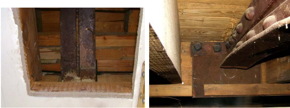
Figure 14: Probe at front corridor ceiling (C108), viewed from below. Note bottom flange of Hall north bracket.
