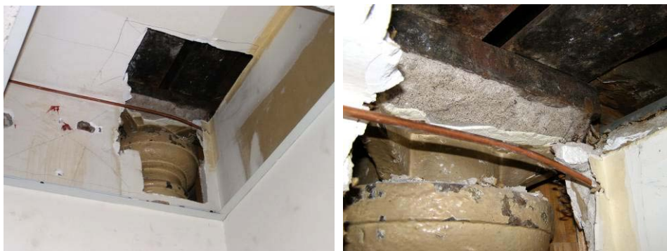
Figure 12: Probe at cast iron column
