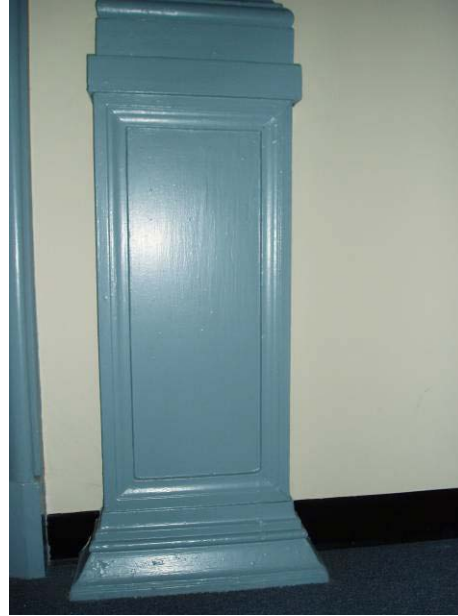
Existing trim at the upper level of the entry lobby, note that the base is extended to a chair rail height
