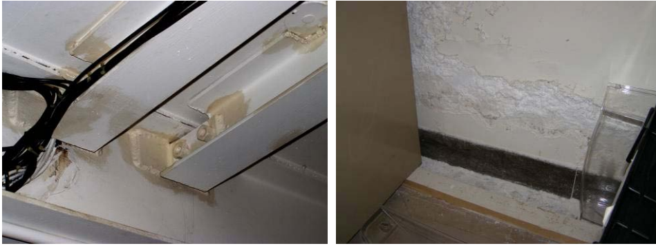
Figure 5: W5 steel beams spanning from west wall to steel beam.
