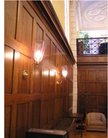
Photo 4: Interior face of North wall, with 1 st floor level wood paneling – Area of inward bowing.
