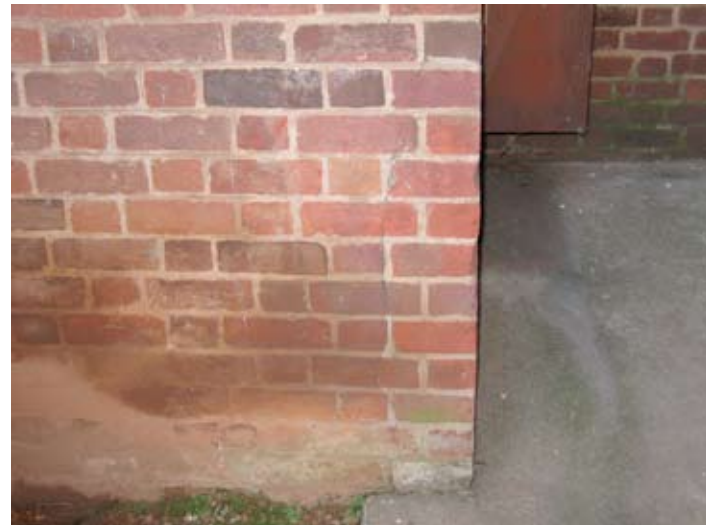
Minor brick cracks
