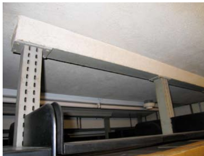
1936 Building Stacks 3 rd Tier Transfer Beam
