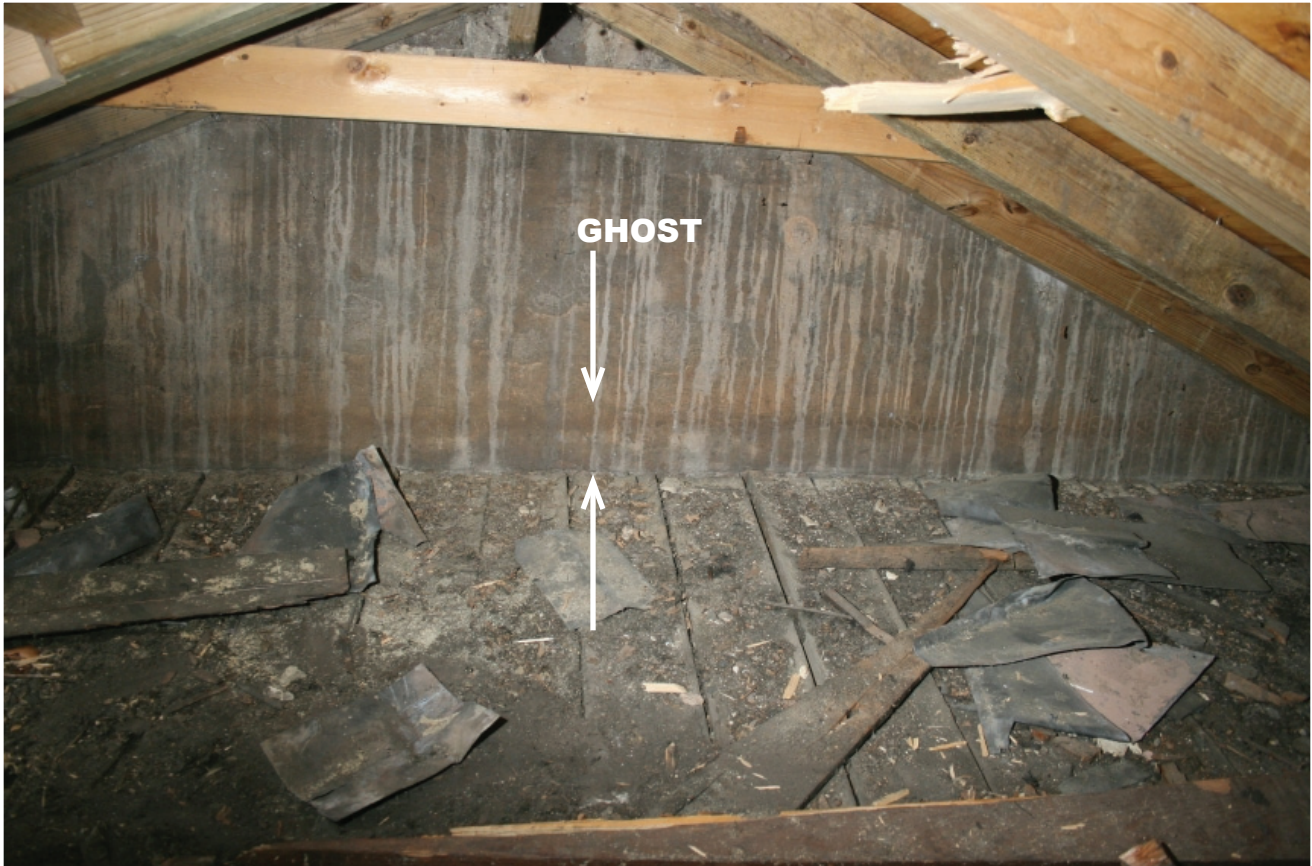
Figure 4 The ghost line along the south stuccoed wall of Pavilion III is believed to be evidence of a deck that would have been placed over the serrated roof.
