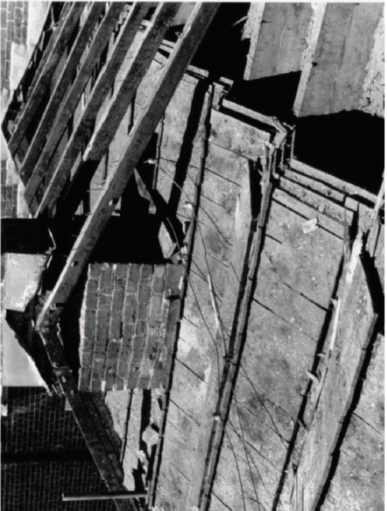
Figure 9 This photograph of the exposed serrated roof above the student rooms to the south of Pavilion III was taken in the 1980s when the upper slate roof was removed.
