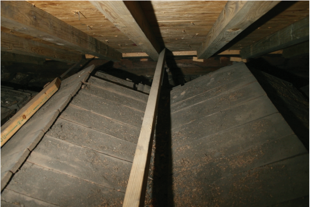
Figure 3 Photograph looking west in the attic above the student room showing the original serrated roof.
