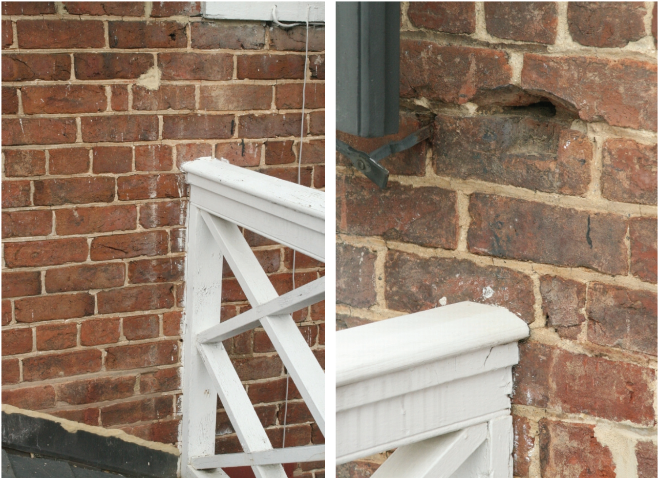
Figures 1 & 2 Evidence of original Chinese rails as found on flanking walls of pavilions. The image on the right shows how the brick was carved away where the original railing met the south wall of Pavilion IX. The image on the left displays a ghost of the original rail on the north wall of Pavilion X as a result of paint marks left on the brick. A patch of mortar covers where an iron pin would have originally been embedded in the wall to assist in securing the end of the rail.
