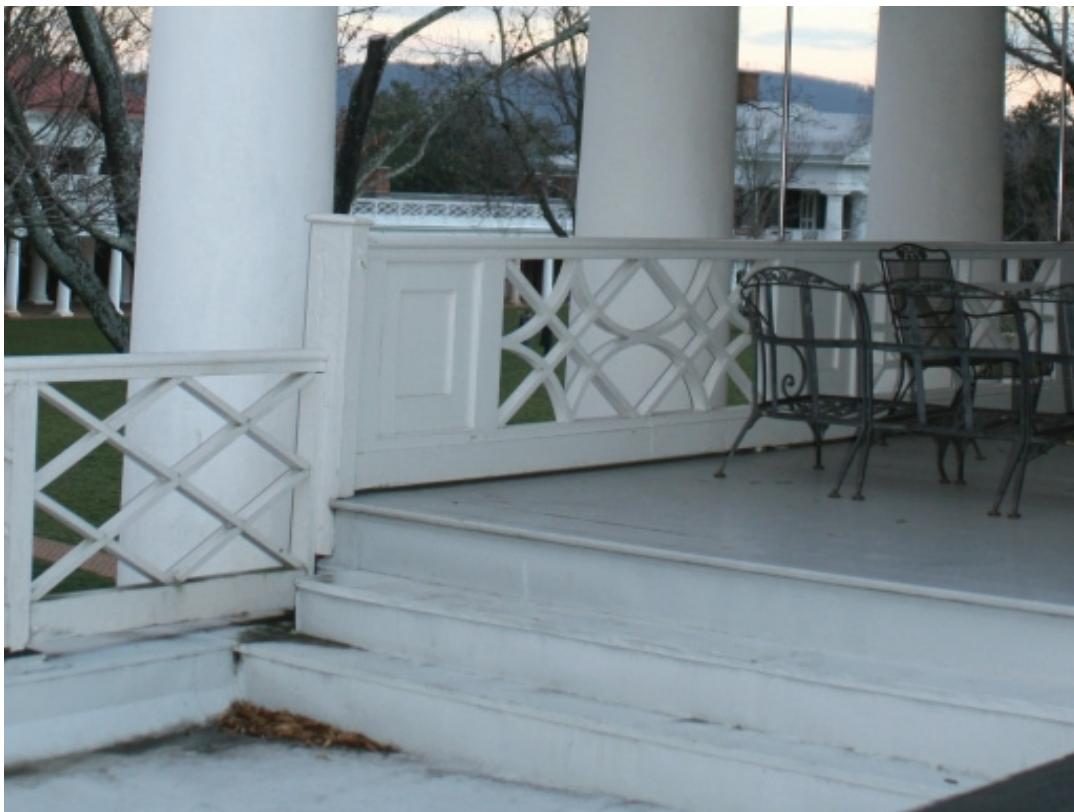
Figure 13 The end post that separates the pavilion rail with the student rail appears to be later, and is believed to have been constructed when the iron rails were installed in the mid-19th century.
