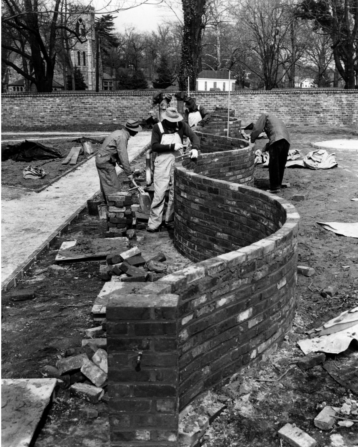
Figure 8.5 Workers make progress on constructing the Pavilion V Garden walls, including this mid-garden serpentine wall that divides the garden into two sections, in this undated ca. 1951 photograph. In the spring of 1952, all five of the West Gardens were finished. (R-JAV-SCL-DSC-nd-Box44Env1712-BW-4-PavVserpwall c1952.jpg)
