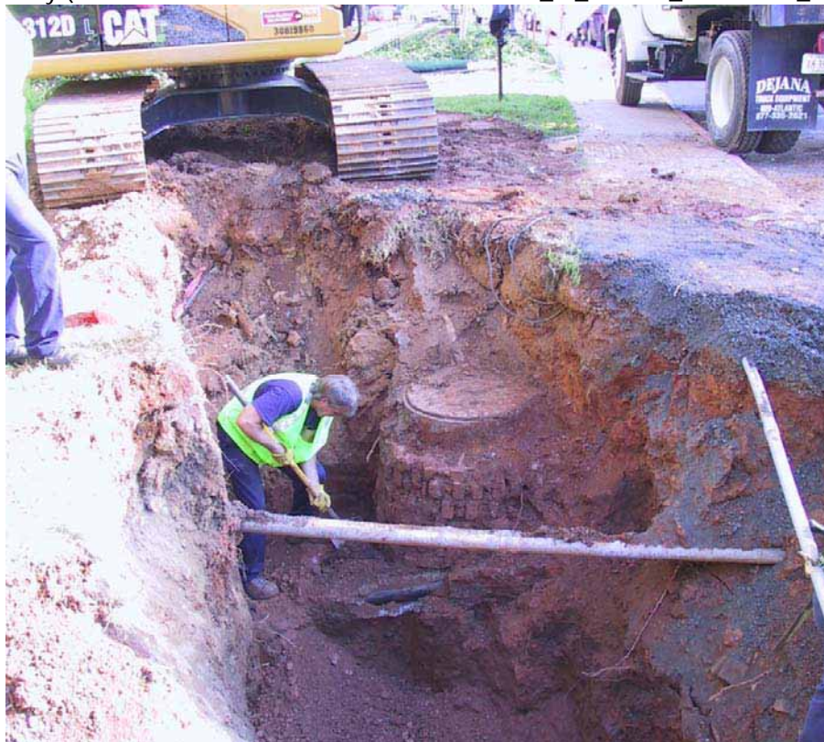
Figure 6.3 Cobblestone-and-brick manhole located off the Southeast Corner of Alderman Library near McCormick Road. The manhole cover is several feet below the 2013 grade. (R-JAV-ARCH-RAS-2009-2-1886-C-2-McCormick_Road_Manhole.jpg)
