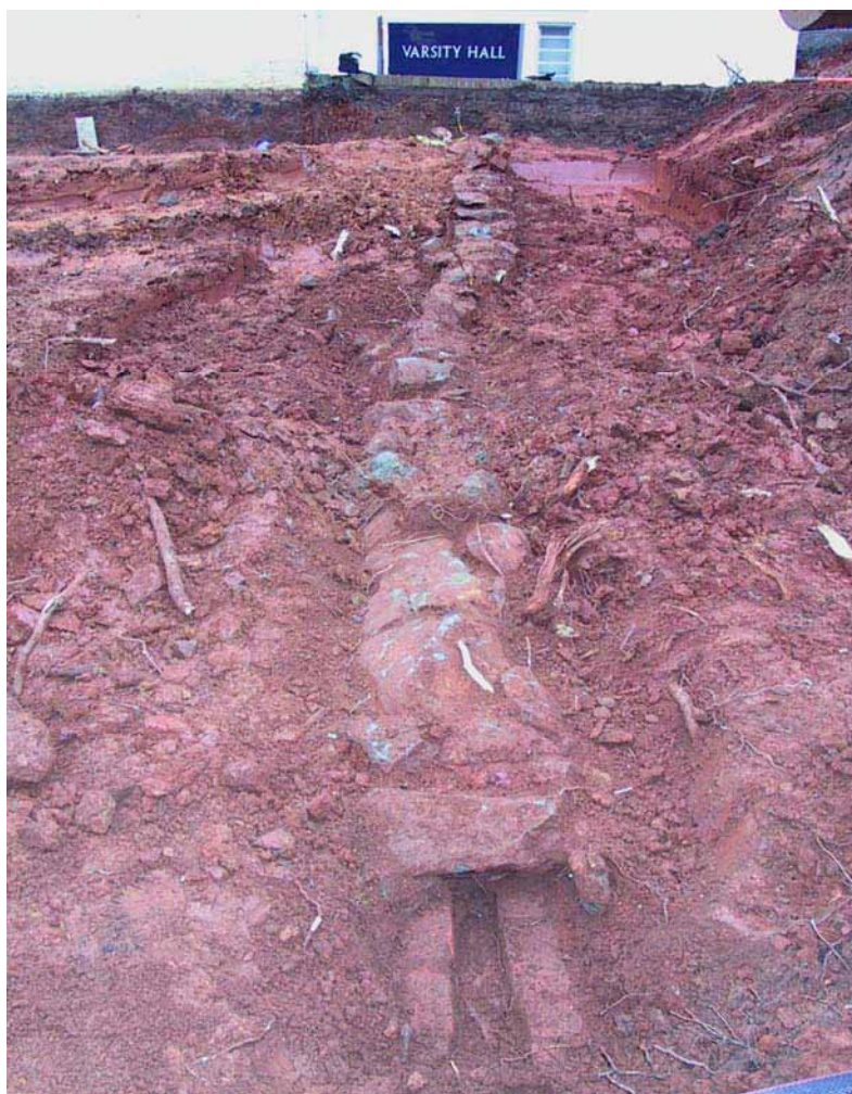
Figure 4.20 This photograph, looking southwest towards Varsity Hall, shows a remnant stone-capped brick-box drain. (R-JAV-ARCH-RAS-2005-3-1859-C-5-Varsity_Hall_Stone_Capped_Brick_Box_Drain.jpg)
