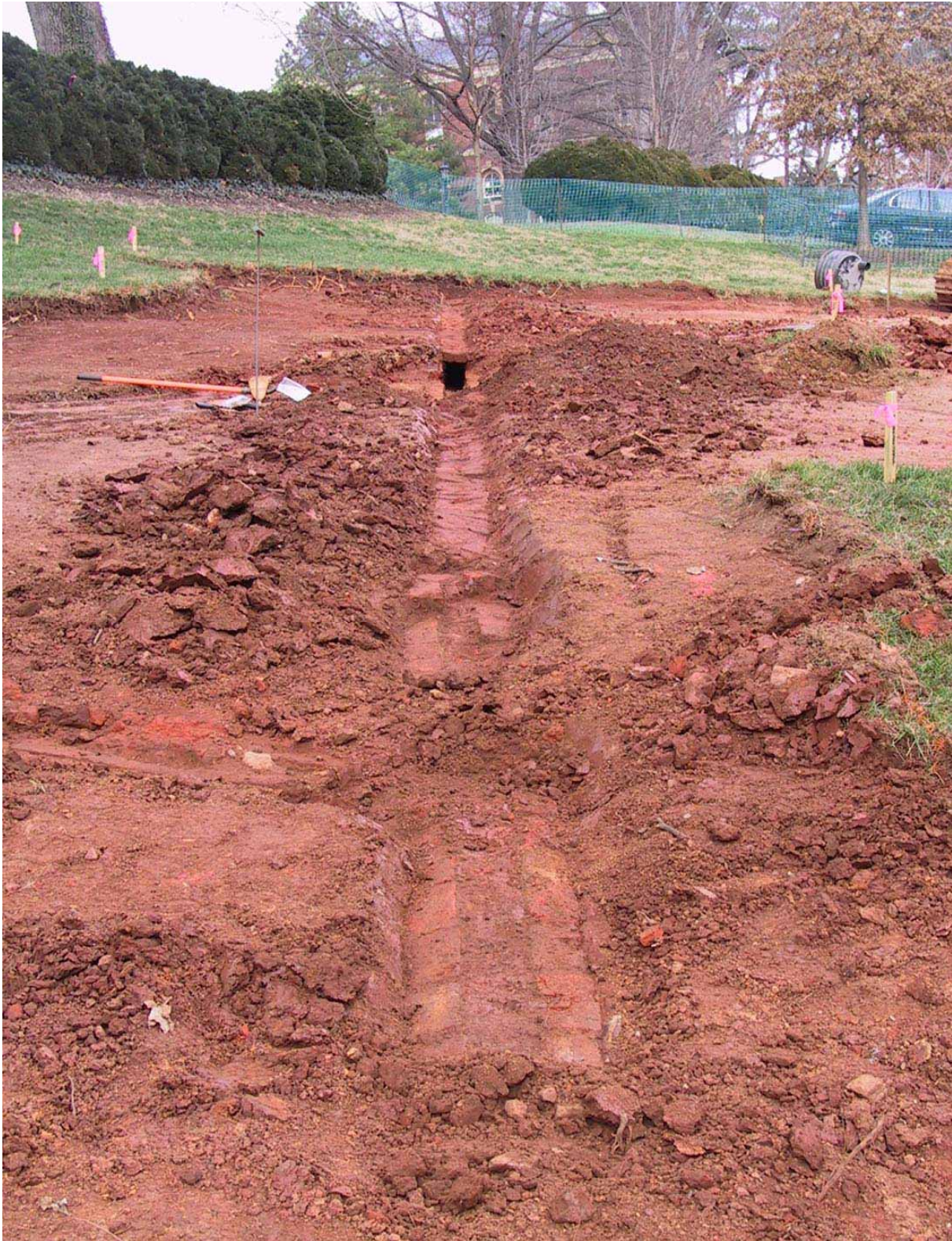
Figure 3.17 This photograph, looking northwest toward Brooks Hall from Hospital Drive, shows a remnant brick-box drain with targeted interior that served to drain Rotunda Alley. The box drain was part of a larger network of drains that emptied to the southeast. (R-JAV-ARCH-RAS-2005-3-1825-C-5-Hospital_Drive_Brick_Box_Drain.jpg)
