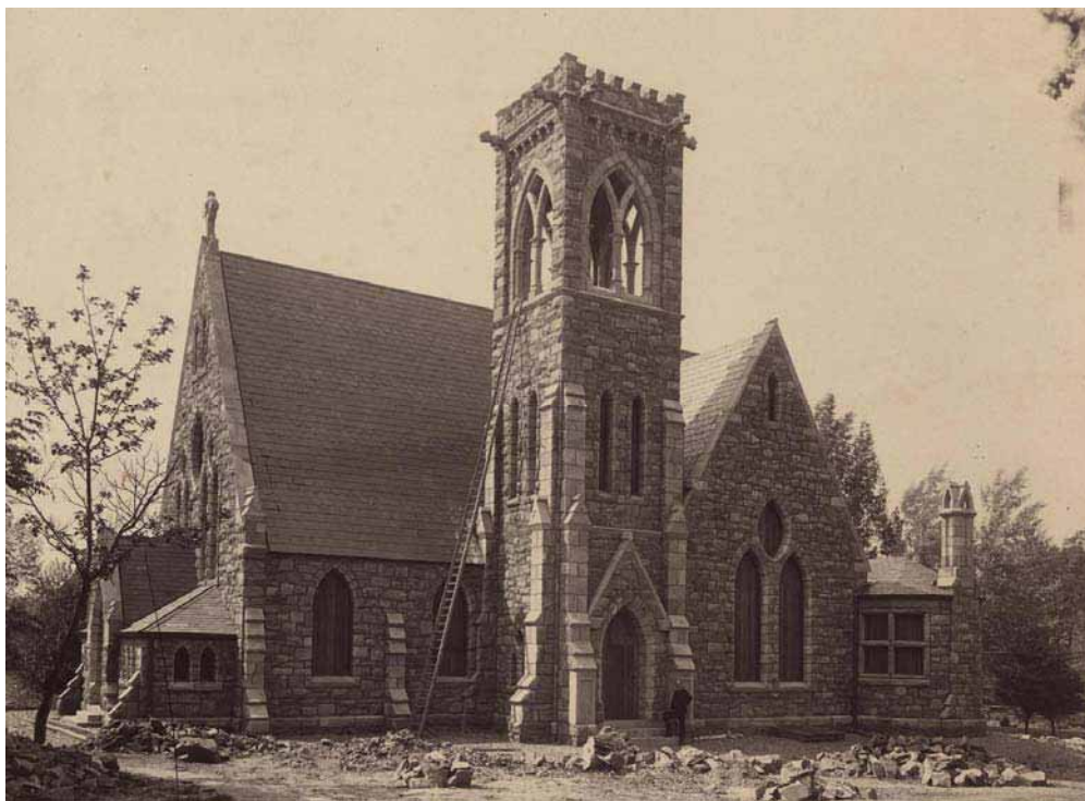
Figure 6.12 This 1889 image shows the construction of the University Chapel. Stones and rubble cover the ground surrounding the new building. (R-JAV-SCL-OVH-1889-prints07853-BW-2 Chapel Construction.jpg)
