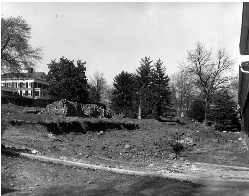
Figure 8.16 Extensive ground disturbance is underway in preparation for a retaining wall. Bricks are stockpiled above the grading activity to be used for reconstructed serpentine and straight garden walls. (R-JAV-SCL-DSC-1962-03-08-Box44Env1702-BW-3-EGardenRest.jpg).
