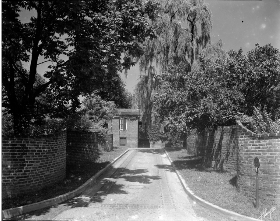
Figure 7.9 In September 1922, the "alleys and drives between West Colonnade and West Range" were paved "with concrete and brick in the same manner as the Poe walk." (R-JAV-SCL-HSC-nd-c1920s-Y26678EB-BW-3-AlleyDecorativePaving.jpg)
