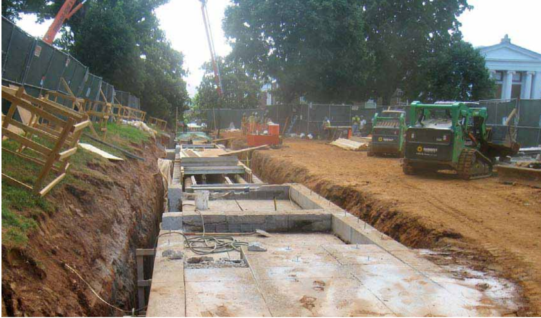
Figure 9.17 A large subsurface utility corridor at the foot of the southernmost terrace of The Lawn was upgraded for emergency vehicle access in 2012. Construction activity was focused on the immediate area and archaeological monitoring was carried out. (R-JAV-HL-2012-07-06-33-C-5-PathUtilityExcavation.JPG).
