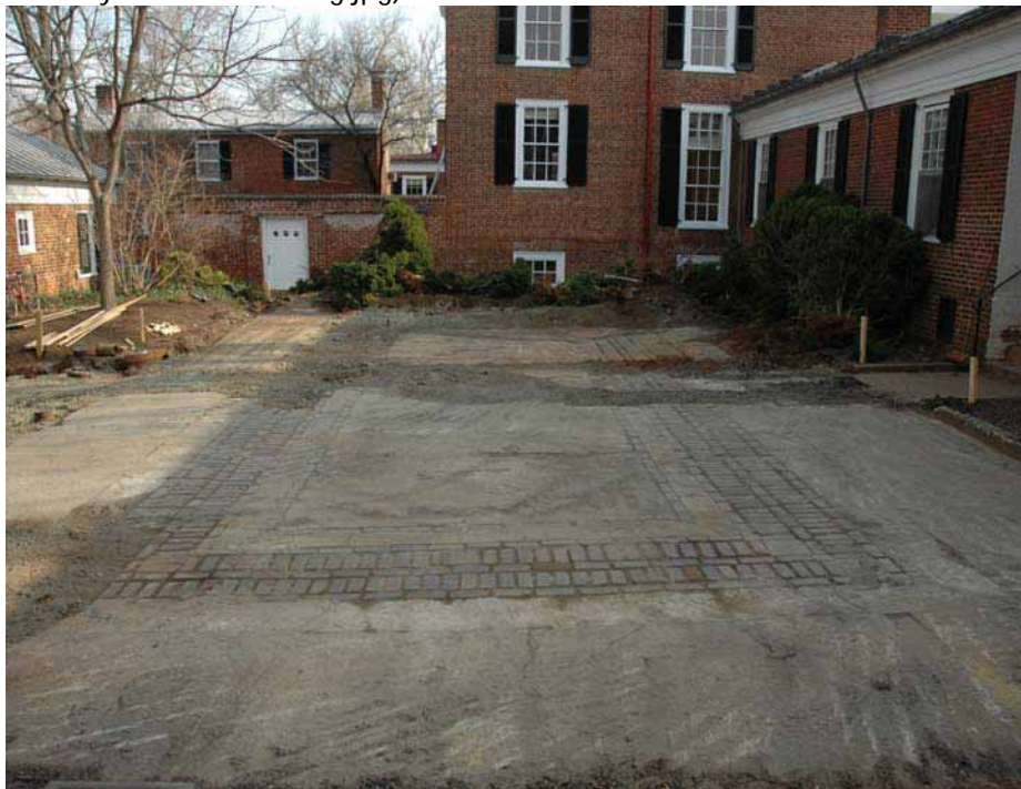
Figure 7.10 Concrete and brick paver surfacing was identified directly below a later cover of asphalt. In the Pavilions III and V courtyard, the surfacing consisted of a single rectangular-shaped band of brick, approximately 32 inches wide and set 6 feet inside of the concrete curbs. (R-JAV-ARCH-RAS-2009-1-1922-C-4-Courtyard_III-V_Concrete_and_Brick_Paver_Surfacing.jpg).
