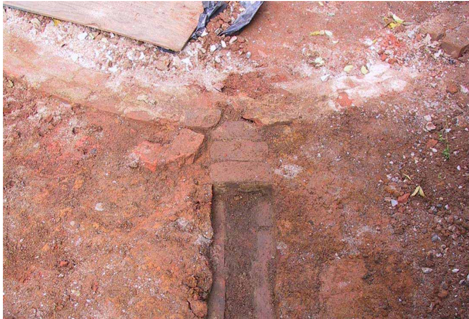
Figure 4.8 This photograph, looking north-northwest, shows a remnant brick-box drain with interior pargeting leading from a non-extant downspout from an adjacent dormitory, to the brick cistern. (R-JAV-ARCH-RAS-2006-2-1833-C-4-Courtyard III_V_Brick_Box_Drain.jpg)
