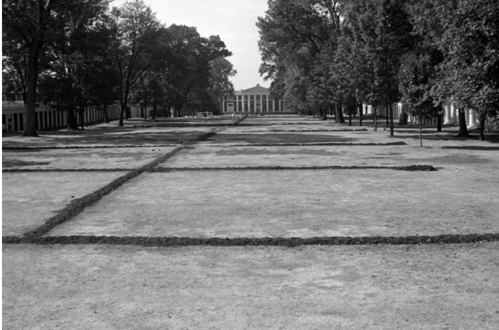
Figure 8.28 Linear trenches for irrigation pipe installation mark the Lawn in this 1967 view. (R-JAV-SCL-DSC-1967-09-11-Box22Fol0846Neg26-BW-1-LawnSprinklerInstallation.jpg).
