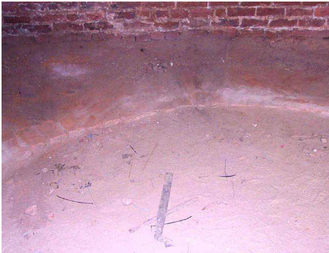
Figure 3.30 This photograph, taken in the interior of basement level East Lawn Room #24, shows the top of a circular buried brick cistern. (R-JAV-ARCH-RAS-2007-1-1822-C-3-East_Lawn_Room_24_Cistern.jpg)
