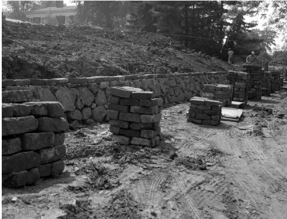
Figure 8.18 A stone retaining wall has been constructed to hold the cut in the slope and brick wall building is in process. (R-JAV-SCL-DSC-1962-Box46Env1837-BW-3-ERangeStoneWall.jpg)
