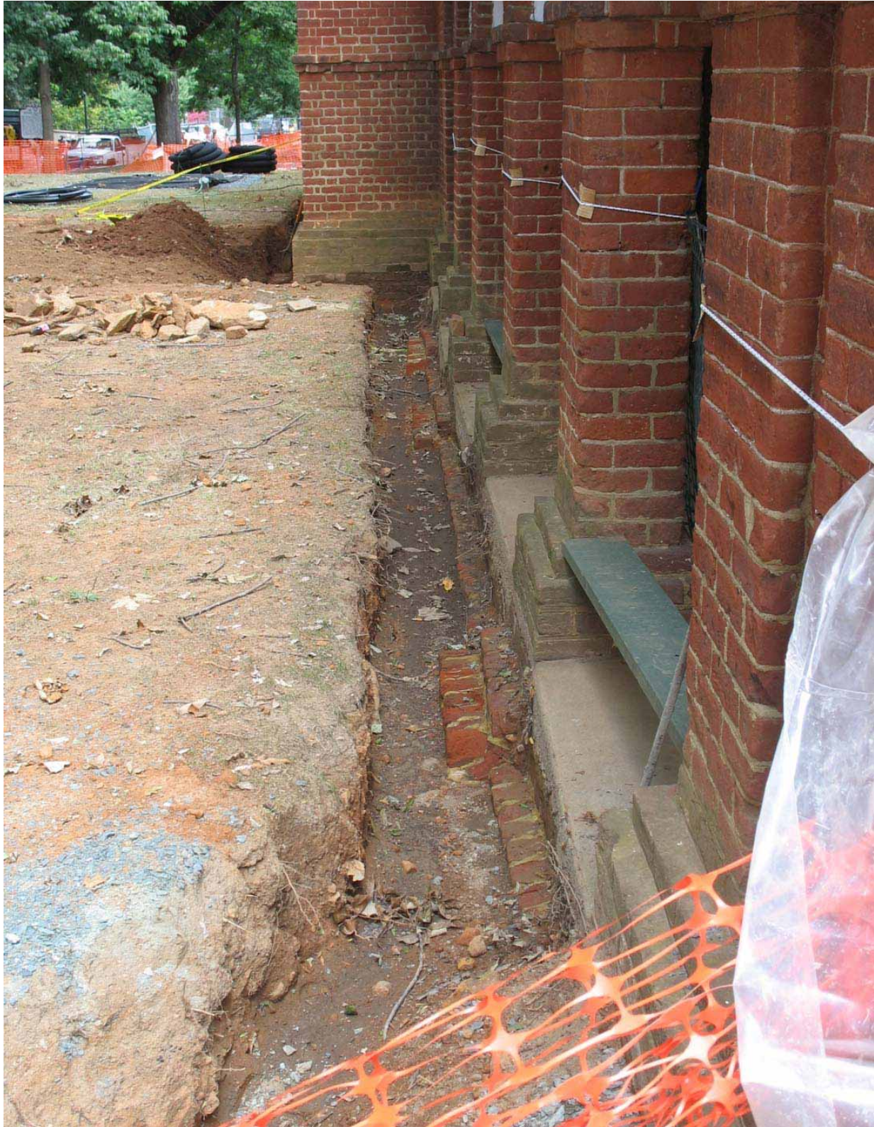
Figure 7.24 Substantial brick and concrete underpinnings, consisting of poured concrete and stepped brick ledges, were identified at numerous locations along the west façade of the West Range. (R-JAV-ARCH-RAS-2012-1-1922-C-4-Hotel_C_Underpinning.jpg)
