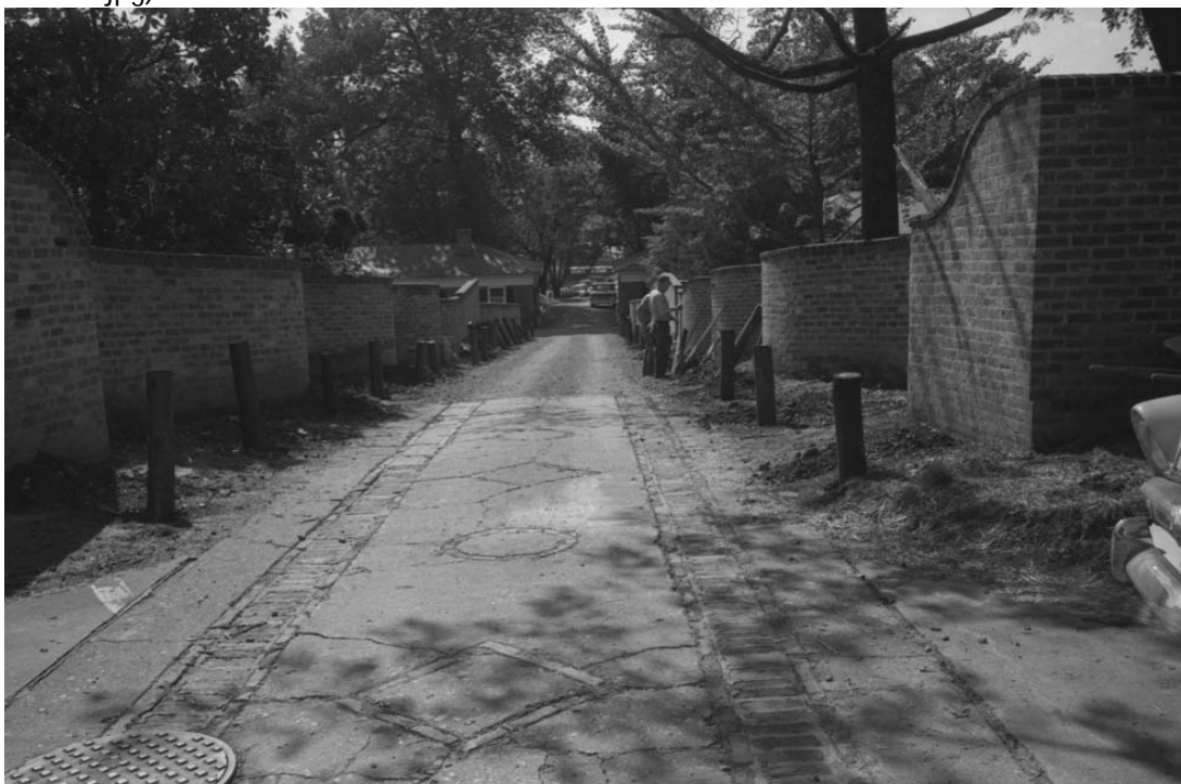
Figure 8.24 Bollards are installed to aid in protecting the single width serpentine walls from vehicle damage. (R-JAV-SCL-DSC-1962-09-Box46Env1839Neg13-BW-3-RotundaAlleyReversedNeg.jpg).
