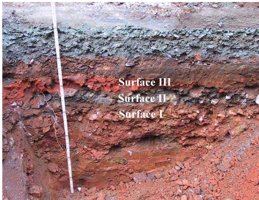
Figure 3.26 This photograph, looking at the north trench profile, shows three distinct strata of road surfacing in McGuffey Drive east of and adjacent to the Colonnade Hotel. Surface I is a quartzite cobble surfacing within a silty clay matrix; stratum 2 is a macadam surfacing with hard, angular rocks; stratum 3 is brick debris and waster material. (R-JAV-CLR-RAS-2007-1-1825-C-4-McGuffey_Alley_Road _Surfacing.jpg)
