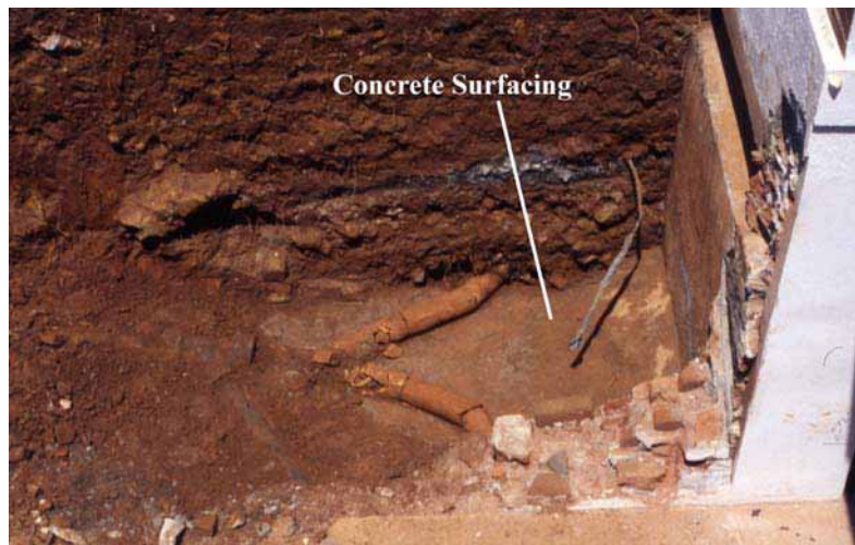
Figure 4.19 This areaway paralleling the south side of the Rotunda's eastern and western southern wings, and defined by a brick wall and pargeted cement floor, was identified archaeologically south of and adjacent to the Rotunda. Terra cotta and iron pipes were used as part of the early drainage system. (R- JAV-ARCH-RAC-2001-1-1840-C-1-Rotunda_West_Areaway_Concrete_Surface.jpg)
