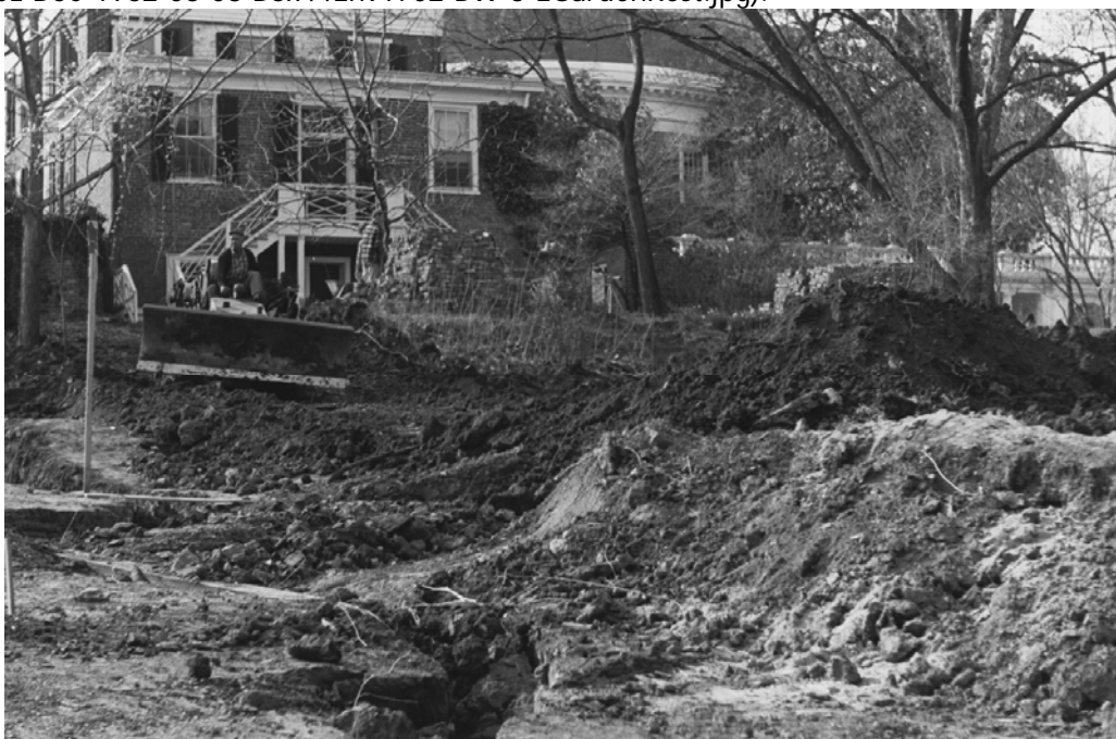
Figure 8.17 Heavy machinery used to grade the garden terraces proposed for Pavilion II is underway in this photograph. (R-JAV-SCL-DSC-1962-Box46Env1837-BW-3-PavII GardenGrading.jpg).
