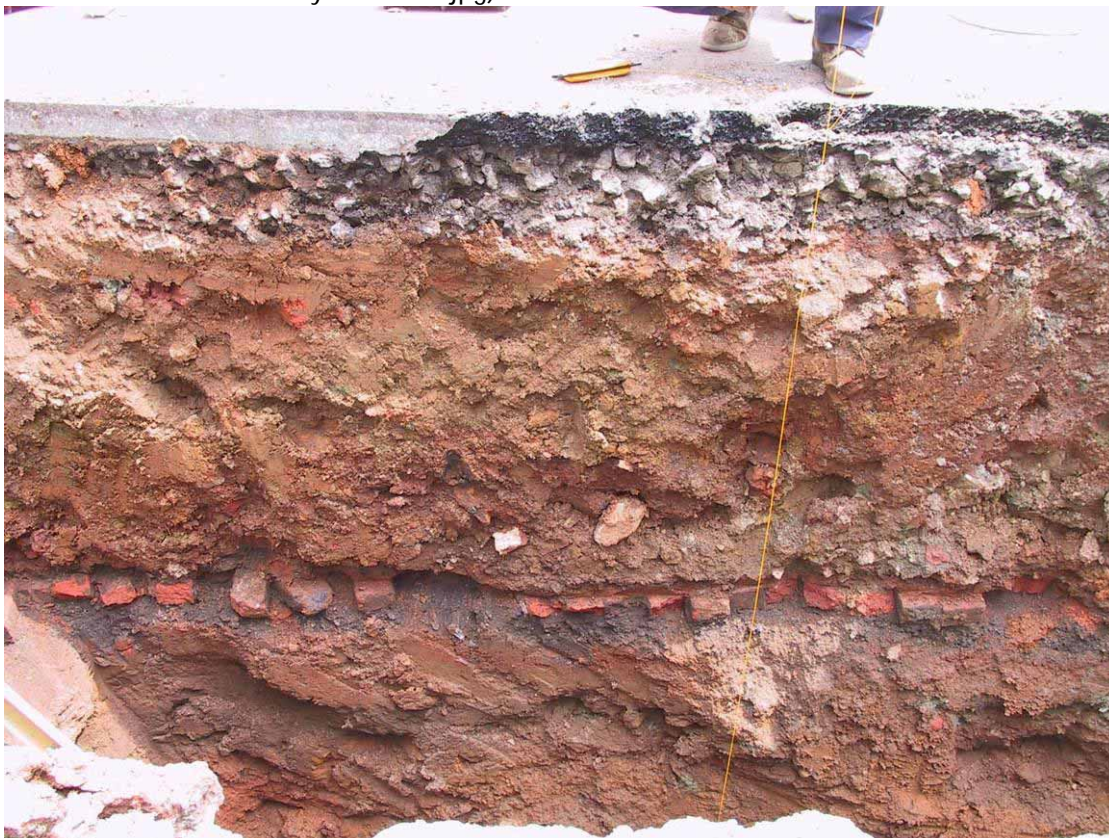
Figure 10.52 A photograph for construction monitoring documents layers of deposition over historic brick walks outside of the East Range. (R-JAV-RAS-CLR-2013-xl-C-4-PoeAlleyBrickWalk.jpg)
