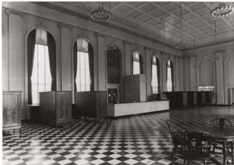
Figure 2- 20. Northeast view of Memorial Hall. Note the tall structure next to the control desk which houses the Snead book conveyor delivery system. [UVa Specail Collections]
