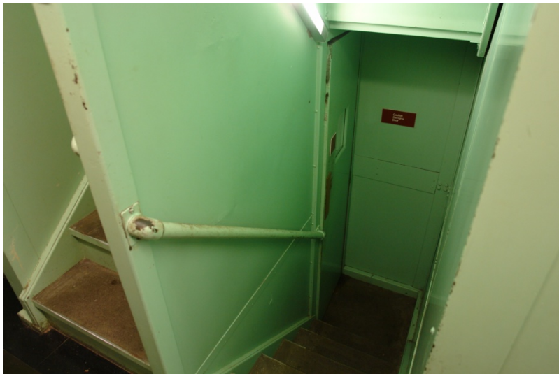
Figure 4- 113. Detail view of submarine stair in the Old Stacks. [QEA, 2014]
