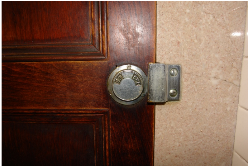
Figure 4- 104. Detail view of stall door hardware. [QEA, 2014]
