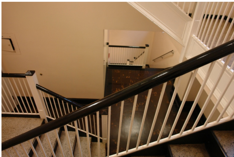
Figure 4- 109. West view of the east stairwell at the second floor landing. Note the switchback in the picture foreground that was modified outside the McGregor Room. Also note the 90 degree turn the stairwell makes between the second and first floor. [QEA, 2014]
