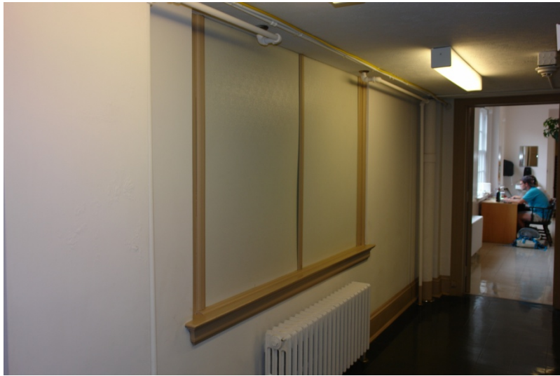
Figure 4- 52. A typical blocked window on the south wall of the Old Stacks. [QEA, 2014]
