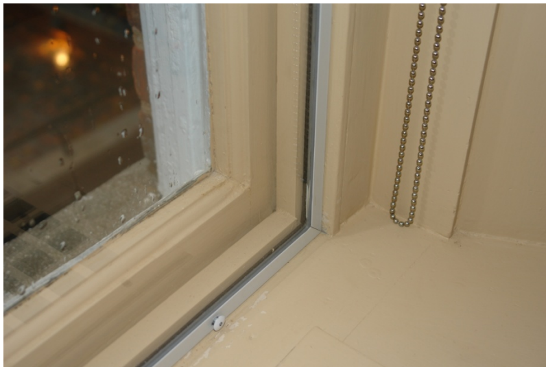
Figure 4- 28. Detail of interior storm sash installed at the windows. [QEA, 2014]
