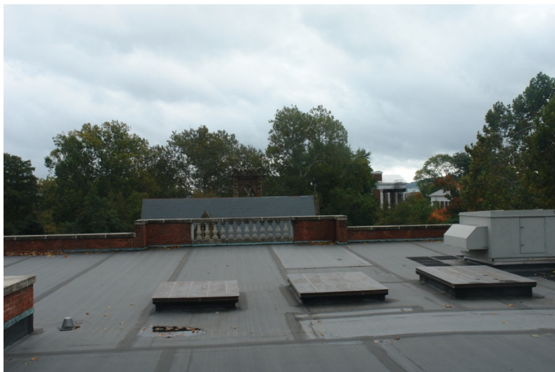
Figure 4- 13: East view of the east wing roof. Note the three skylights that have been concealed. [QEA, 2014]
