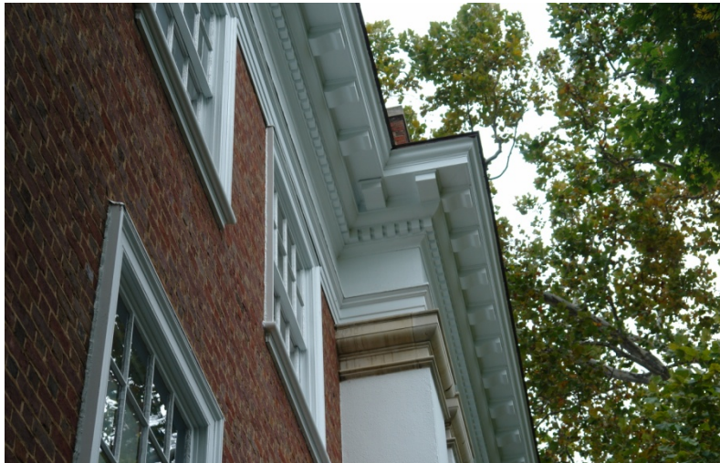
Figure 4- 6: Detail view of the engaged pilaster and cornice. [QEA, 2014]
