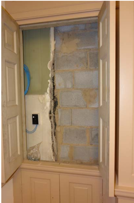
Figure 4- 49. Detail of north wall beyond Mount Vernon Room finishes. Note the concrete masonry units installed in the former window opening. [QEA, 2014]
