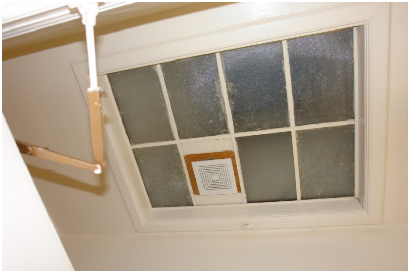
Figure 4- 106. Detail view of the laylight in Room 569A-Womens Restroom. [QEA, 2014]
