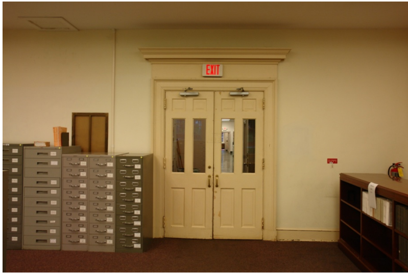
Figure 4- 62. Detail of doors and casing on the west wall leading into the corridor. Note the brass case installed in the wall to the left of the door. [QEA, 2014]
