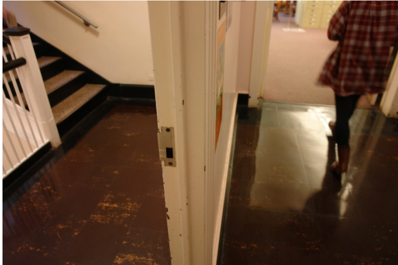
Figure 4- 108. East view of the east stairwell and corridor at the third floor. Note how the black border extends from the landing into the corridor. It was not modified when the fire-rated partition was added. [QEA, 2014]
