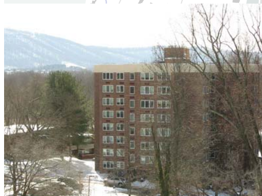
Bice House provides undergraduate housing in close proximity to the Health System
