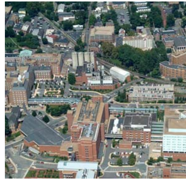
Lee Street existing conditions
