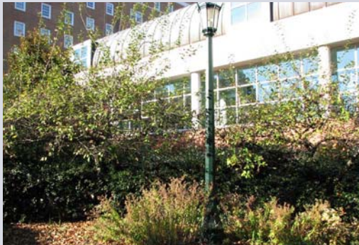
E: An example of a well screened section of the hospital link
