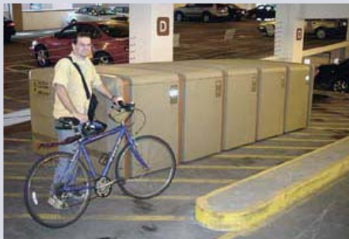
I1: Example of a bike locker system installed in a parking garage
