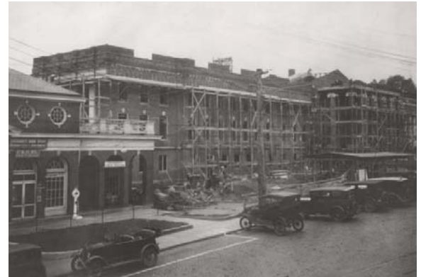
Medical School portico under construction, ca. 1928
